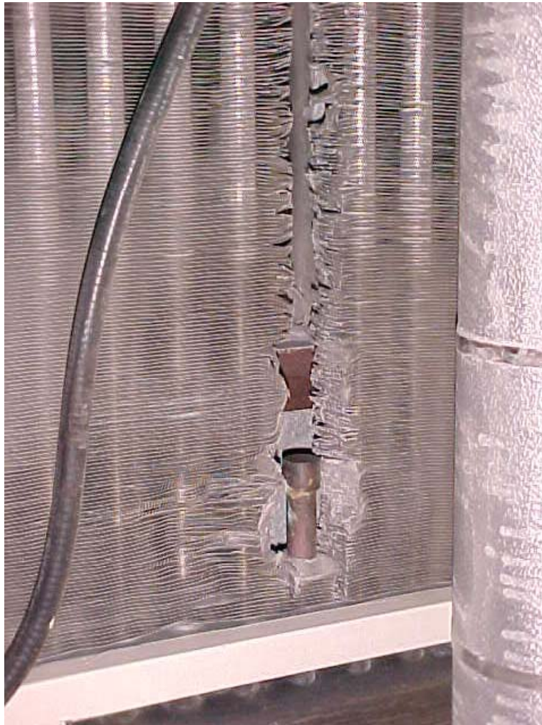
Steam coil with one ruptured tube removed and its connection capped
