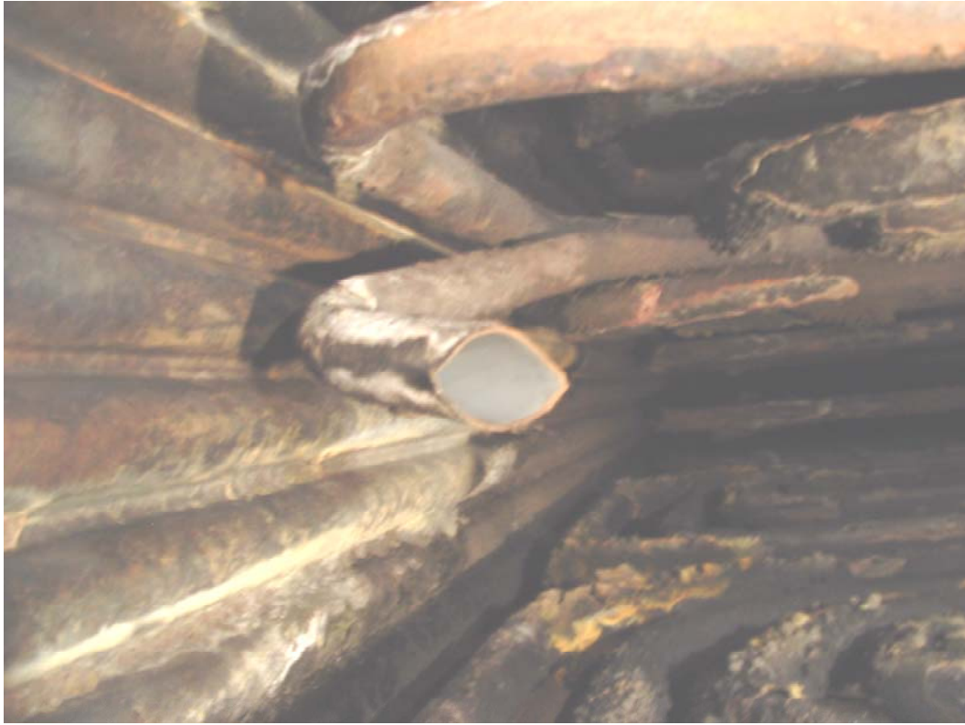
Failed superheater tube 2005-02-05
