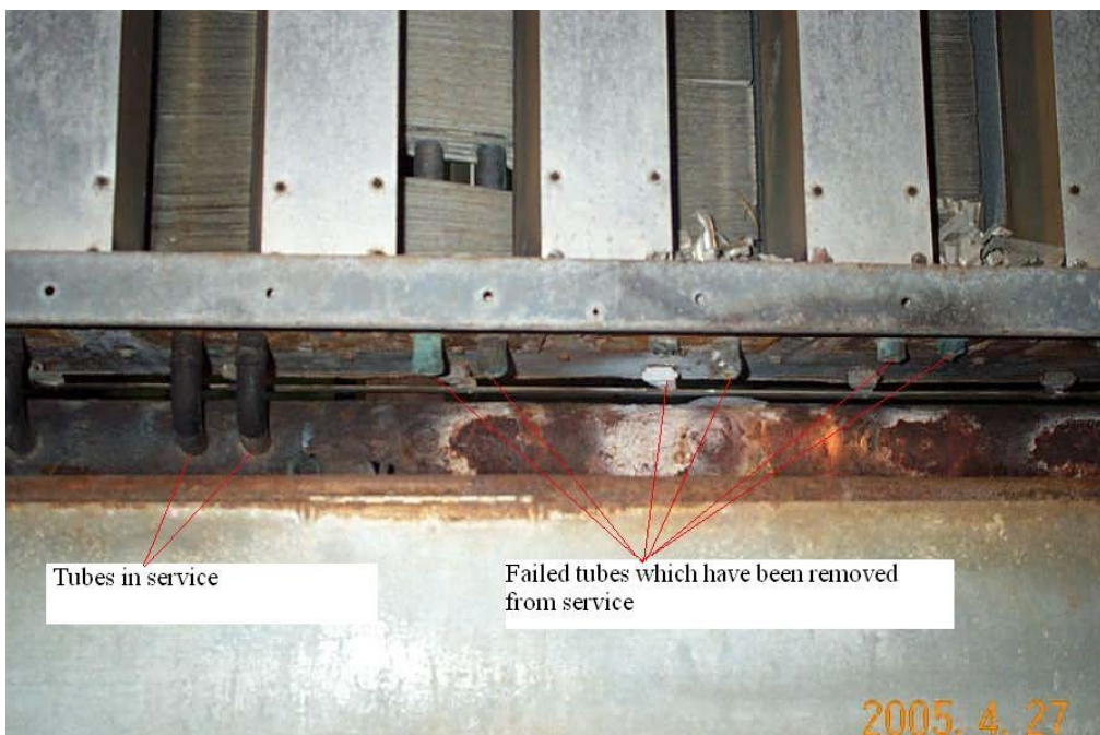
Steam coil section with failed tubes
