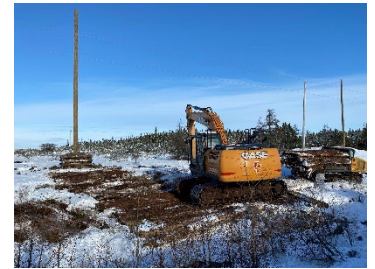
Installation of bog mat for transmission line 55L.
