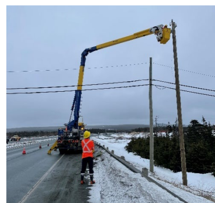
Work on distribution feeder OXP-01 in St. John’s
