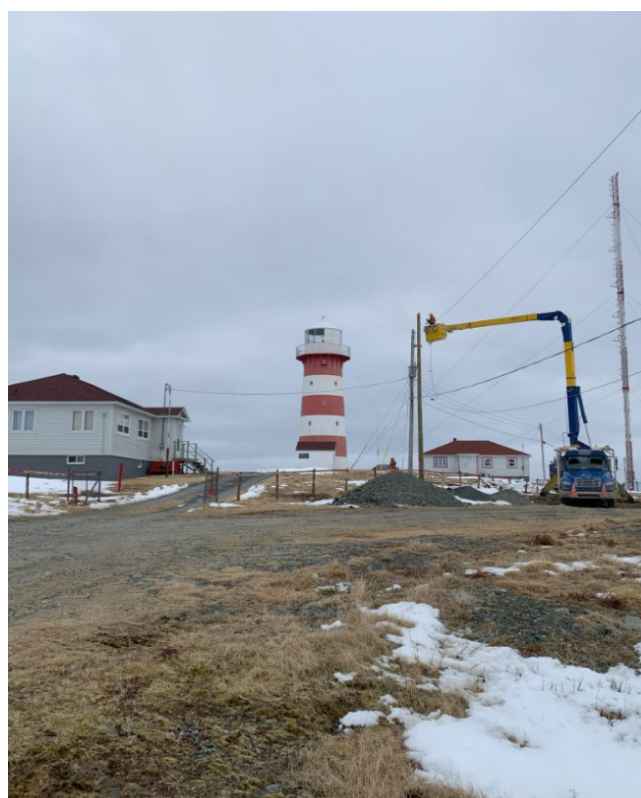
Crews repairing distribution line in Cape Pine after winter storm.
