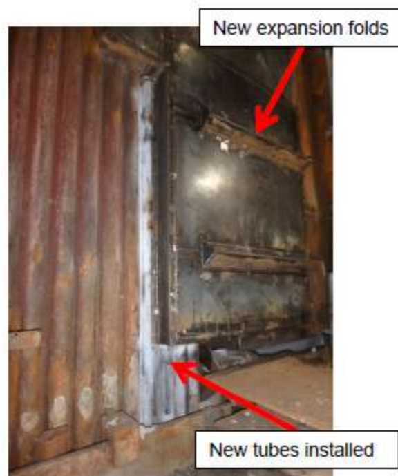
Figure 3: New Expansion Folds in the Windbox
