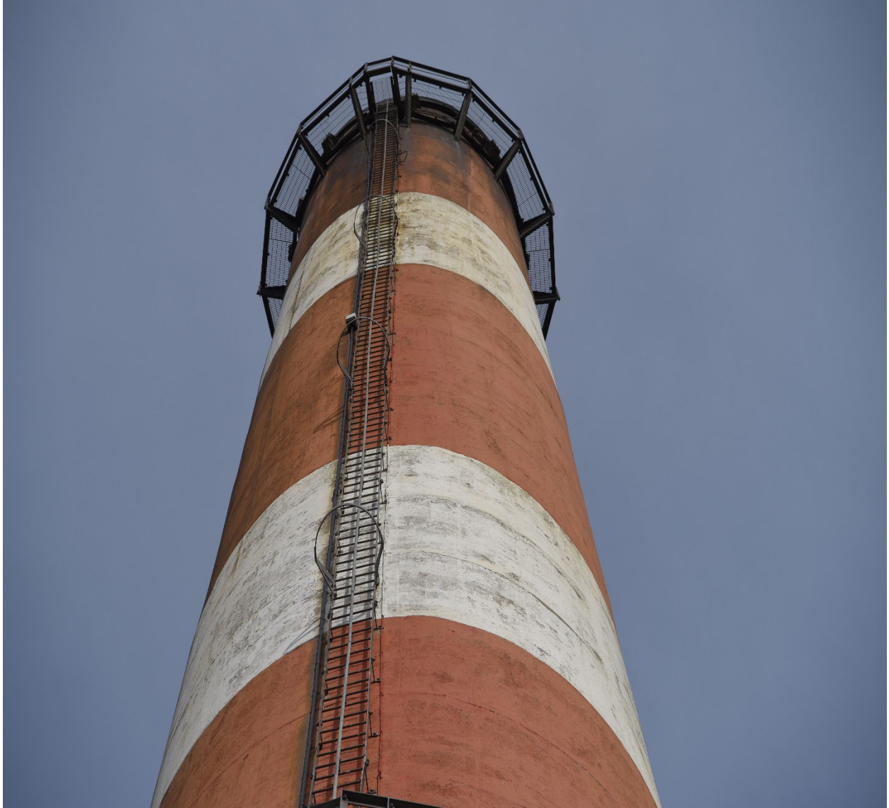
Exhaust Stack No. 2 View Looking Upward from the West Side
