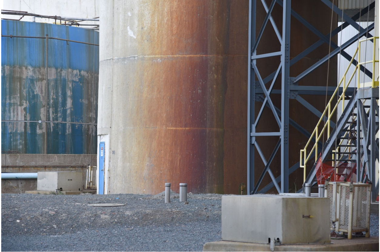
Base of Exhaust Stack No.2
