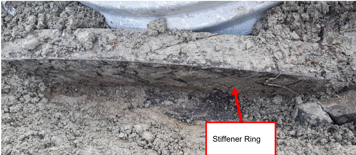
Figure 3-3: Excavated Stiffener Ring – Penstock No. 2
