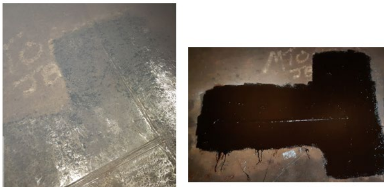
Figure 3-4: Coating Prep (Left) Final MC Tar (Right) – Penstock No. 2
