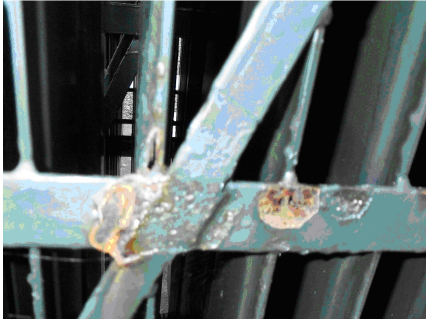
Deteriorated radiator fin edges – Blaketown Substation
