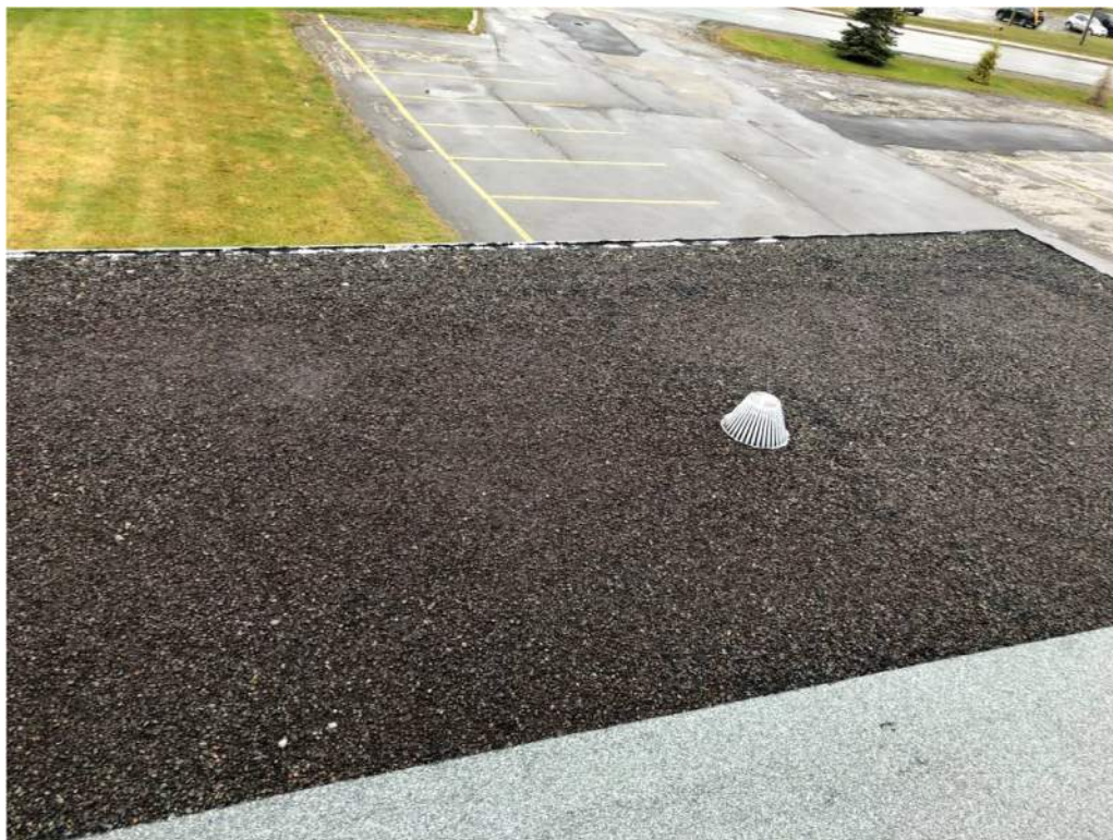
PHOTO 2: ROOF #4 BUILT-UP ROOF.
