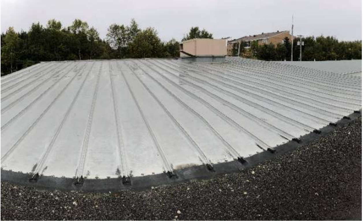
PHOTO 3: ROOF #2 - PITCHED STANDING SEAM METAL ROOF.
