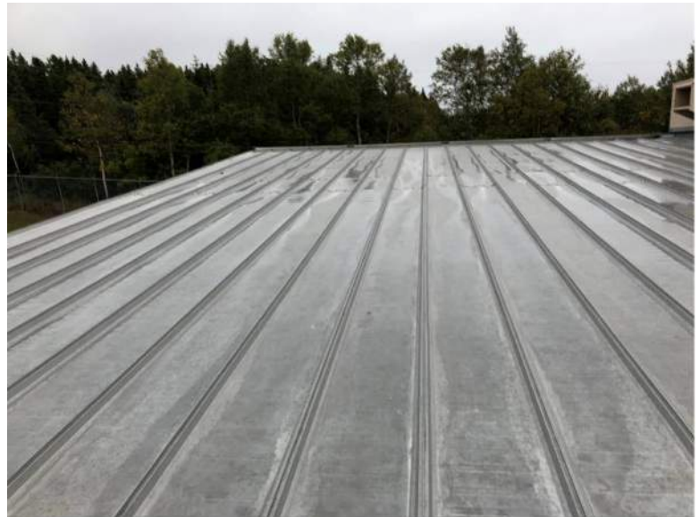
PHOTO 14: NORTH SIDE OF THE PITCHED STANDING SEAM ROOF.
