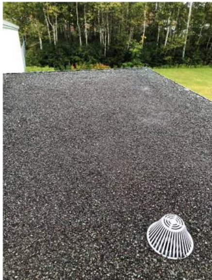
PHOTO 7: VESTIBULE BUILT-UP ROOF WITH ROOF DRAIN.
