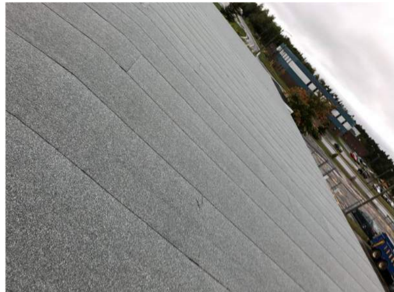
PHOTO 12: CAPP SHEET OF SINGLE-PLY MODIFIED BITUMEN ROOF.
