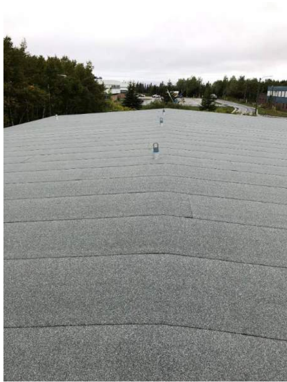
PHOTO 1: ROOF #1 SINGLE-PLY MODIFIED BITUMEN GABLE ROOF WITH ROOF ANCHORS
