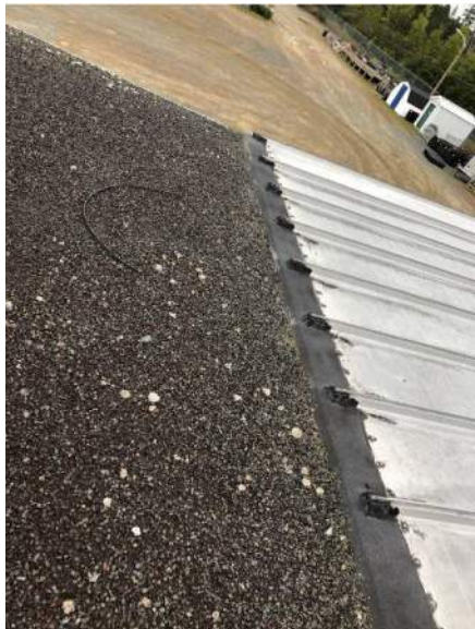
PHOTO 19: ROOF TRANSITION BETWEEN STORAGE METAL ROOF AND STAGGING AREA BUILT-UP ROOF.
