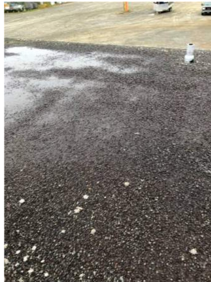
PHOTO 20: EAST END OF THE STAGGING AREA BUILT-UP ROOF WITH VENT.
