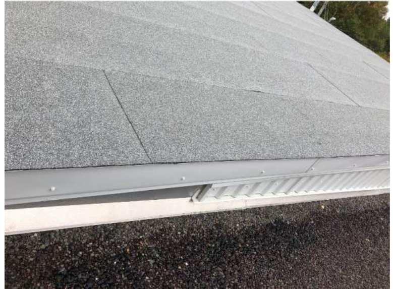
PHOTO 10: TRANSITION WALL AT VESTIBULE ROOF AND MAIN OFFICE BUILDING ROOF.
