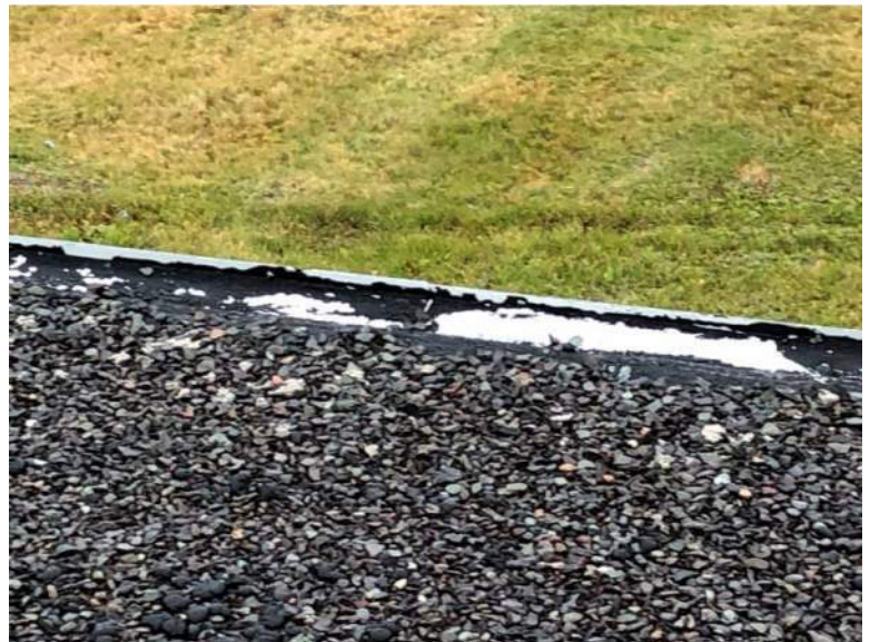
PHOTO 8: VESTIBULE ROOF EDGE AT THE METAL FLASHING/FASCIA.
