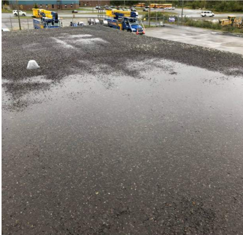
PHOTO 4: ROOF #3 BUILT-UP ROOF.
