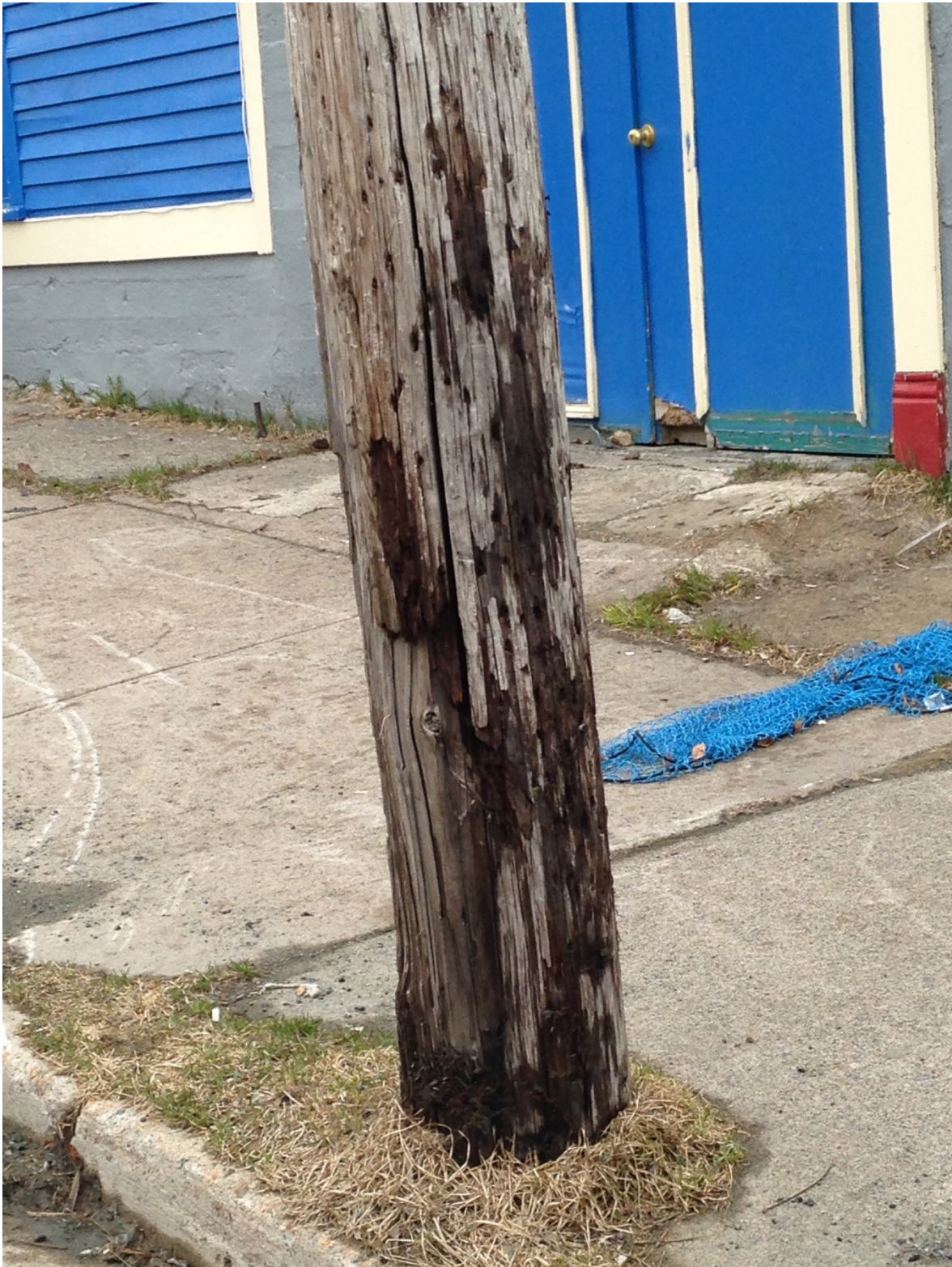
Figure 6 - Deteriorated Pole
