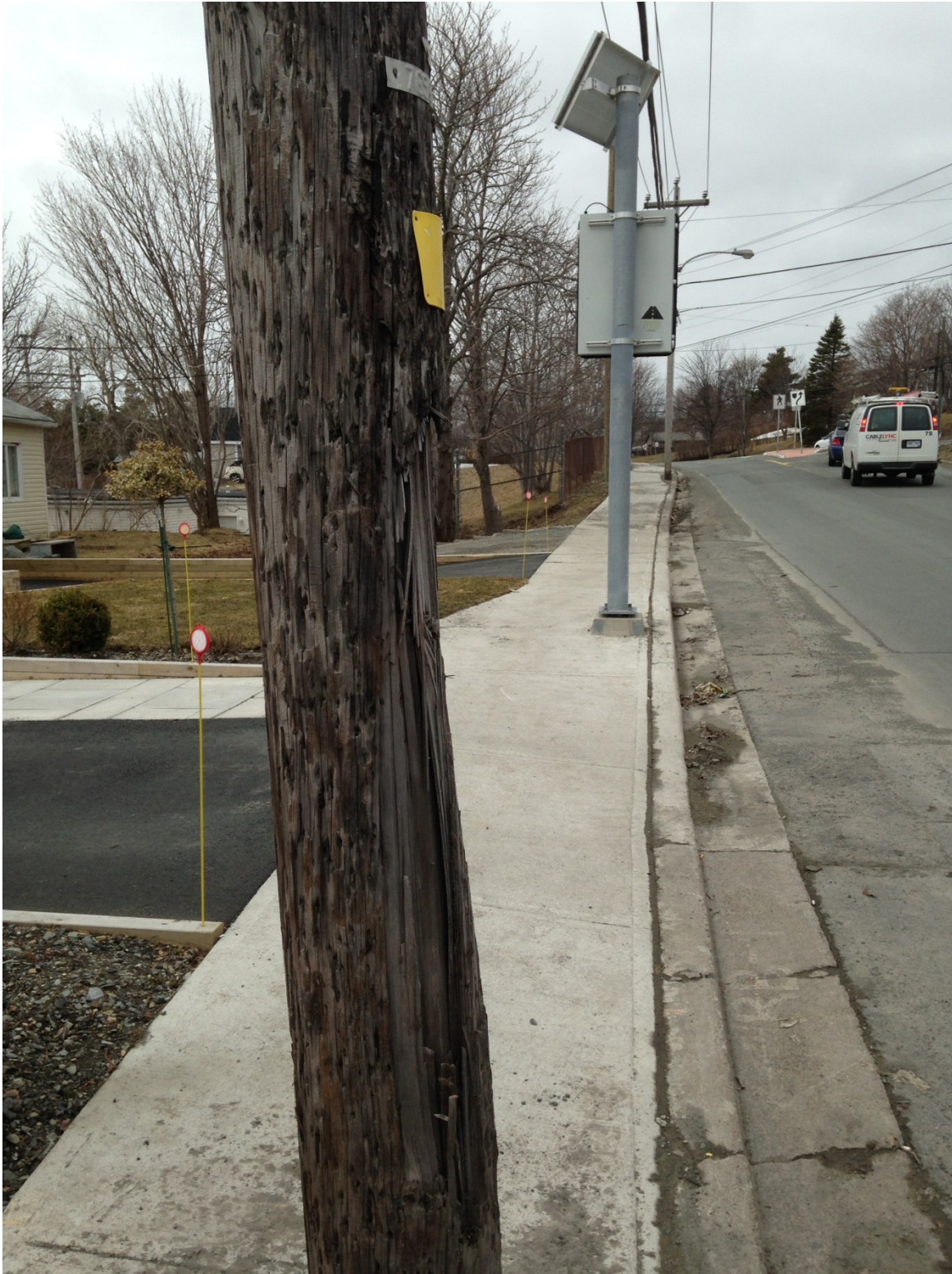
Figure 1 – MOL-09 Pole Damage
