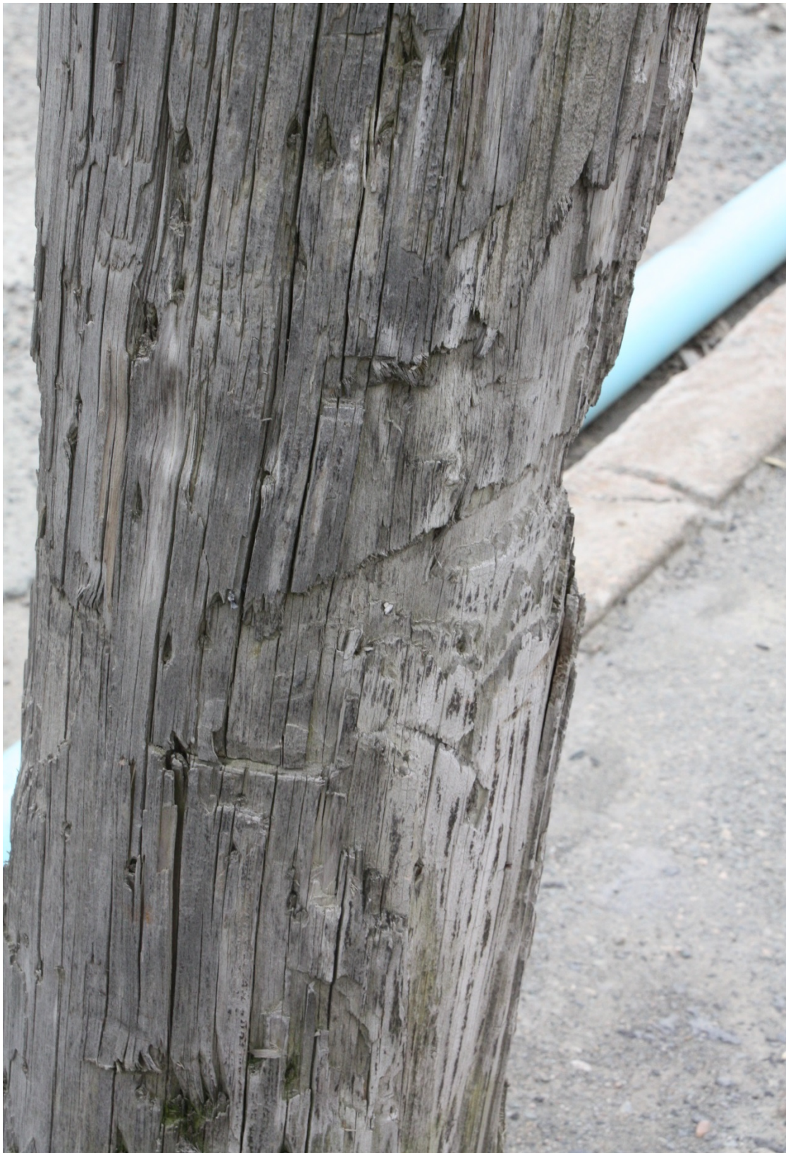
Figure 6 – Pole Damage near Base
