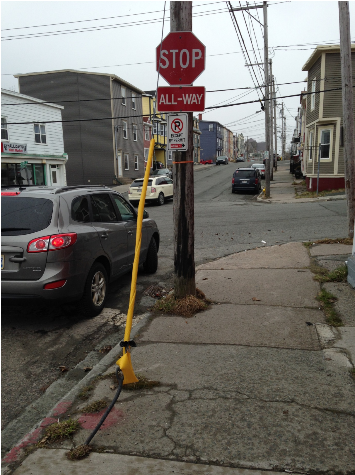
Figure 5 - Guy Bent Towards Sidewalk
