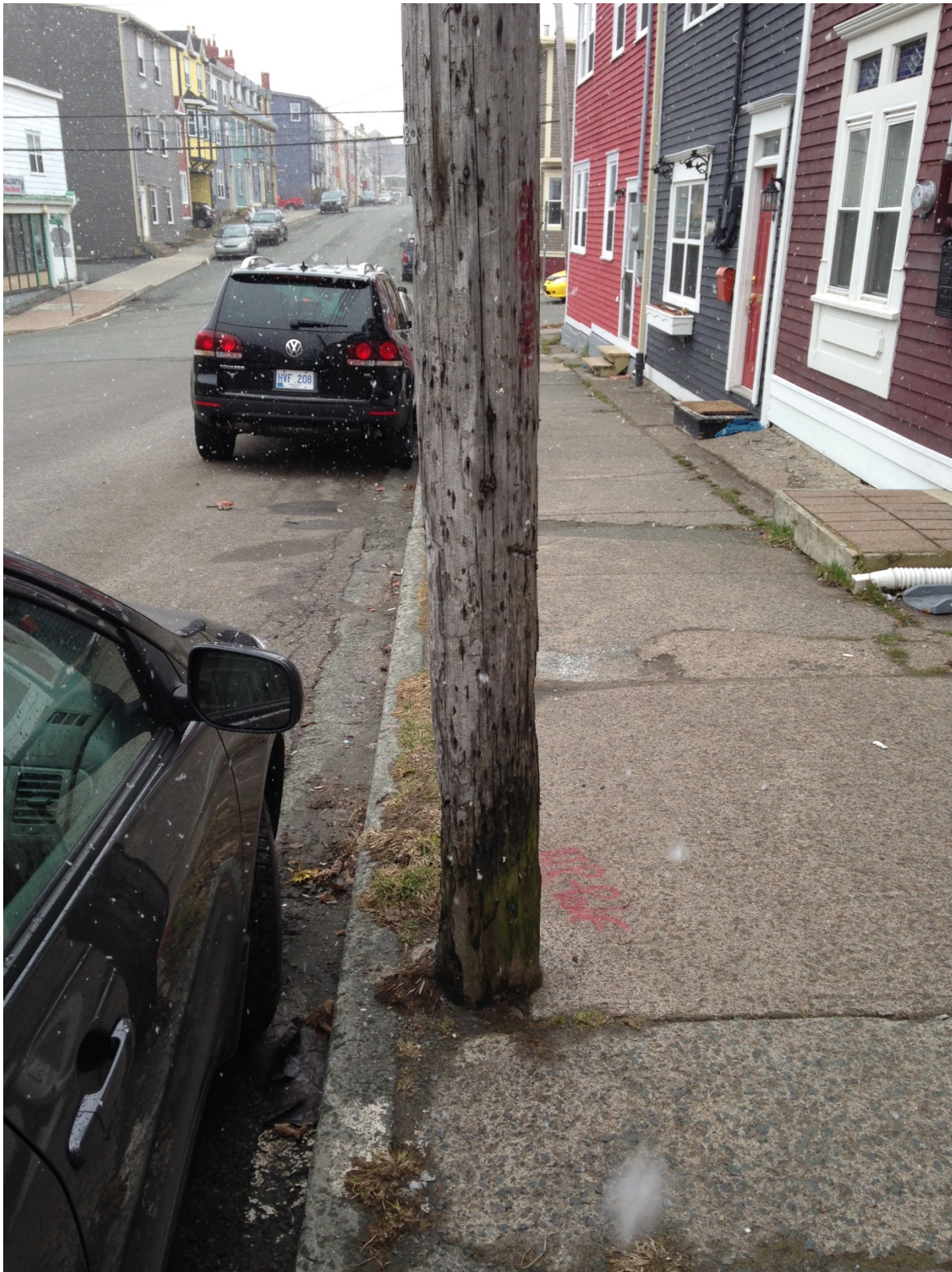
Figure 4 - Loss of Pole Diameter at Base
