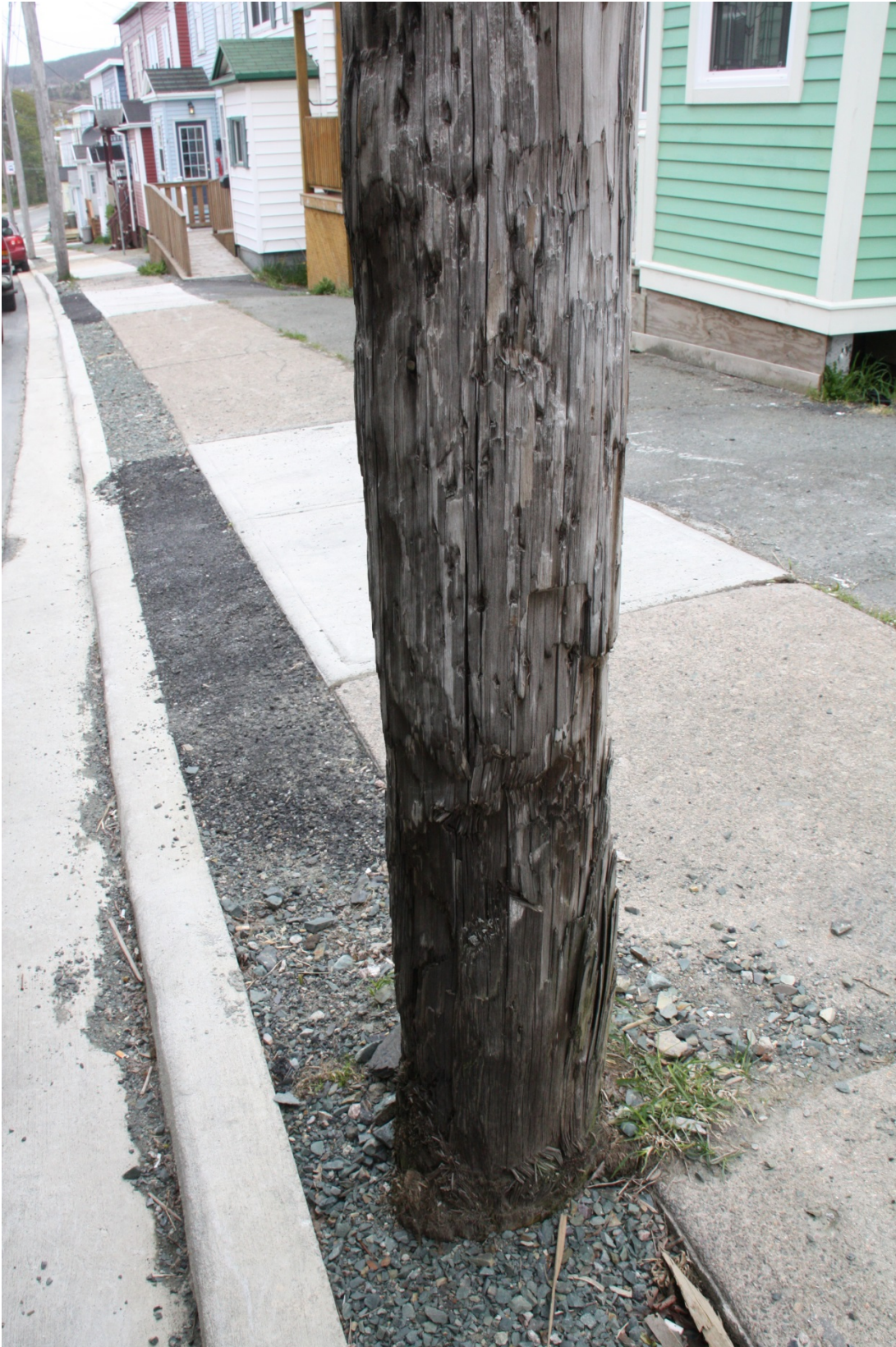
Figure 5 – Pole Damaged by Vehicles
