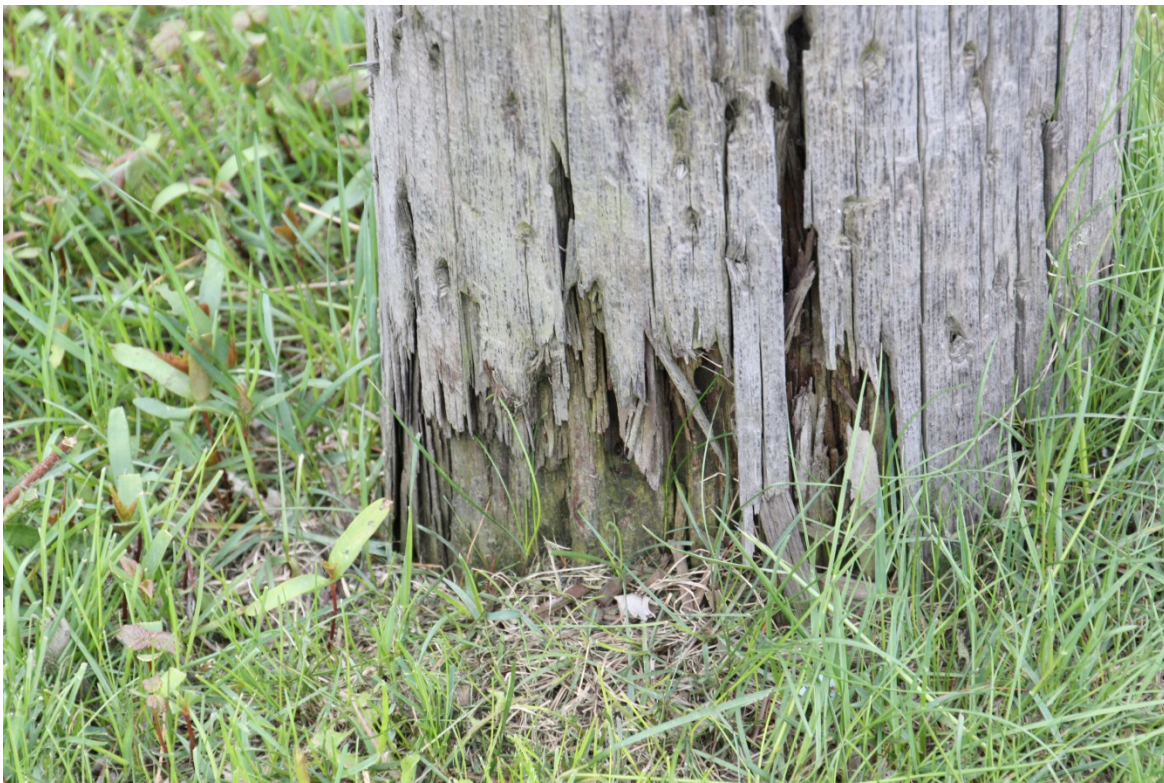
Figure 7 – Pole Deteriorated at ground line
