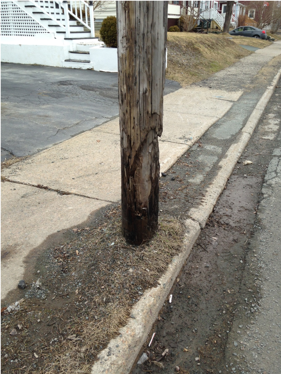
Figure 2 - Pole Damage at Base
