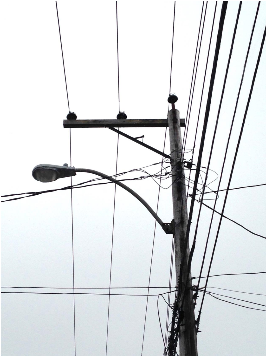
Figure 1 - KBR-10 Pole with Alley Arm Type Crossarm
