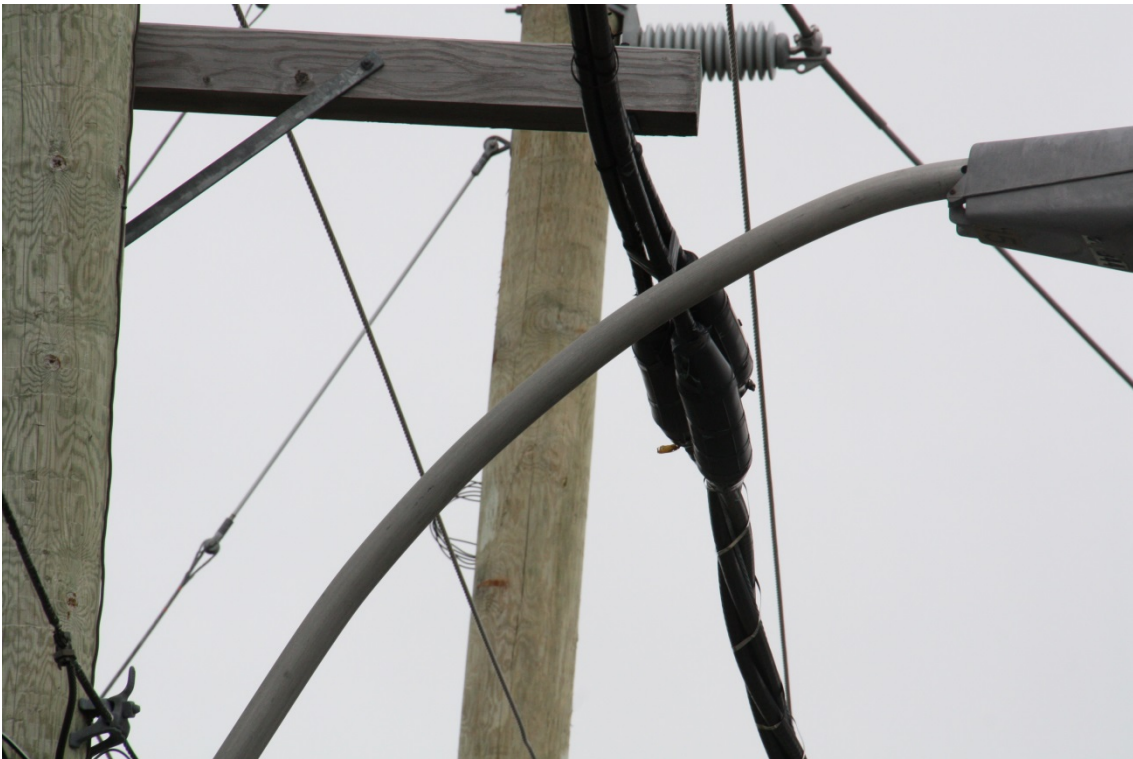
Figure 7 – Aerial Cable Splice
