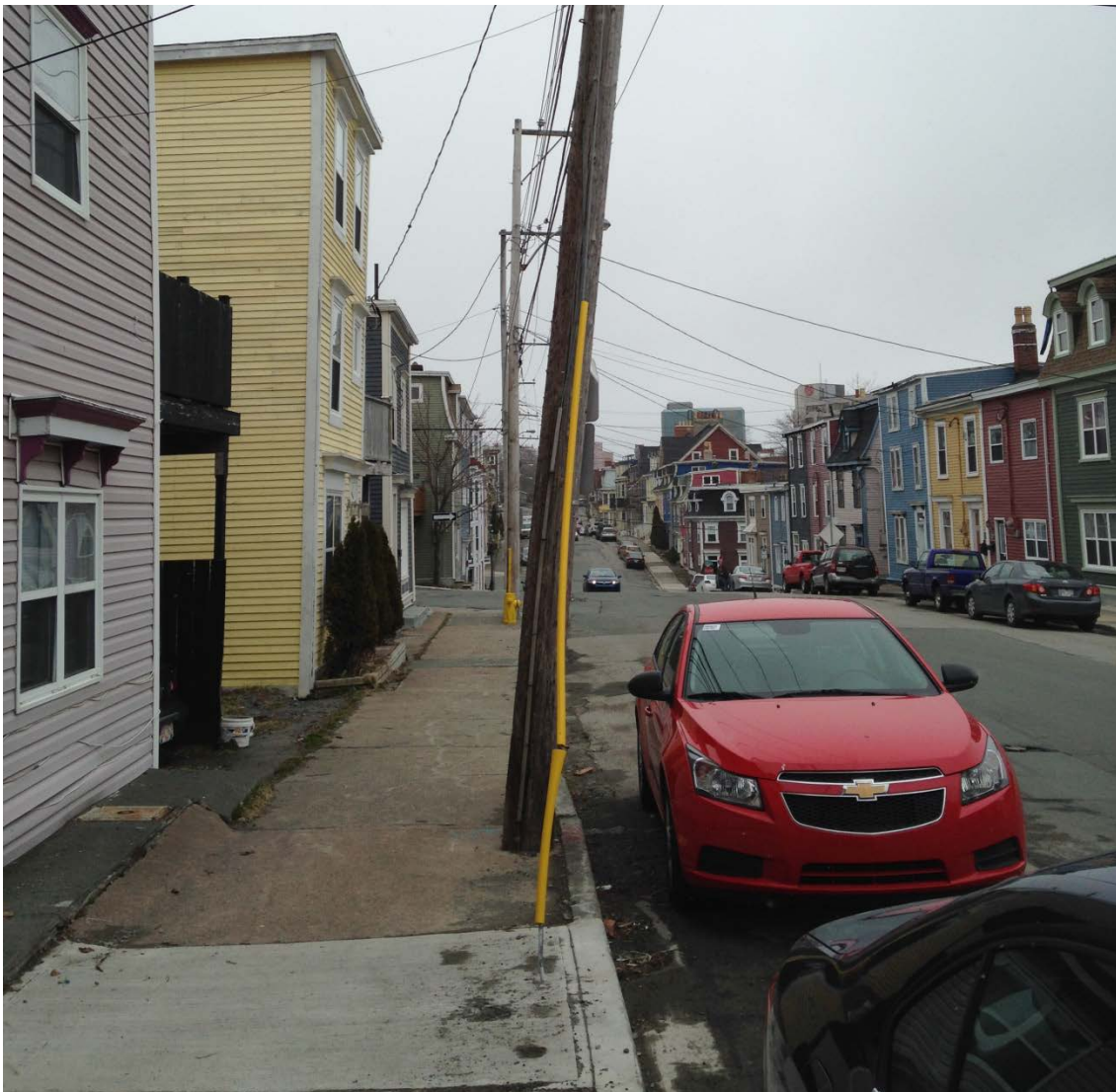
Figure 3 - Pole Leaning Towards Traffic
