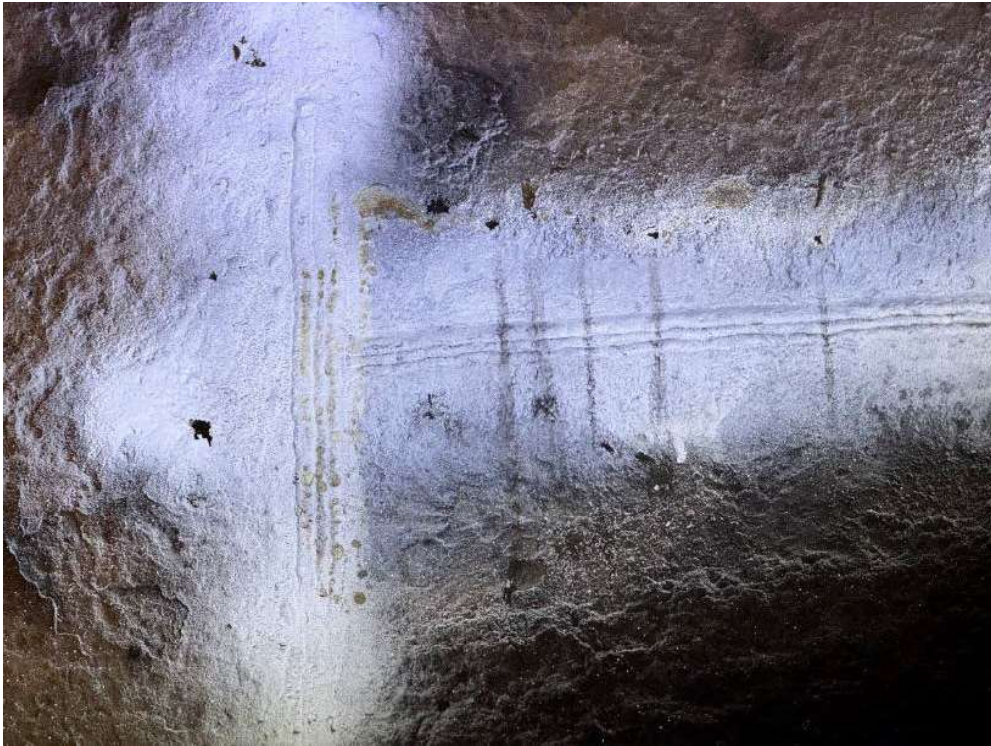
Photo 13 Close-up of circumferential and longitudinal weld tested at Can 7N
