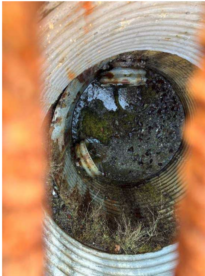
Photo 35 Condition of observation well downstream and to left of surge tank
