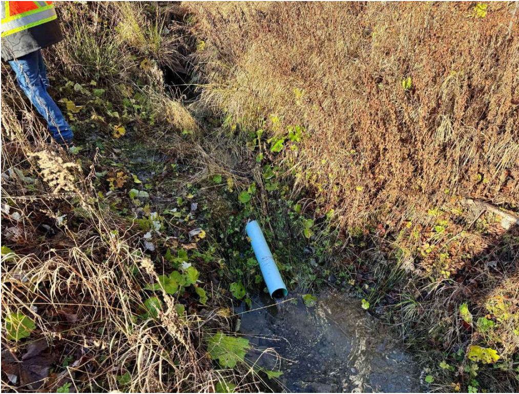
Photo 33 Flow through drainage pipe at STA. 0+903
