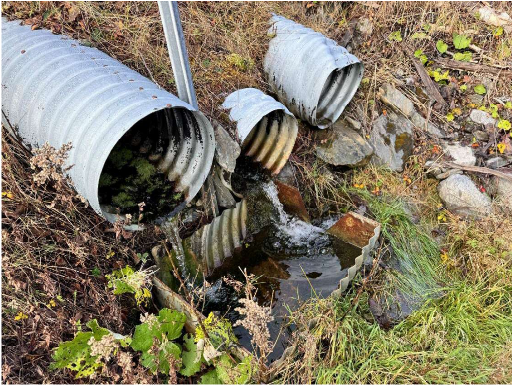
Photo 37 Condition of culverts at N-2 Weir
