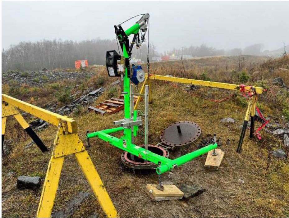
Photo 1 TRR's Access Setup at Manhole 2
