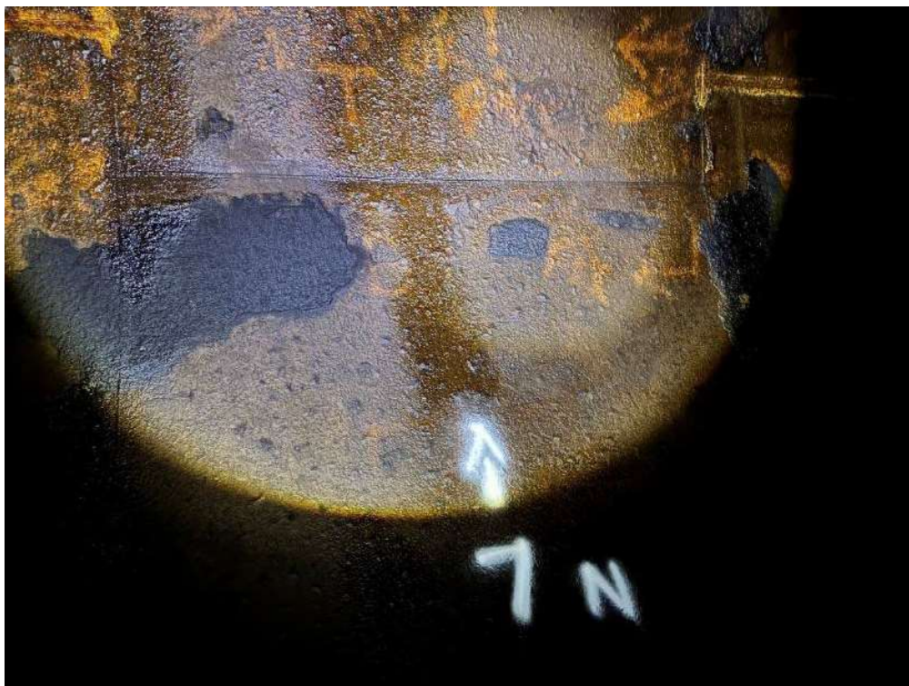
Photo 10 Weld 7N prior to being cleaned and tested
