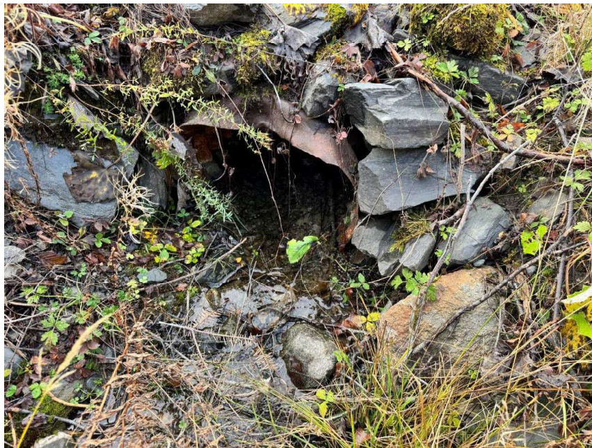
Photo 36 Condition of culvert directly upstream of bridge crossing
