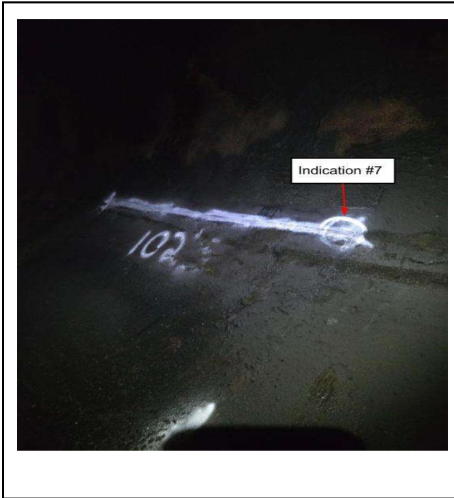
Figure 12. Can 102 South - Indication Noted
