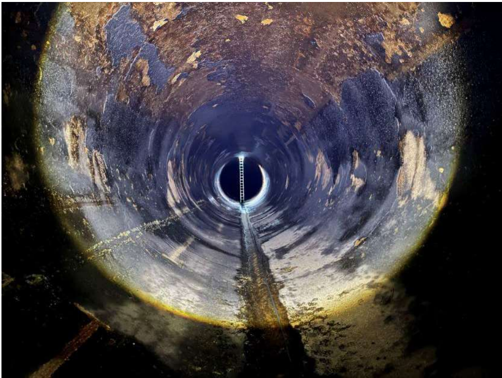
Photo 8 Interior surface condition of penstock by Manhole 3
