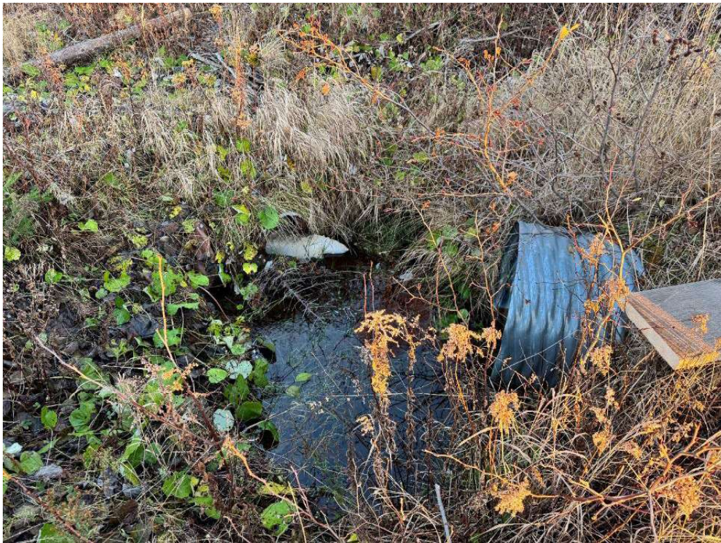
Photo 32 Condition of culvert with water flow to weir at N-1
