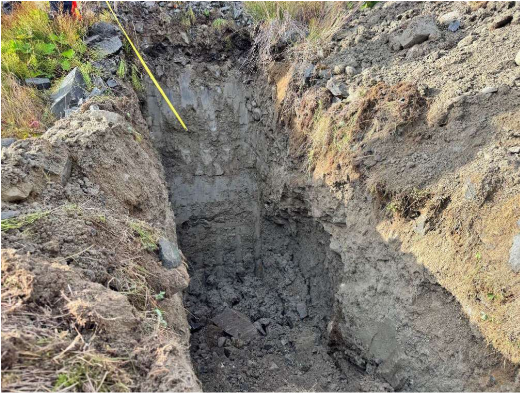
Photo 43 Test pit conducted at exterior of P3 (Sept 23 rd 2025)
