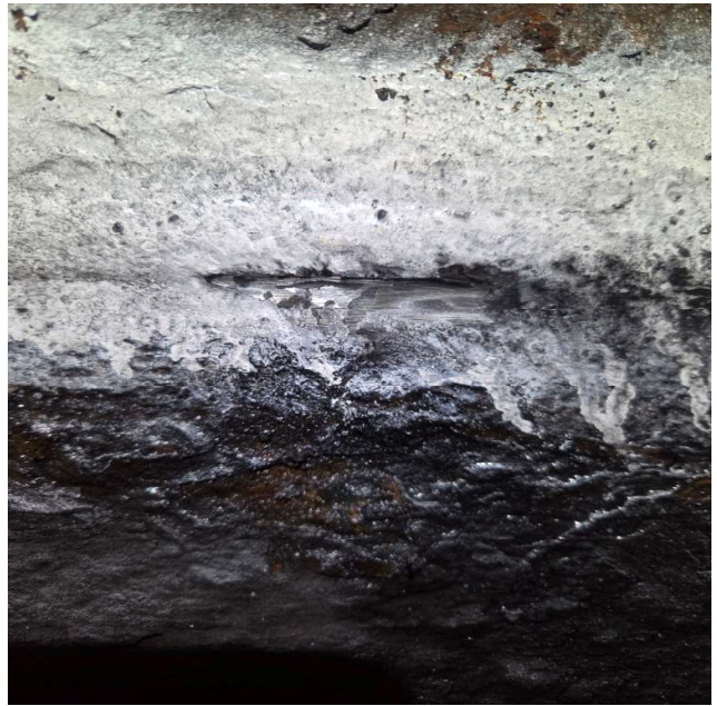
Figure 24. Can 353 North - Post Grinding
