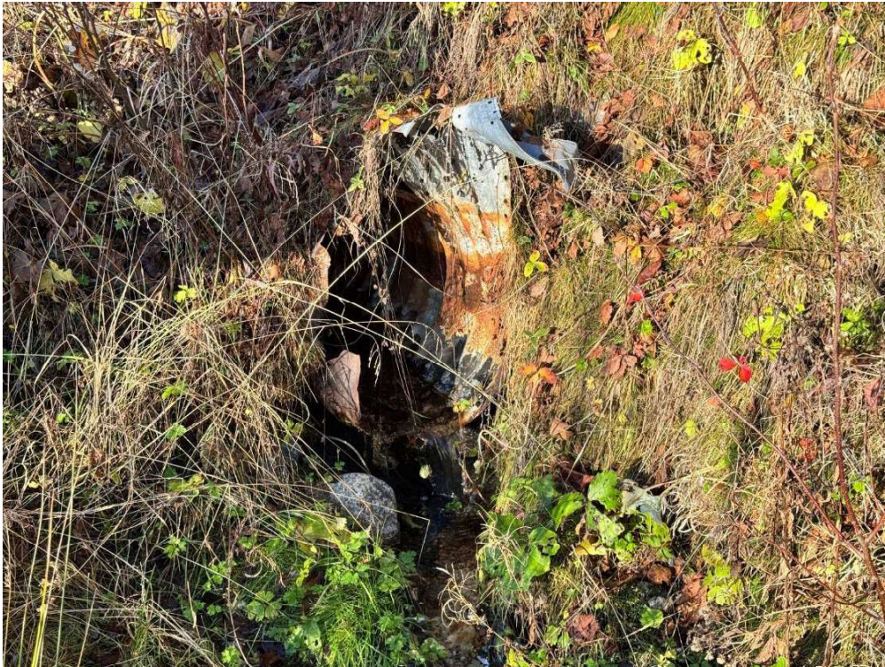
Photo 34 Condition of culvert at STA. 0+722
