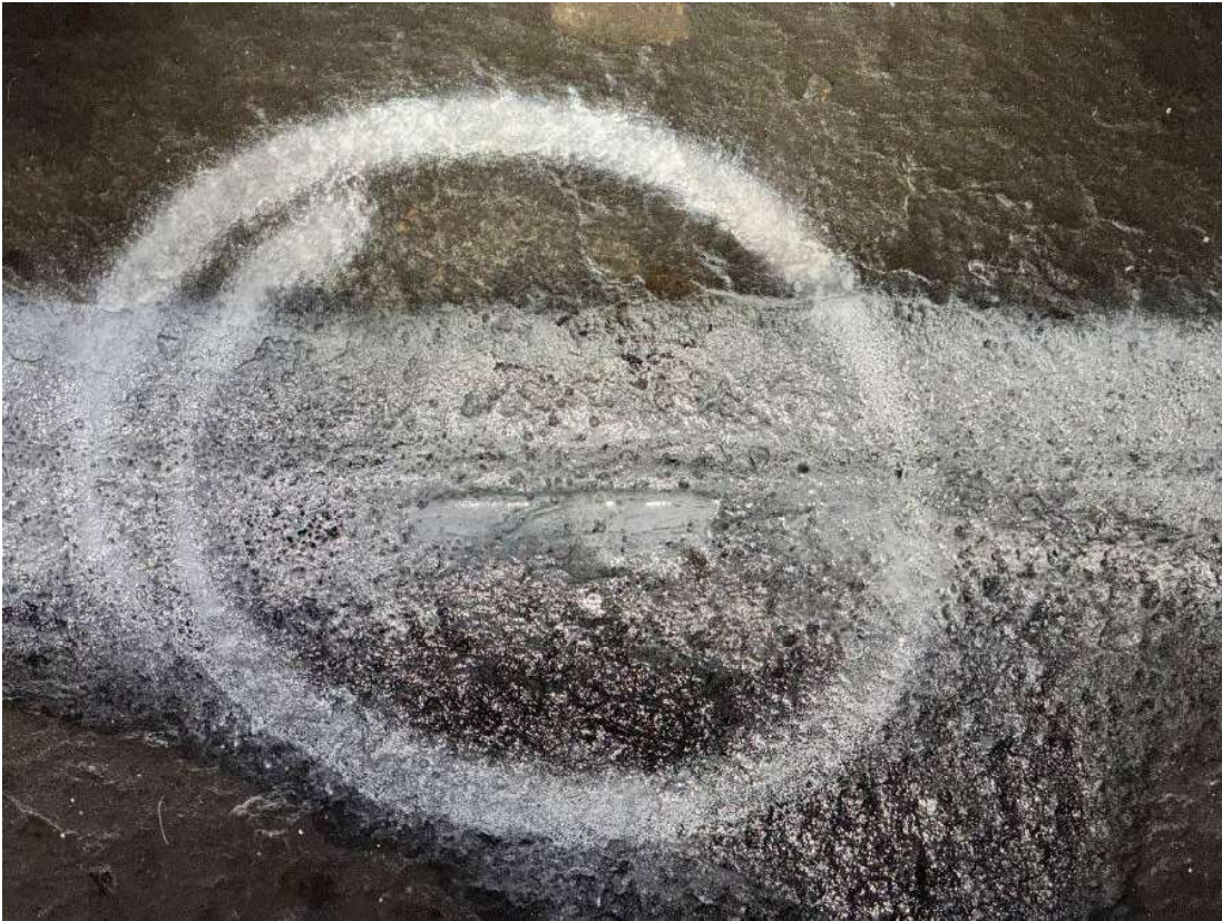
Photo 21 Close-up of weld indication at Can 254N
