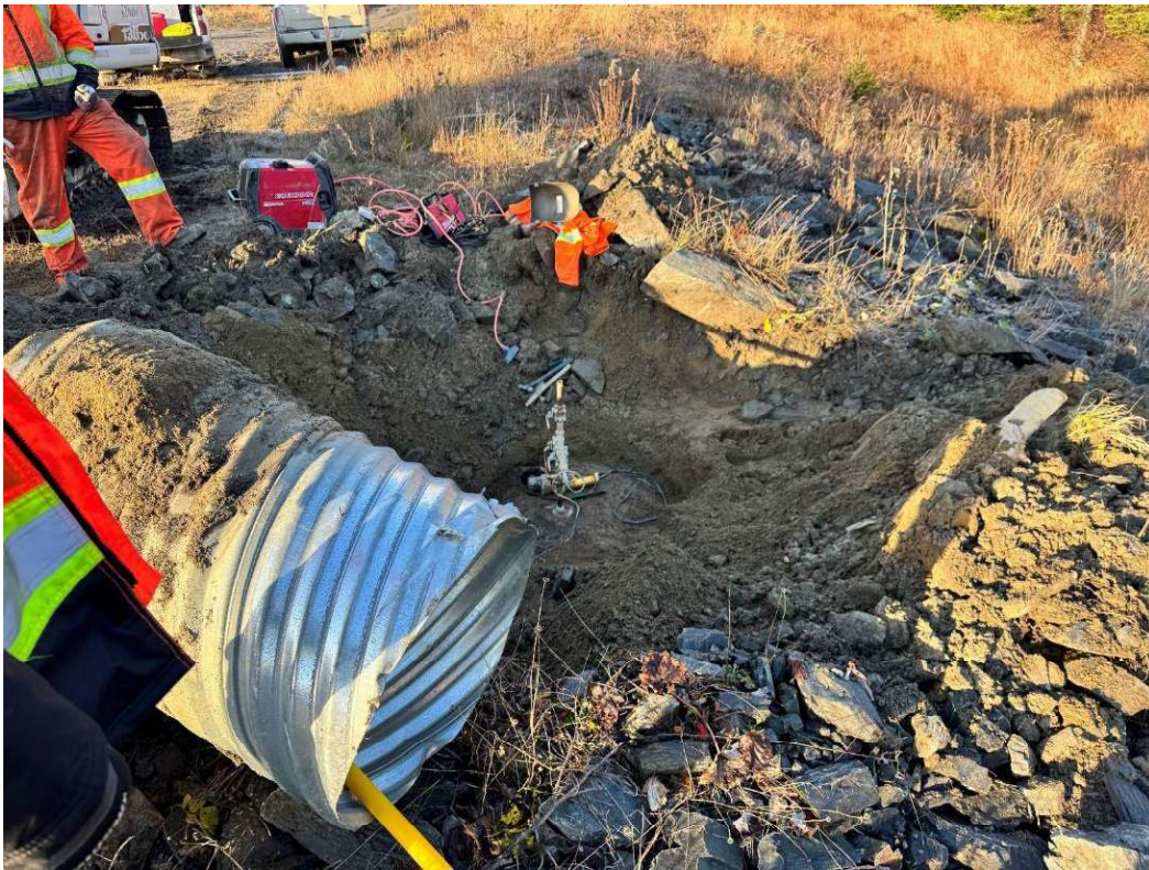
Photo 45 Work conducted by NLH crew along exterior of penstock during inspection
