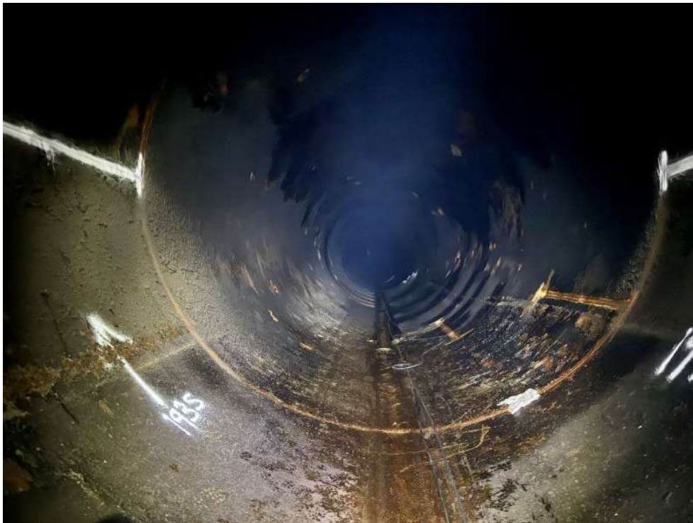
Photo 9 Interior surface condition of penstock by Can 193
