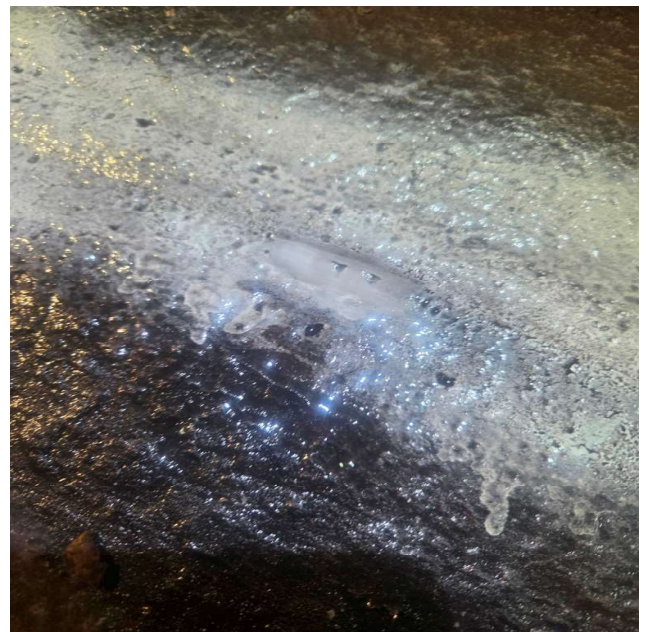
Figure 19. Can 303 North - Post Grinding - Indication Removed
