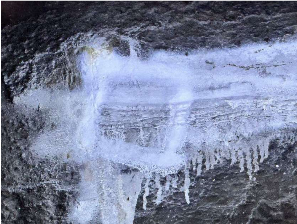
Photo 15 Close-up of weld indication at Can 17S
