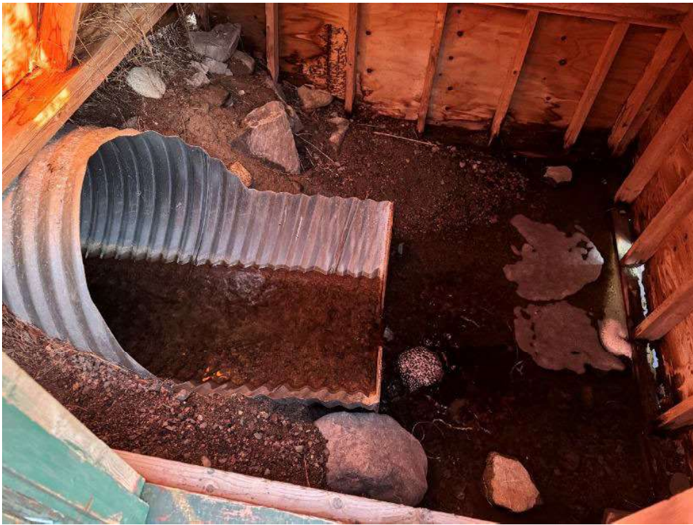
Photo 31 Condition of monitoring weir at N-1
