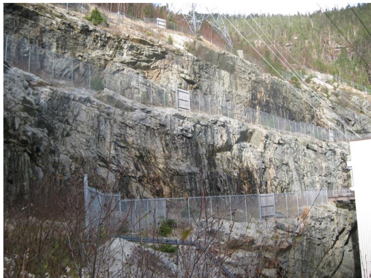
Figure 1: Chain-Link Fencing on Each Benched Section of Powerhouse Slope
