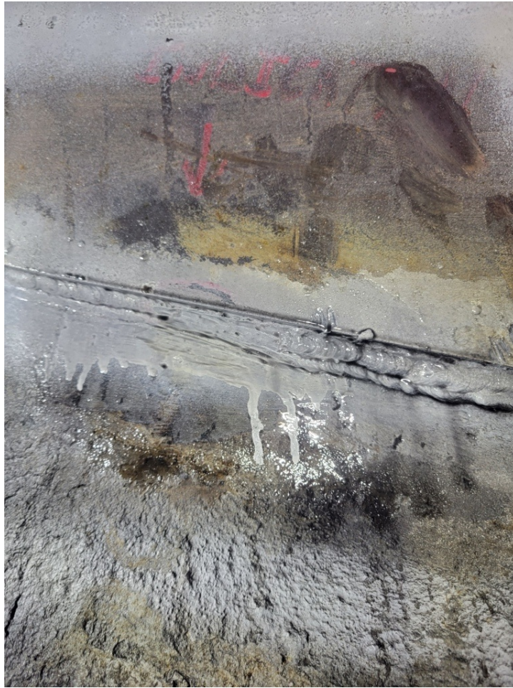
Figure 7. Can 146N - Indication Removed With Grinding - No Welding Needed
