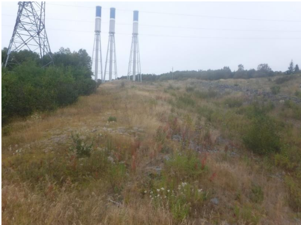
PHOTO 30 LOOKING UPSTREAM TOWARD SURGE TANKS FROM TRANSMISSION LINE
