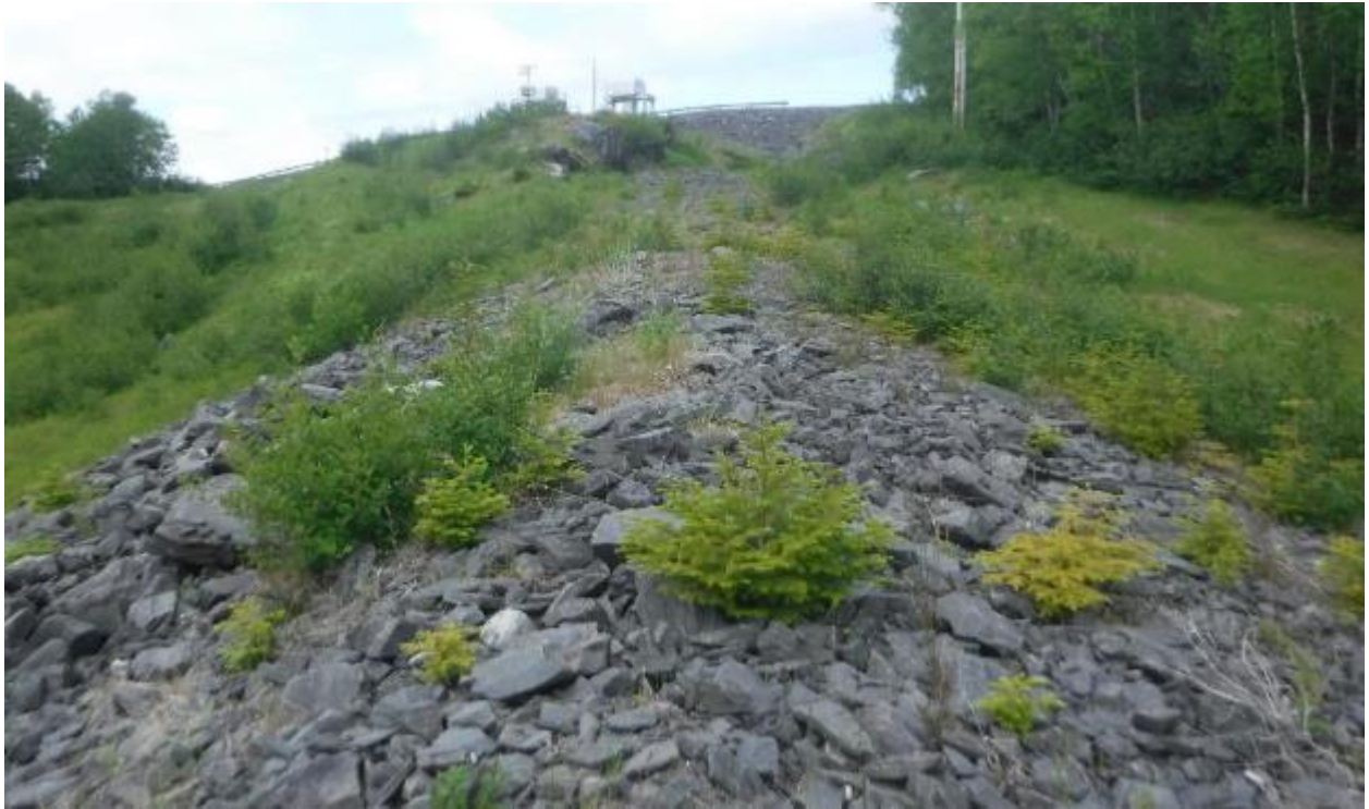
Photo 45 Typical Penstock 2 cover conditions. Looking upstream at Intake.
