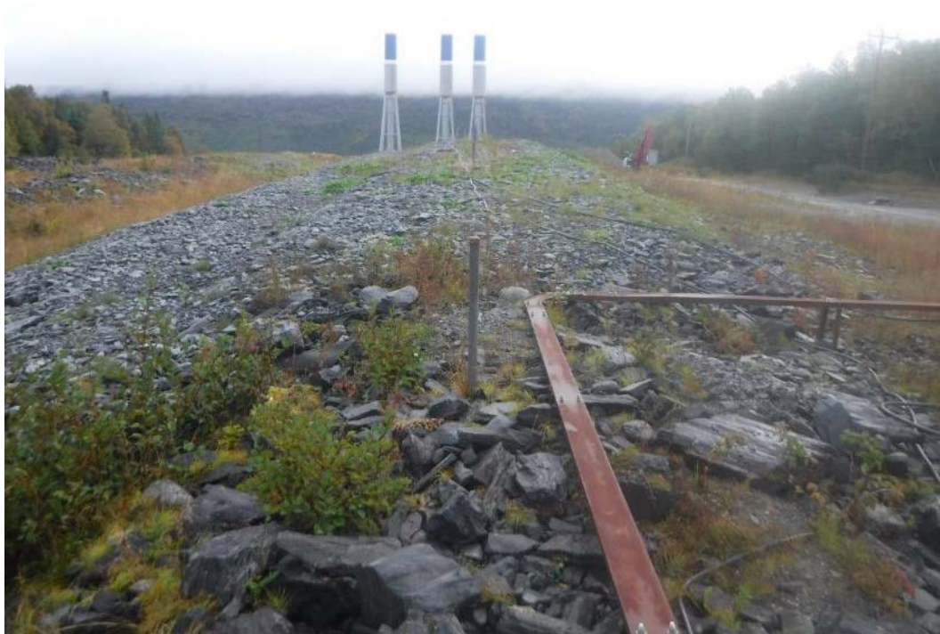
PHOTO 26 LOOKING DOWNSTREAM TOWARD SURGE TANKS ALONG PREVIOUSLY REPAIRED AREA
