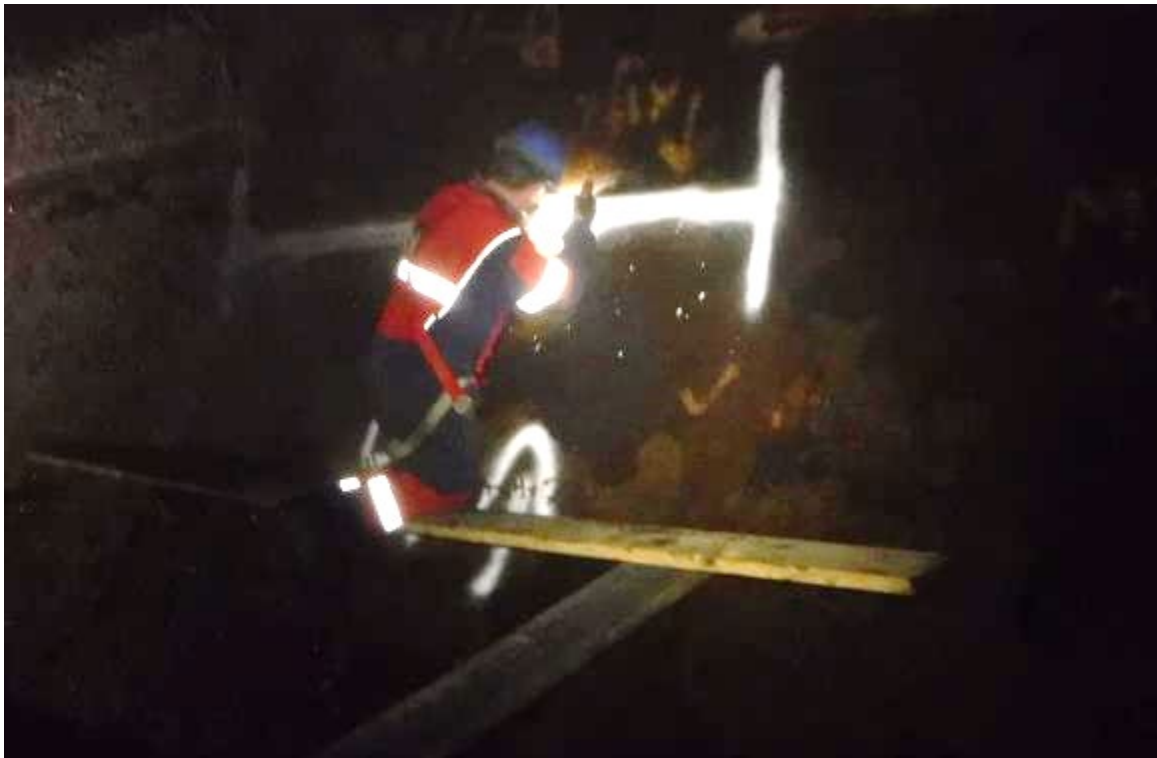
Photo 12 Connor performing MT on weld
