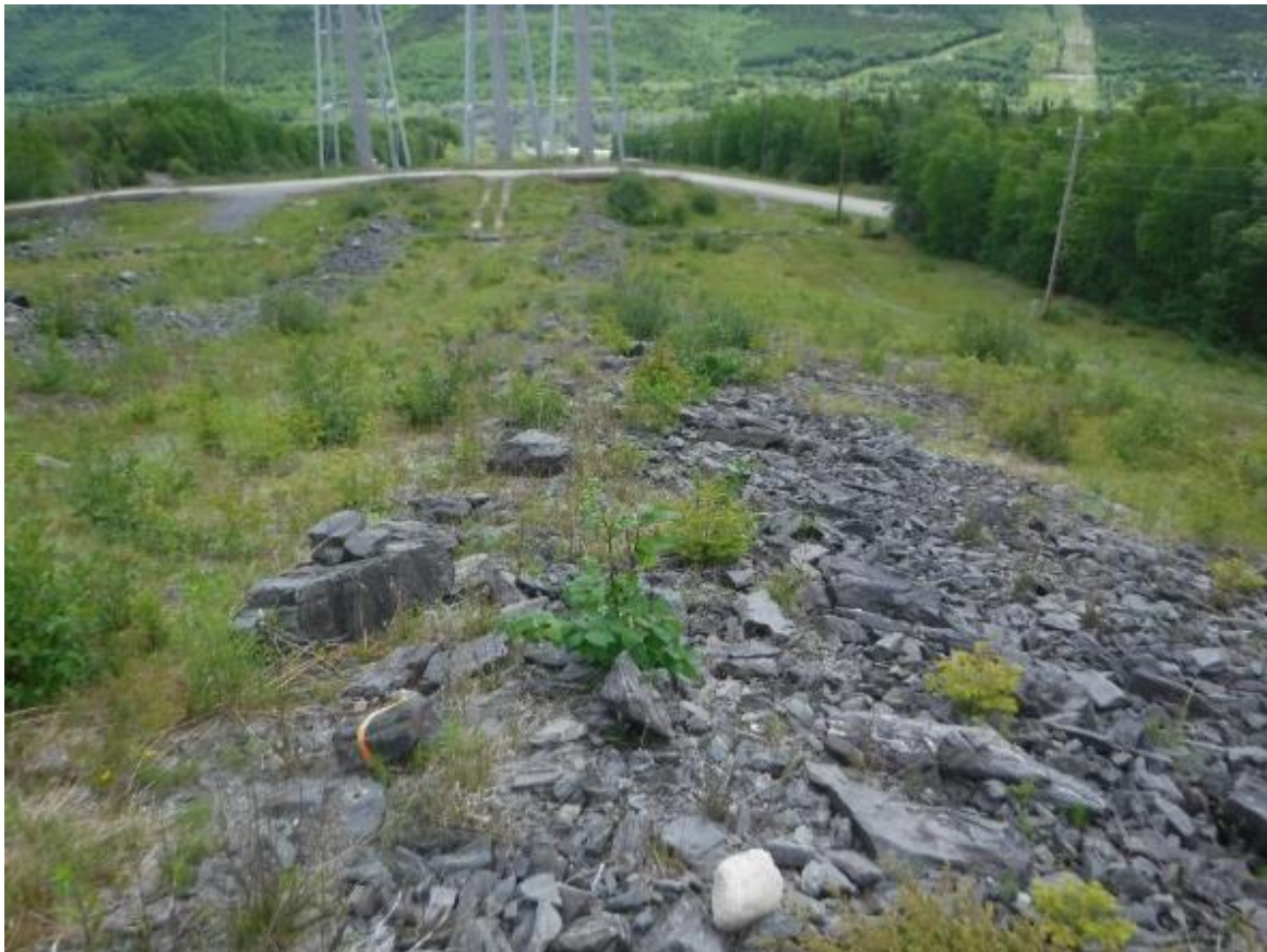
Photo 34 Looking downstream along Penstock 1 upstream of surge tanks
