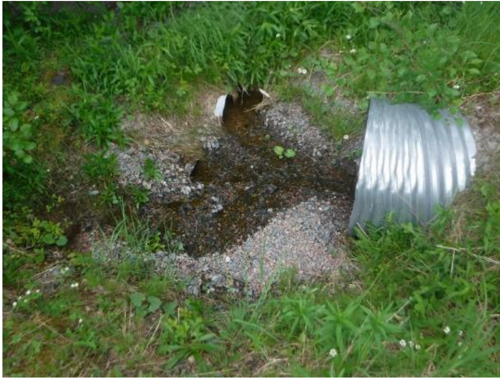
Photo 43 Drain at N1 upstream of monitoring shed
