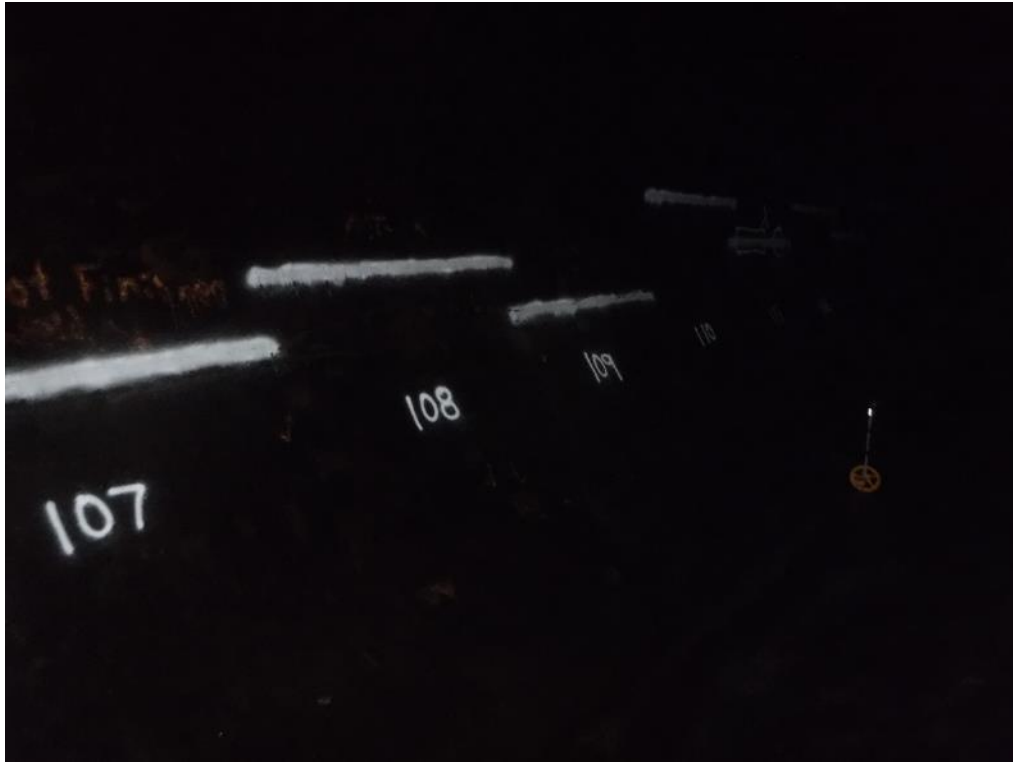
PHOTO 9 WELD TESTING OF EVERY CAN NEAR CAN 106'S CRACKED WELD
