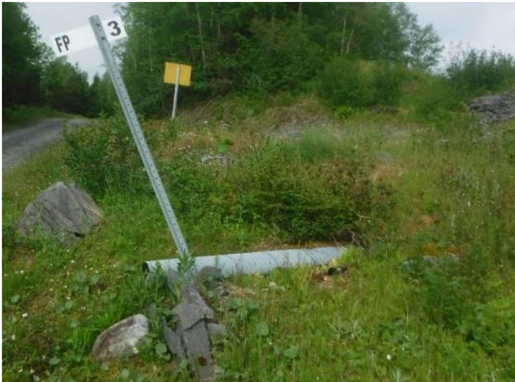
Photo 31 Upstream Drain at FP 3
