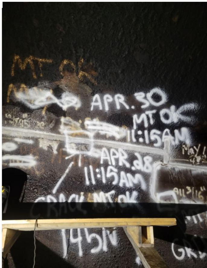
Photo 14 Weld repaired and marked Can 145
