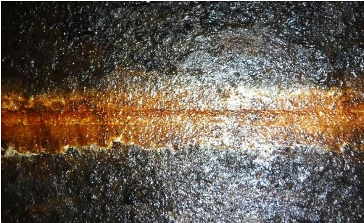
Photo 9 Typical original weld previously tested but not in 2020
