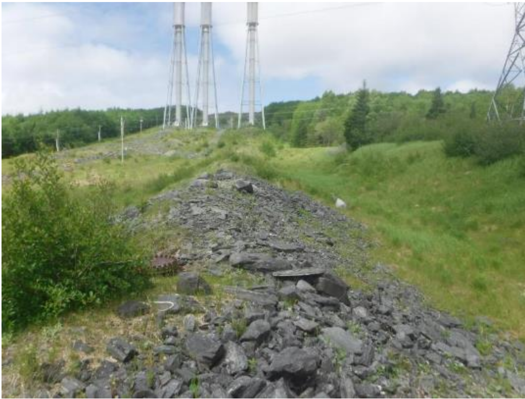
Photo 41 Looking upstream along Penstock 3 from last downstream manhole
