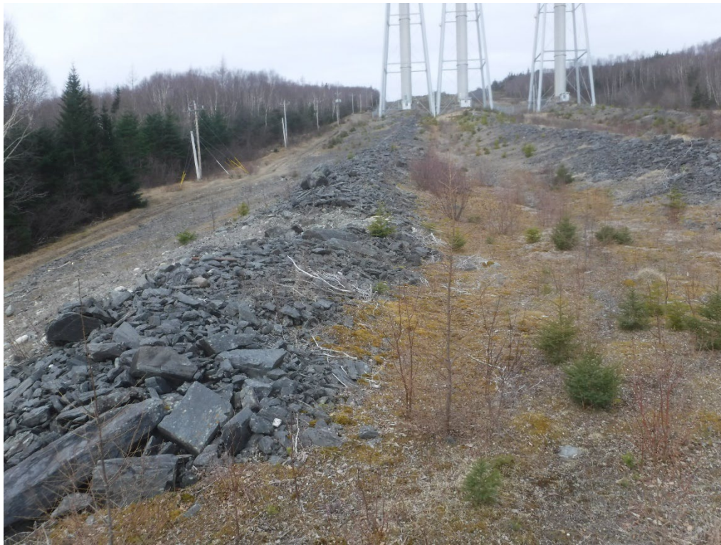
Photo 16 Looking Upstream from just downstream of surge tanks
