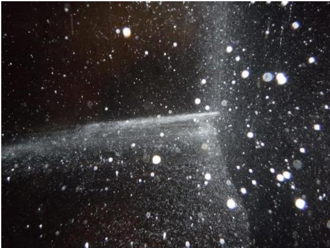
Photo 1 Leakage Bottom Left Corner of Gate
