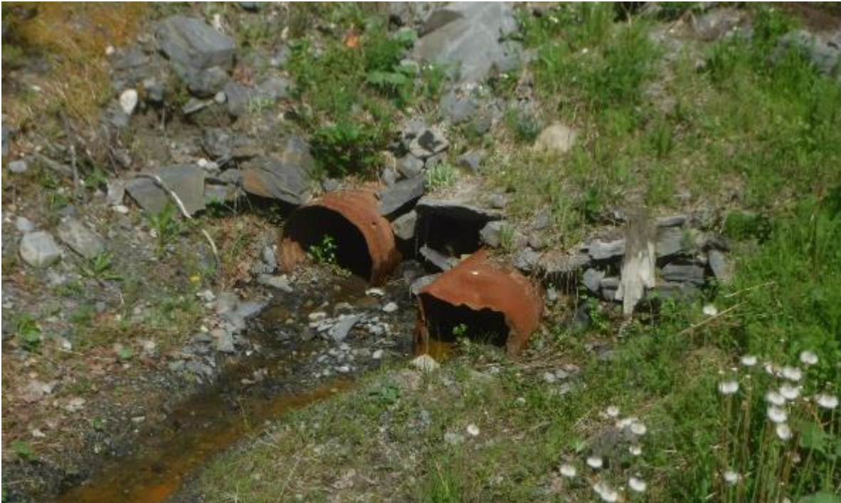
Photo 33 Drain pipes at FP 5
