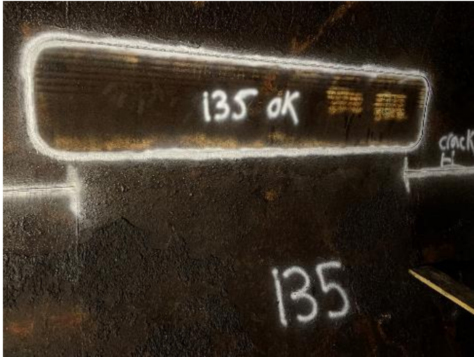
PHOTO 3 TYPICAL REINFORCING PLATE
