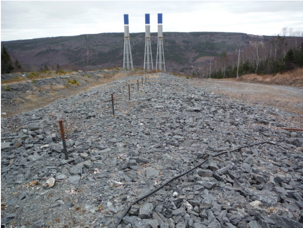
Photo 19 Previously repaired area; Rip-rap in good shape
