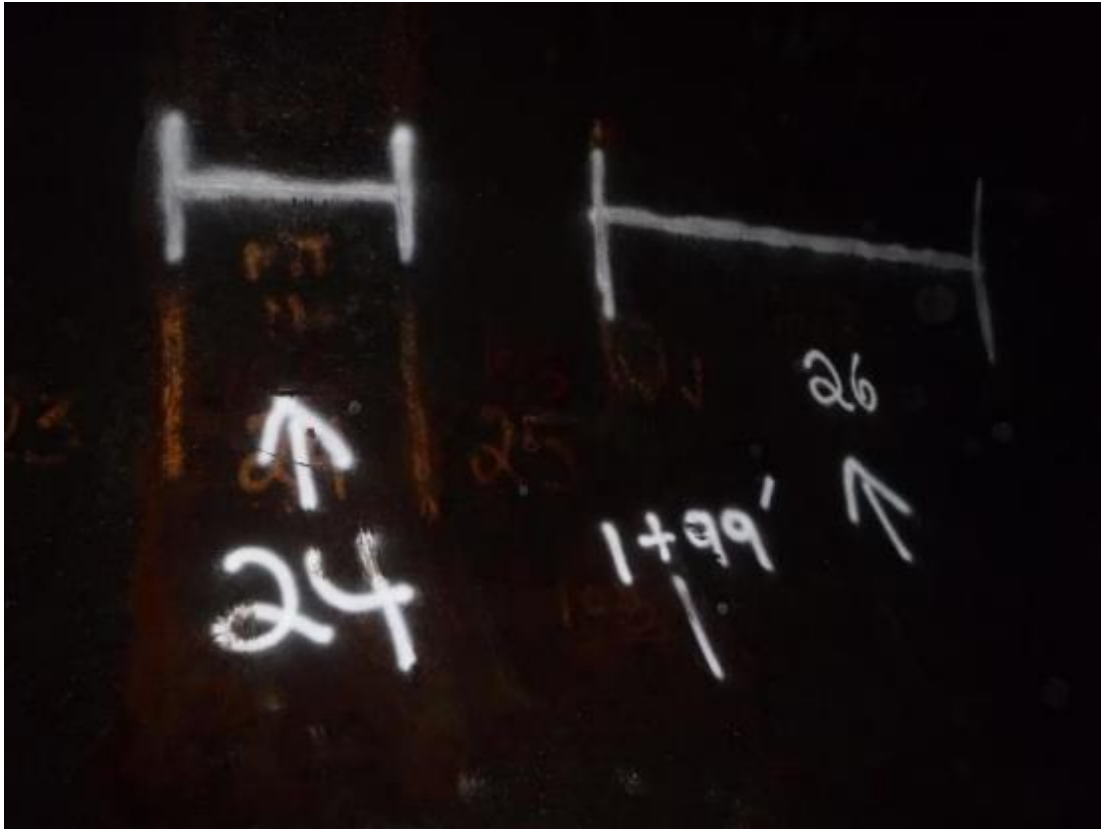
Photo 5 Typical markings for numbering cans, welds, and stationing 2020
