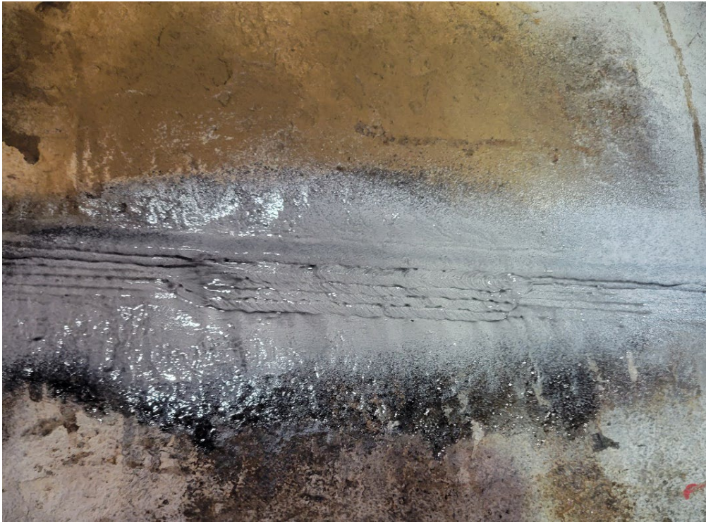
Photo 15 Weld repaired; Can 145
