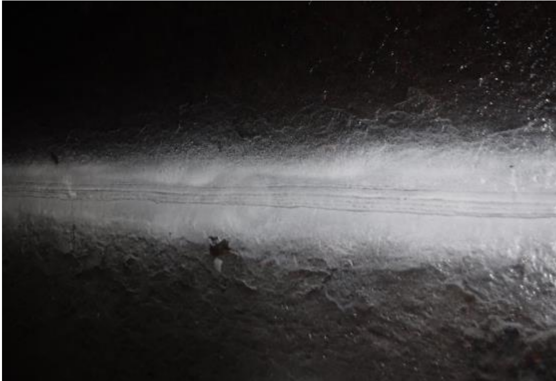
Photo 6 Typical repaired weld with contrast paint tested this year
