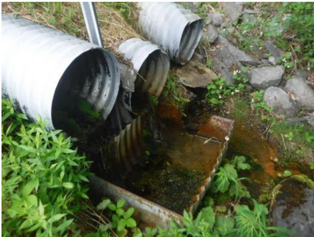
Photo 42 Drain outlet at N2
