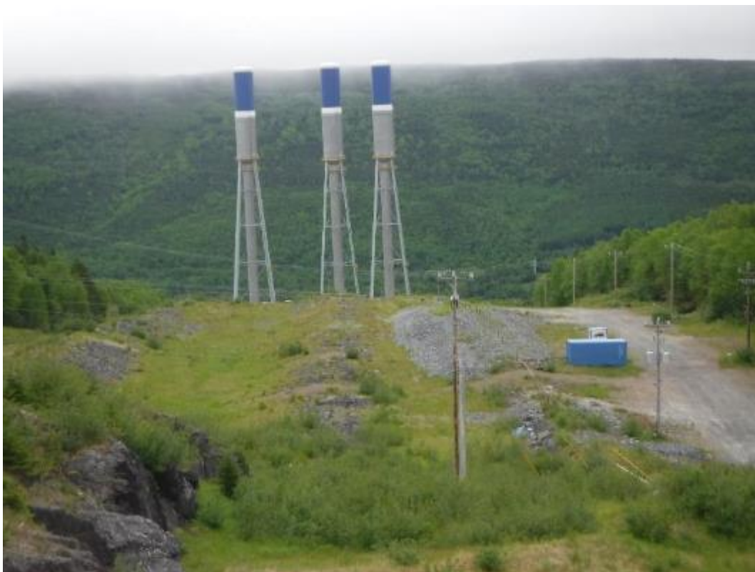
Photo 30 Looking downstream along Penstock 1 from the intake
