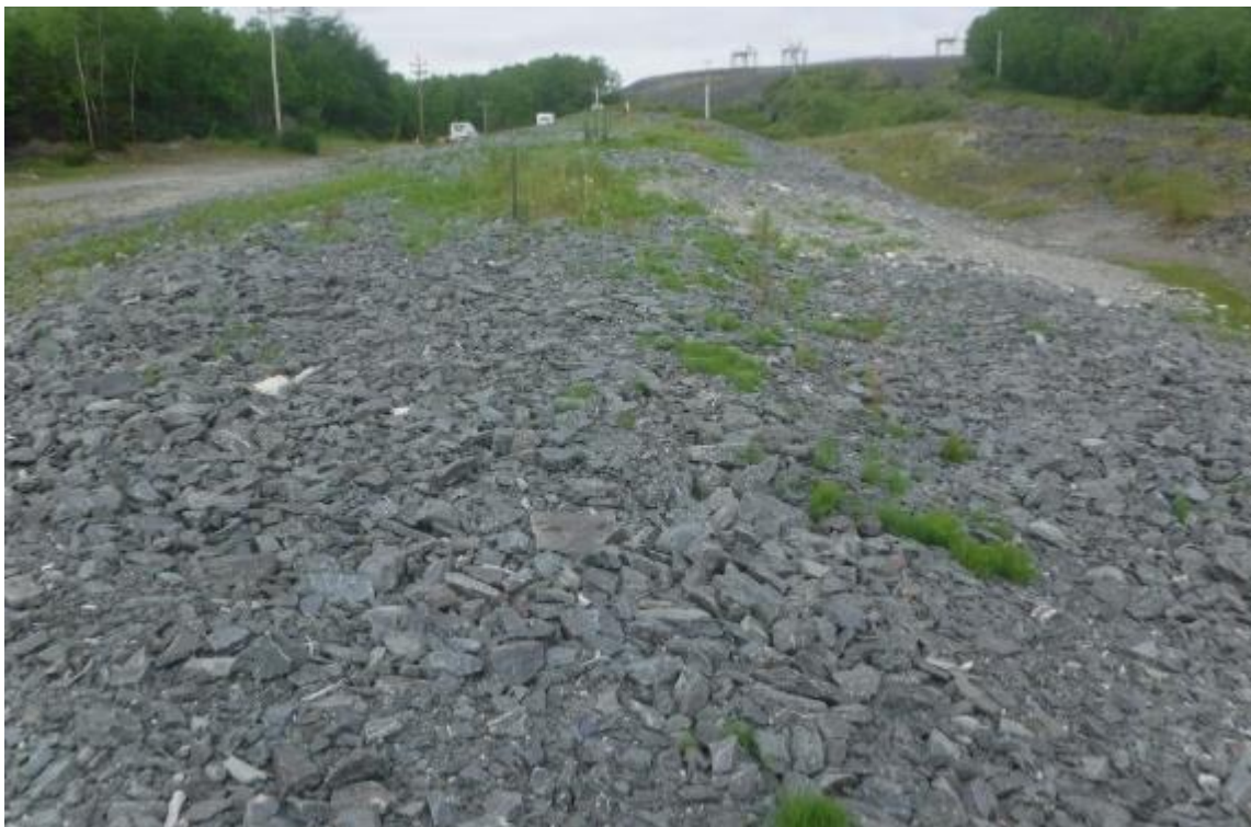
Photo 32 Riprap over repaired area of penstock
