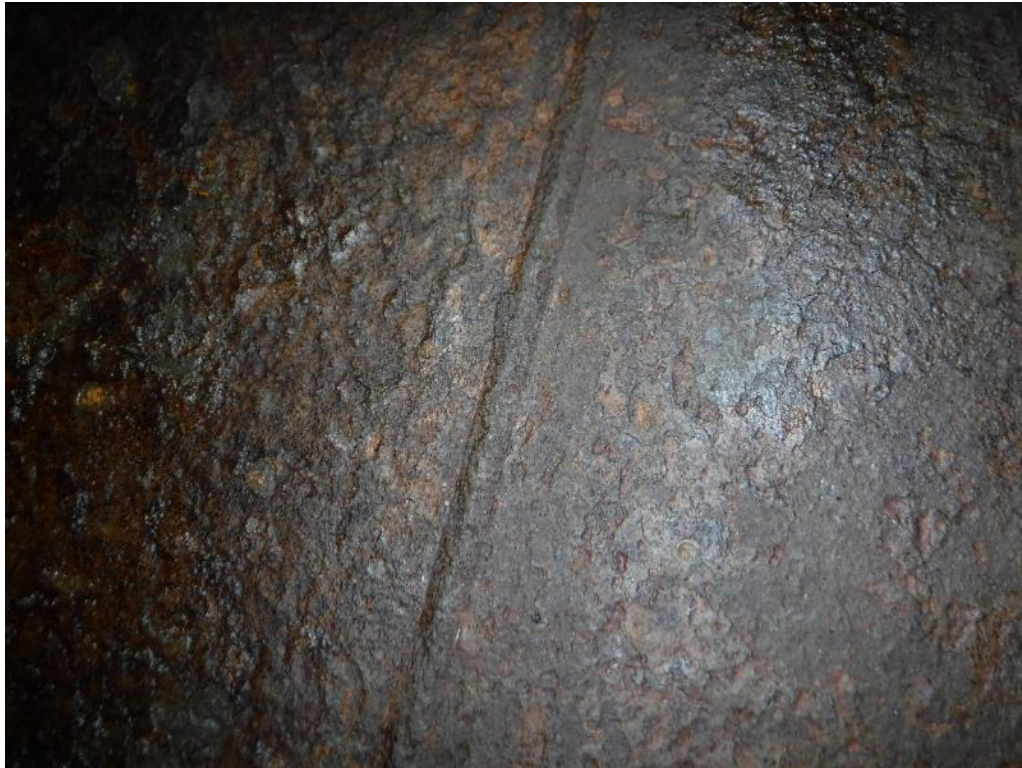
PHOTO 13 ORIGINAL CIRCUMFERENTIAL WELD CAN 194
