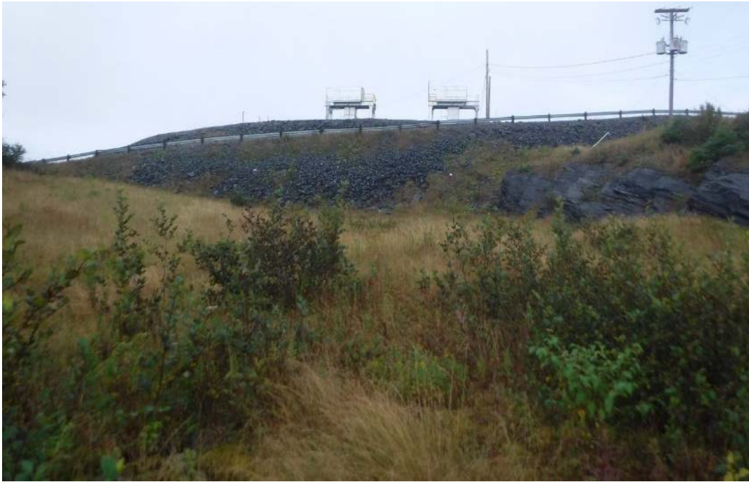
PHOTO 23 LOOKING UPSTREAM ALONG PENSTOCK 1 FROM NEAR TOE OF DAM
