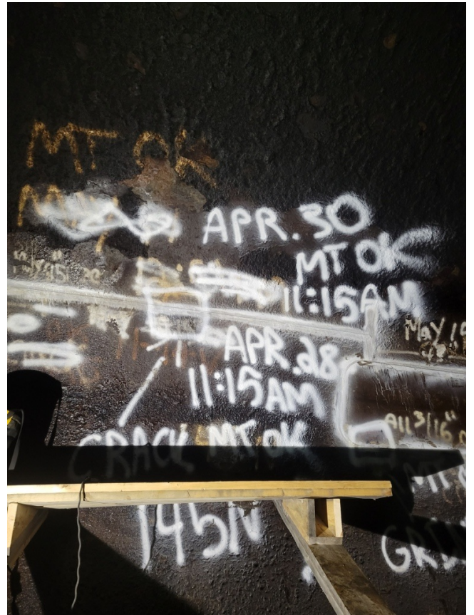
Figure 4. 145N Weld Repairs - Post 48 Hour Hold - Checked at 11:15 AM April 30 th 2022
