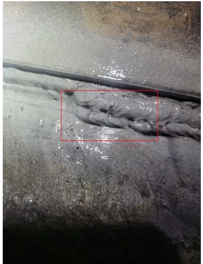
Figure 8. Can 145N - Indication Noted *Refer To Report 22-318 For Repair
