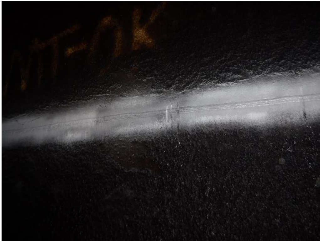
PHOTO 4 PREVIOUSLY REPAIRED WELD WITH CONTRAST PAINT
