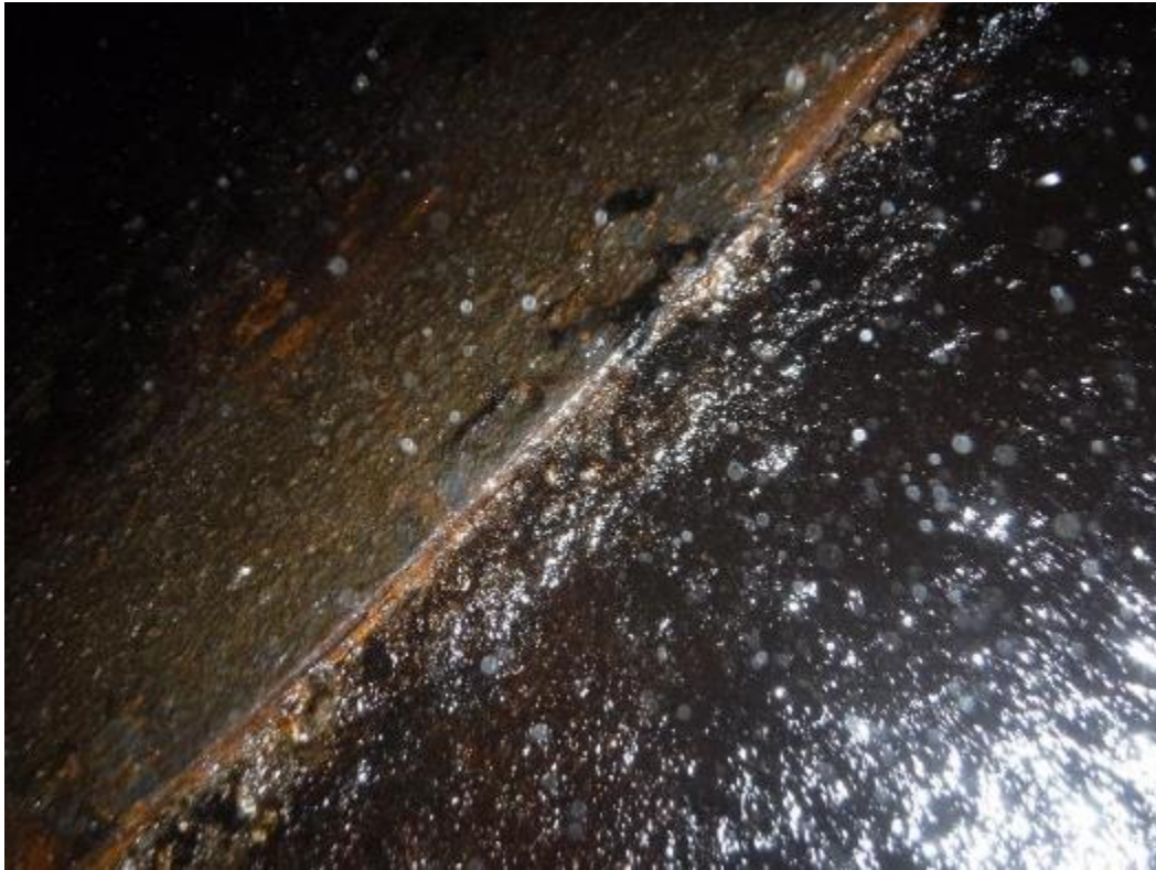
Photo 3 Concrete to Steel Transition Right Side
