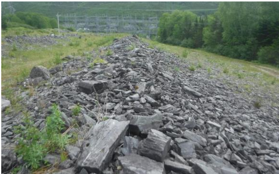
Photo 36 Looking downstream from surge tank
