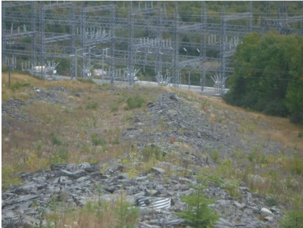
PHOTO 31 LOOKING DS ALONG PENSTOCK JUST DS OF TRANSMISSION LINE
