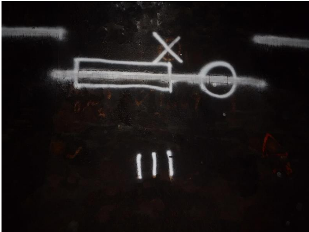
PHOTO 10 MT TEST SHOWED INDICATION OF ISSUE LEFT SIDE CAN 111 NEAR SPRING LINE
