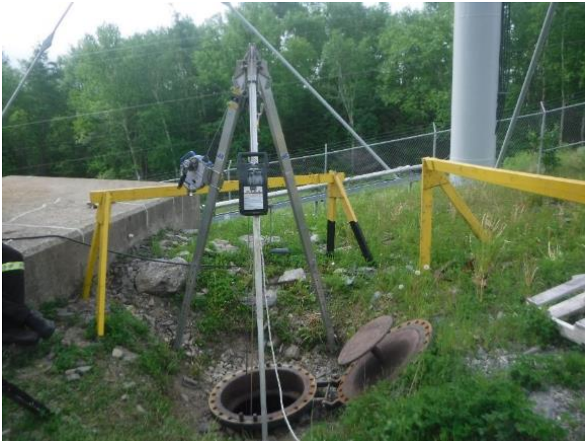
Photo 35 Manhole access immediately upstream of surge tank
