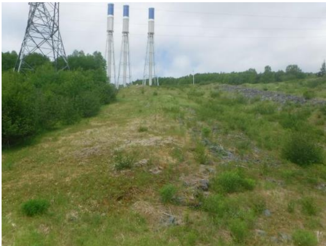
Photo 38 Looking Upstream from the switch yard
