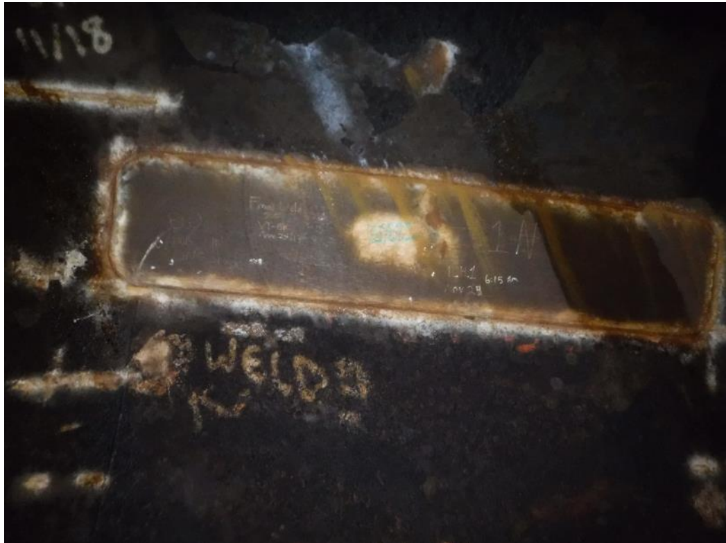
PHOTO 12 DOUBLER PLATE REPAIR
