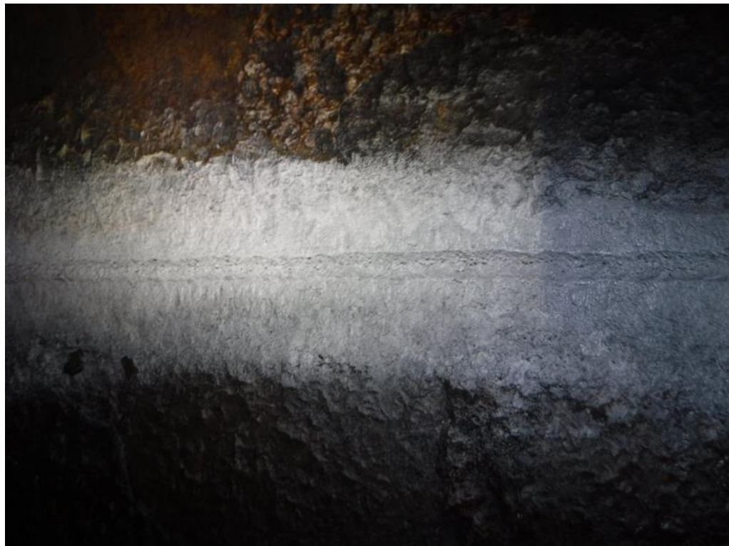
PHOTO 14 ORIGINAL HORIZONTAL WELD CAN 201
