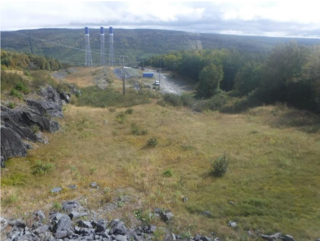
PHOTO 24 LOOKING DOWNSTREAM ALONG PENSTOCK 1 FROM NEAR TOE OF DAM
