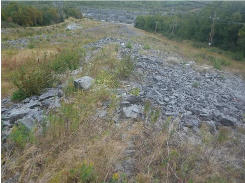
PHOTO 29 LOOKING DS ALONG PENSTOCK JUST DS OF SURGE TANK
