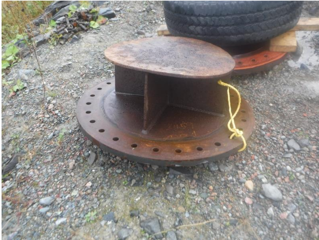
PHOTO 25 MANHOLE 1 COVER WITH REINFORCING PLATES
