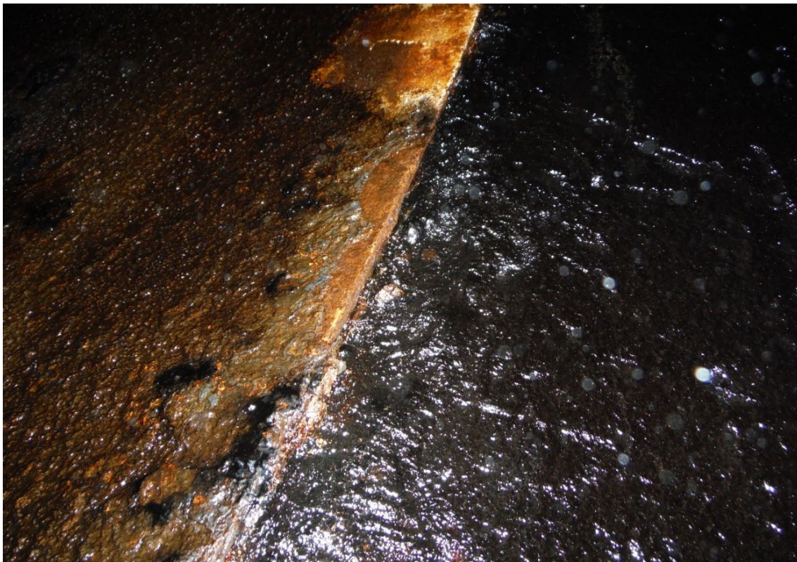
Photo 2 Concrete to Steel Transition
