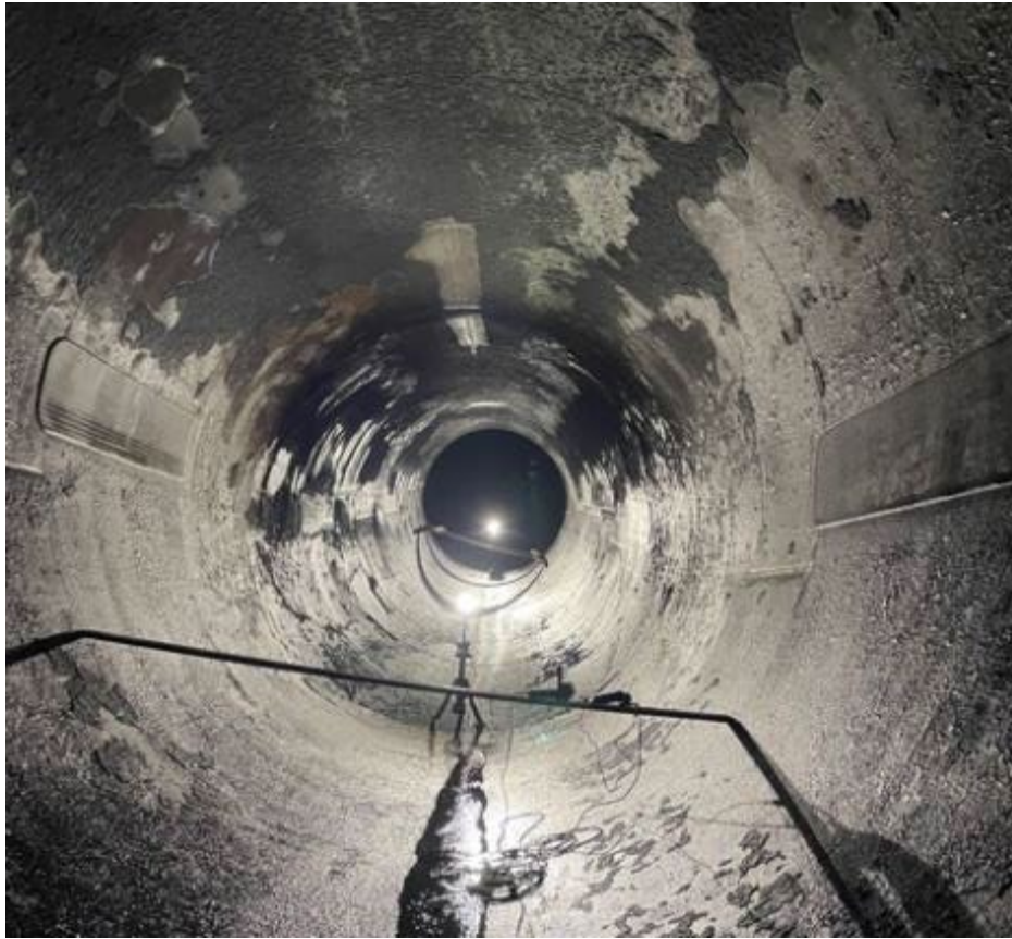
PHOTO 1 TYPICAL CONDITIONS IN 17 FT DIAMETER SECTION
