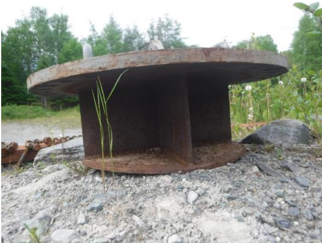
Photo 27 Cover for Manhole No. 2 (Second Downstream of Intake)
