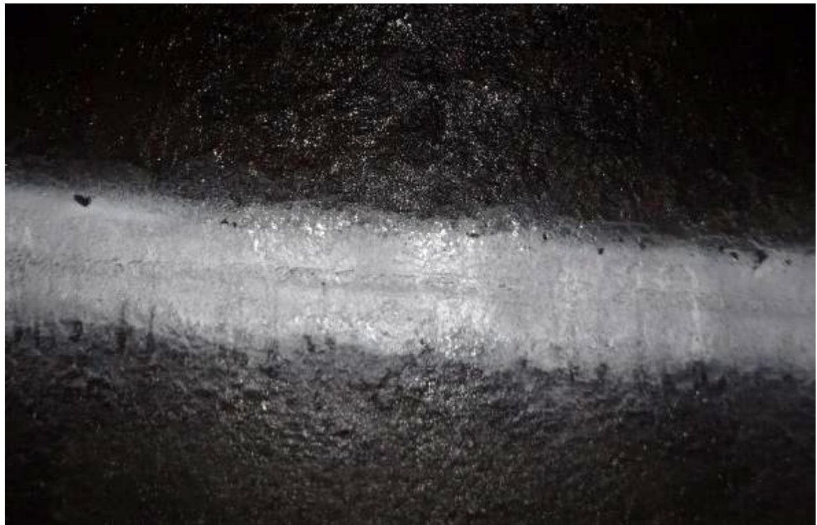
Photo 10 Typical original weld with contrast paint tested this year
