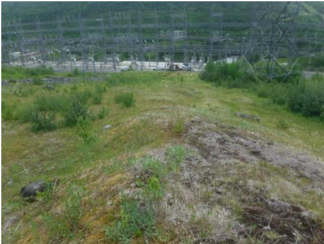
Photo 37 Looking downstream from surge tank
