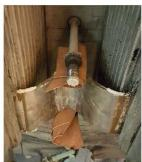
Figure 1 - Jumper with all insulation stripped. Added rubber insulation between copper and studs
