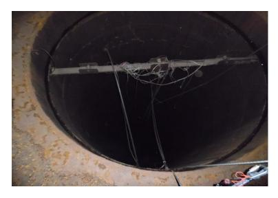
General condition of riser cross braces and coatings inside of riser. Bent and missing bolts.
