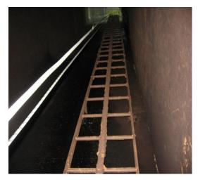
Figure 3-1: General Condition of Ladder from Headgate to Bottom of Penstock, Corrosion Present
