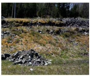
Figure 22 - Backfill Slope Failure
