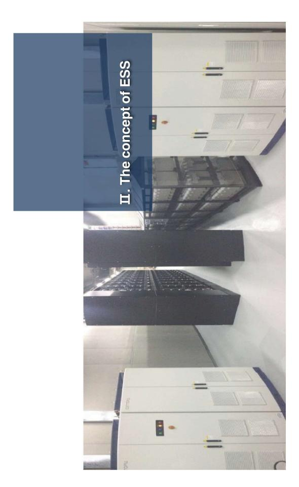
BESS(Battery Energy Storage System), so-called ESS, is a system used for storing electrical energy to secondary battery for timely use.
