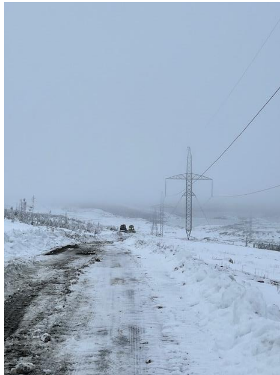
Figure 11: Snow Conditions at Structure 1872
