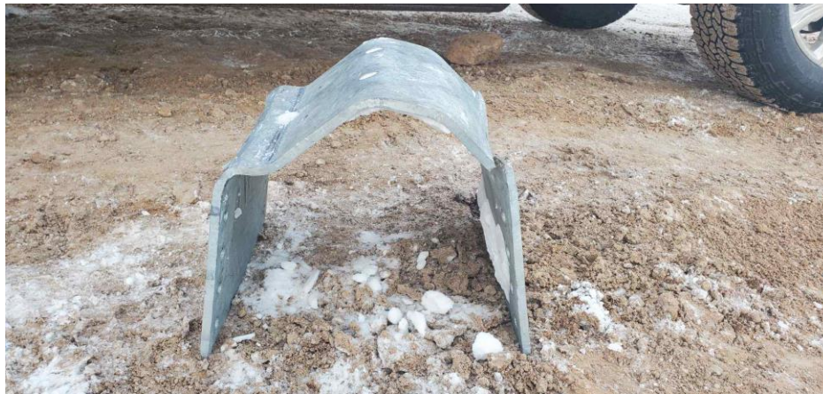
Figure 5: Bent Top Plate after Removal from Tower
