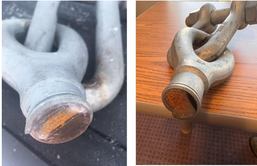
Figure 18: Failed Turnbuckle Faces from February 2021 (left) and December 2022 (right)
