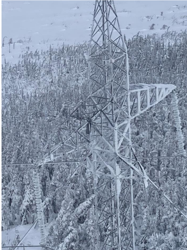
Figure 8: Ice on Structure 2135
