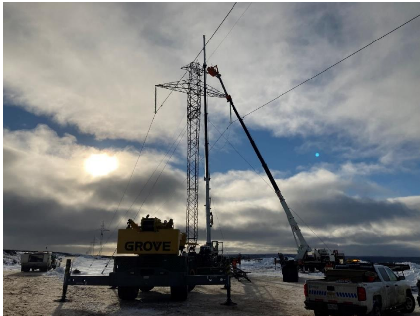
Figure 11: Repair work to OPGW Peak
