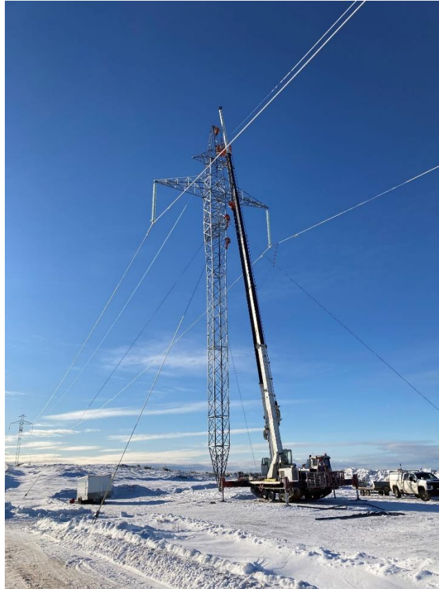
Figure 12: New OPGW Tower Peak Installed
