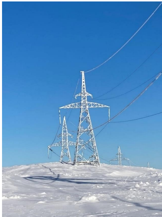
Figure 14: Snow at Site near Structure 1014 Failure
