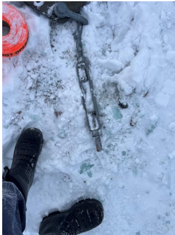
Figure 7: Failed Turnbuckle on the Ground at Structure 1806
