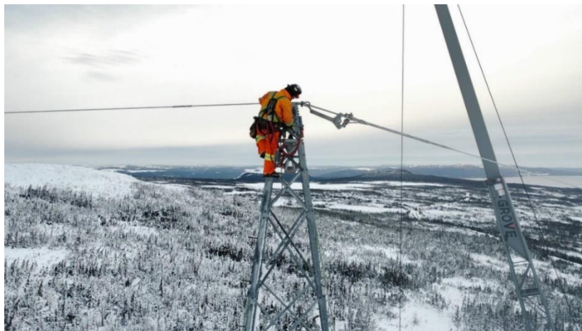
Figure 9: Repair Work to OPGW Peak
