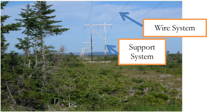
Figure 2.6 A Typical Wood Pole H-Frame Line System
