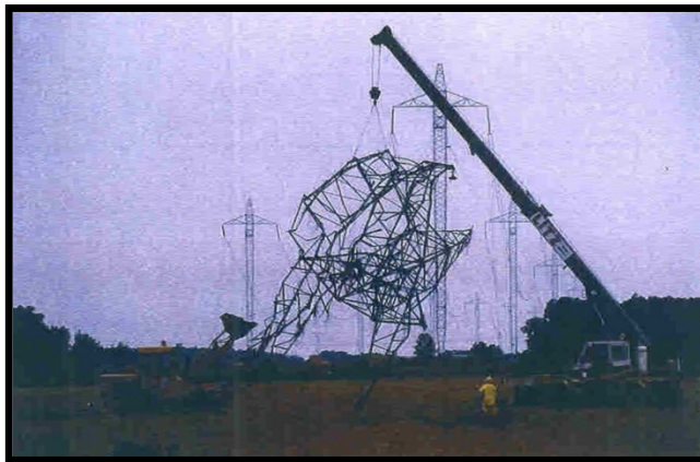
Figure 3.4 DC Tower Failure under Microburst (High Intensity Wind, MH Bipole Lines)
