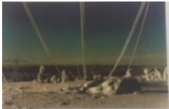
Figure 3.3 735 KV AC Line Failure at Churchill Falls (Heavy Icing on Conductors)
