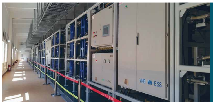
Figure 5.2.2 Typical VRB ESS installation.
