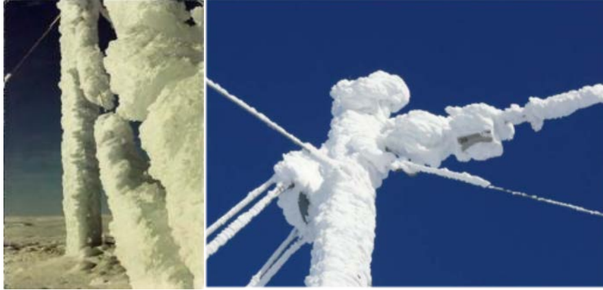
Figure 1.5 (a) Rime Icing in Labrador, 1977 (courtesy NLH) and (b) Rime Icing on a test Span (2010, LRM)
