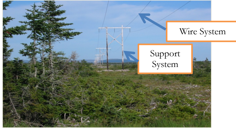
Figure 2.6 A Typical Wood Pole H-Frame Line System
