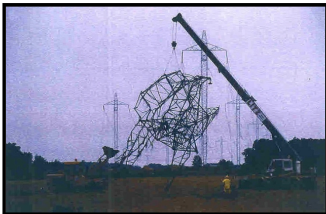
749 Figure 3.4 DC Tower Failure under Microburst (High Intensity Wind, MH Bipole Lines)
