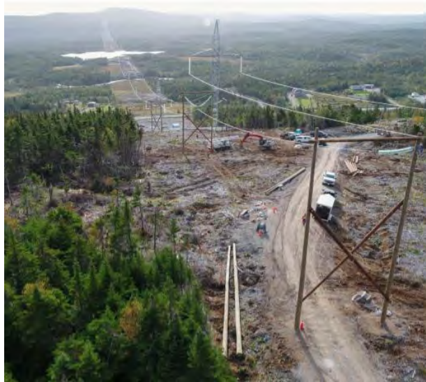
Figure 2: Wooden Pole Solution Used in 2018 Mock Exercise
