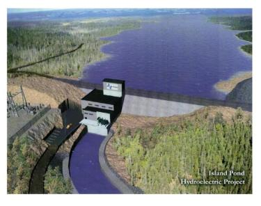
12 respectively. Electricity would be produced by one 36 MW turbine and generator assembly. The
