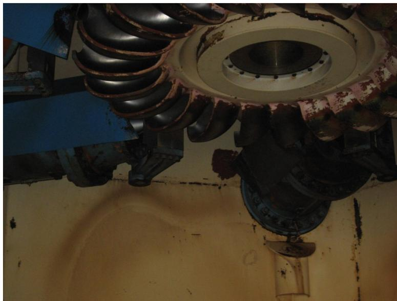
**Figure 2: Cat Arm Pelton Turbine (Runner and jets)**
