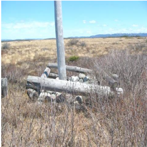
Figure 3: Pole Crib Requiring Repairs
