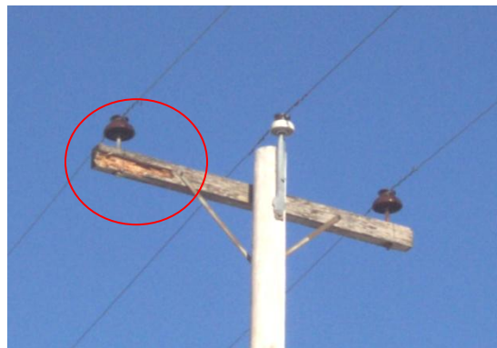
Figure 2: Rotten Crossarm
