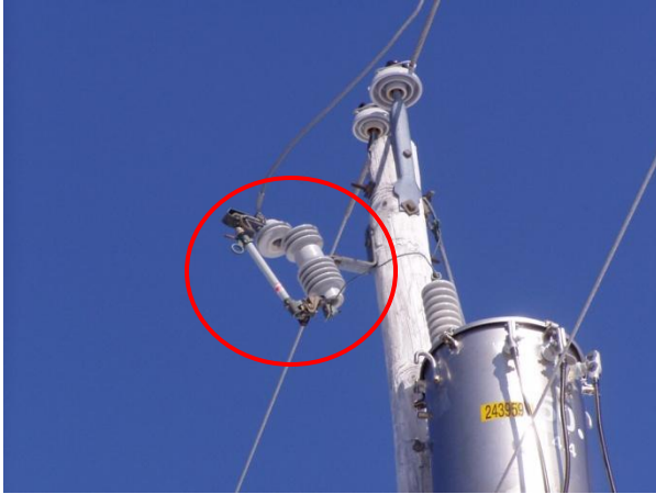
Figure 11: Broken Porcelain Cutout In Service
