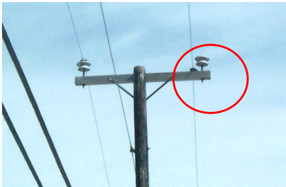
Figure 6: Broken Insulator In Service
