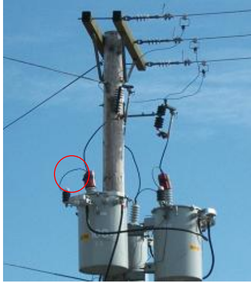
Figure 5: Lightning Arrestors In Service
