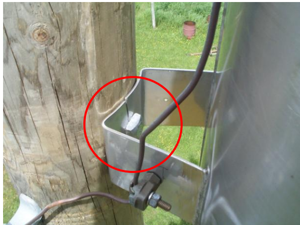
Figure 14: Broken Stainless Steel Transformer Hanging Bracket
