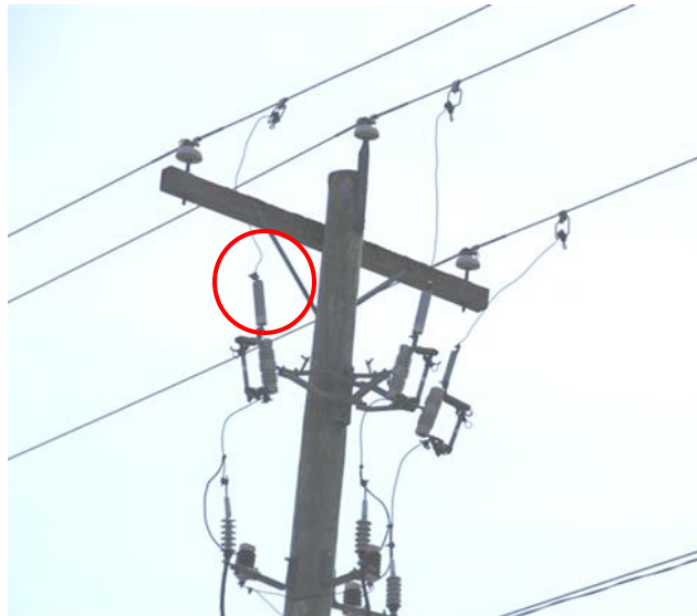
Figure 8: Current Limiting Fuses In Service
