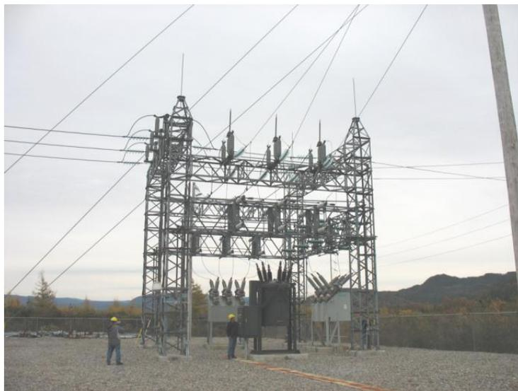
**66kV Steel Structures & Bus**
