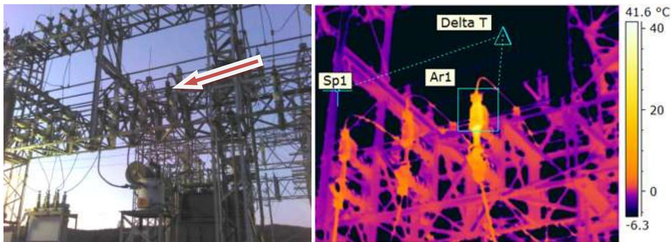
**CAR-T1-D Switch Replacement (Hot spots visible with infrared camera)**
