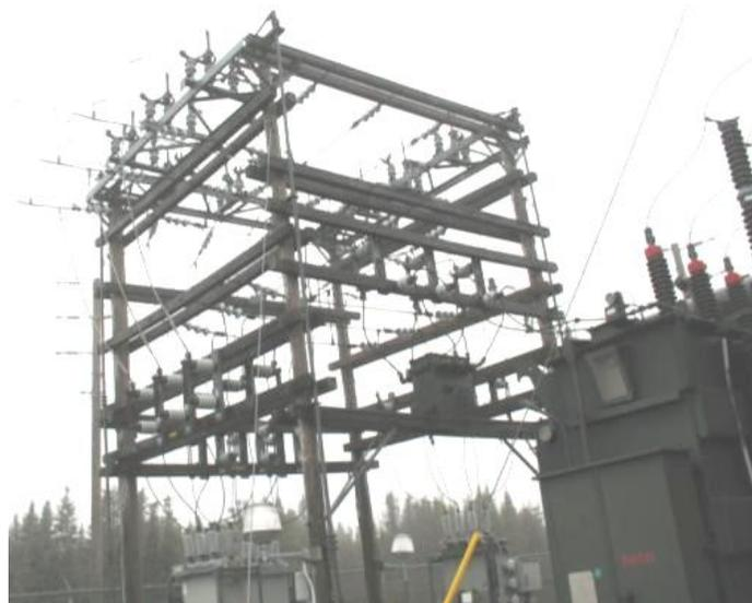
**12.5 kV Wooden Structures & Bus**
