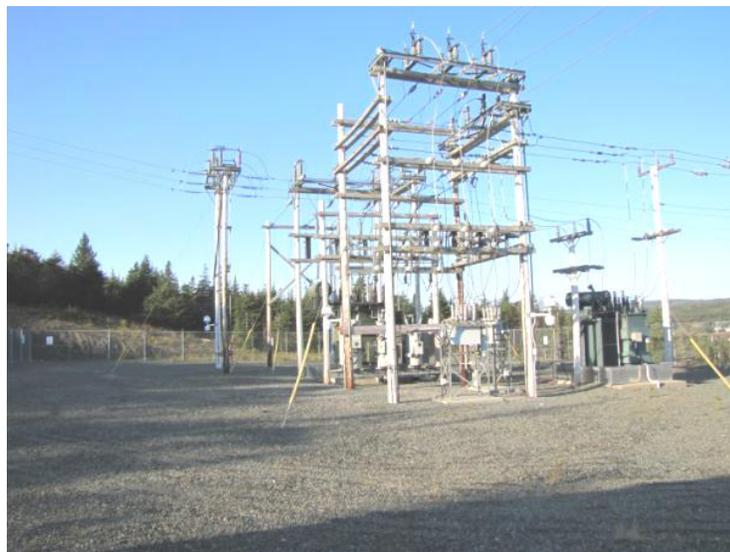
**66 kV & 15 kV Wood Pole Structures and Bus**
