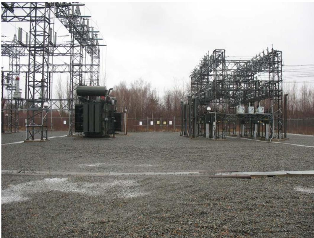
**138kV & 25 kV Steel Structures & Bus**
