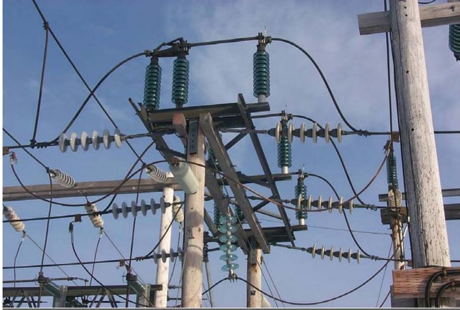
**Bus Tie Switch Bypassed Goulds Substation**
