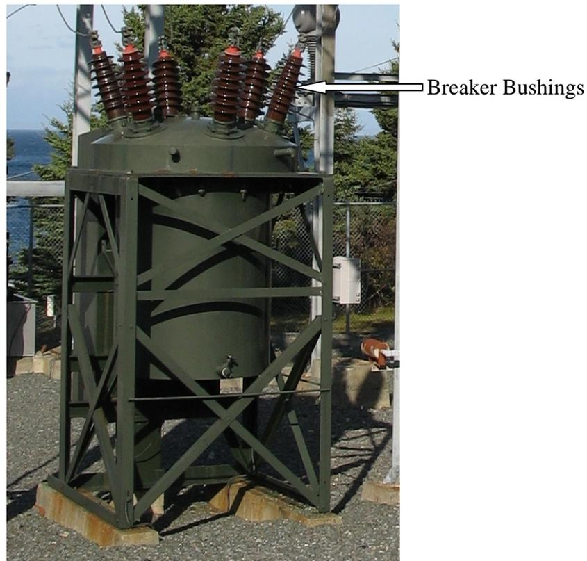
**Figure 2 - 66 kV Bulk Oil Breaker**
