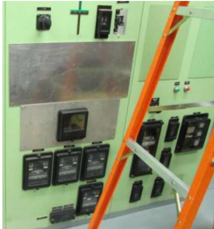
**Transformer Protection Panel (Electromechanical Relays)**
