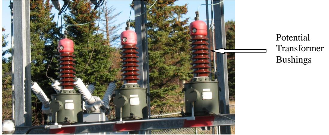
Figure 3 - 66 kV Potential Transformers
