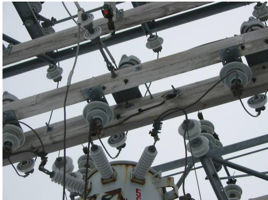
Cracked crossarm Garnish Substation
