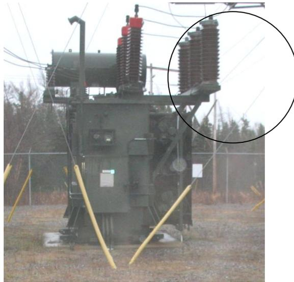
**Power Transformer with Silicon Carbide Arrestors**
