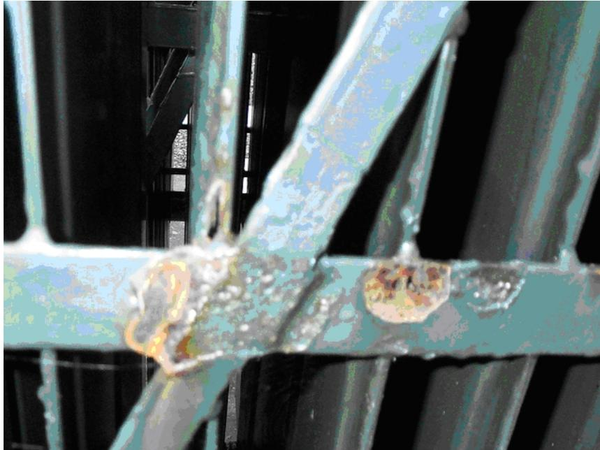
Deteriorated radiator fin edges – Blaketown Substation
