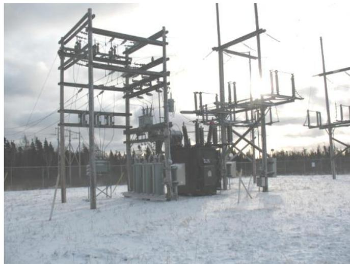
**138kV & 25 kV Wooden Structures & Bus**
