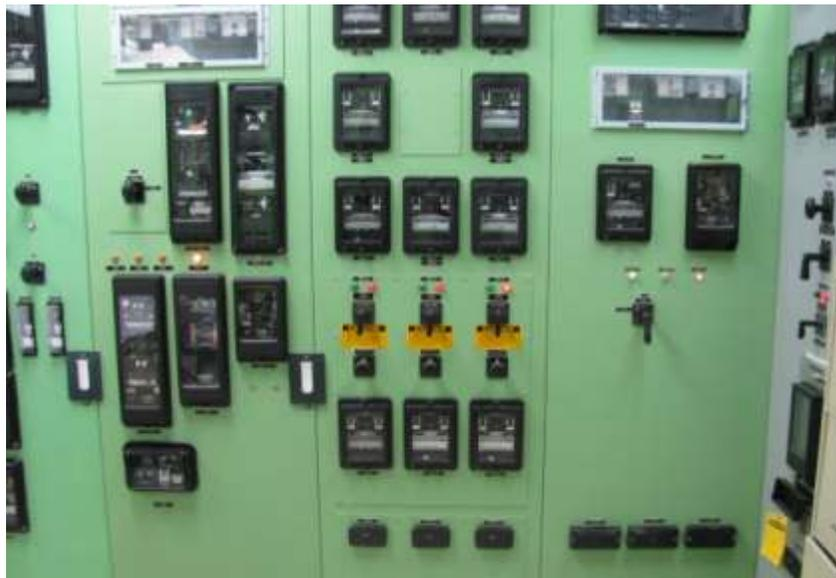
**Transmission Line Electromechanical Relay Panels and RTU**
