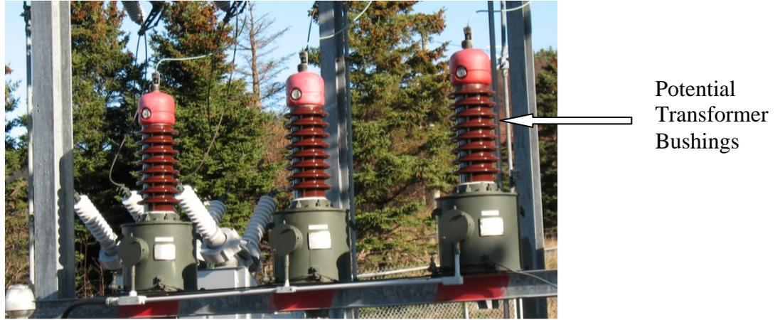
Figure 3 - 66 kV Potential Transformers
