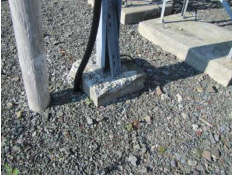
**Deteriorated 15kV Pothead Structure Column Foundation**
