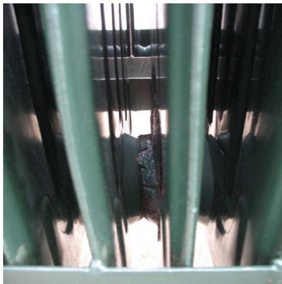
**Gillams Transformer Radiator Deterioration**
