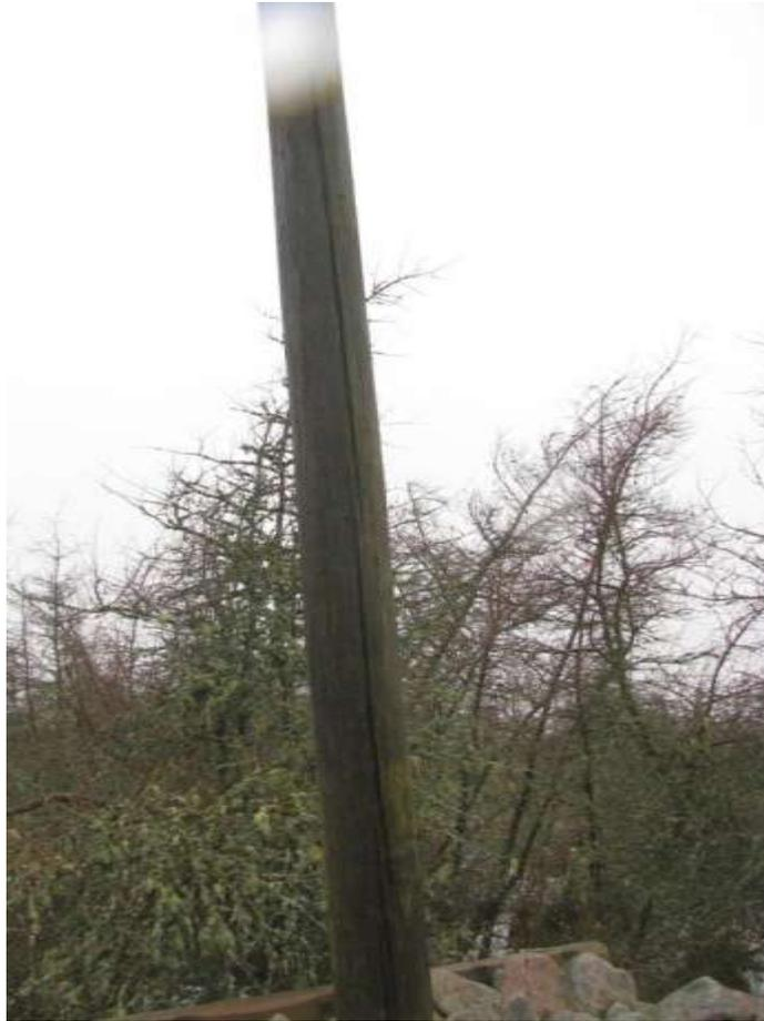
Figure 11 – 18L - Pole with severe checks
