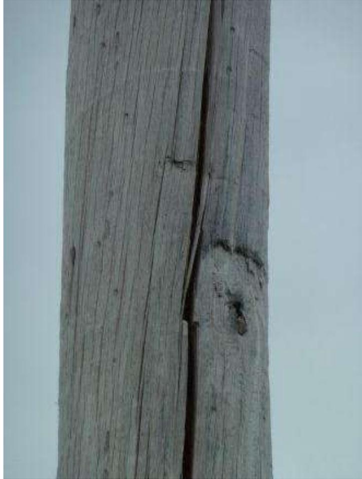
**Figure 19 – 68L - Pole showing shell separation**
