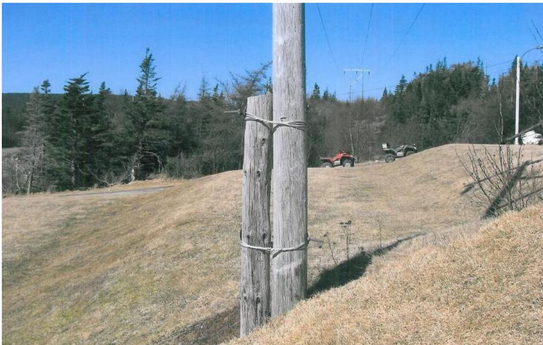
**Figure 8 – Pole requiring temporary support 21L**
