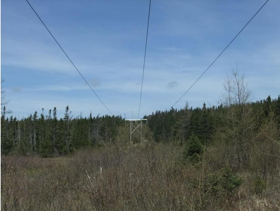
**Figure 19 – Location with Reduced Ground Clearance 124L**
