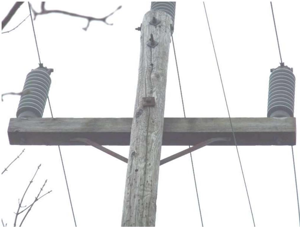
**Figure 1 – 12L - Pole showing checking around bolts**
