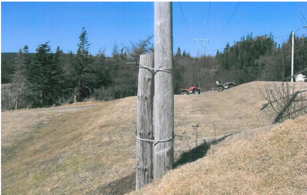
**Figure 6 – Pole requiring temporary support 21L**
