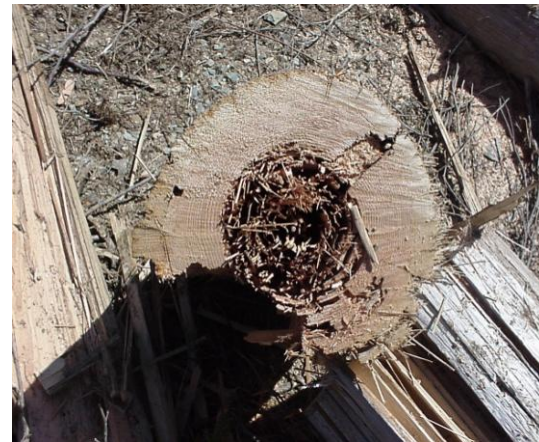
Fig. 3.19b – Carpenter Ant Damage
