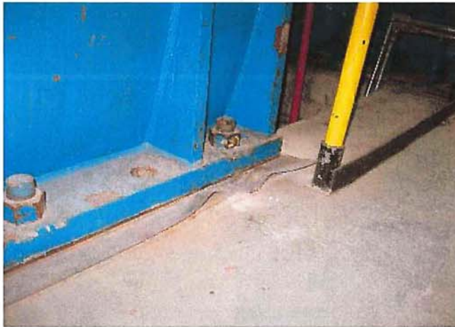
Figure 1 Generator Shim – LHS Turbine End
