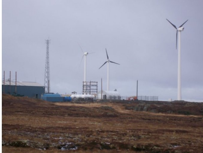
Overall Project Site Showing (l-r) the Diesel Plant/Storage Tanks, Meteorological Tower, Hydrogen Electrolyser, 3 Hydrogen Storage Tanks, Distribution Box Structure, 3 Wind Turbines, and Quonset Hut Housing the Hydrogen Genset.
