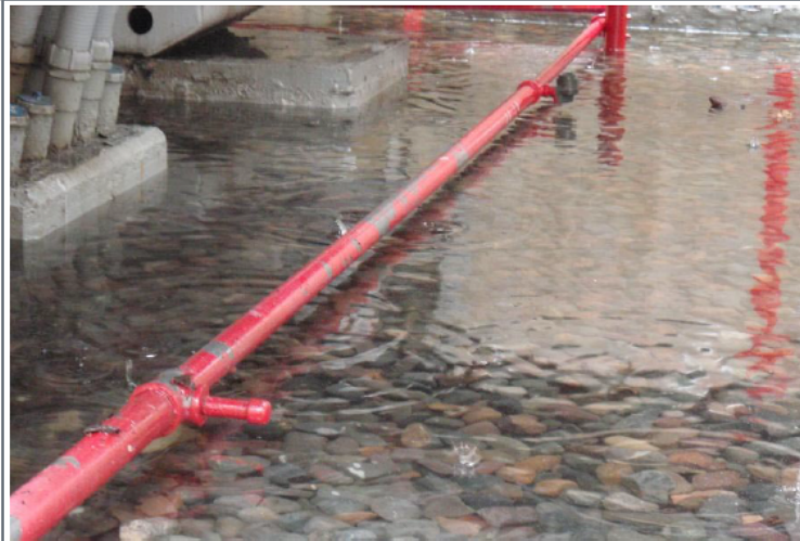
Missing Spray Nozzle on Transformer No. 1
