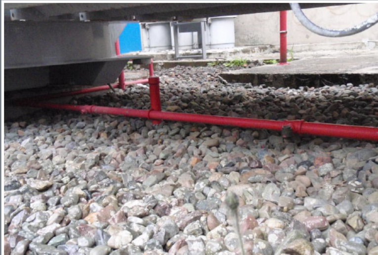
Missing Nozzle Transformer No. 4
