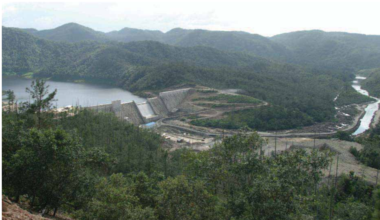
In Belize, the Chalillo storage and hydroelectric generating facility is expected to double the average annual energy production from the Macal River to 160 GWh.
