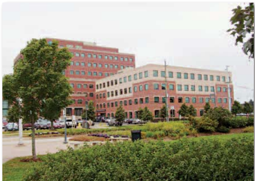
Growth in the Real Estate Division was primarily derived from completion of the $6.2 million, 57,000-square foot expansion of the Blue Cross Centre in Moncton, New Brunswick.
