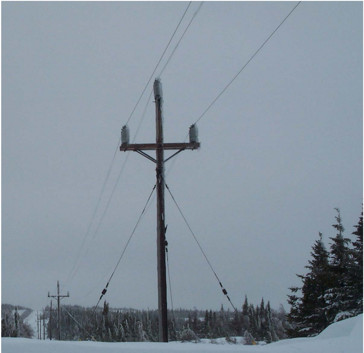
Figure 9 – Failed Guy Wire and Ice Loading on 111L
