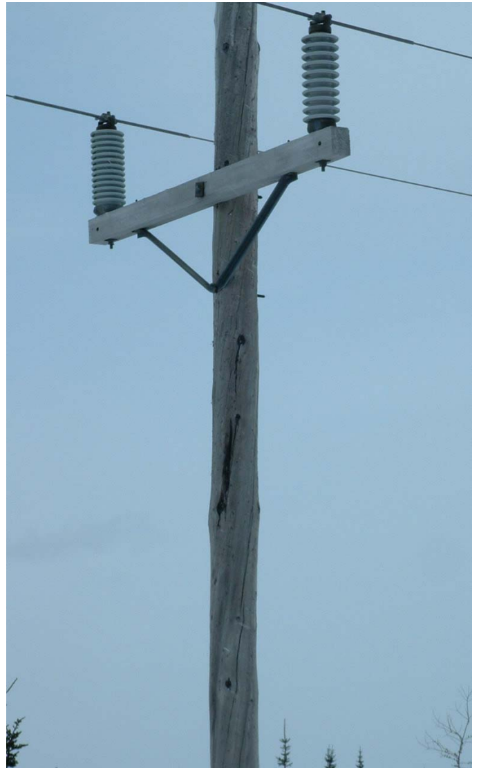
Figure 6 - Deteriorated Pole 111L
