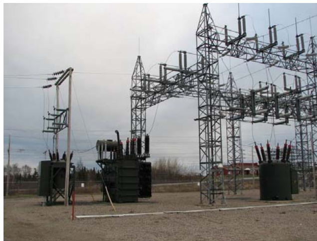
66 kV Breaker By-pass Switch To Be Installed On 110L
