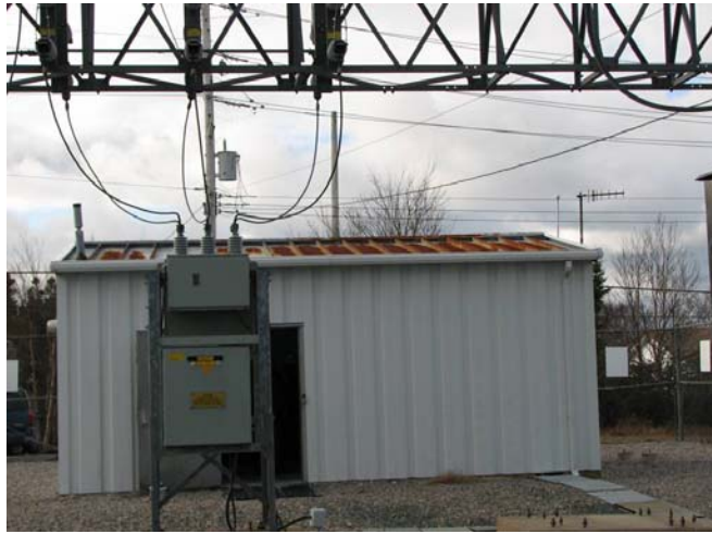
Control Building Roof Deterioration
