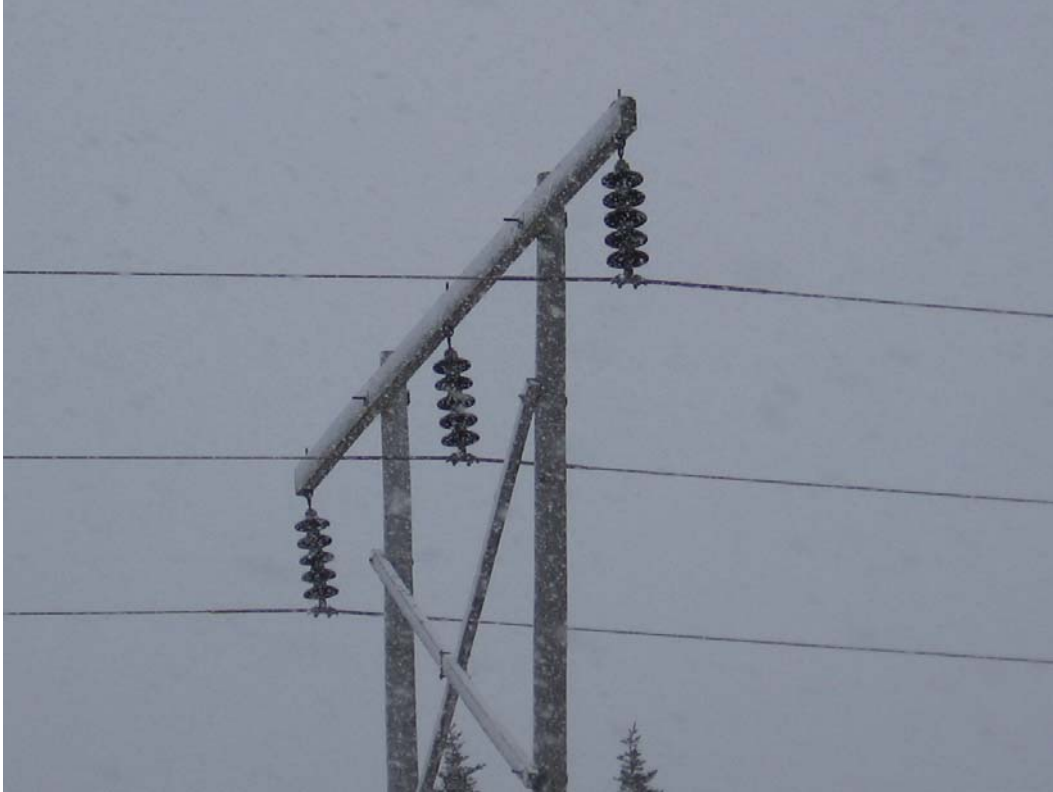
Figure 3 - Old Insulators 20L
