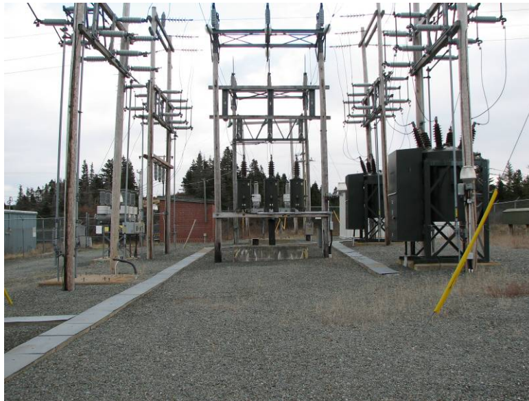
66 kV Potential Transformers
