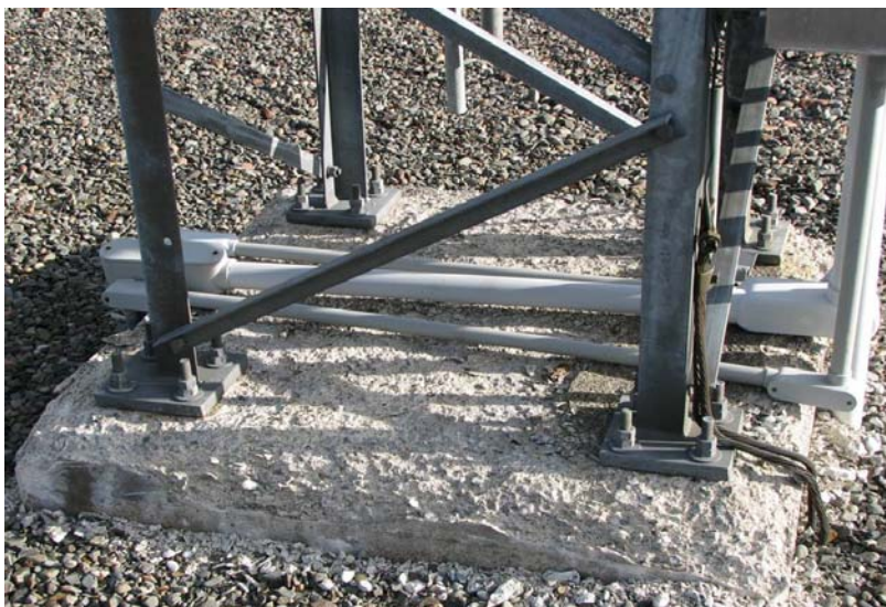
25 kV Structure Foundation
