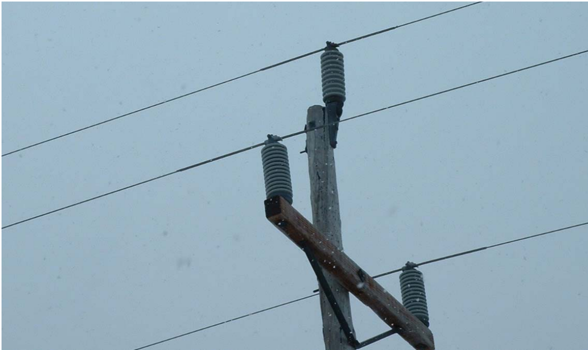
Figure 7 – Deteriorated Pole (Top Split) 111L
