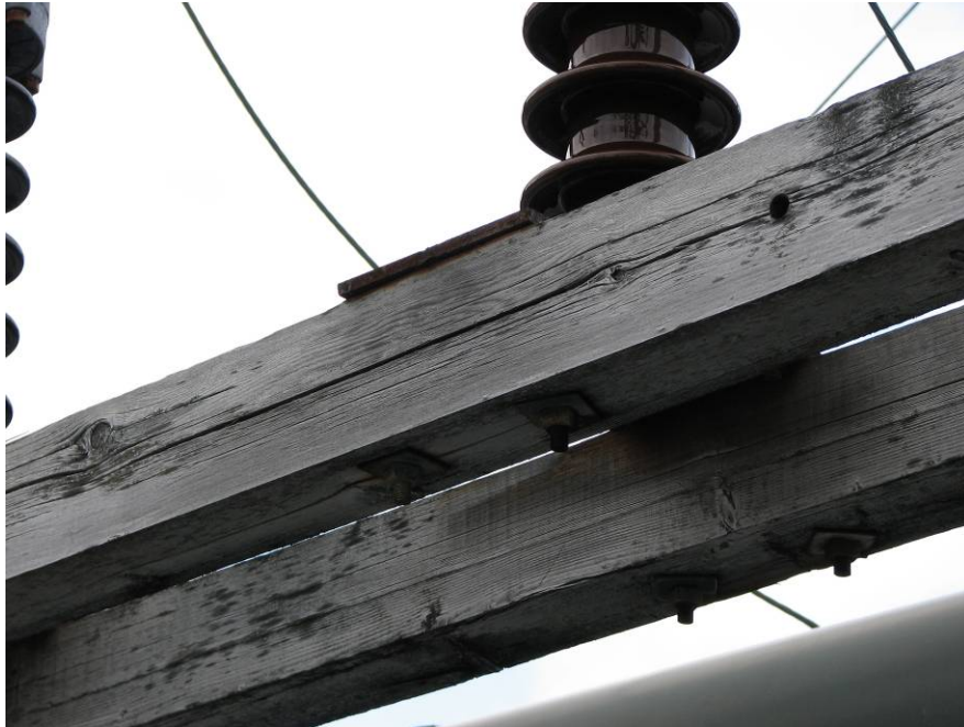
Deteriorated Crossarms 66 kV Structure
