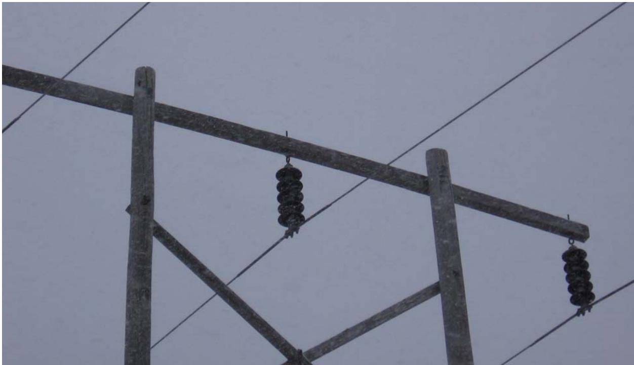
Figure 4 - Deteriorated Poles (top split) 20L
