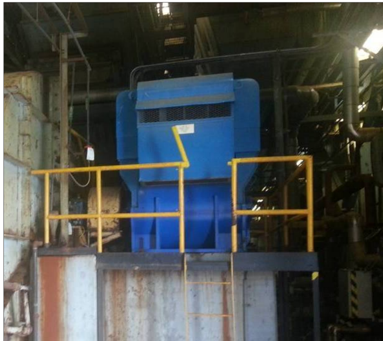
Figure 1: Holyrood Stage 1 Forced Draft Fan Motor
