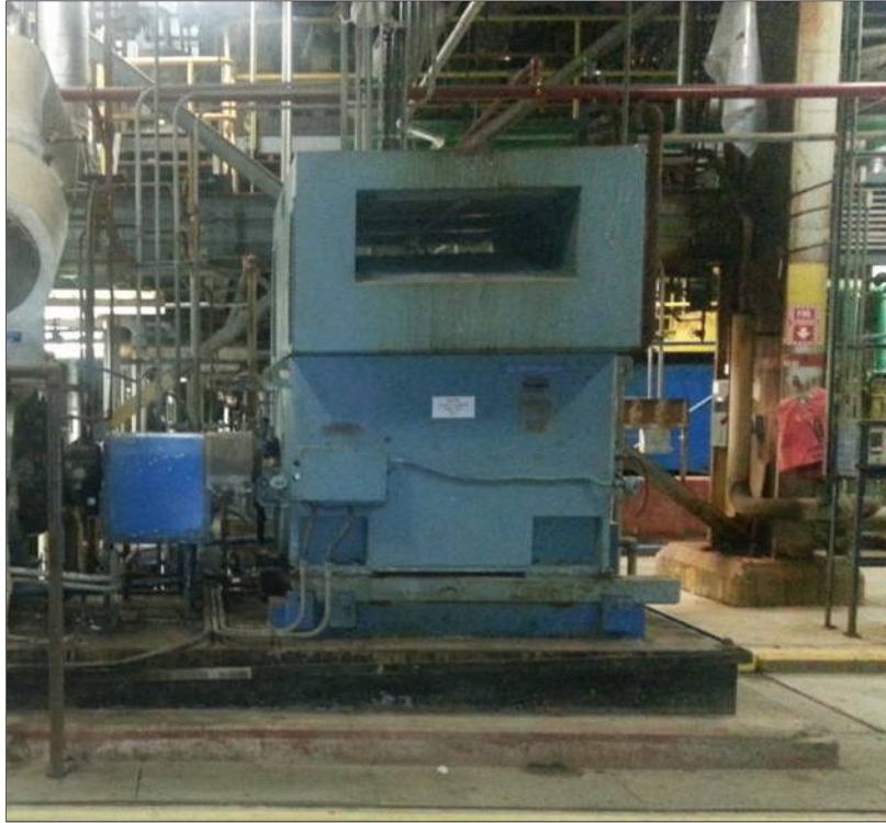
Figure 2: Holyrood Boiler Feed Pump Motor
