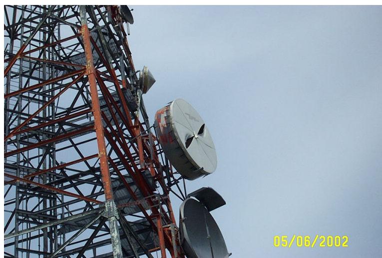
Figure 3: Heavily Damaged Radome
