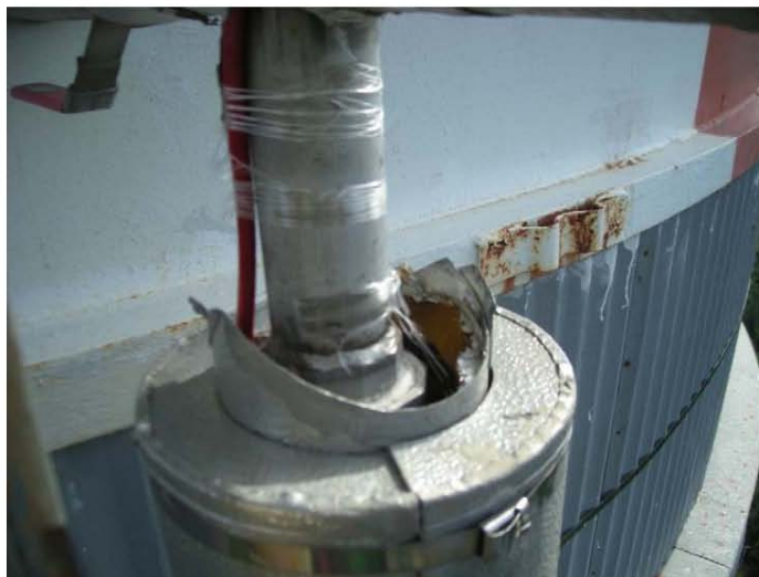
Figure 5-6: Top of Hot Water Heating System Piping Insulation
