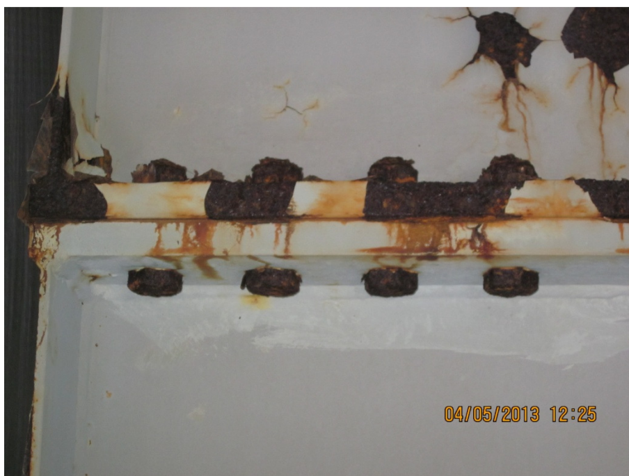
Figure 2: Corrosion on Bolted Connection
