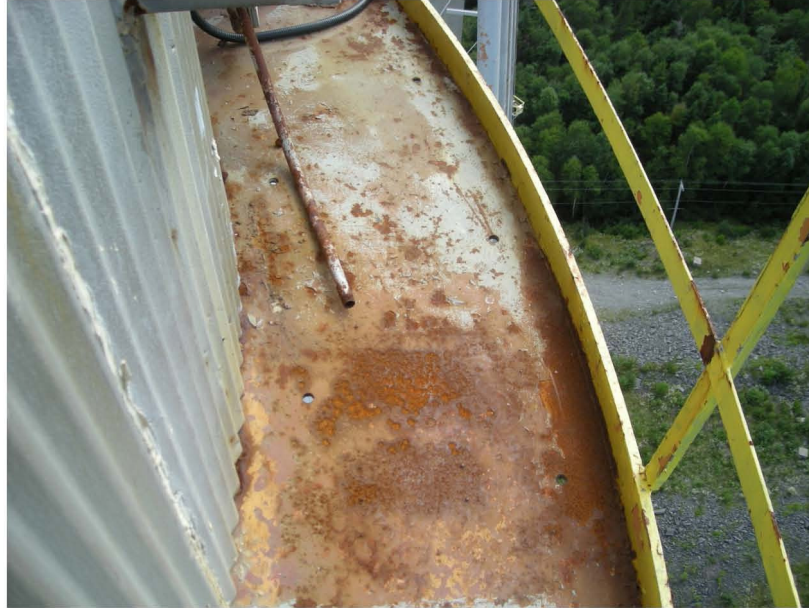
Figure 4-6: Compression Ring / Upper Balcony
