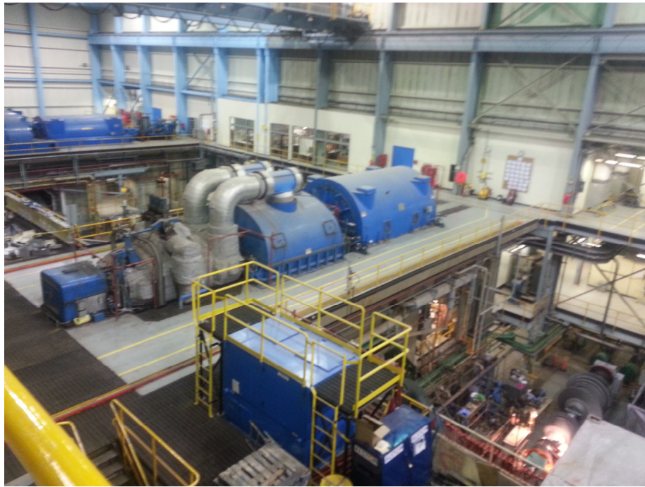
Figure 1: Unit 2 Turbine Generator Assembled
