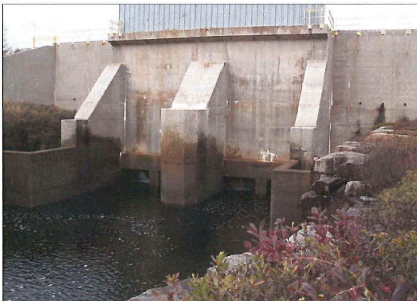
Photo 98: Victoria - Downstream View of Victoria Control Structure - Notice Leakage from Gates
