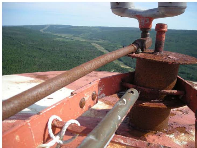
Figure 5-11: Tank Top Obstruction Lighting Conduit
