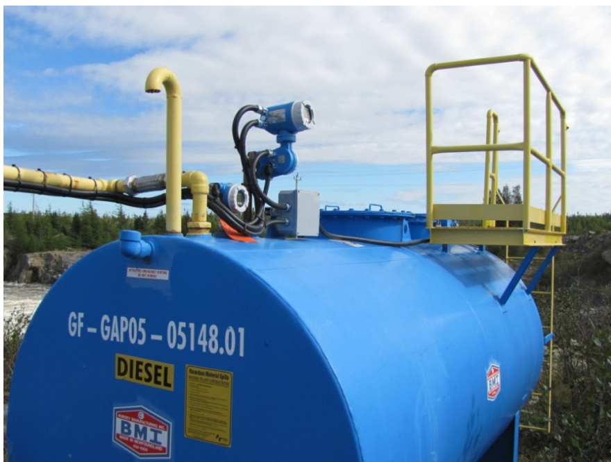
Photo 2: Ebbegunbaeg Main Fuel Tank with New Monitoring Devices
