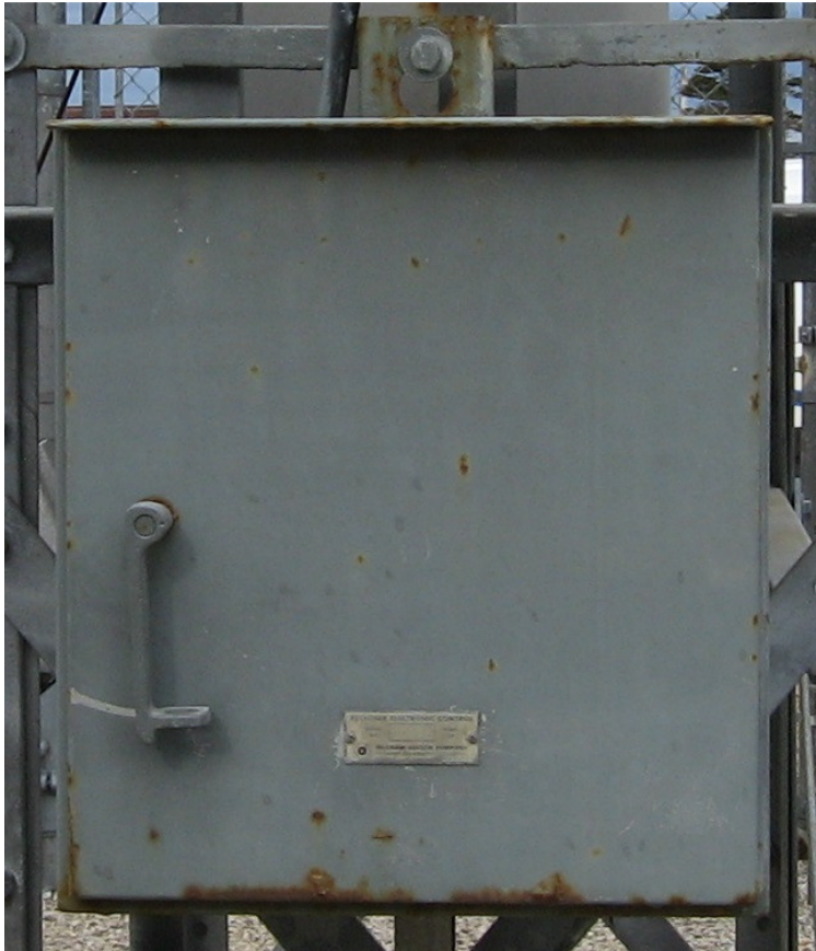
Figure 1: Hawke's Bay HB3-R2 Recloser Control Cabinet
