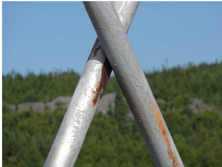
Figure 4-14: Cross Member Showing Signs of Wear
