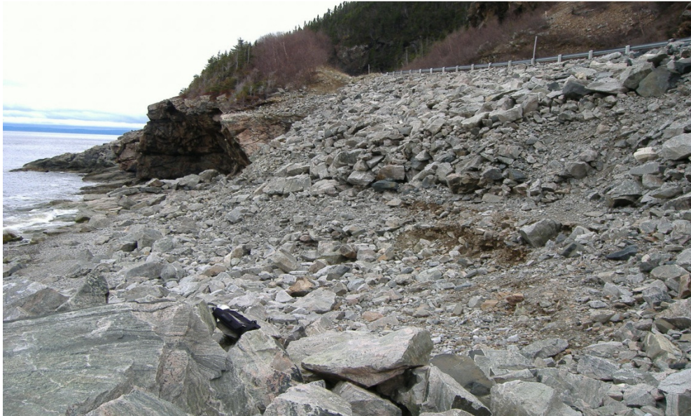
Figure 2: Eroded Section of Road Embankment
