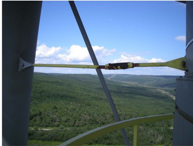
Figure 4-10: Erection Rods on Lower Balcony
