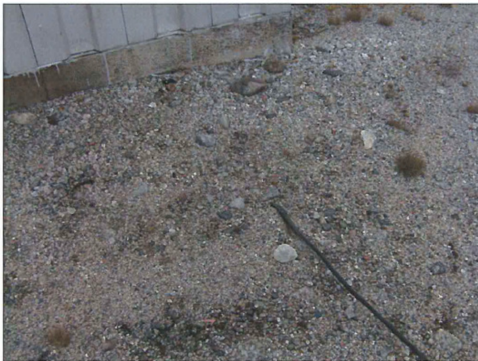
Photo 108: Victoria Control Structure - Exposed Grounding Conductors
