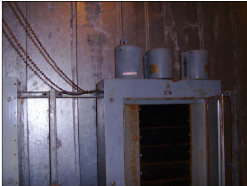
Photo 116: Victoria Control Structure - Lighting Ballasts
