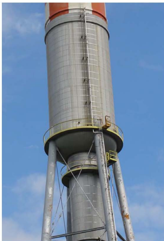
Figure 4-4: Surge Tank Shell and Top of Riser External Insulation
