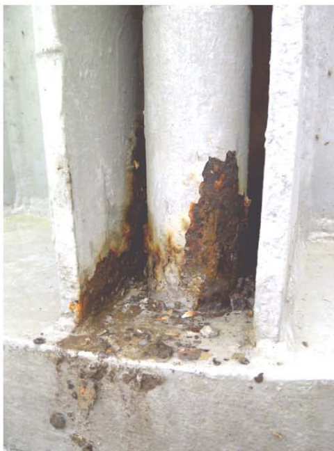
Figure 4-18: Corroded Anchor Bolt on North Leg Foundation
