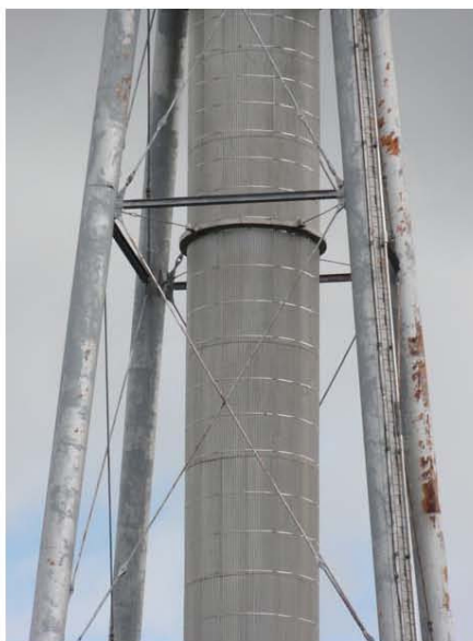
Figure 4-12: Structural Support Showing Coating Breakdown
