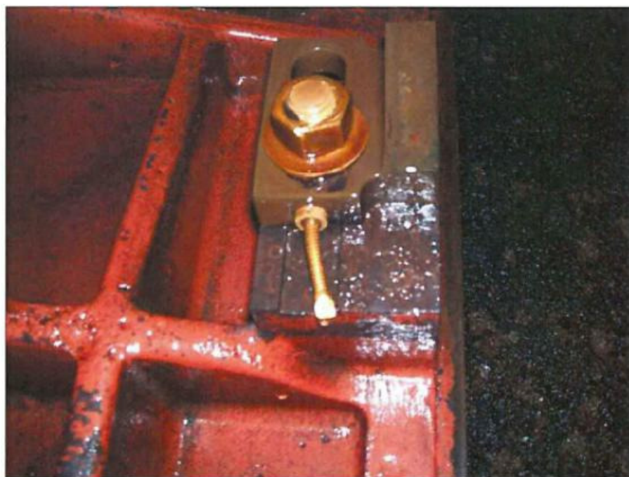
Photo 101: Bent Wedge Set Screw on Victoria Control Gate 2
