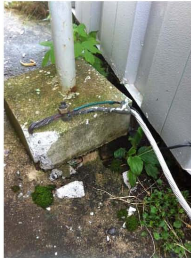
Figure 5-9: Electrical Grounding Connection
