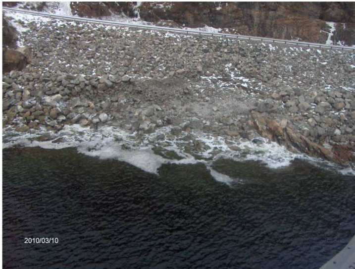
Erosion area March 10, 2010 with larger armour stone remaining at the shoreline.
