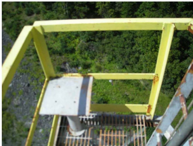
Figure 4-11: Lower Rest Platform (Crow's Nest)
