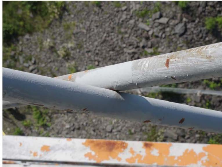
Figure 4-13: Typical Cross Member with Very Little Wear Present
