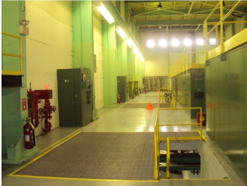
Figure 2: Deluge Valve (left) with respect to Generating Unit (right)
