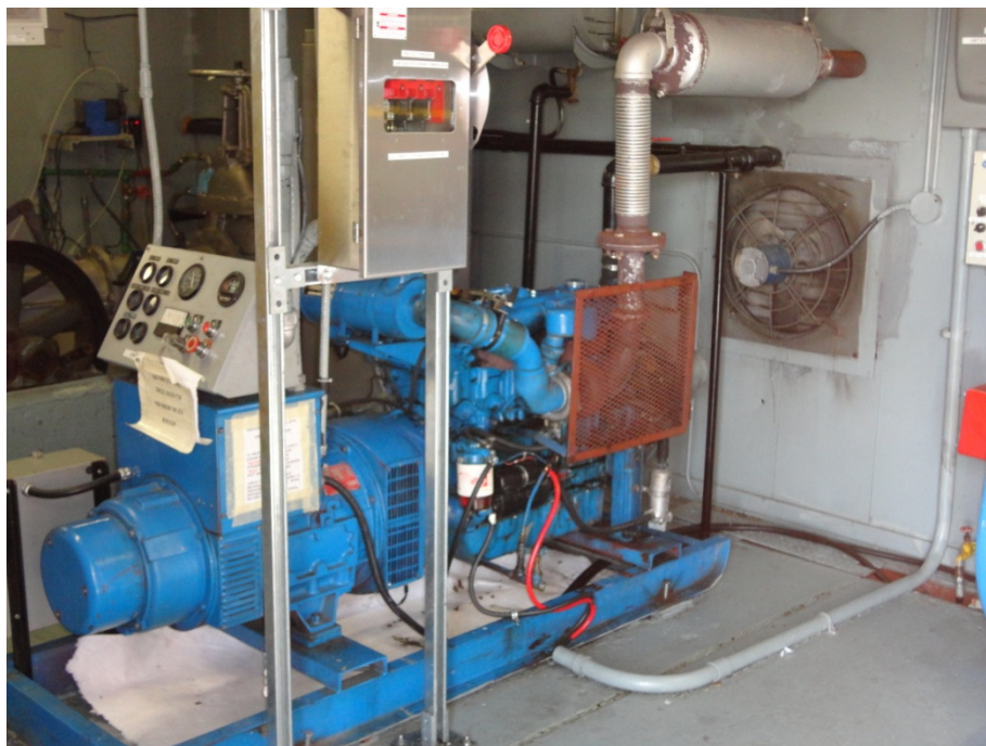
Figure 4: 75 kW Diesel Generator Set
