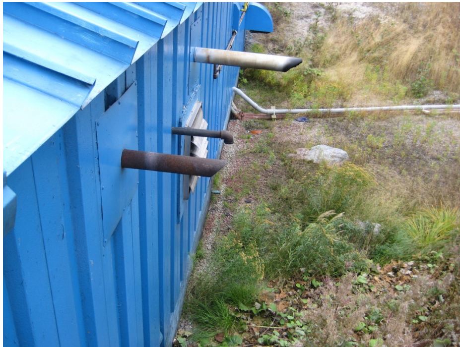
Figure 6: Cable Penetrations, Exhaust Stacks and Intake/Exhaust Vents
