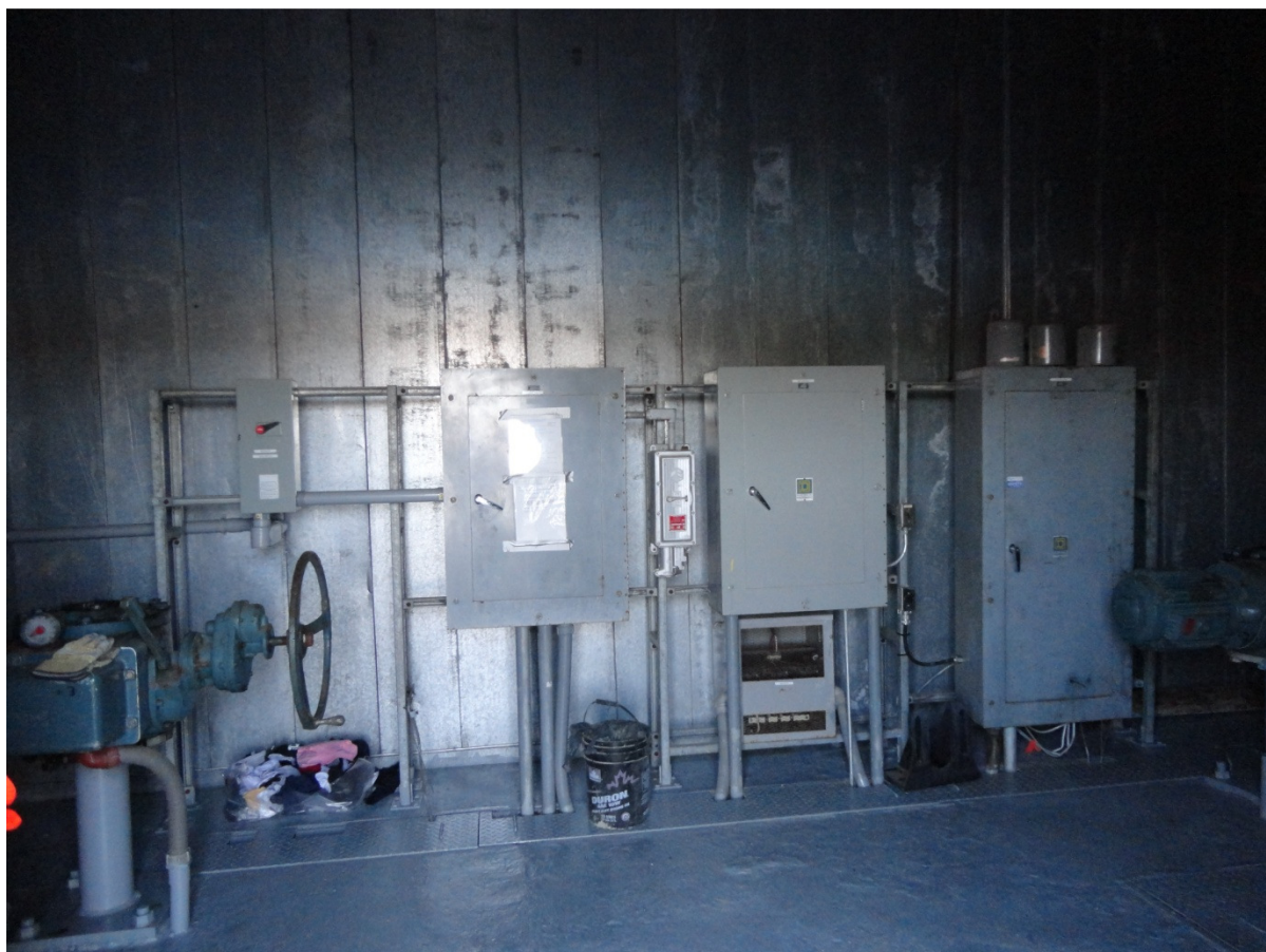
Figure 3: Victoria Control Structure - Electrical Panels and Power Cables
