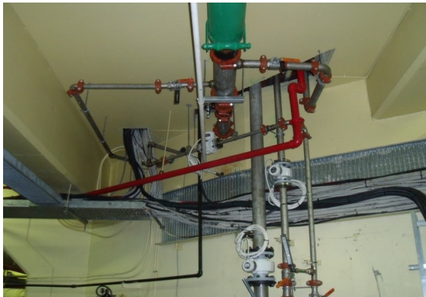
Figure 3: New Electromagnetic Flow meters at Cat Arm
