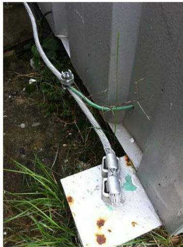
Figure 5-8: Electrical Grounding Connection
