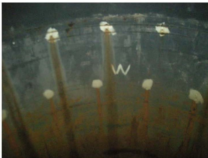
Figure 3-3: Tank Shell Interior at Mid-height Near Hot Water Heating System Inlets
