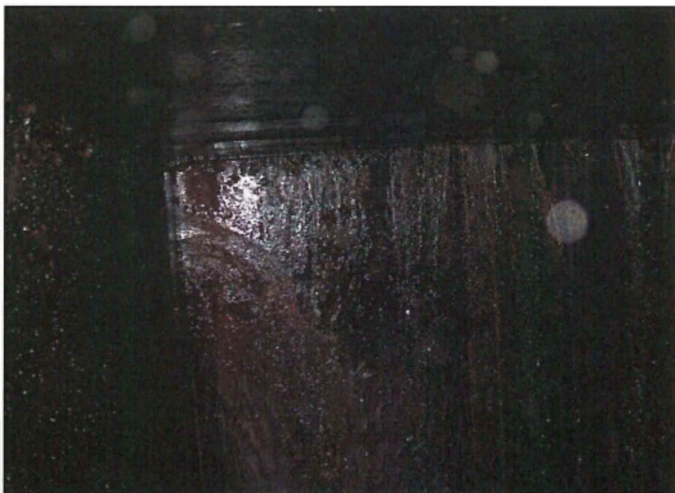
Photo 105: Leakage Past Bulkhead Gates Upstream of Victoria Control Gates 3 and 4
