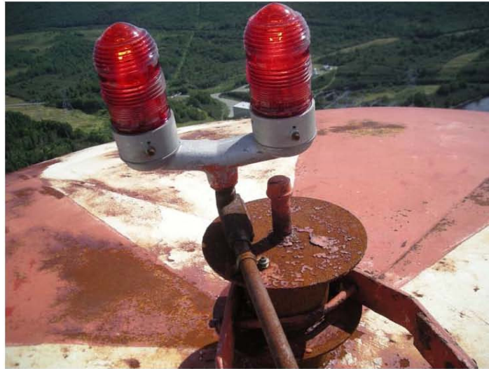
Figure 5-10: Tank Top Obstruction Lighting
