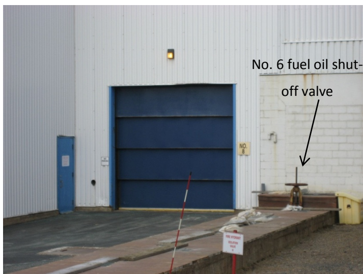
Figure 2: No. 6 Fuel Oil Shut-off Valve
