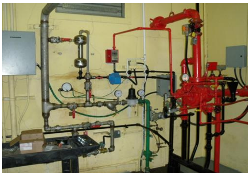
Figure 1: Existing Orifice Plate Flow Meters at Upper Salmon
