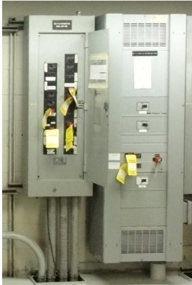
Figure 1: Unit 1 129 V and 258 V DC panels locked out and tagged
