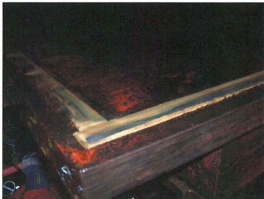
Photo 100: View of Brass Seals on Victoria Control Gate 2
