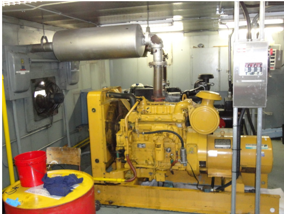
Figure 5: 25 kW Diesel Generator Set
