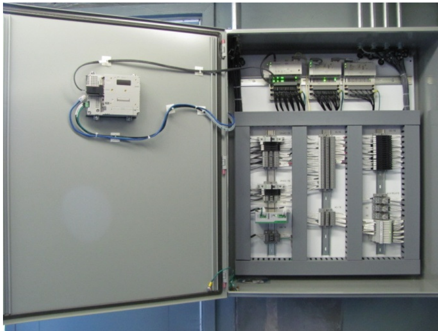
Photo 4: Ebbegunbaeg Automated Fuel Monitoring System Cabinet (door open)
