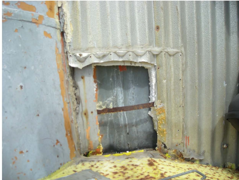
Figure 4-3: Cladding Removed Adjacent to Leg
