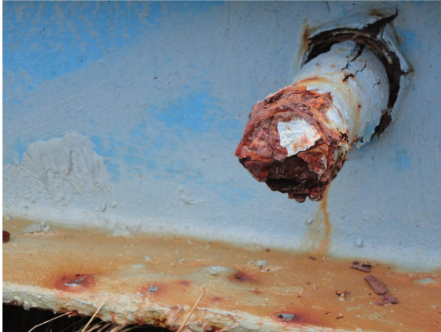
Figure 1: Corroded Dyke Drain Valve
