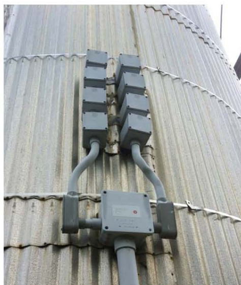
Figure 5-2: Cathodic Protection System on Tank Riser
