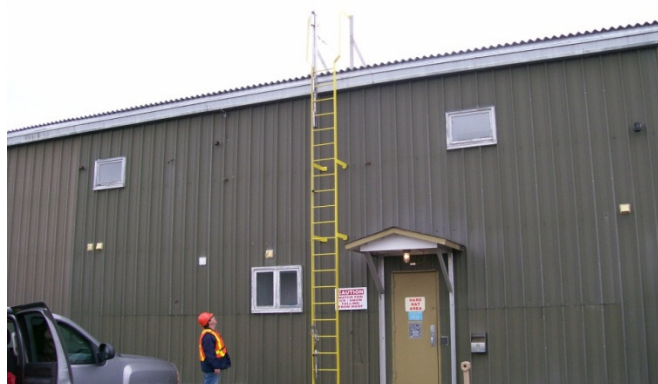
Figures 2 and 3: Ladder Fall Protection System
