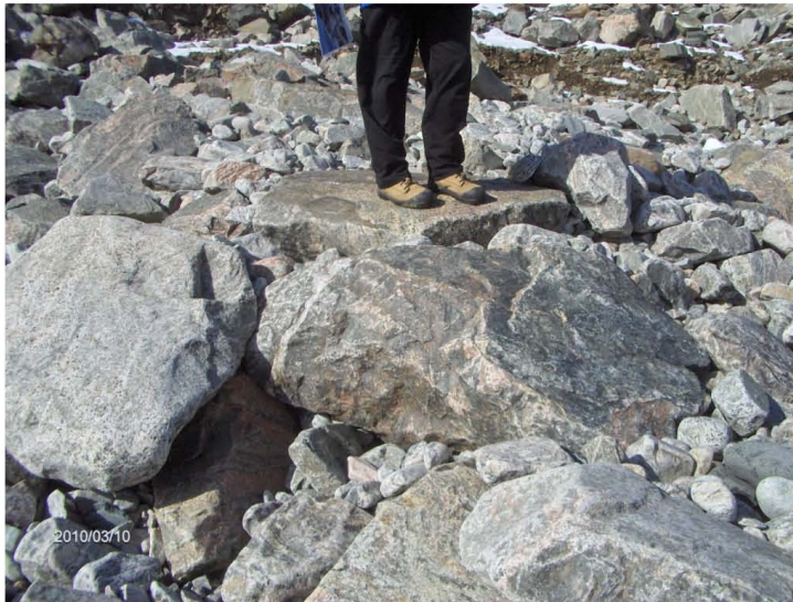
Some armour and filter stones remain in eroded area.
