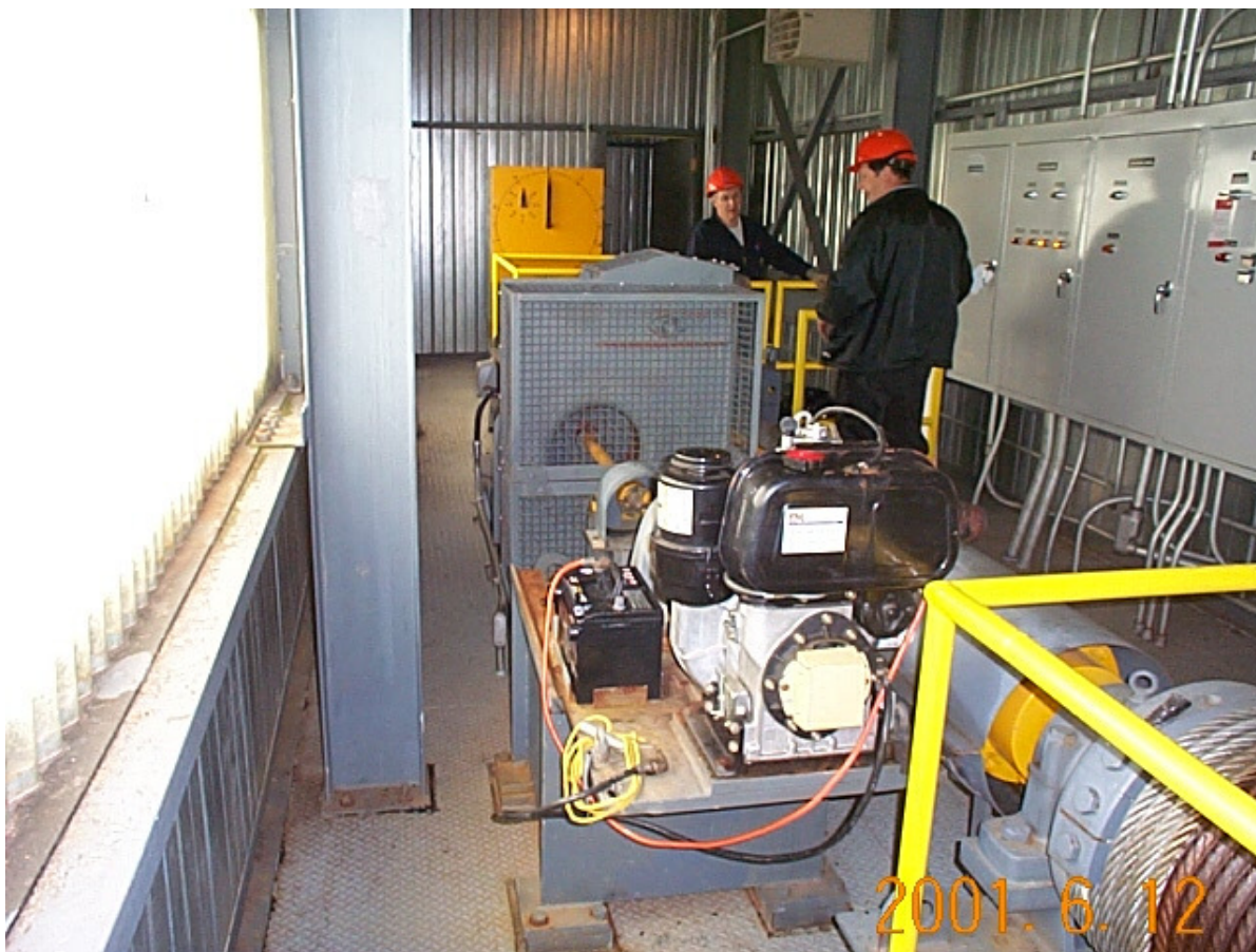
Figure 1: Diesel Engine for Emergency Drive at West Salmon Spillway
