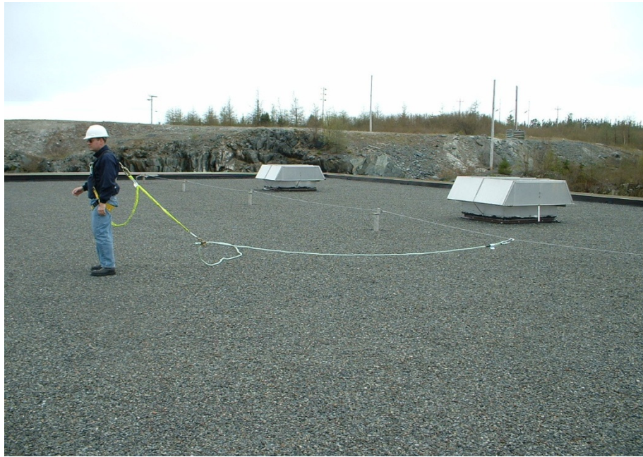
Figure 1: Roof Fall Protection System
