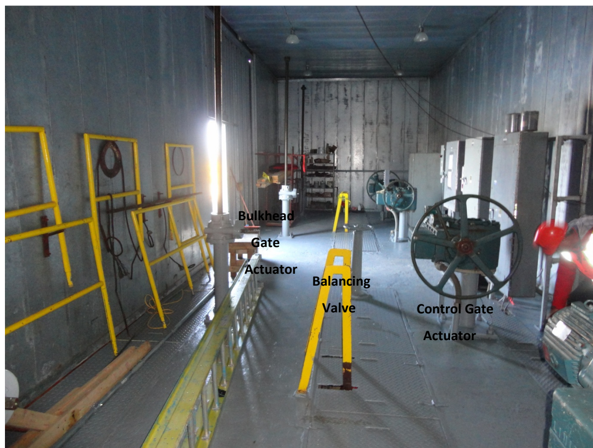
Figure 4: Victoria Control Structure – Actuators and Balancing Valve
