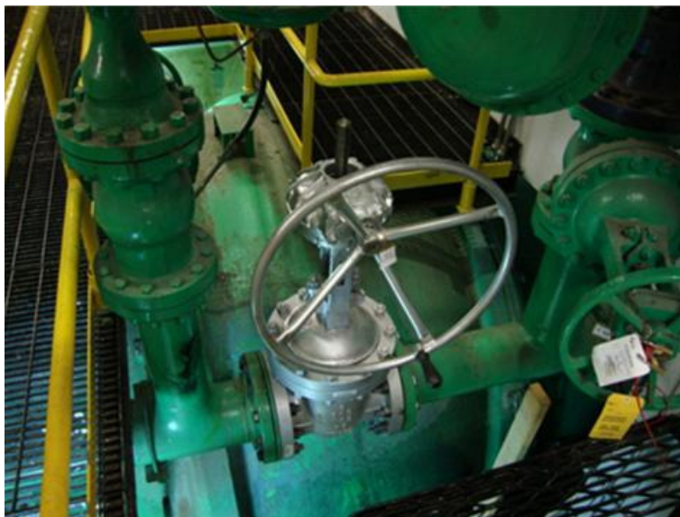
Figure 1: Spherical Valve By-Pass Assembly
