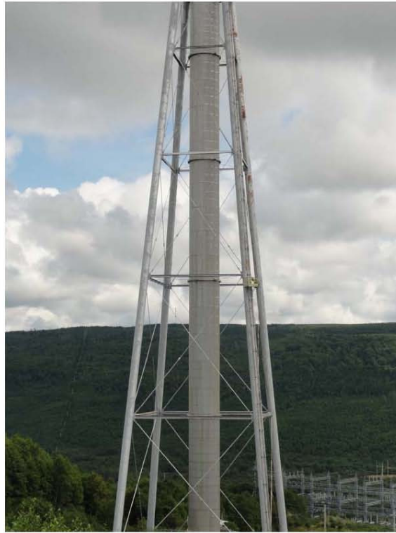
Figure 4-5: Riser and Structural Support
