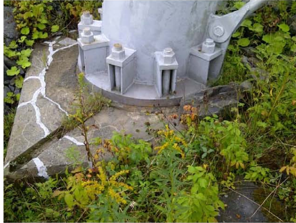
Figure 4-17: Leg Foundation and Anchor Bolt Arrangement
