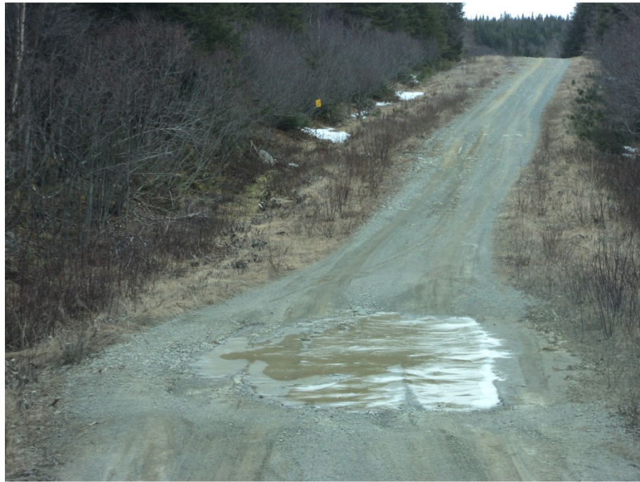
Figure 3: Inadequate Drainage
