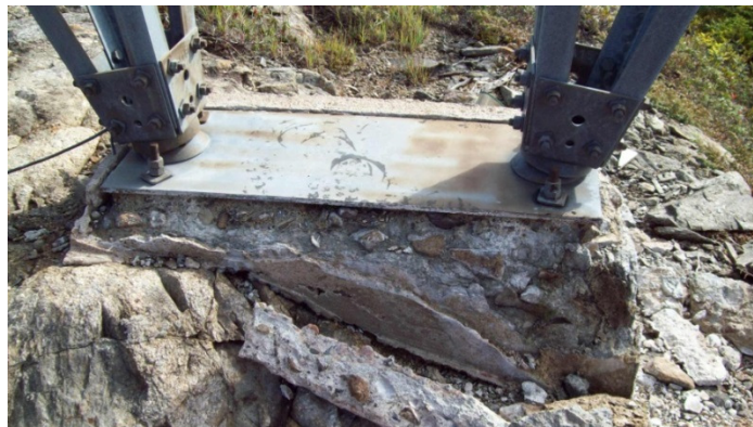
Figure 2: Deteriorated Concrete Footing on Structure 52 of TL202
