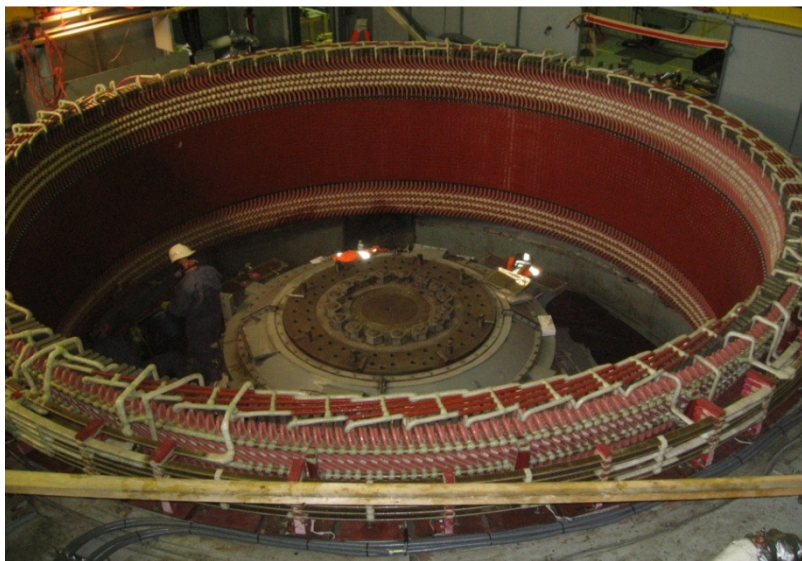
Figure 2: Stator at Bay d'Espoir with Rotor Removed
