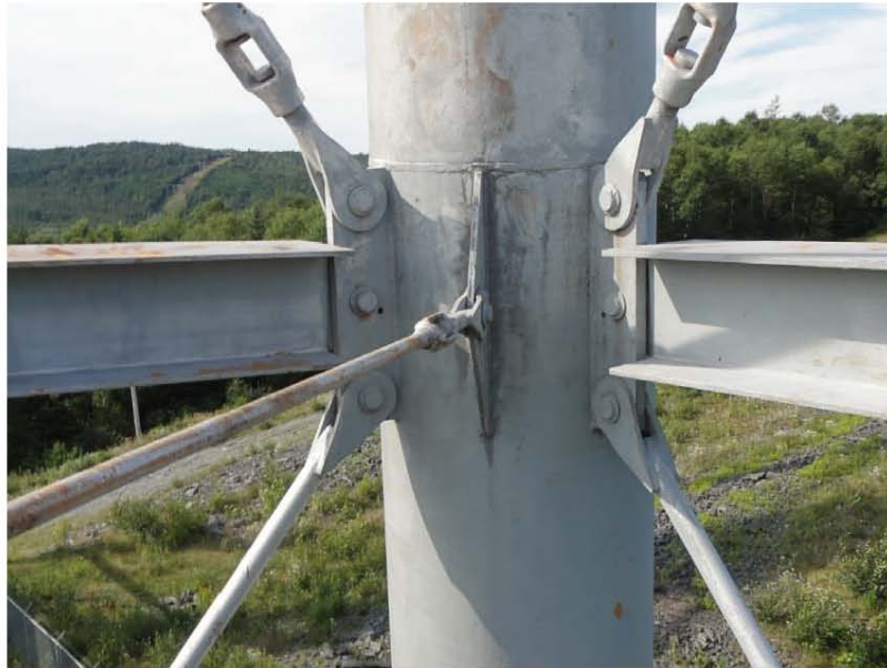
Figure 4-15: Typical Structural Support Connection
