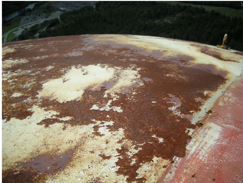
Figure 4-1: Tank Top Showing Significant Coating Breakdown
