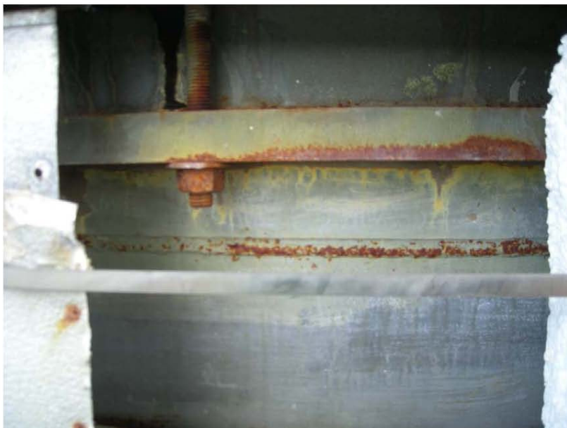
Figure 4-7: Cladding Removed Showing Expansion Joint at Lower Balcony
