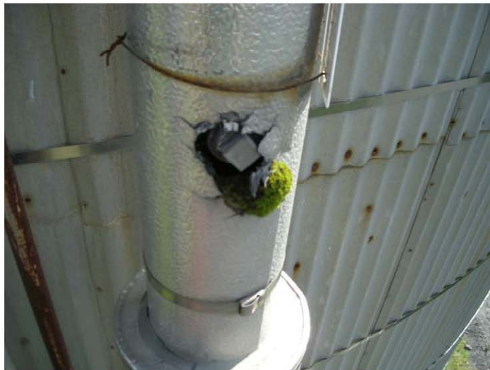
Figure 5-5: Damaged Insulation on the Hot Water Heating System Piping
