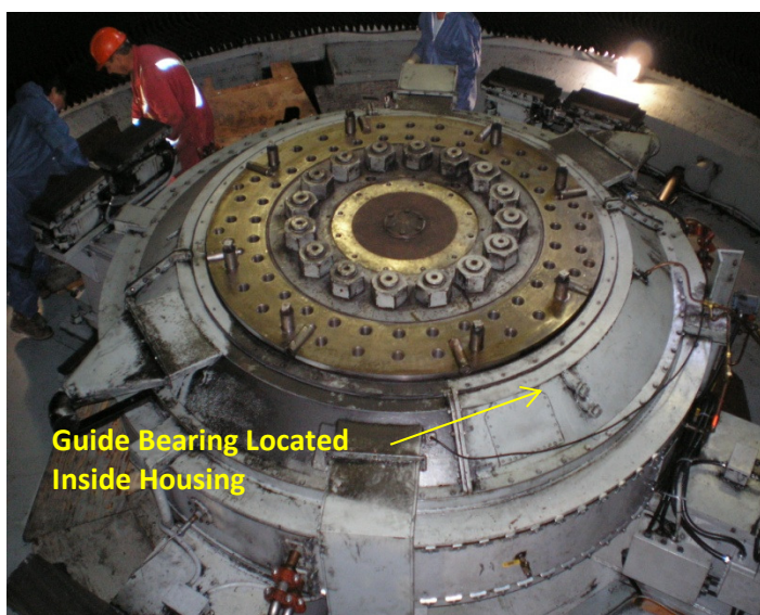
Figure 1: Generating Bearing Housing
