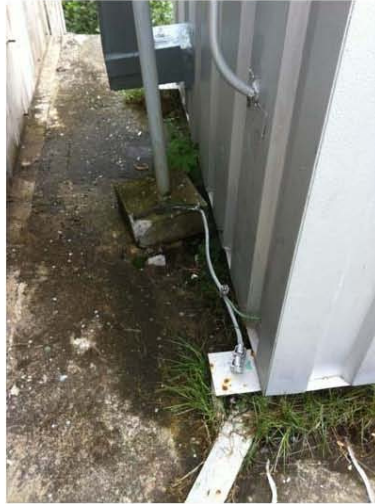
Figure 5-7: Electrical Grounding at the Electrical Shed
