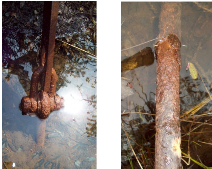
Figure 1: Corroded Anchor Rods on Structures 71 and 73 of TL202
