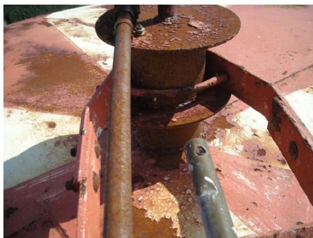
Figure 4-21: Painters Post for Ladder on Tank Top
