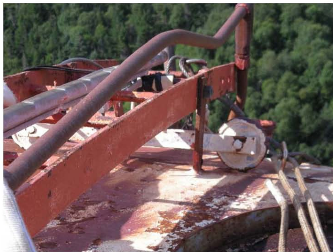
Figure 5-12: Tank Top Obstruction Lighting Conduit
