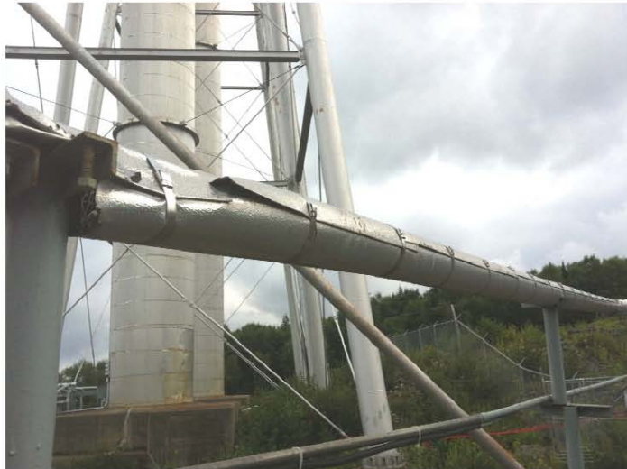
Figure 5-4: Damaged Insulation on the Hot Water Heating System Piping
