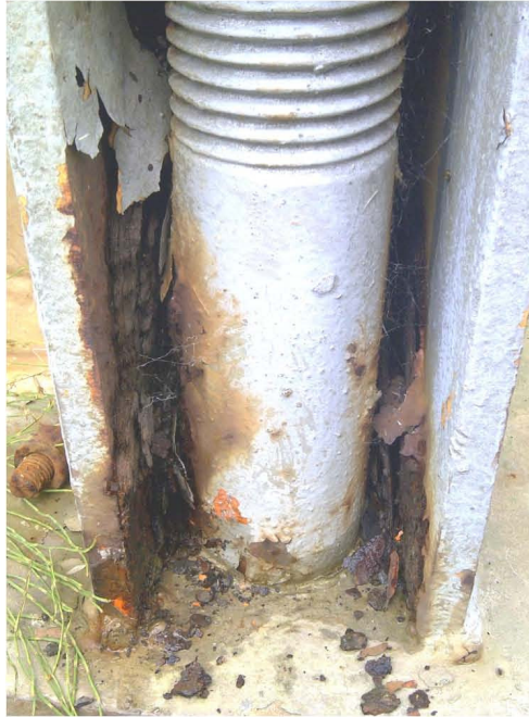
Figure 4-19: Corroded Anchor Bolt on West Leg Foundation
