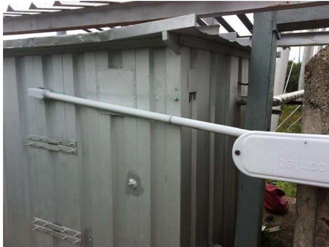
Figure 5-3: Cathodic Protection System Conduit at Electrical Shed
