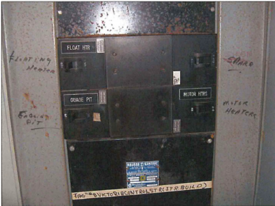
Photo 113: Victoria Control Structure - 120/240V Distribution Panel
