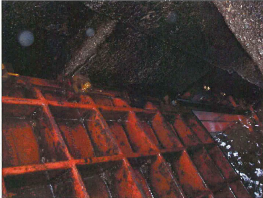
Photo 102: Victoria Control Gate 1 - Notice Missing Wedge Block in Centre of Photograph
