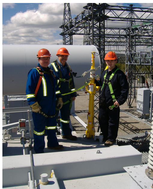
Figure 4: Transformer Fall Protection System
