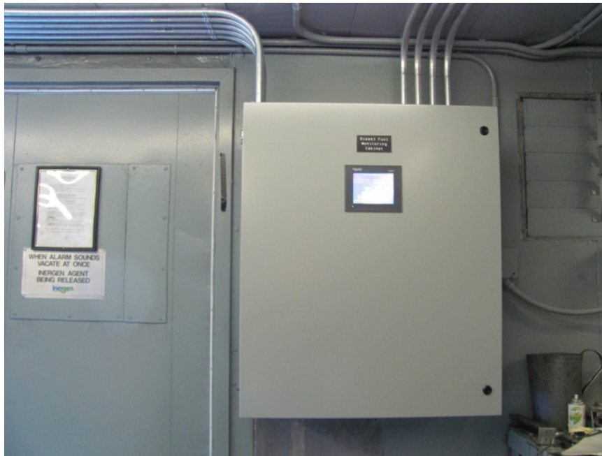
Photo 3: Ebbegunbaeg Automated Fuel Monitoring System Cabinet (door closed)
