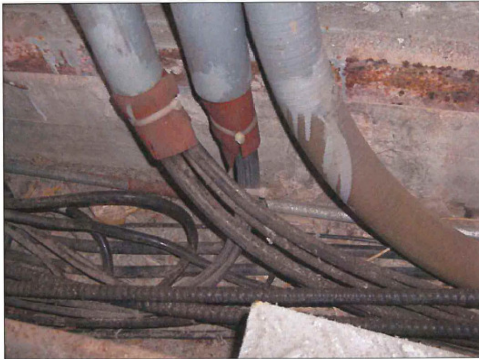
Photo 110: Victoria Control Structure - Cables Exiting Conduits
