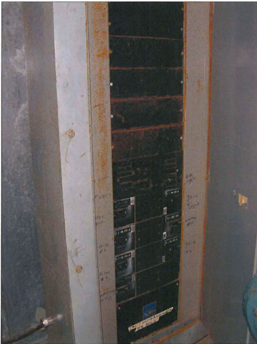
Photo 114: Victoria Control Structure - 120/208V Distribution Panel
