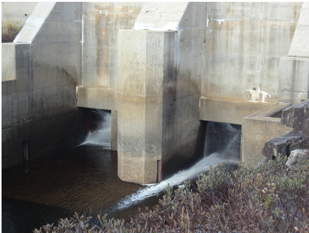
Figure 5: Victoria Control Structure – Gate Leakage
