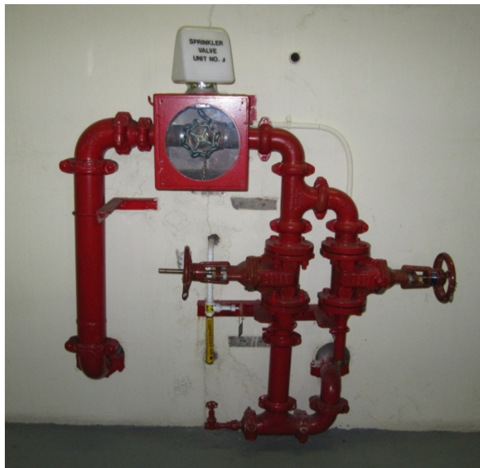
Figure 1: Typical Deluge Valve Arrangement on Units 1 – 6
