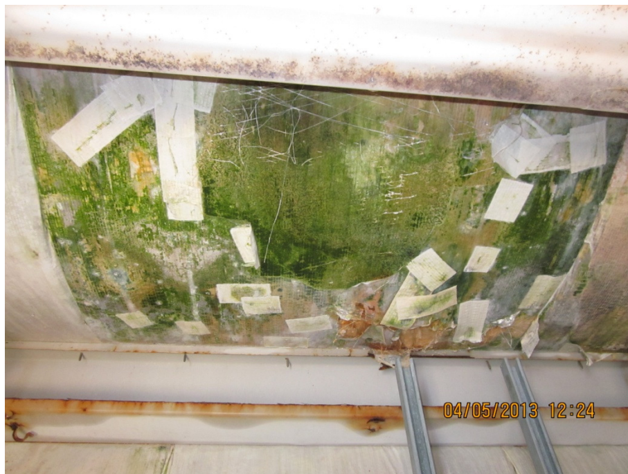
Figure 1: Mold Growth on Interior Face of Roof Insulation
