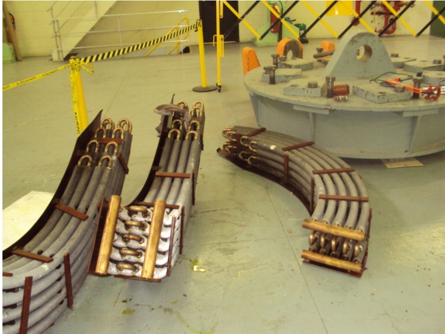
Figure 1: Bay d'Espoir Units 1- 6 – Generator Bearing Coolers
