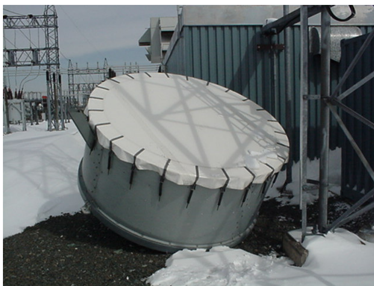
Figure 1: Microwave Antenna with Radome
