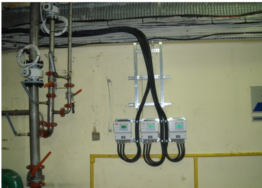
Figure 4: New Electromagnetic Flow Meters at Cat Arm
