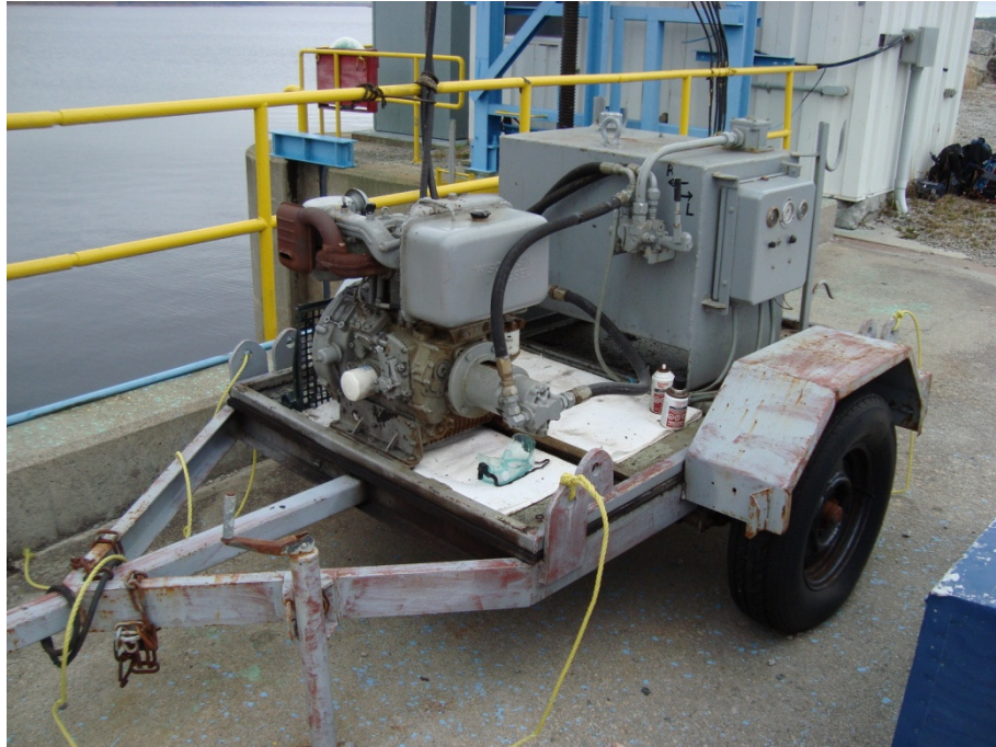
Figure 3: Portable Emergency Hydraulic Drive
