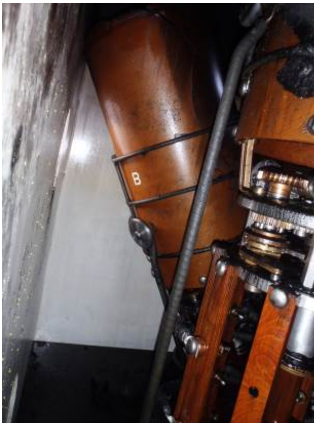
Photo 9 – LTC Compartment (Phases 2 & 3)
