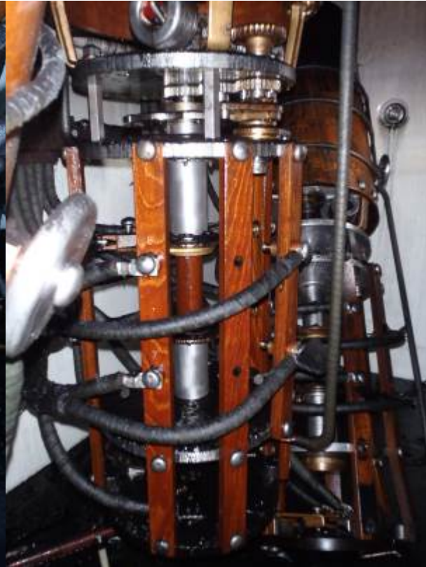
Photo 12 – LTC Compartment (Phases 2 & 1)
