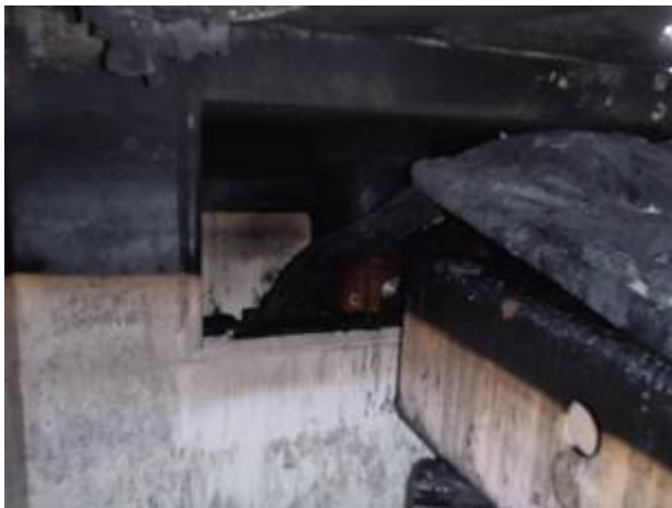
Photo 13 – Fire Line on Tank Wall & Core Clamp
