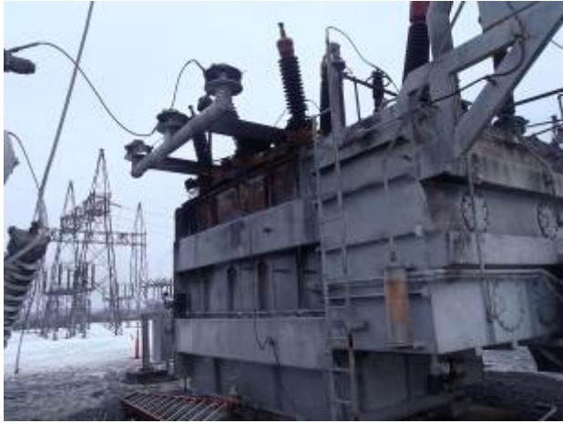
Photo 1 – Cover Open & Broken Bolts
