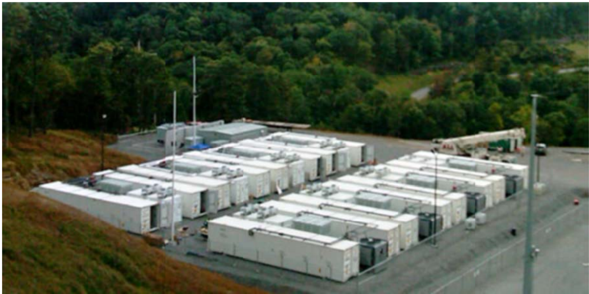
Figure 5: Laurel Mountain 32 MW, 8 MWh Lithium-ion Battery Storage near a 98 MW Wind Farm [16]
