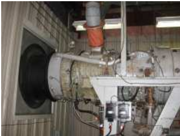
FIGURE 2-1 GTG GAS ENGINE & GENERATOR
