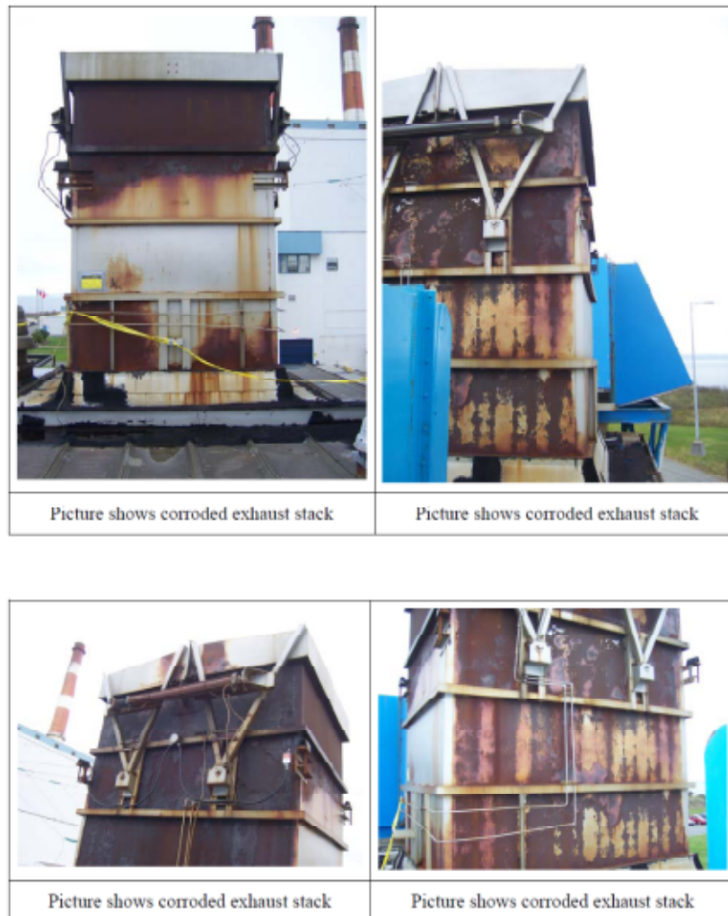
FIGURE 2-7 CORRODED EXHAUST STACK (GAS TURBINE PLANT)
