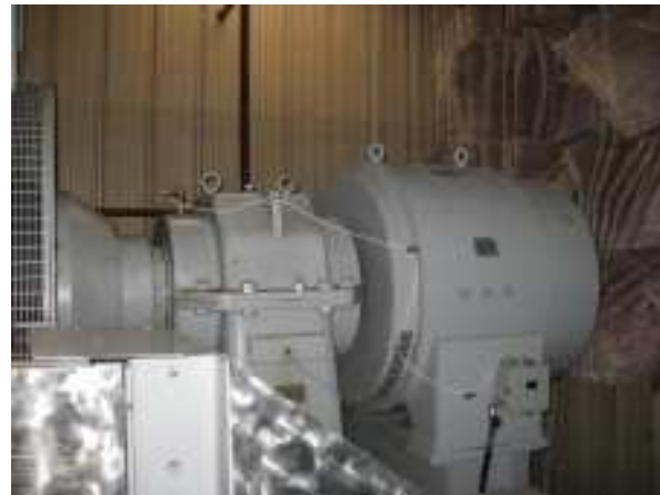
FIGURE 2-1 GTG GAS ENGINE & GENERATOR
