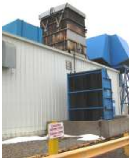
FIGURE 2-4 LIGHT OIL RECEIVING & LUBE OIL RADIATOR
