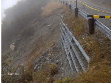
Photo 5 – Bin wall between Post 35-39, Guide Rail Section 1
