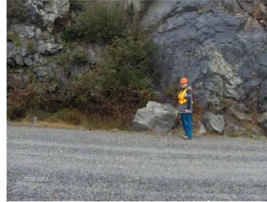
Photo 2 – Fallen rock debris at Post 0, Guide Rail Section 1
