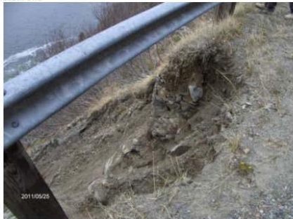
Photo 3 – Section 1, Area 2 – Erosion progressing into the driving surface of the road. Existing gabions are starting to be undermined.
