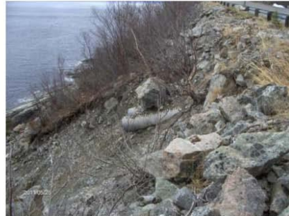
Photo 10 – Section 2, Area 3 – Eroding embankment and tilted culverts
