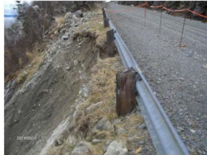
Photo 6 – Section 2, Area 1 – Continuing Erosion has Progressed to Undermining a Guiderail Post
