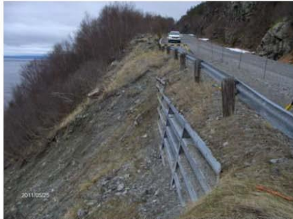
Photo 1 – Section 1, Area 1 – Bin wall showing some erosion at the south end
