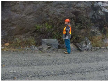
Photo 3 – Fallen rock debris at Post 20-21, Guide Rail Section 1
