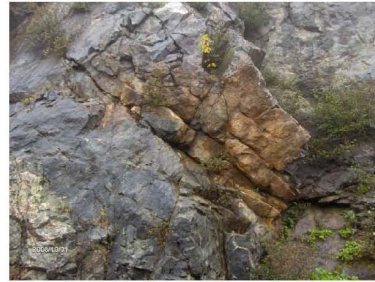
Photo 4 – Area where rock has recently fallen from the rock cut near Post 1, Guide Rail Section 1, as shown by the brown discolouration
