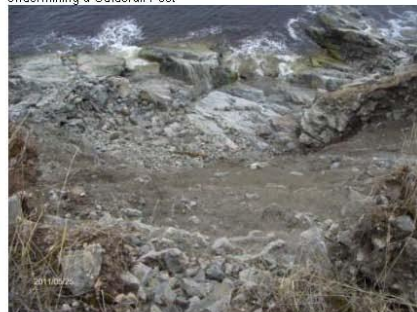
Photo 8 – Section 2, Area 2 – Beach conditions and rapidly eroding slope comprising a high proportion of sand and gravel
