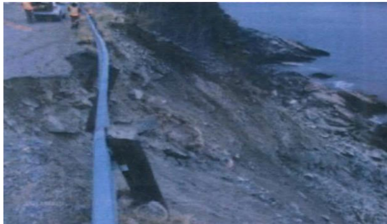
Figure 1: Embankment Erosion at Shoulder of Access Road
