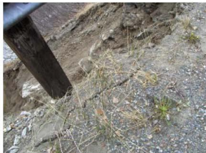
Photo 4 – Section 1, Area 2 – Tension cracks at edge of road and guiderail post suspended
