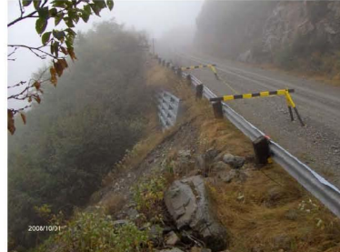
Photo 6 – Bin wall between Post 70-73, Guide Rail Section 1
