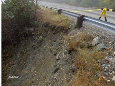
Photo 9 – Embankment erosion between Post 43-45, Guide Rail Section 2
