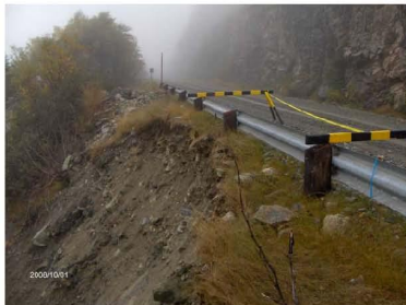
Photo 7 – Embankment erosion between Post 6-12, Guide Rail Section 2
