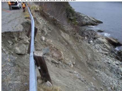
Photo 7 – Section 2, Area 2 – Erosion reaching driving surface and undermined four guiderail posts. Tension crack visible at crest of road
