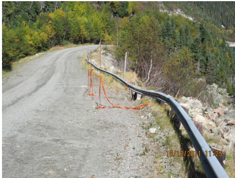
Figure 3: Barricades Erected in Vicinity of Undermined Guardrail
