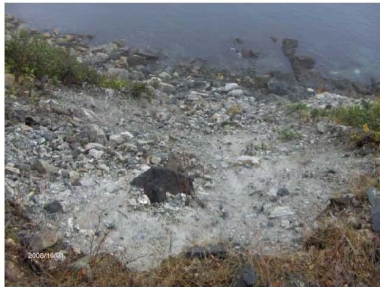
Photo 15 – Erosion gully in soil embankment, north of Guide Rail Section 3
