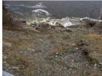
Photo 2 – Section 1, Area 1 – Erosion of the embankment
