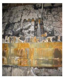
Fig. 19: Unit 2 - Missing insulation blocks
