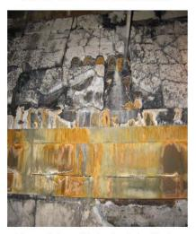
Fig. 19: Unit 2 - Missing insulation blocks
