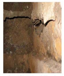
Fig. 9: Unit 1 - Duct corroded through
