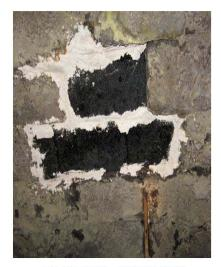
Fig. 12: Unit 1 – Replaced blocks
