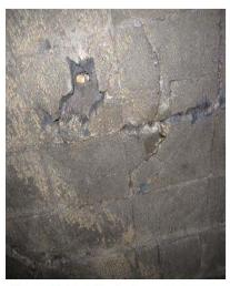
Fig. 18: Unit 2 - Missing insulation blocks
