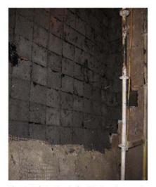
Fig. 8: Unit 1 - Insulating block replacement
