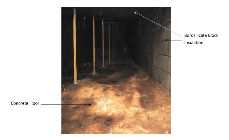
Figure 3 - Typical Stack Breeching Cross Section
