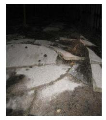
Fig. 20: Unit 2 – Cracked cement floor
