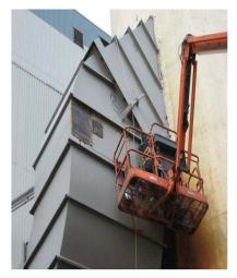
Fig. 17: Unit 1 - External duct repairs
