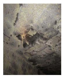
Fig. 13: Unit 1 – Missing block overhead
