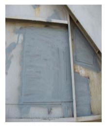
Fig. 16: Unit 1 - External duct repairs
