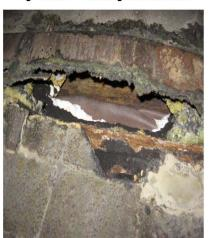
Fig. 15: Unit 1 - Damaged expansion joint
