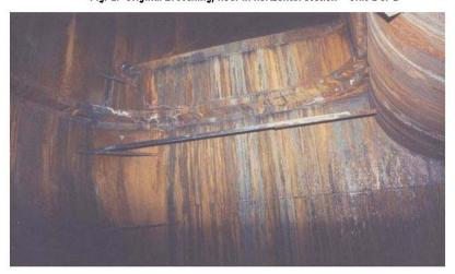
Fig. 2: Original Breeching, pantleg inlet - Unit 1 or 2
