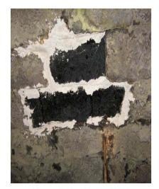
Fig. 12: Unit 1 – Replaced blocks
