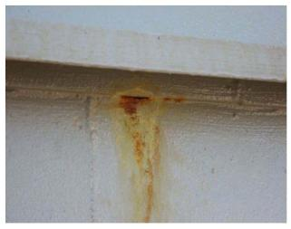
Fig. 22: Unit 2 – External coating break down
