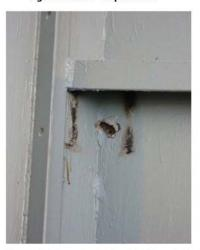
Fig. 25: Unit 3 – Patched casing (from inside)
