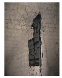
Fig. 24: Unit 3 – Crotch repairs
