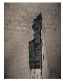
Fig. 24: Unit 3 – Crotch repairs
