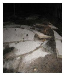
Fig. 20: Unit 2 - Cracked cement floor
