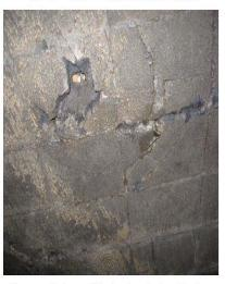
Fig. 18: Unit 2 - Missing insulation blocks
