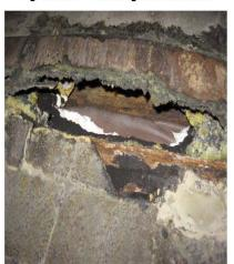
Fig. 15: Unit 1 - Damaged expansion joint
