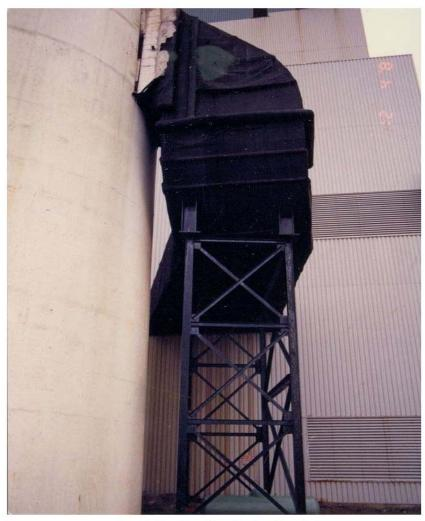
Fig. 7: Original Breeching, elevation view - Unit 1
