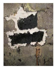
Fig. 12: Unit 1 – Replaced blocks
