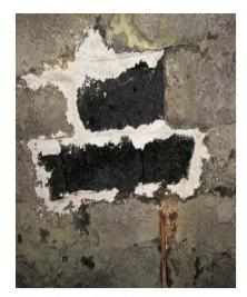
Fig. 12: Unit 1 – Replaced blocks
