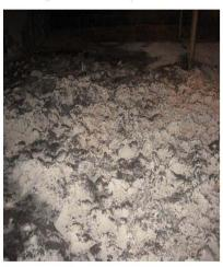
Fig.14: Unit 1 – Ash accumulated on the floor
