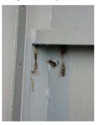
Fig. 25: Unit 3 – Patched casing (from inside)
