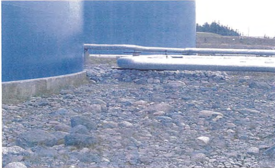
Figure No. 7 Rocks In Compound On West Side
