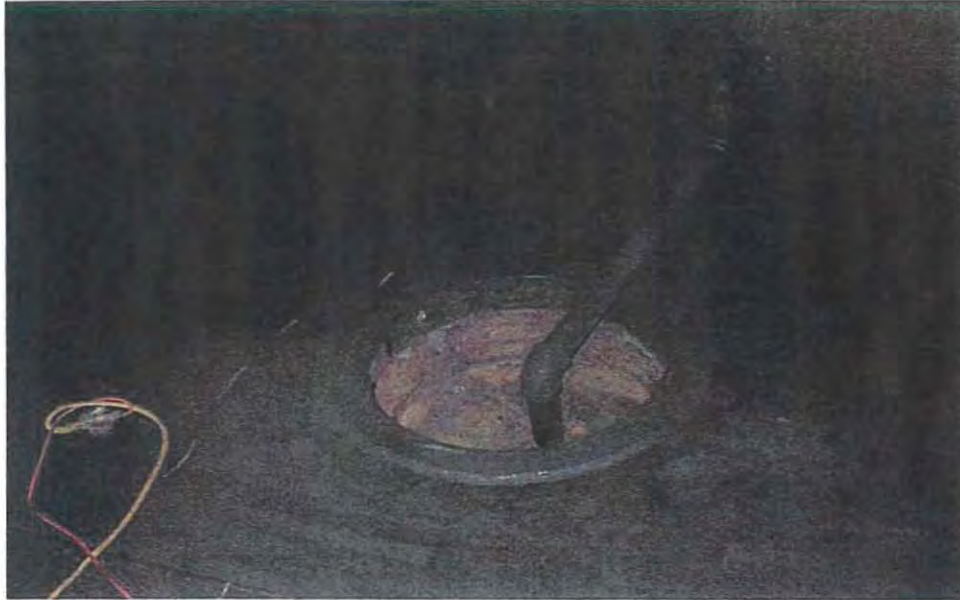
Figure No. 1 Floor sump
