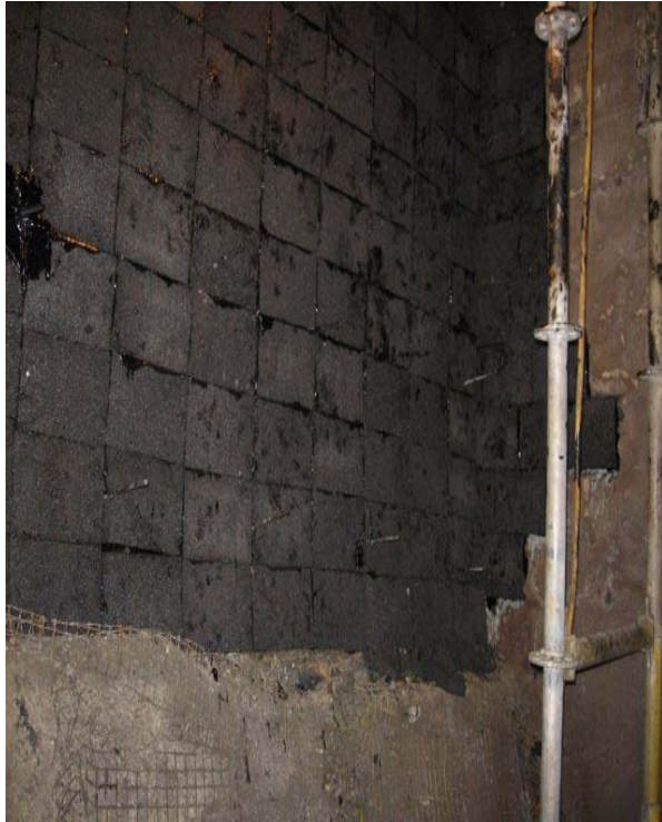
Fig. 8: Unit 1 – Insulating block replacement
