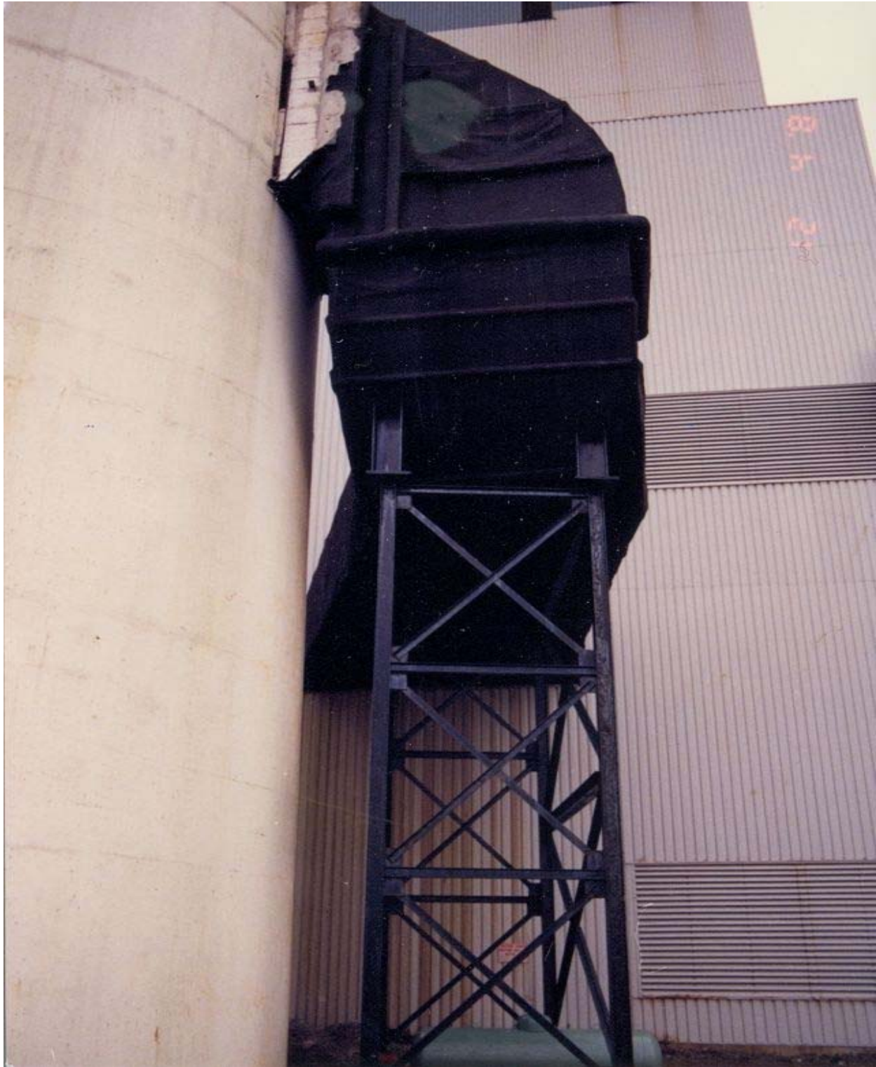
Fig. 7: Original Breeching, elevation view – Unit 1
