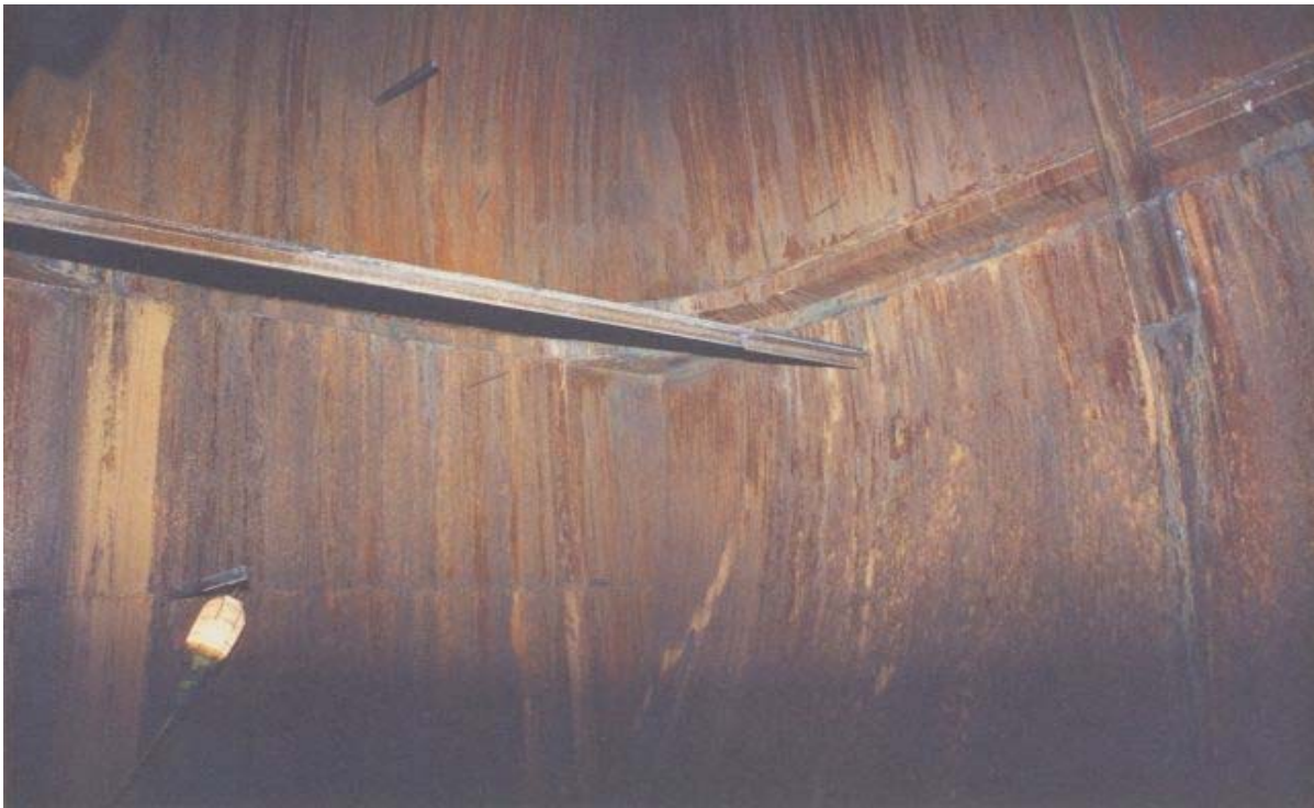
Fig. 4: Original Breeching, bend section – Unit 1 or 2
