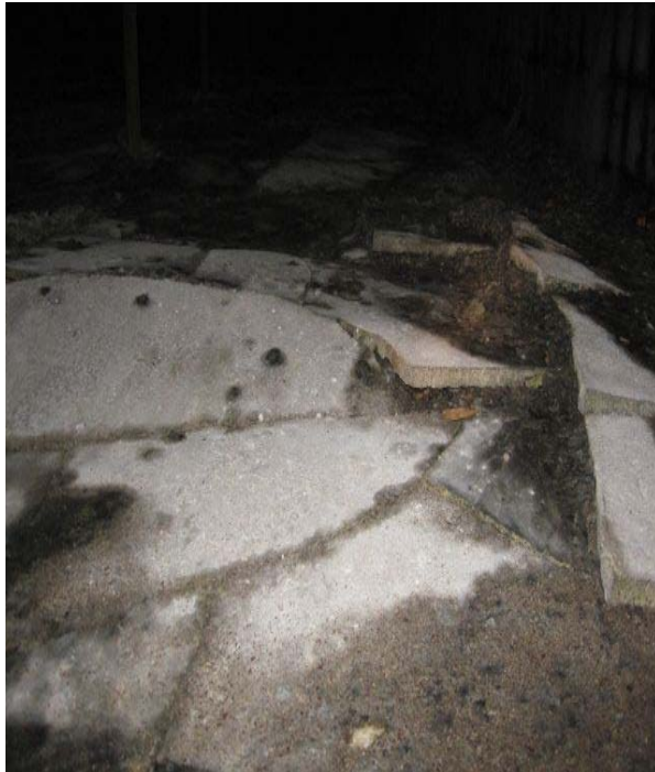
Fig. 20: Unit 2 – Cracked cement floor
