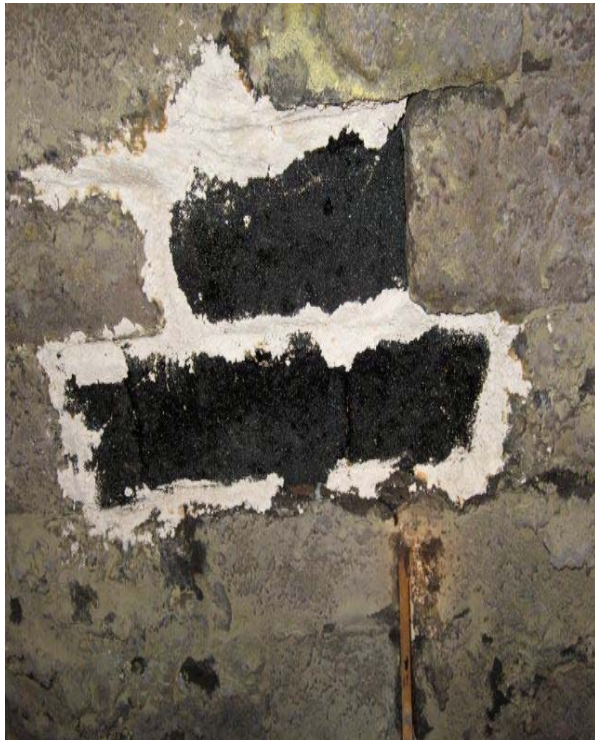
Fig. 12: Unit 1 – Replaced blocks
