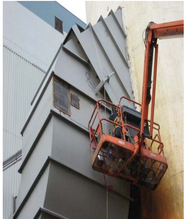
Fig. 17: Unit 1 – External duct repairs
