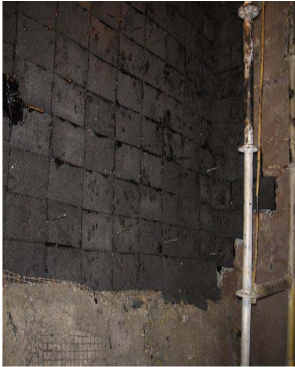
Fig. 8: Unit 1 – Insulating block replacement
