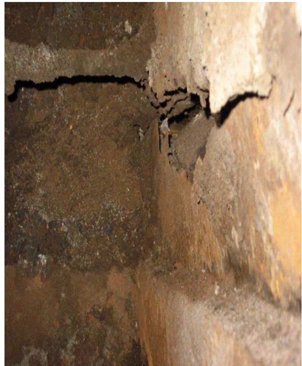
Fig. 9: Unit 1 – Duct corroded through
