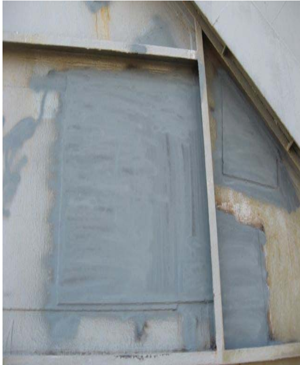
Fig. 16: Unit 1 – External duct repairs
