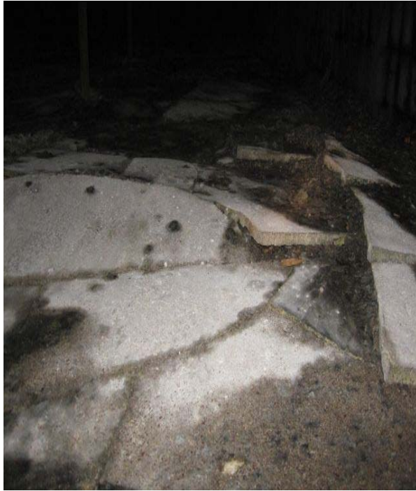
Fig. 20: Unit 2 – Cracked cement floor
