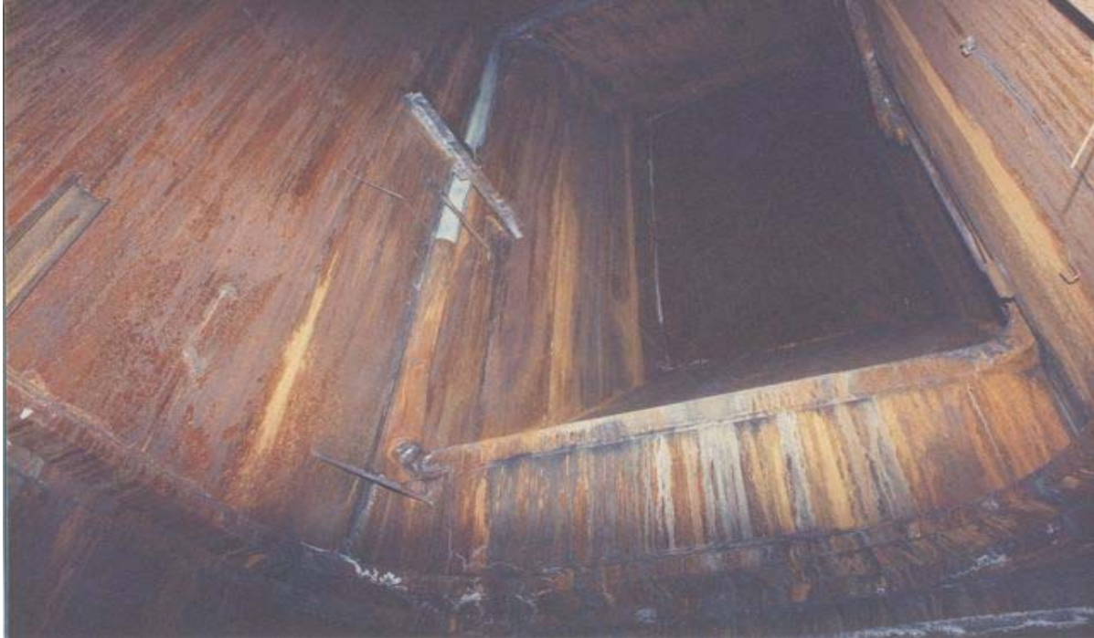
Fig. 3: Original Breeching, sloping section – Unit 1 or 2
