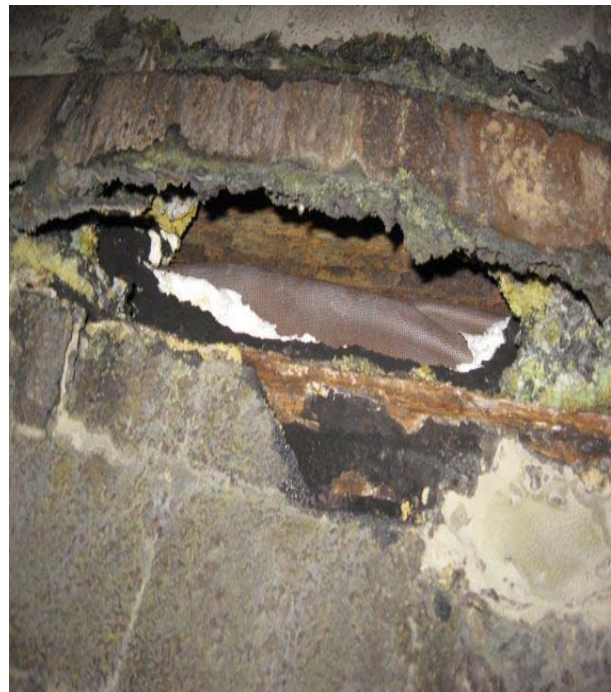
Fig. 15: Unit 1 – Damaged expansion joint
