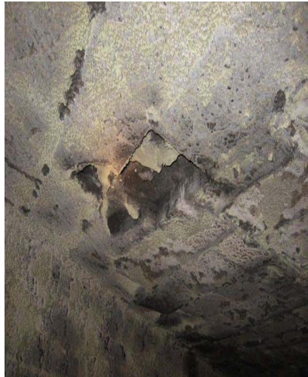
Fig. 13: Unit 1 – Missing block overhead
