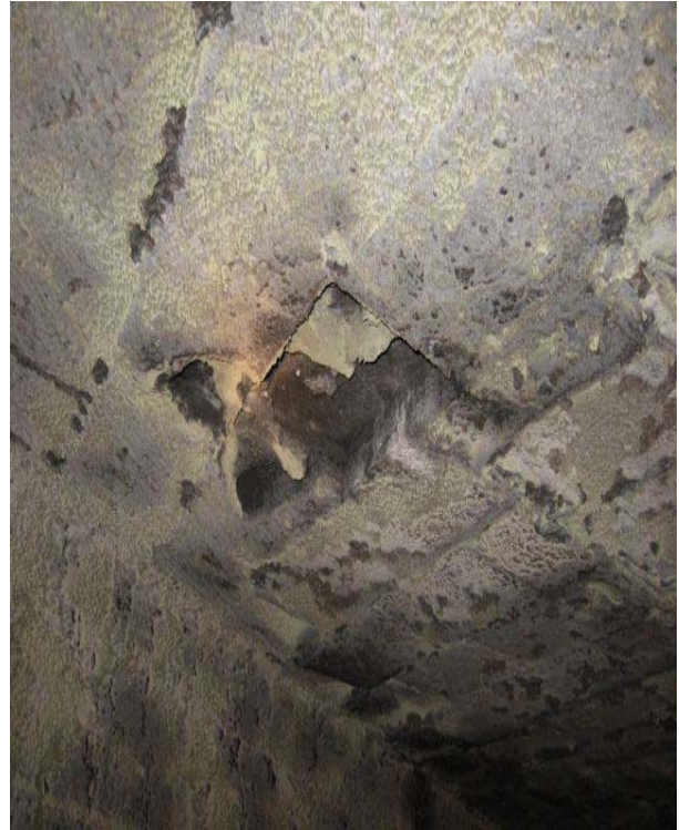
Fig. 13: Unit 1 – Missing block overhead
