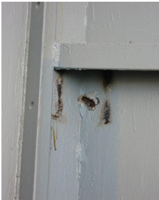
Fig. 25: Unit 3 – Patched casing (from inside)
