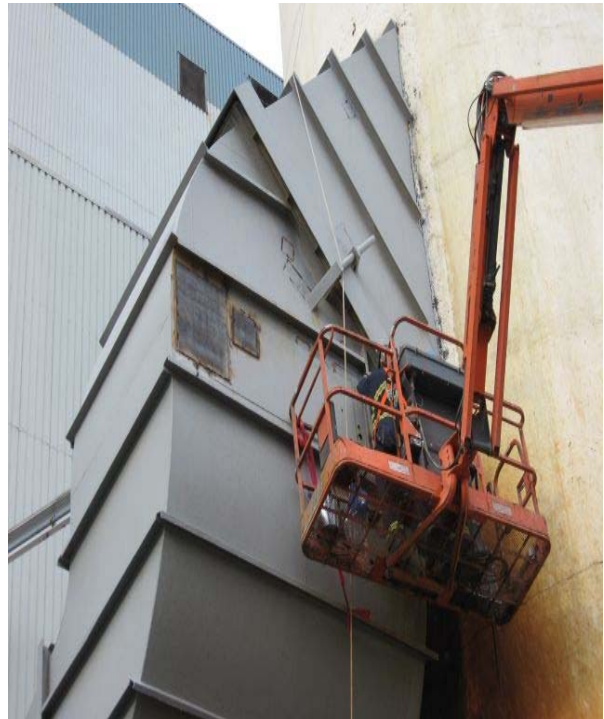
Fig. 17: Unit 1 – External duct repairs
