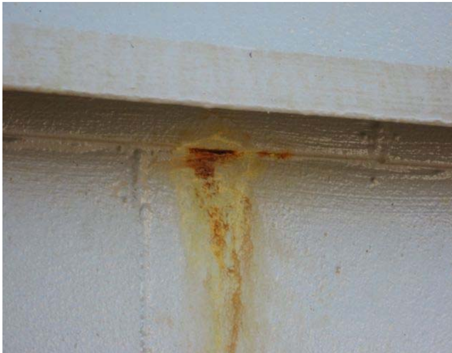
Fig.22: Unit 2 – External coating break down
