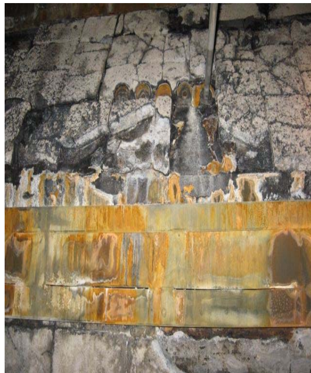
Fig. 19: Unit 2 – Missing insulation blocks
