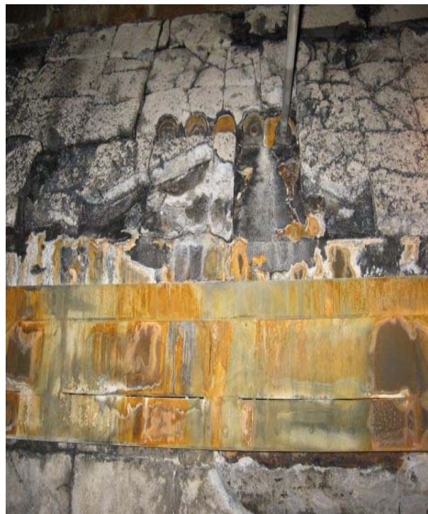
Fig. 19: Unit 2 – Missing insulation blocks
