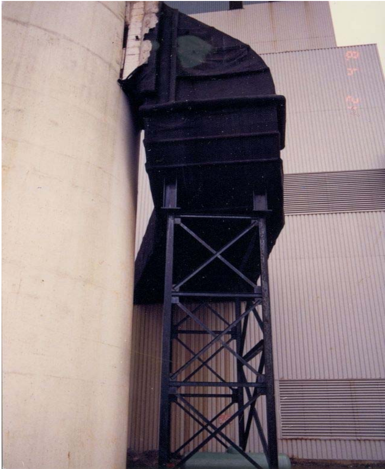
Fig. 7: Original Breeching, elevation view – Unit 1
