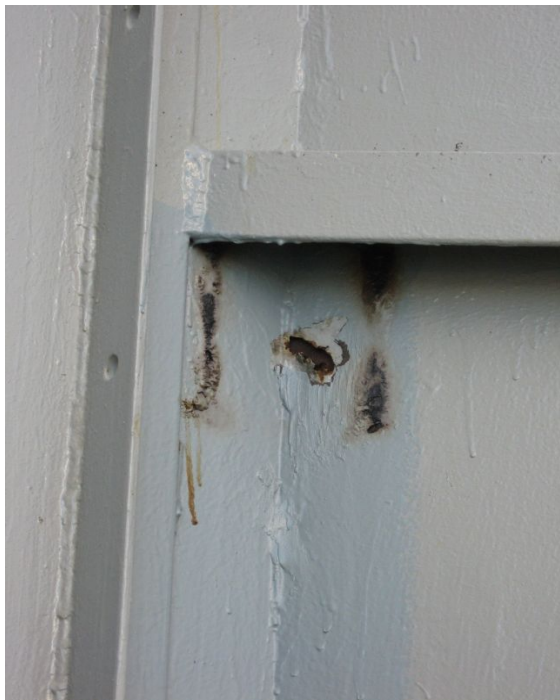
Fig. 25: Unit 3 – Patched casing (from inside)
