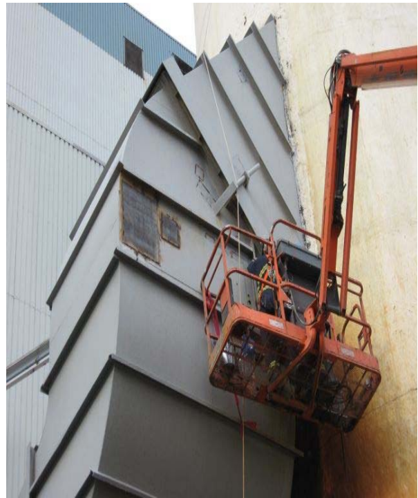
Fig. 17: Unit 1 – External duct repairs
