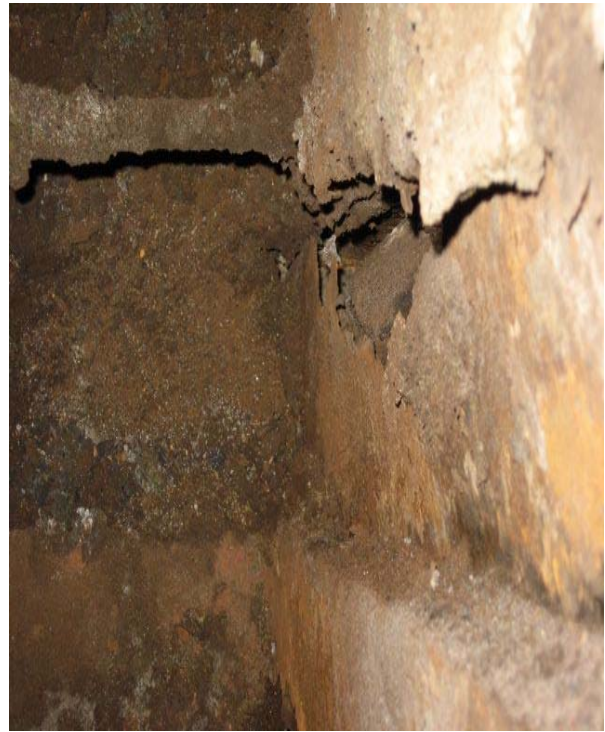
Fig. 9: Unit 1 – Duct corroded through
