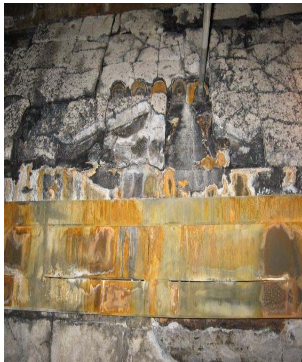
Fig. 19: Unit 2 – Missing insulation blocks
