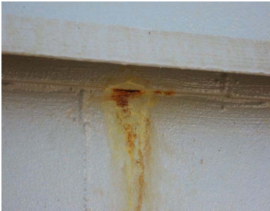
Fig.22: Unit 2 – External coating break down
