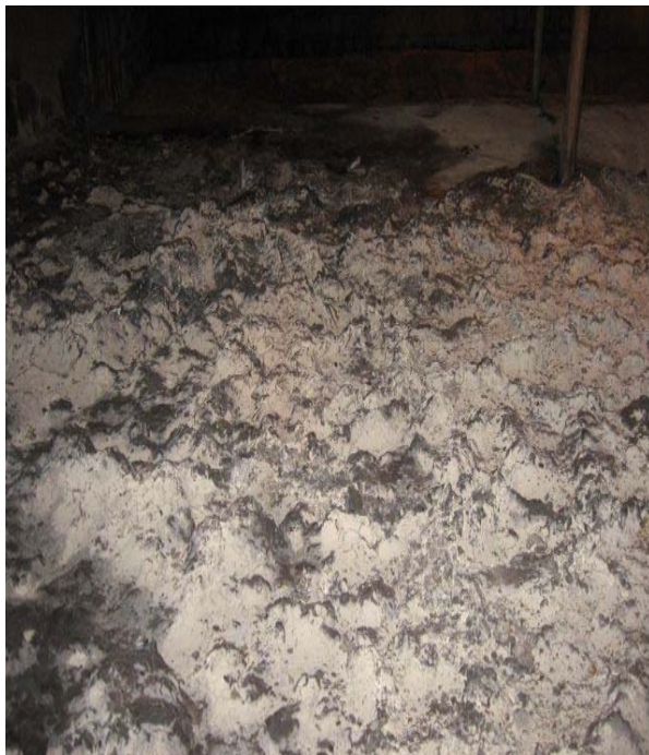
Fig.14: Unit 1 – Ash accumulated on the floor
