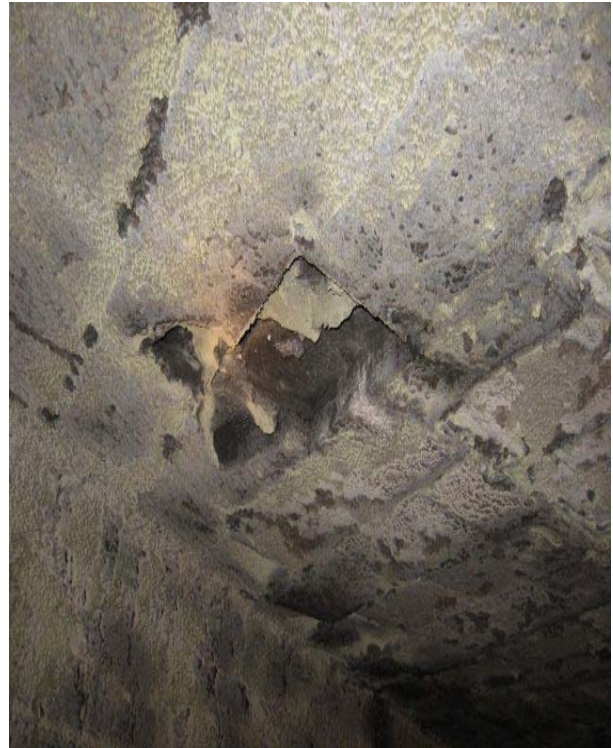
Fig. 13: Unit 1 – Missing block overhead
