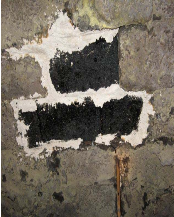
Fig. 12: Unit 1 – Replaced blocks
