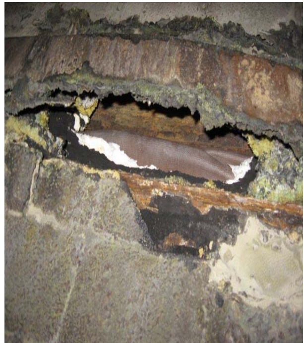
Fig. 15: Unit 1 – Damaged expansion joint
