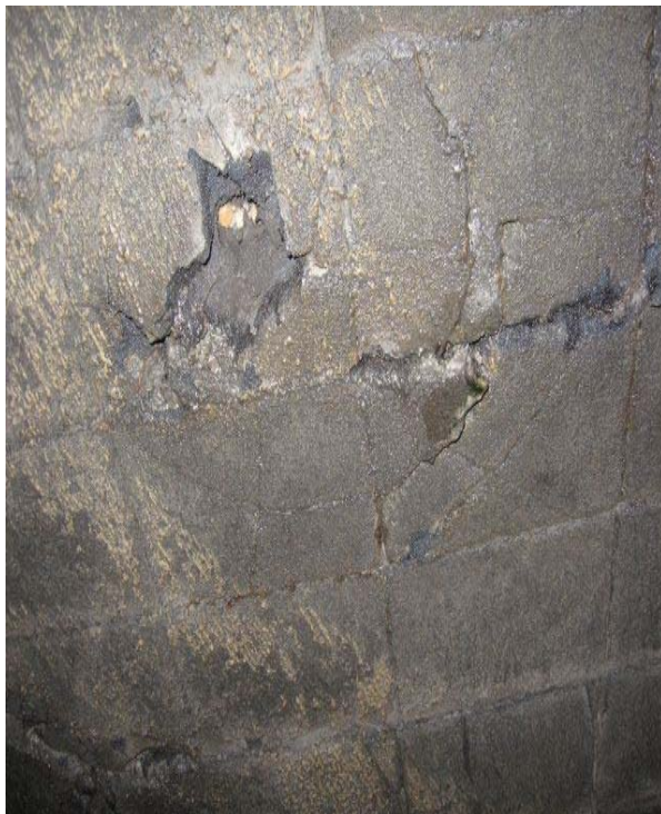
Fig. 18: Unit 2 – Missing insulation blocks
