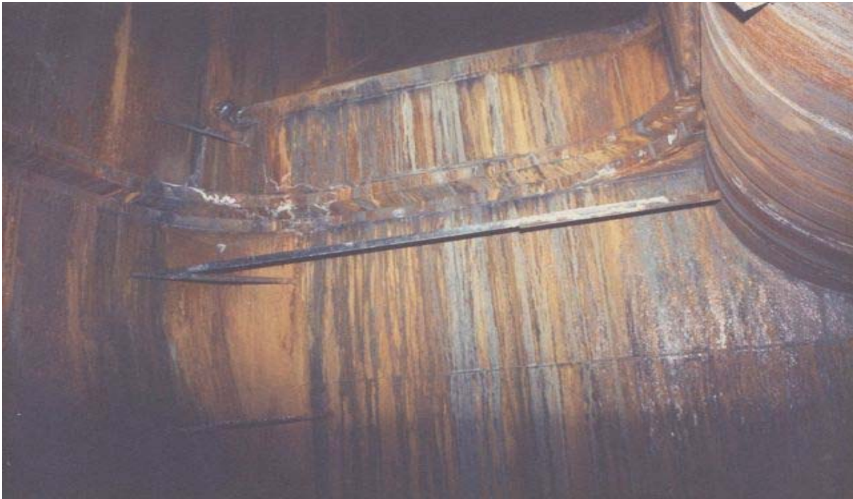
Fig. 2: Original Breeching, pantleg inlet – Unit 1 or 2
