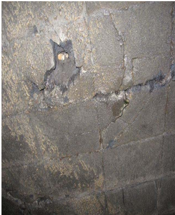
Fig. 18: Unit 2 – Missing insulation blocks
