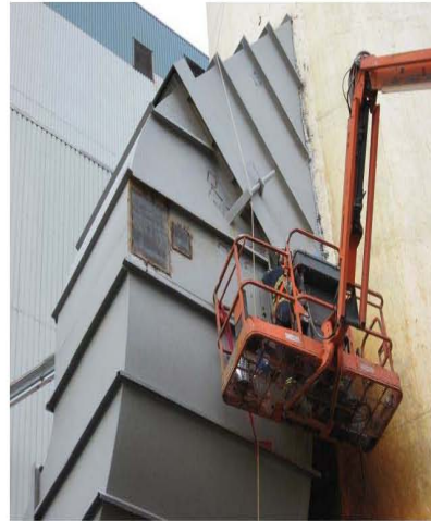
Fig. 17: Unit 1 – External duct repairs
