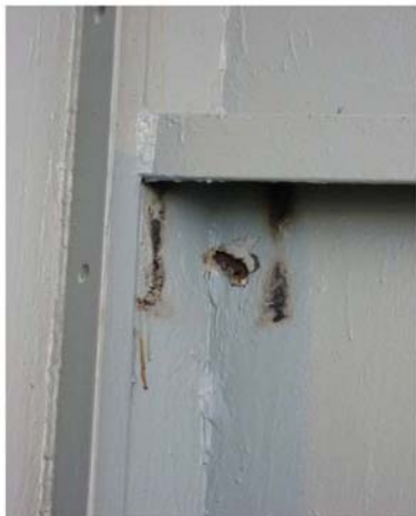
Fig. 25: Unit 3 – Patched casing (from inside)
