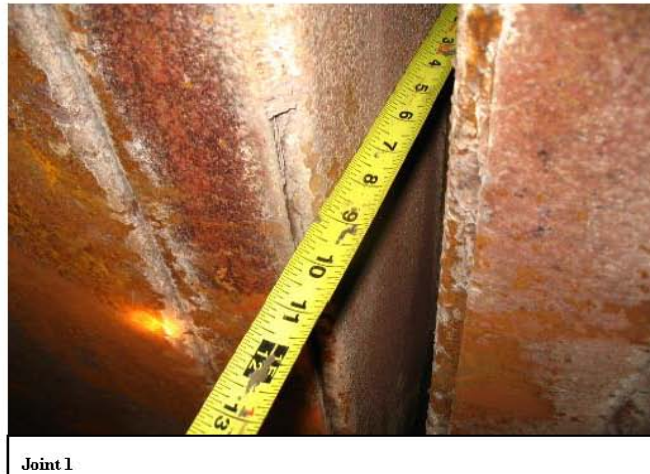
Fig. 30: Unit 3 – Expansion joint, hot air duct from air heater
