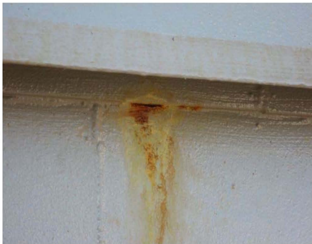
Fig.22: Unit 2 – External coating break down
