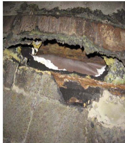
Fig. 15: Unit 1 – Damaged expansion joint
