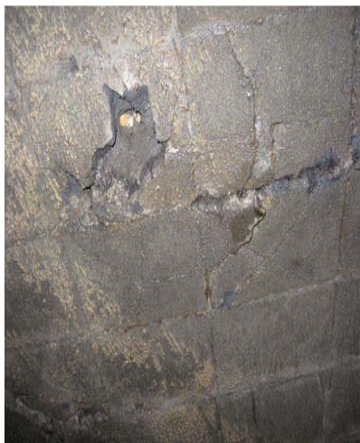
Fig. 18: Unit 2 – Missing insulation blocks
