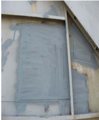
Fig. 16: Unit 1 – External duct repairs
