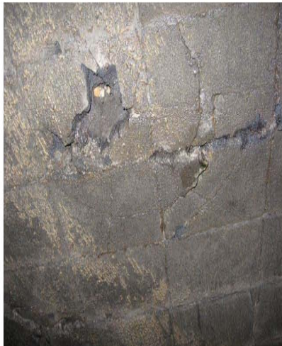
Fig. 18: Unit 2 – Missing insulation blocks
