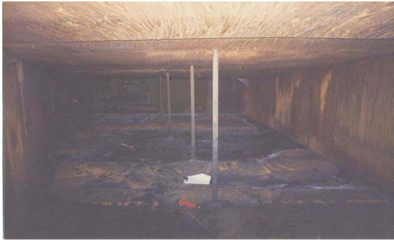
Fig. 1: Original Breeching, floor in horizontal section – Unit 1 or 2
