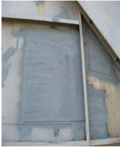
Fig. 16: Unit 1 – External duct repairs
