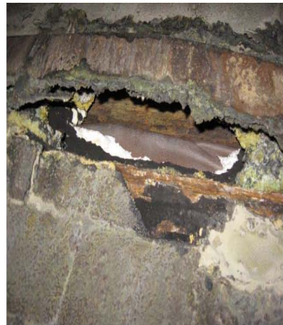
Fig. 15: Unit 1 – Damaged expansion joint
