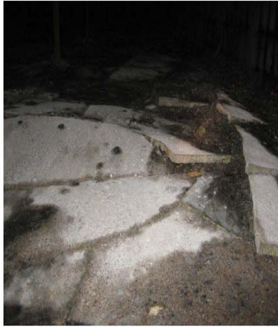
Fig. 20: Unit 2 – Cracked cement floor
