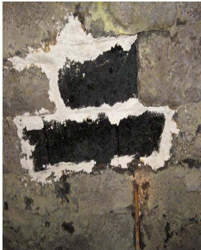
Fig. 12: Unit 1 – Replaced blocks
