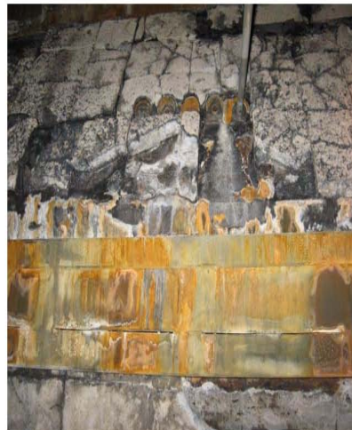
Fig. 19: Unit 2 – Missing insulation blocks
