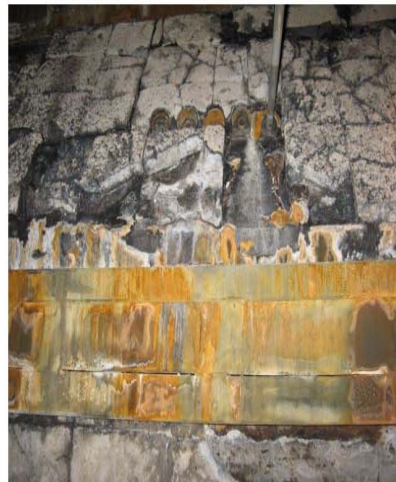
Fig. 19: Unit 2 – Missing insulation blocks
