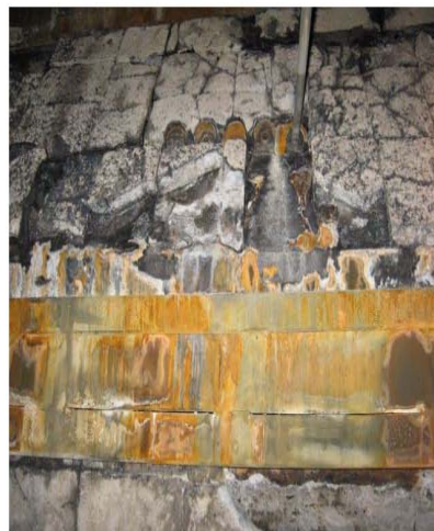
Fig. 19: Unit 2 – Missing insulation blocks
