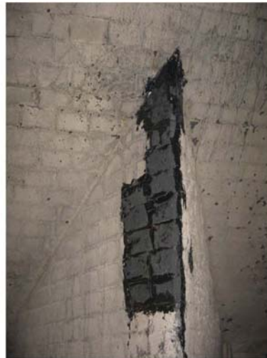
Fig. 24: Unit 3 – Crotch repairs
