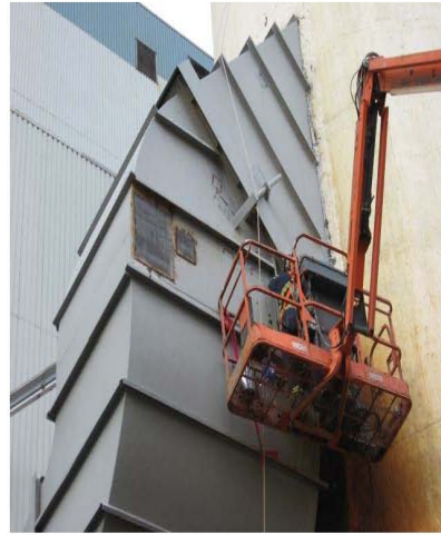
Fig. 17: Unit 1 – External duct repairs
