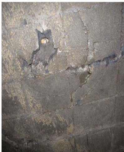
Fig. 18: Unit 2 – Missing insulation blocks
