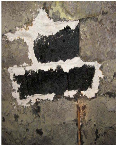
Fig. 12: Unit 1 – Replaced blocks
