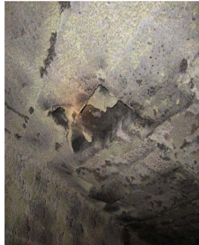
Fig. 13: Unit 1 – Missing block overhead
