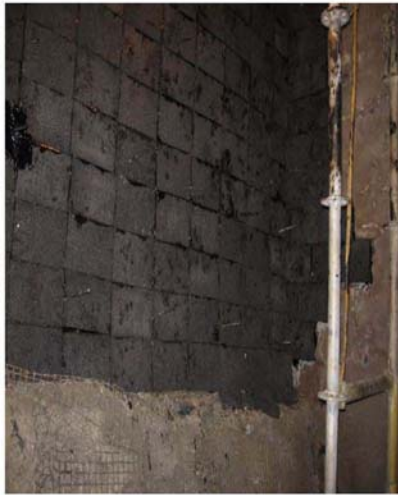
Fig. 8: Unit 1 – Insulating block replacement
