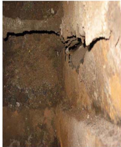
Fig. 9: Unit 1 – Duct corroded through
