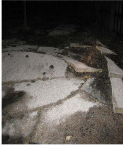
Fig. 20: Unit 2 – Cracked cement floor
