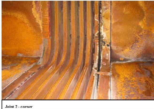
Fig. 31: Unit 3 – Expansion joint, hot air duct from air heater
