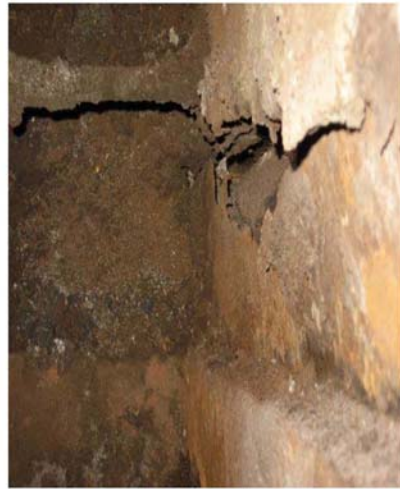
Fig. 9: Unit 1 – Duct corroded through
