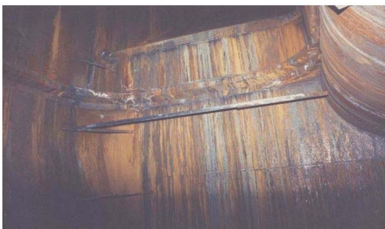
Fig. 2: Original Breeching, pantleg inlet – Unit 1 or 2
