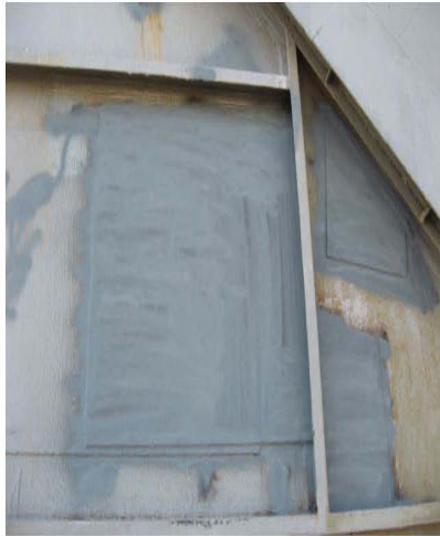
Fig. 16: Unit 1 – External duct repairs
