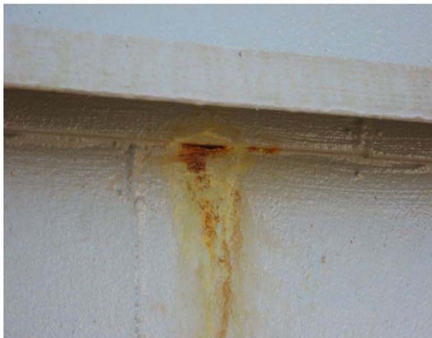
Fig.22: Unit 2 – External coating break down
