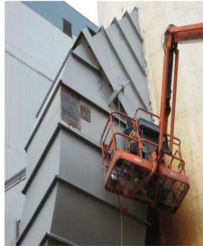
Fig. 17: Unit 1 – External duct repairs
