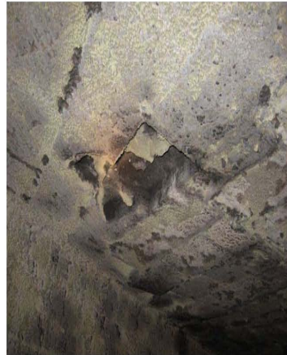
Fig. 13: Unit 1 – Missing block overhead
