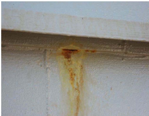
Fig.22: Unit 2 – External coating break down
