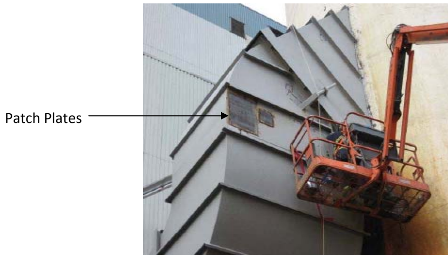
Figure 4 – Unit 1 Breeching Plate Repairs
