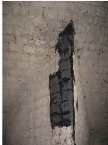
Fig. 24: Unit 3 – Crotch repairs
