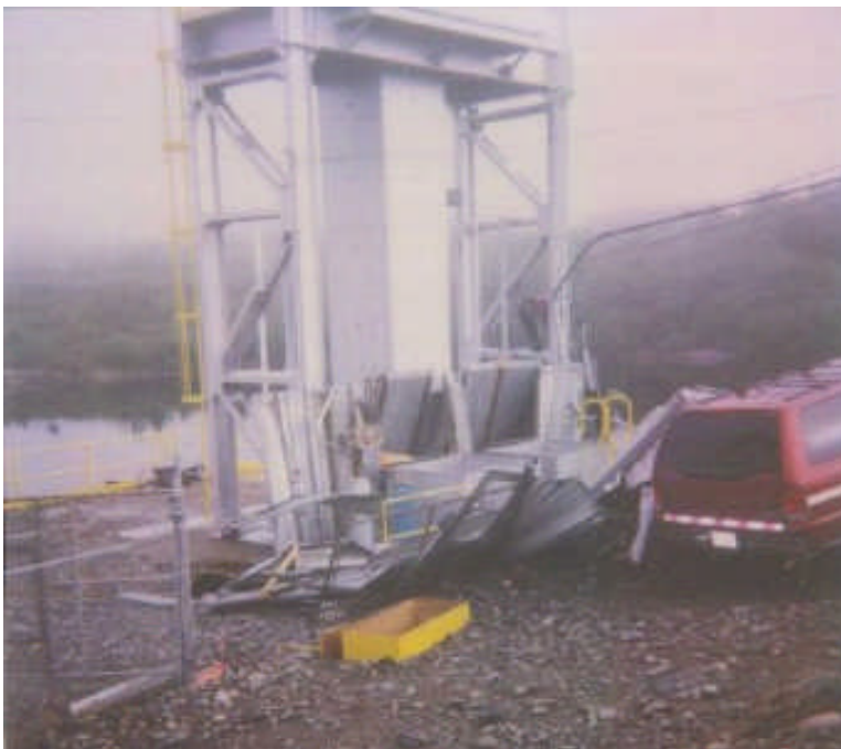
Bay D'Espoir Intake #2 after the failure in 2000.
