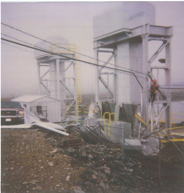
Bay D'Espoir Intake #1 (shown on left) and Intake #2 (shown on right) after the failure in 2000. Notice that the vent house structure has been completely destroyed as it previously resembled that of
