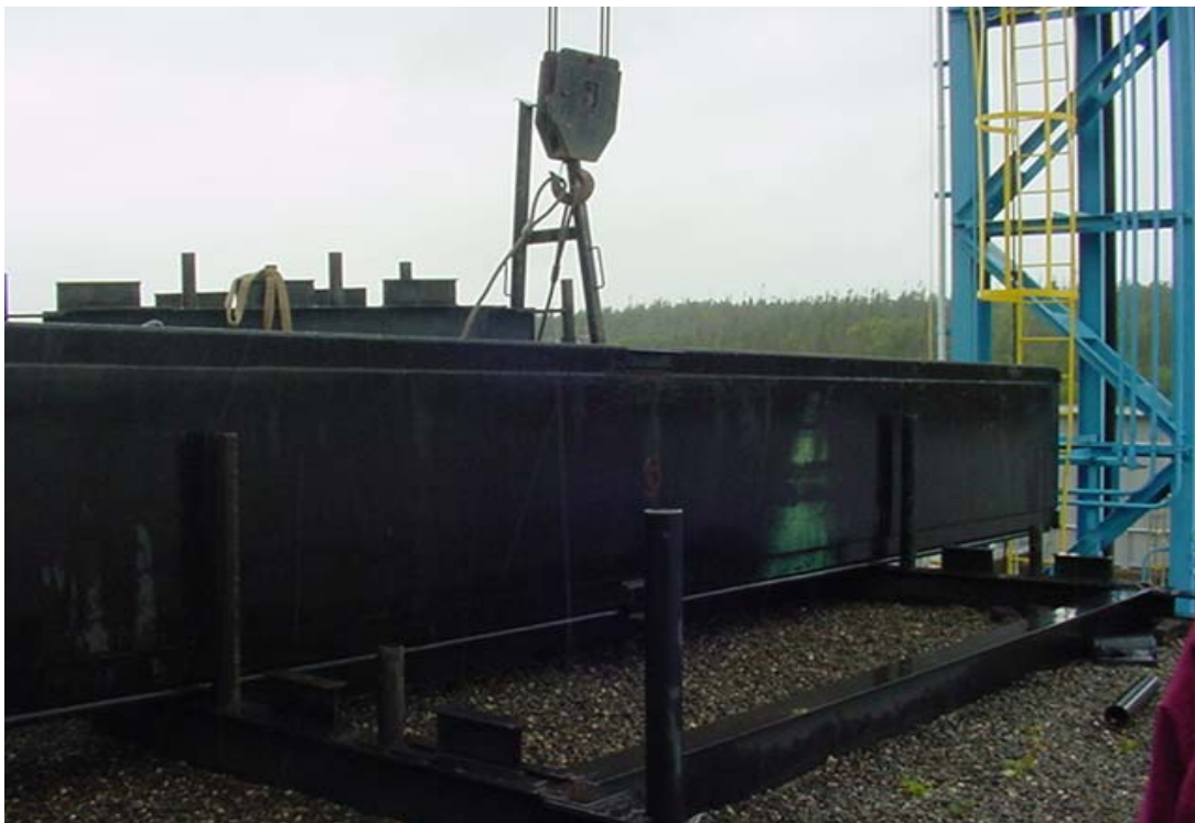
Picture # 8: Stop Log Transfer to Boom Truck
