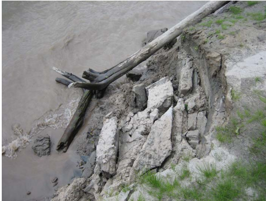
Erosion at downstream slope toe (Site Visit -1)
