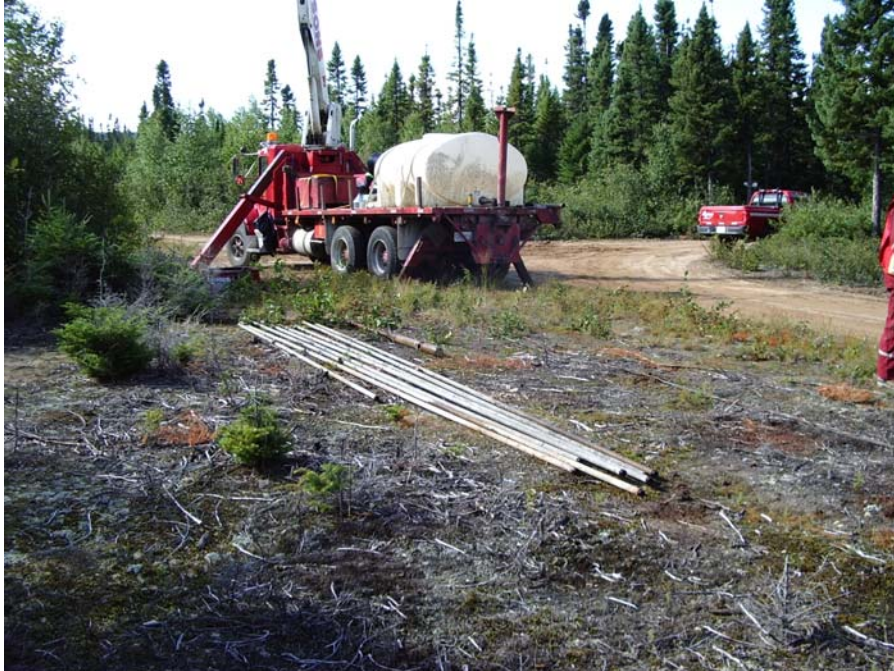
Photograph 3: The risers and pump were laid down on the ground for inspection.
