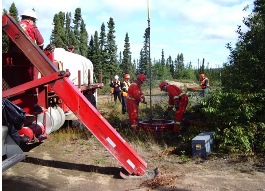
Photograph 2: The risers, wiring and pump were removed from each well.
