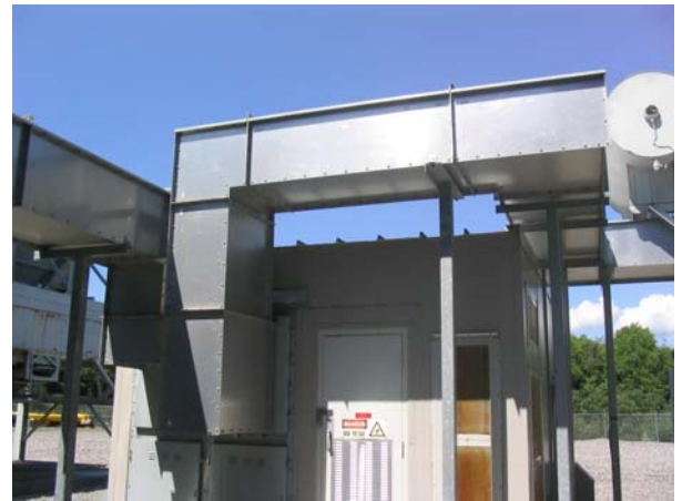
SVL-030 – 13.8 kV Bus Duct
