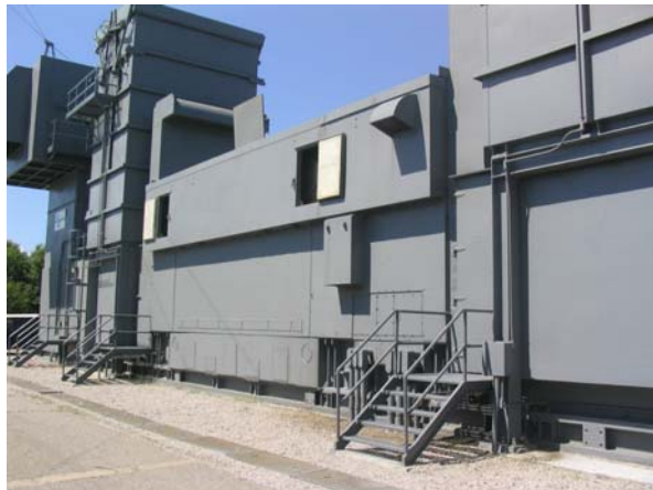
SVL-019 – Alternator Enclosure
