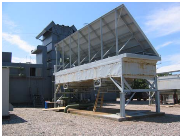
SVL-021– Alternator Glycol Cooler
