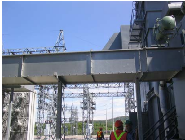
SVL-029 – 13.8 kV Bus Duct
