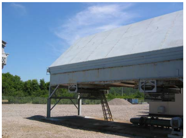
SVL-022– Alternator Glycol Cooler
