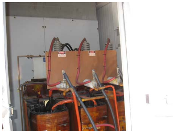
SVL-033 – 15 kV Transformer Cabling
