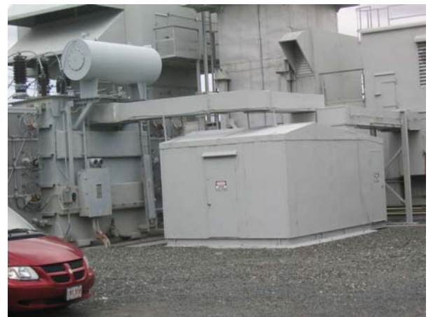
HWD-032 – 13.8 kV Bus Duct
