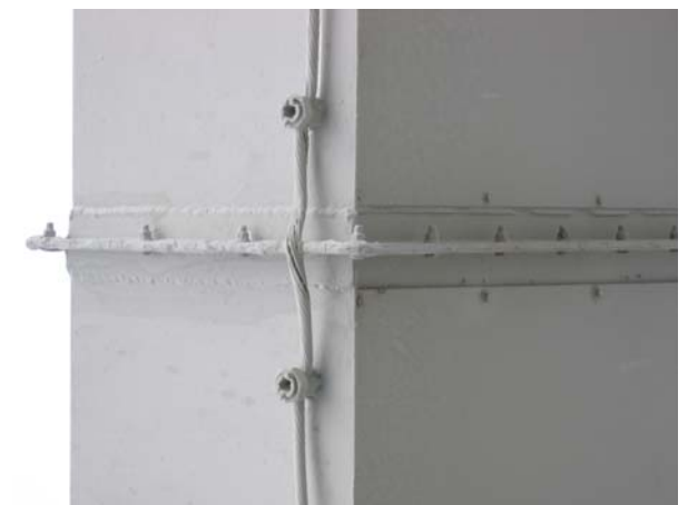
HWD-034 – 13.8 kV Bus Duct
