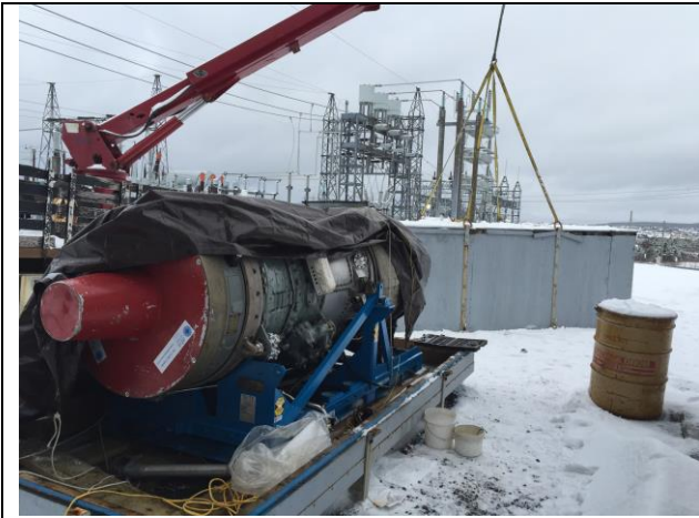
202205 removal of fuel pumps for Stephenville
