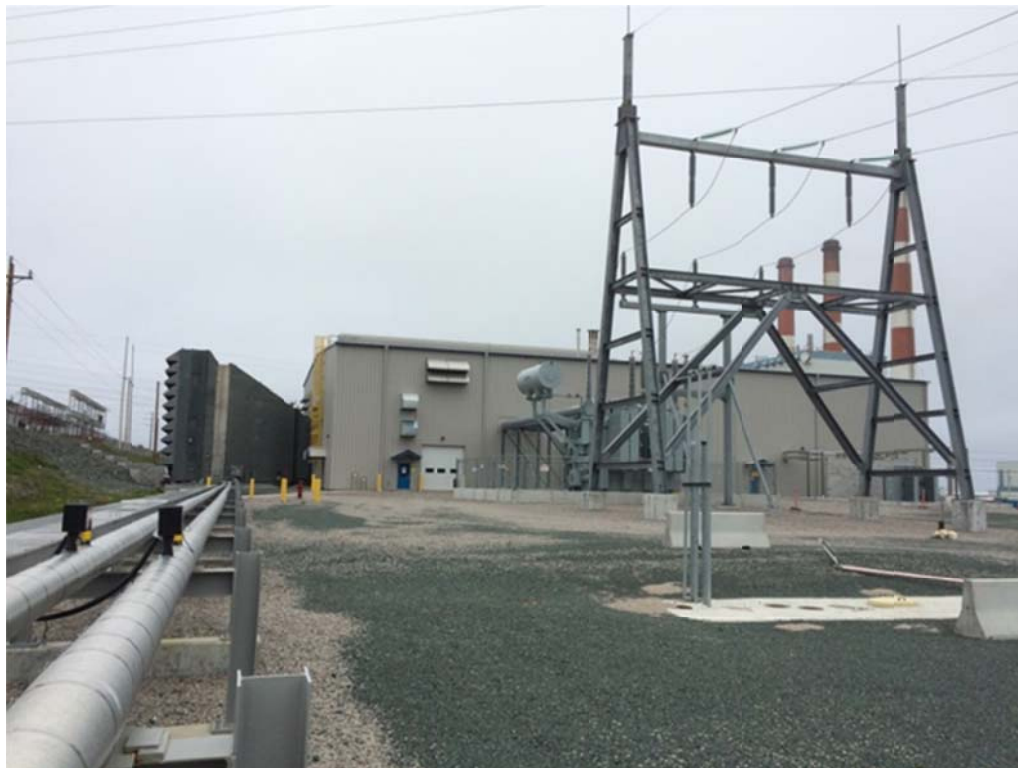
Figure 2: Holyrood Combustion Turbine Plant
