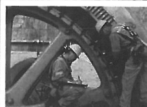
Refurbishment of a generating unit's air-gap at Hull-2 generating station
