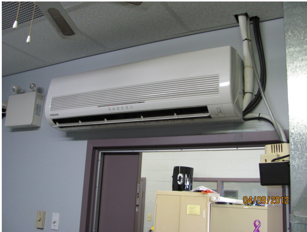
Existing Metering Mini-Split A/C Unit
