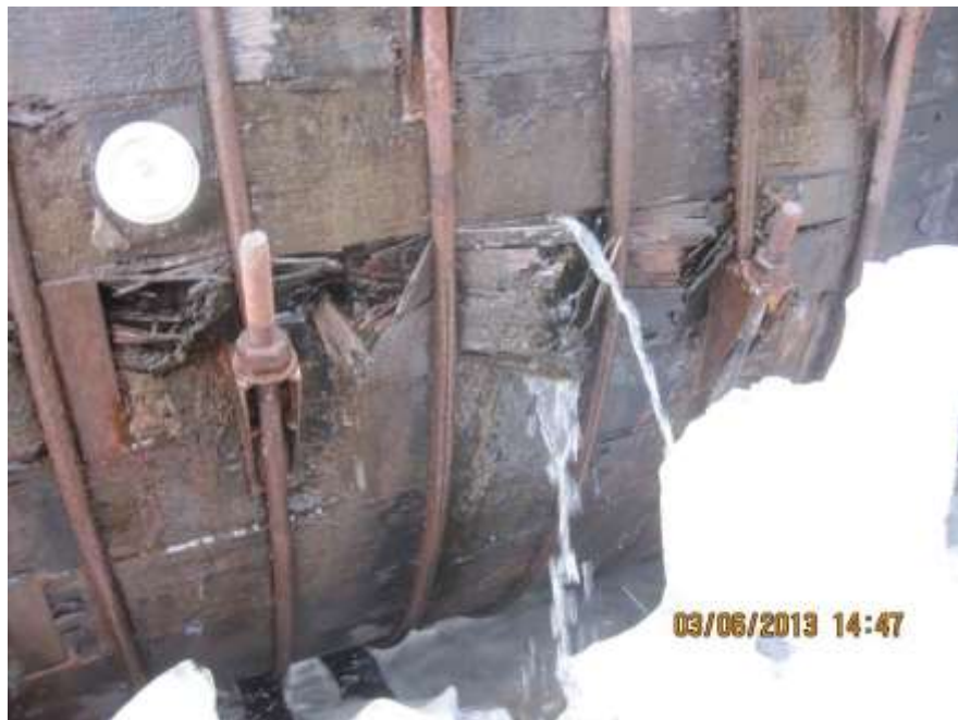
Figure 10: Crushed Stave
