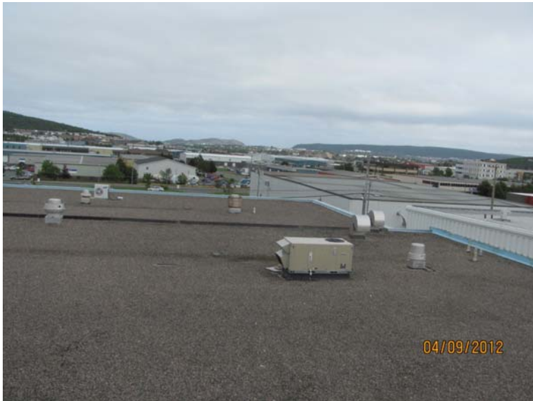
Existing Mini-Split Condensing Unit and Packaged A/C Units Serving: Metering, Newly Added Offices and Mezzanine
