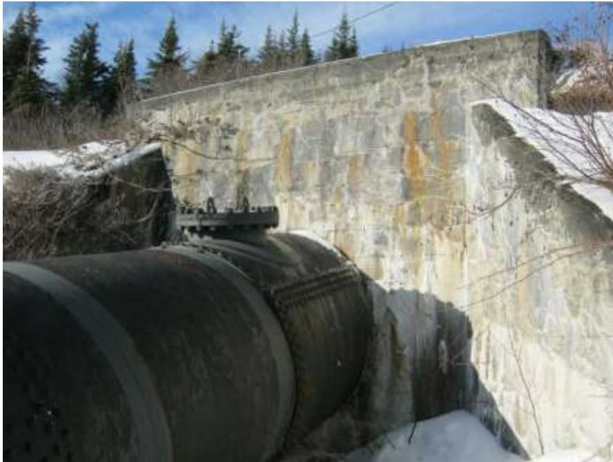
Photo C-13: Anchor block at upstream end of steel penstock
