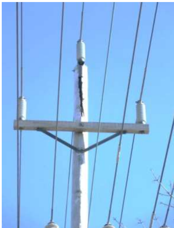
Figure 12 – Burned Pole
