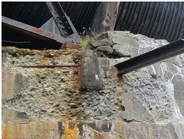
Photo No. 2.4.1.15 – Severe Deterioration Below Baseplate on East Abutment
