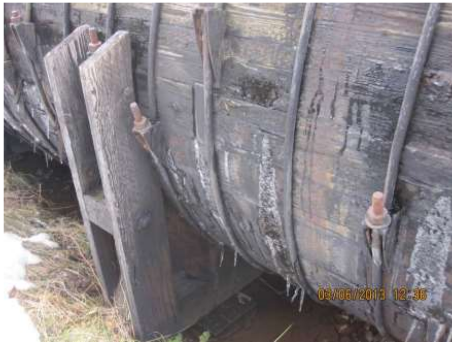
Figure 17: Typical 190 Degree Cradle (Note: Top of cradle not supporting pipe)
