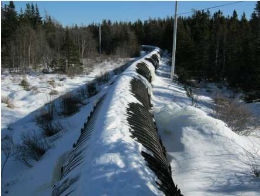
Photo C-60: Leakage along springline of penstock
