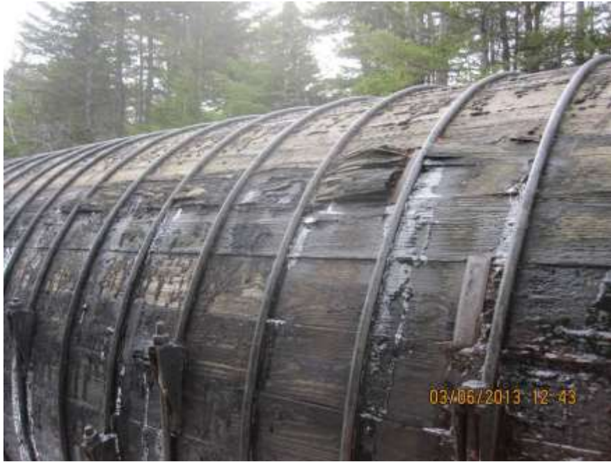
Figure 19: Deteriorated Stave
