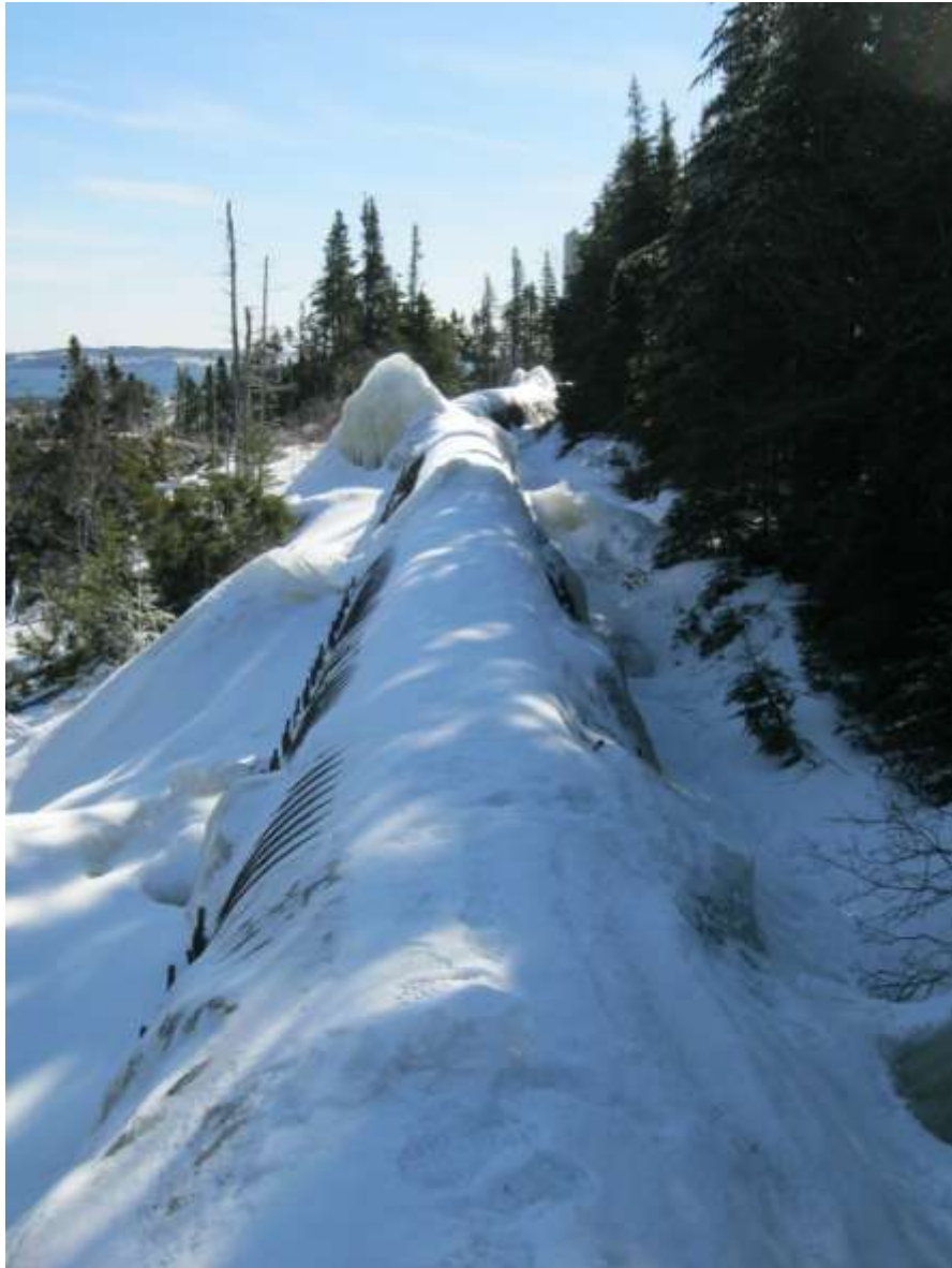
Photo C-37: General view of penstock upstream of surge tank showing leakage
