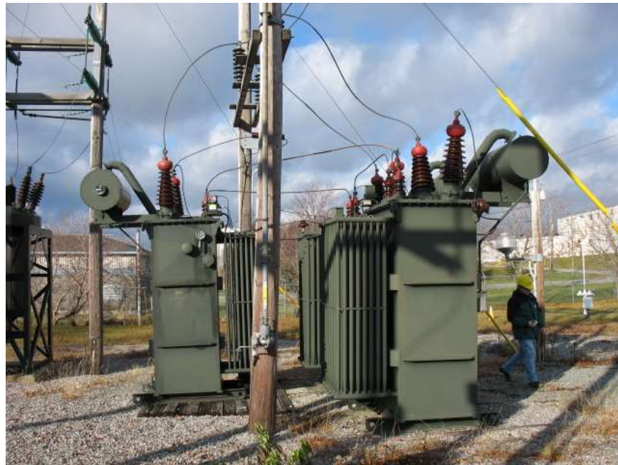
Existing Grounding Transformers T3
