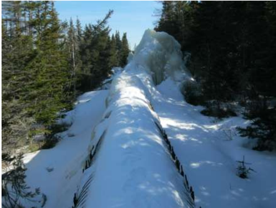
Photo C-40: General view of penstock showing leakage
