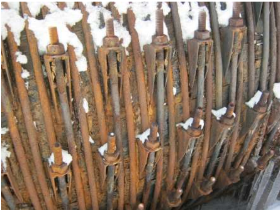
Photo C-17: Deteriorated wood staves near downstream end of penstock
