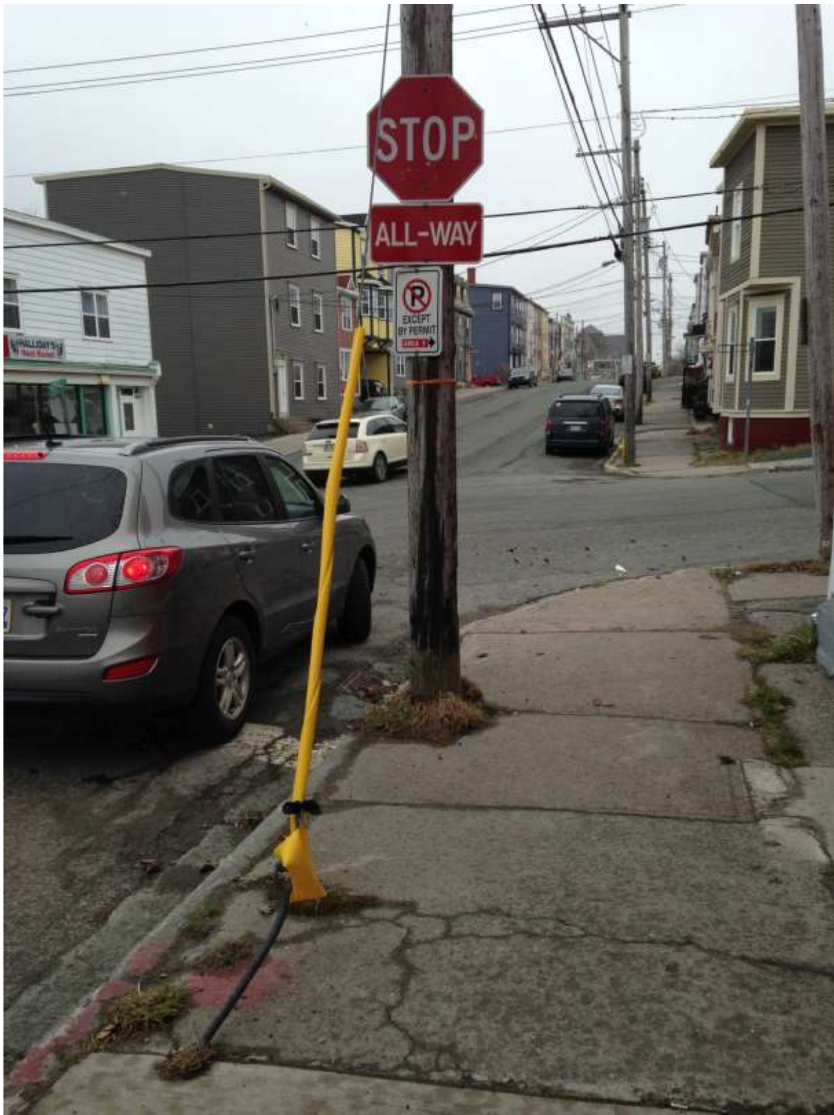
Figure 5 - Guy Bent Towards Sidewalk
