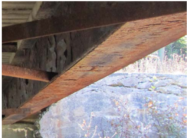
Photo No. 2.3.1.6 – Remaining Section of Steel Column, Typical
