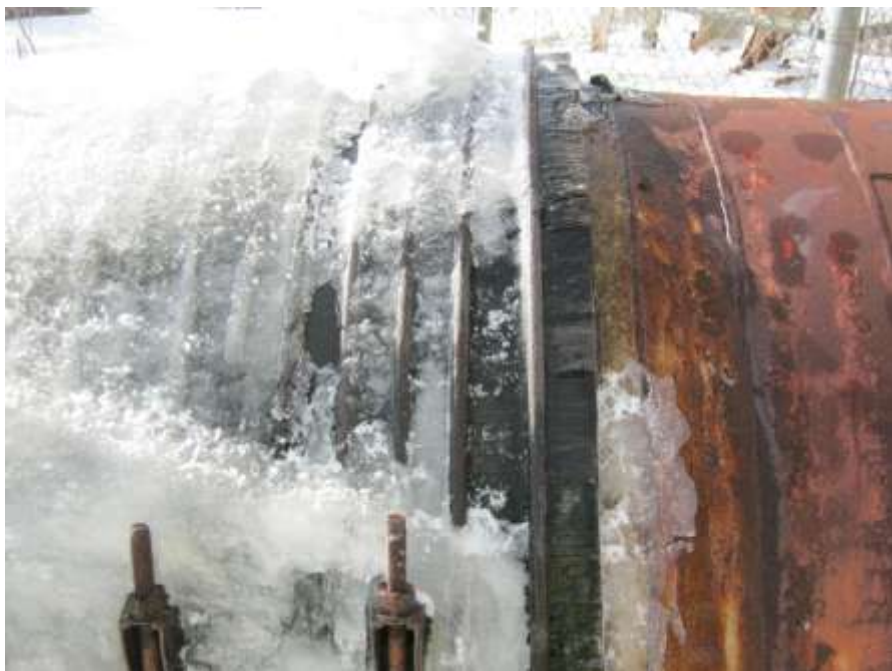
Photo C-27: Wood stave connection to downstream end of surge tank tee
