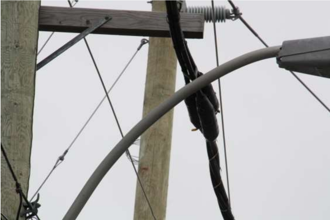
Figure 7 – Aerial Cable Splice
