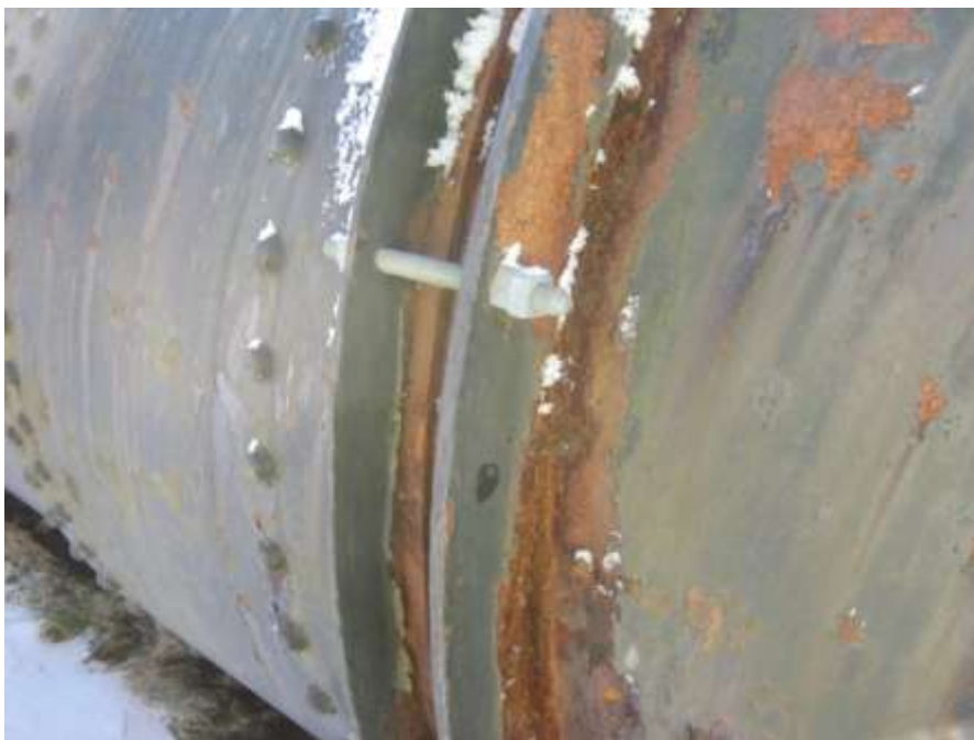
Photo C-8: Mechanical expansion joint
