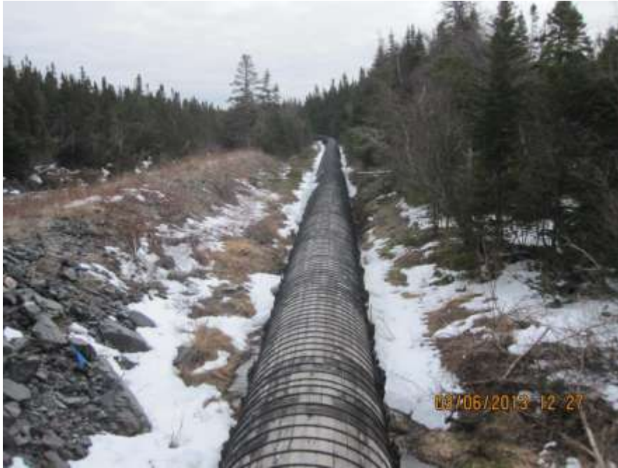
Photo C-64: Penstock immediately downstream of dam
