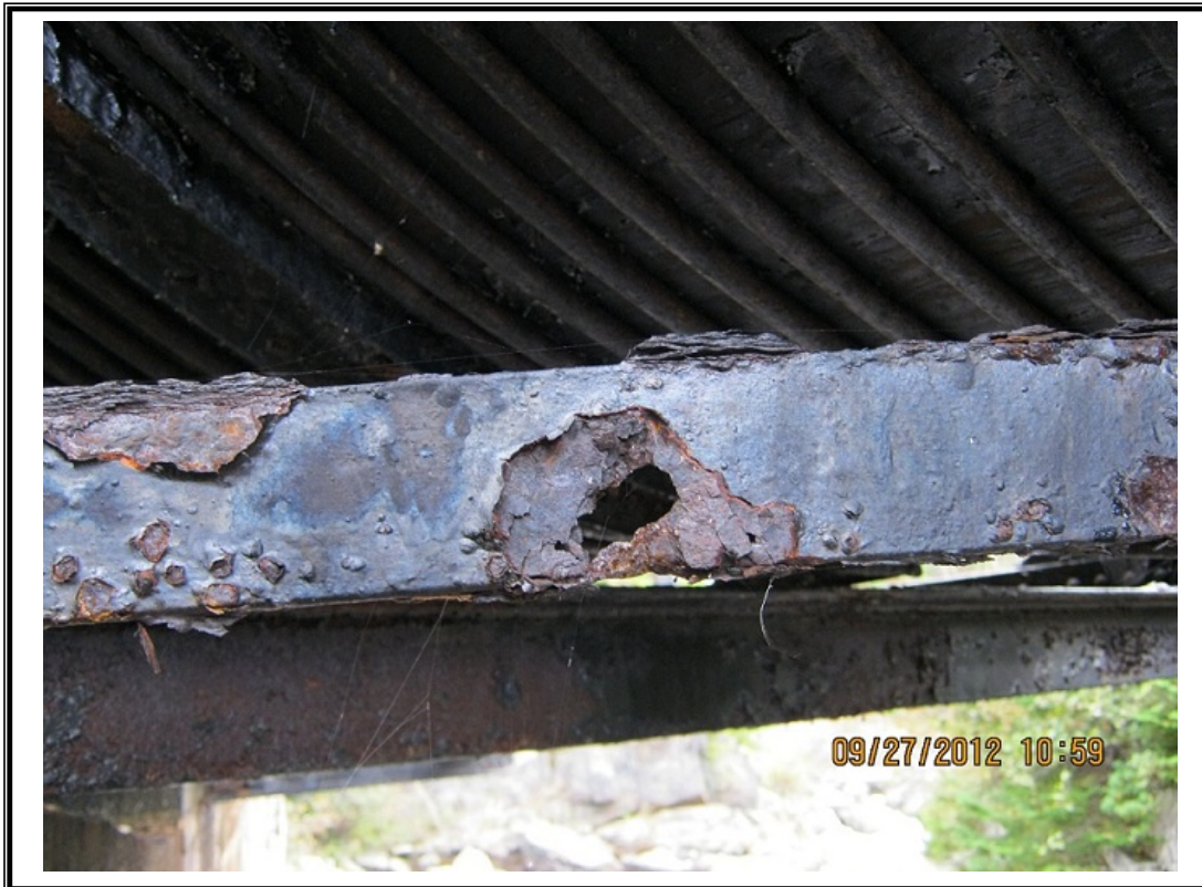
Photo No. 3 – Deteriorated Bottom Truss Horizontal Cross Brace
