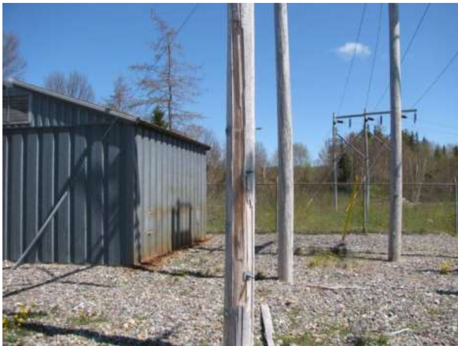
Figure 38 - Bolts Keeping Broken Pole Together
