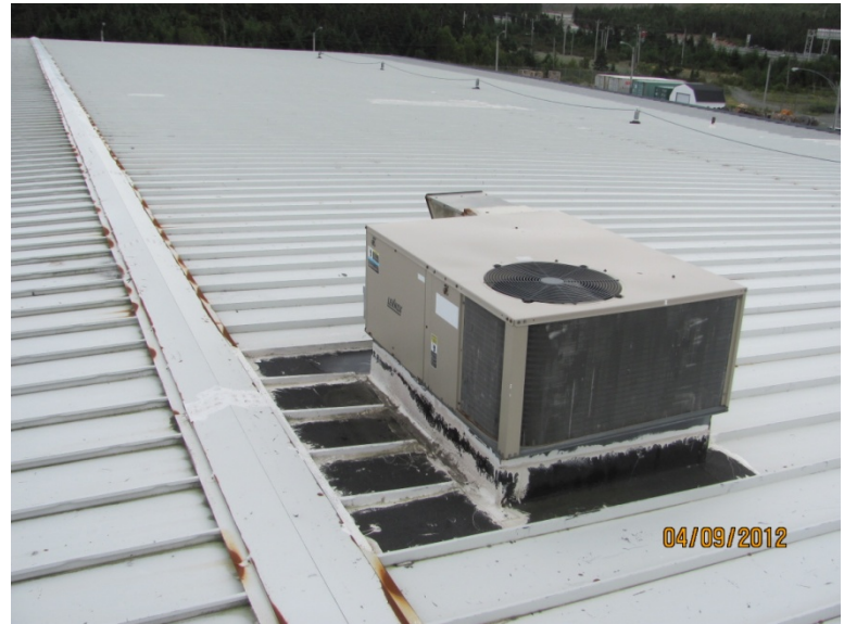
Existing Mini-Split Condensing Unit and Packaged A/C Units Serving: Metering, Newly Added Offices and Mezzanine
