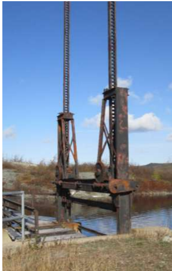
Figure 3 – Stop Log Lift
