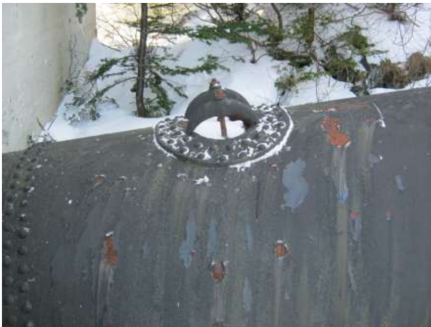
Photo C-3: Access hole near powerhouse
