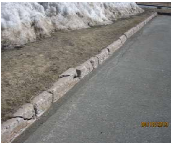
Figure 12 - Damaged Curbs
