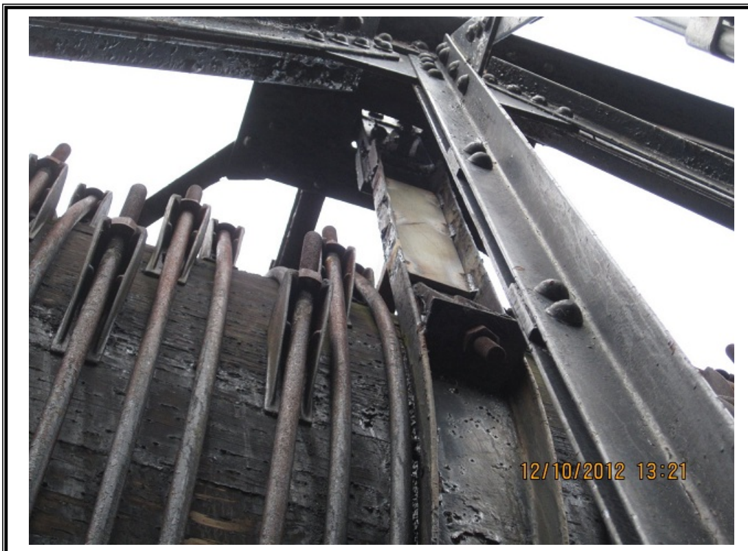
Photo No. 6 – Hanging Support Repair Detail
