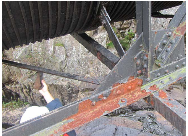
Photo No. 2.4.1.8 – Rust on North-Bottom Chord Connection, Typical
