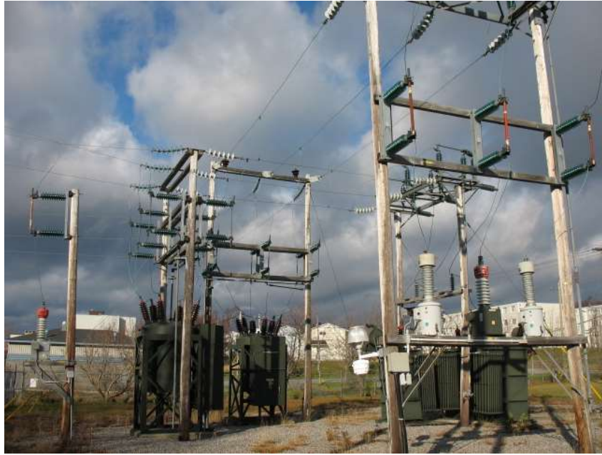
66 kV Wood Pole Structures that Requires Replacement
