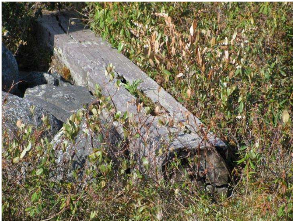
Figure 40 – Deteriorated Pole Crib Timber
