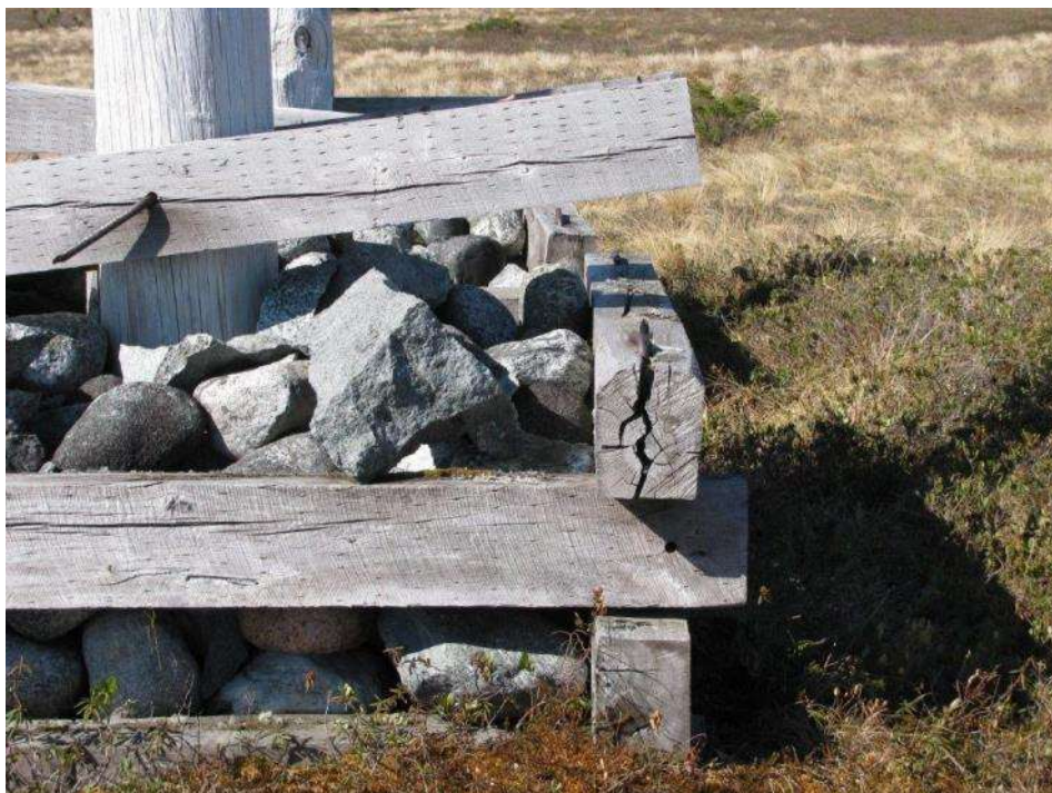
Figure 42 – Deteriorated Pole Crib Timber
