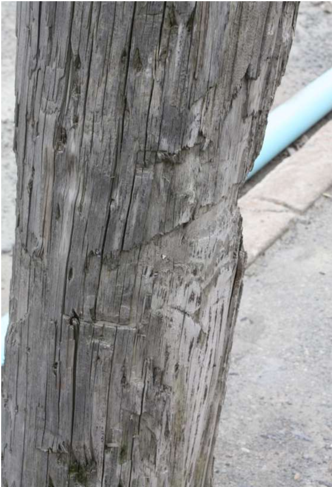
Figure 6 – Pole Damage near Base
