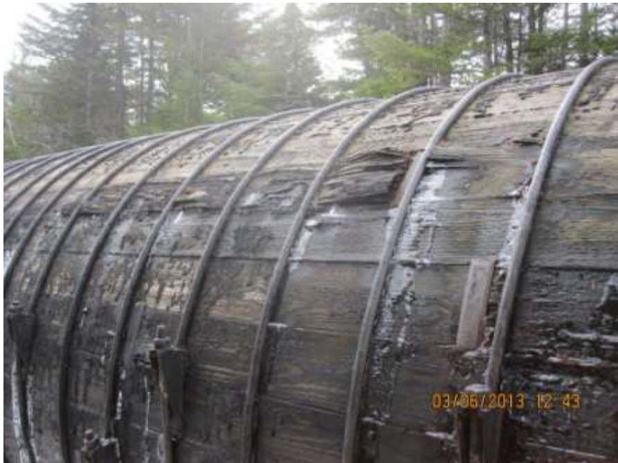
Photo C-53: Delaminated wood stave with broomed end
