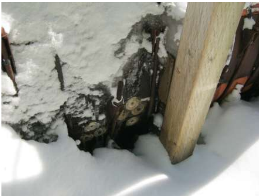
Photo C-35: Patching at springline at location of previous blow-out
