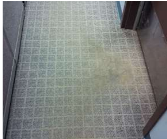
Figure 6 - Deteriorated Carpet
