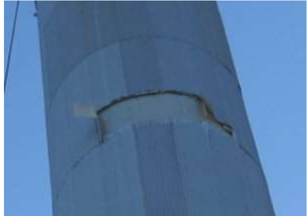
Figure 7 - Frost Casing Failure 2013
