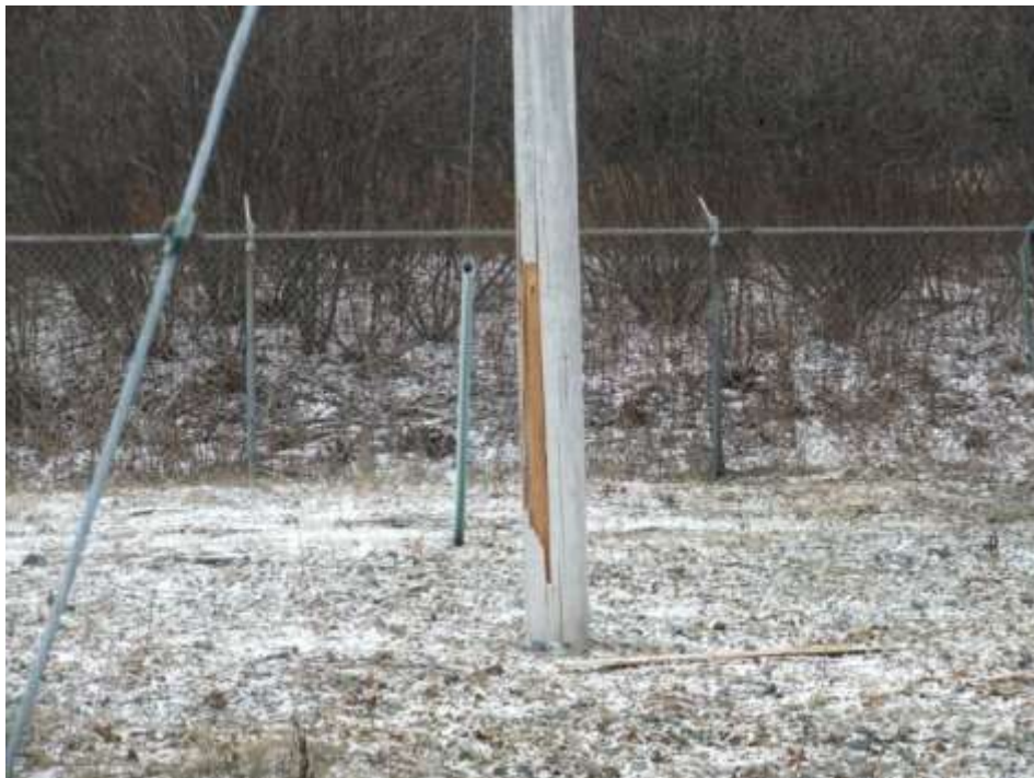
Figure 32 – Exposed Inner Wood
