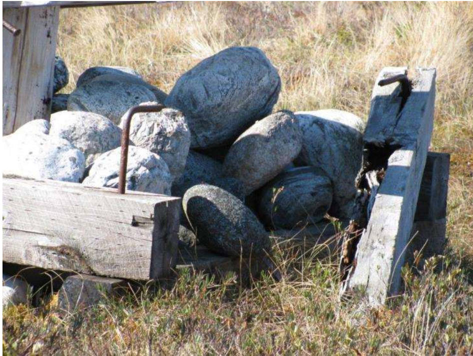
Figure 41 – Rock Ballast No Longer Contained
