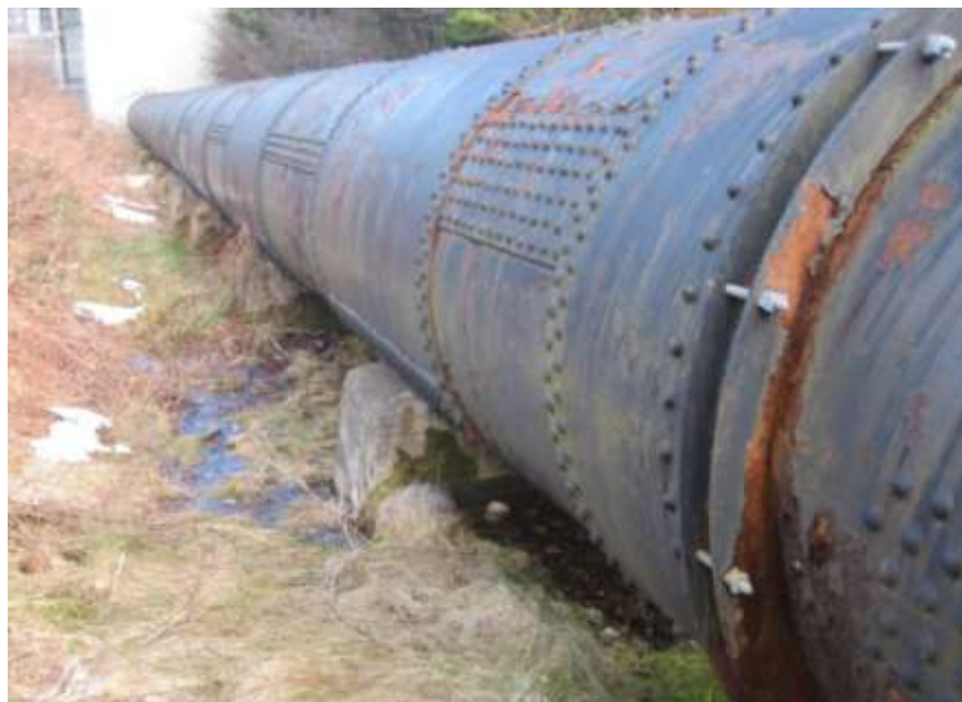
Figure 6: Steel Expansion Joint
