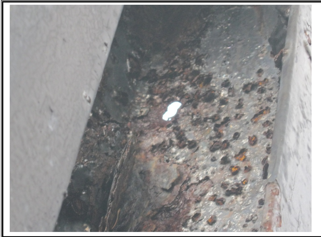
Photo No. 5 – Deteriorated Hanging Support
