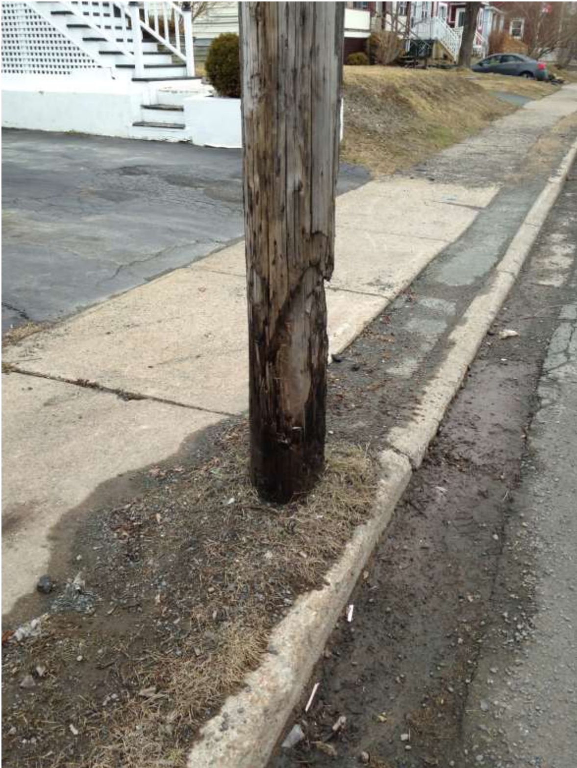
Figure 2 - Pole Damage at Base
