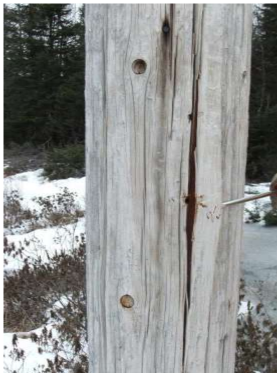
Figure 22 – Pole Shell Separation
