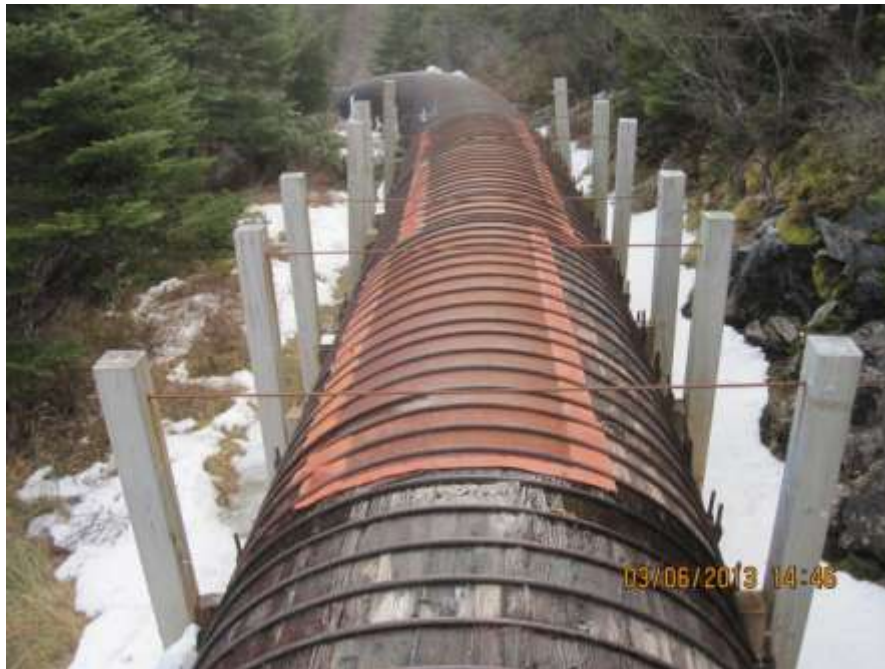
Photo C-34: Modifications at location of previous blow-out
