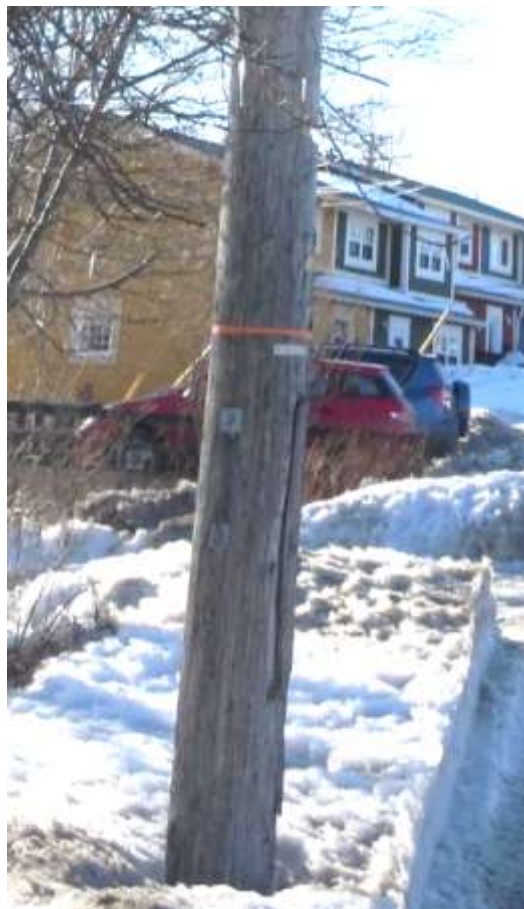
Figure 14 – Bolts Provide Temporary Repairs to Damaged Pole
