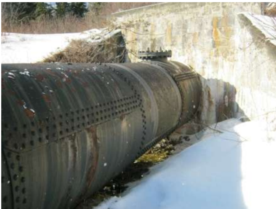
Photo C-6: General condition of steel penstock shell
