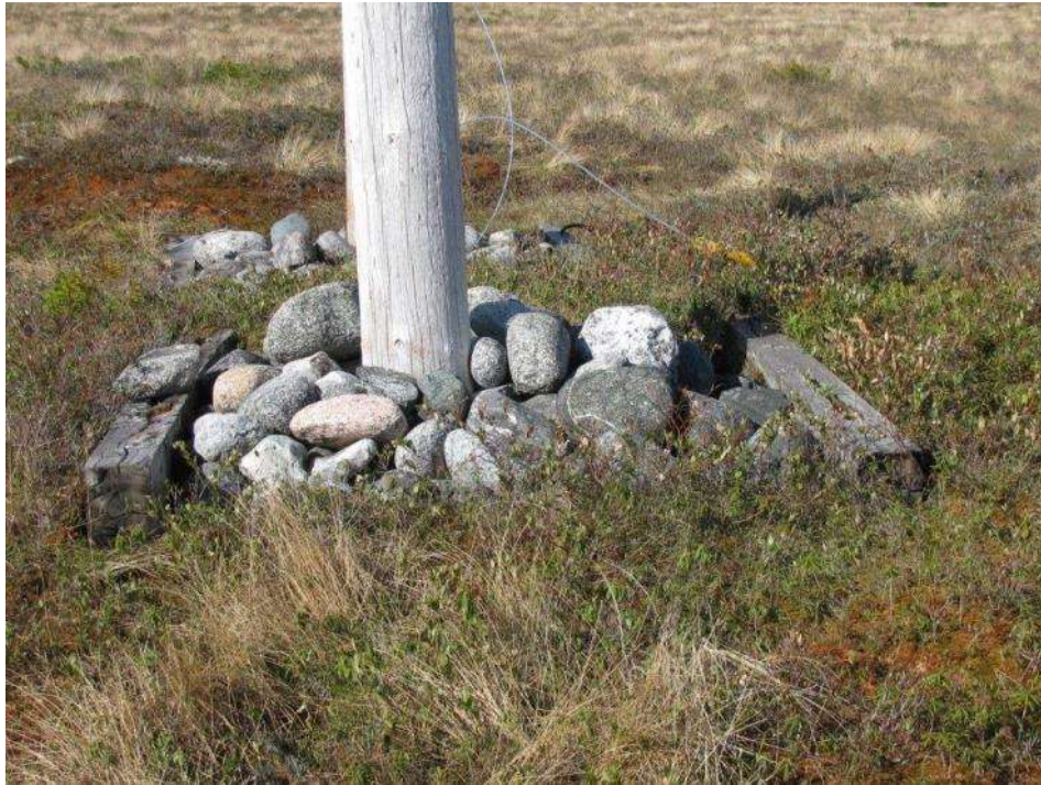
Figure 39 – Deteriorated Pole Crib
