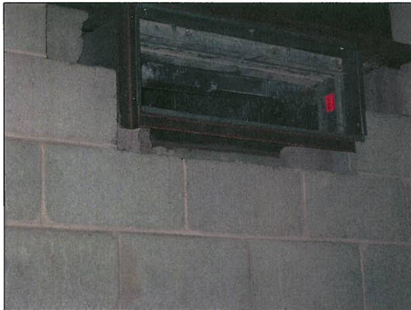
Picture 13: Exhaust ventilation duct opening. Note missing grille and grouting for fireproofing
