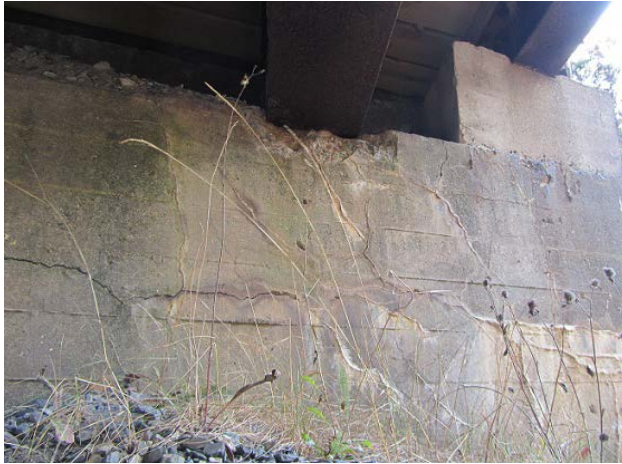
Photo No. 2.2.1.9 – Concrete Severely Deteriorated Under Beam
