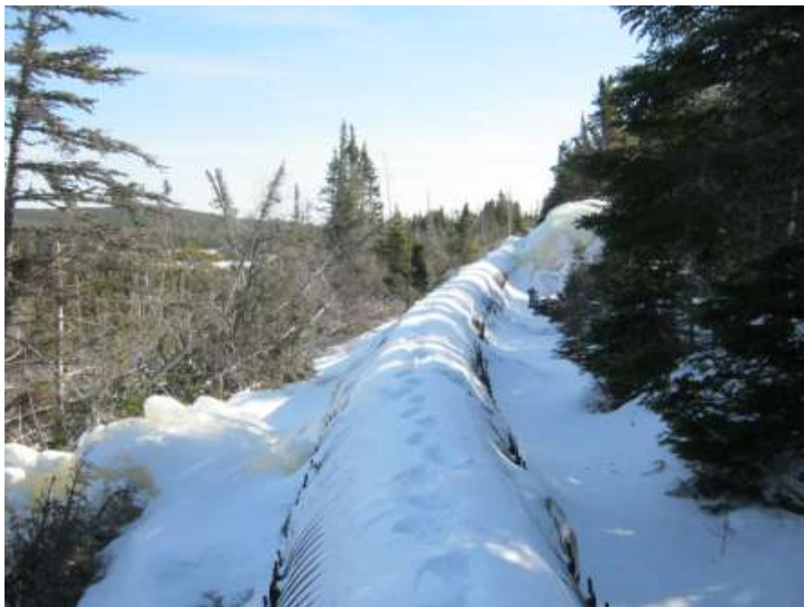
Photo C-39: General view of penstock showing leakage
