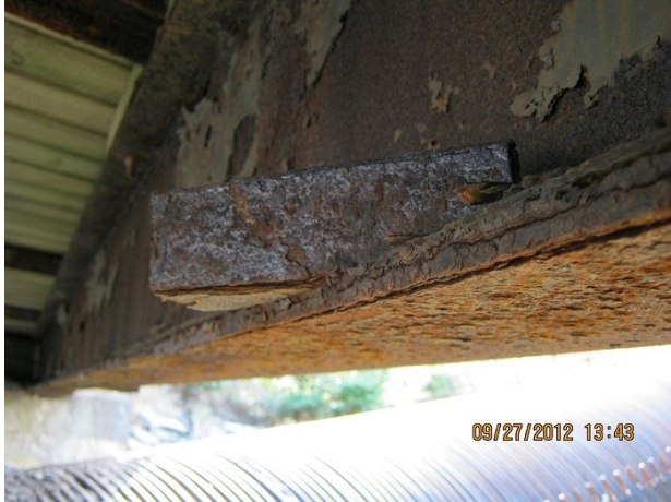
Photo No. 2.2.1.5 – Remaining Section of Steel Angle Cross-bracing, Typical
