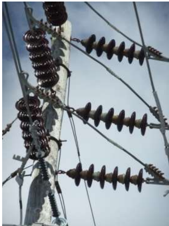
Figure 10 – 1950's Vintage Insulators and Hardware
