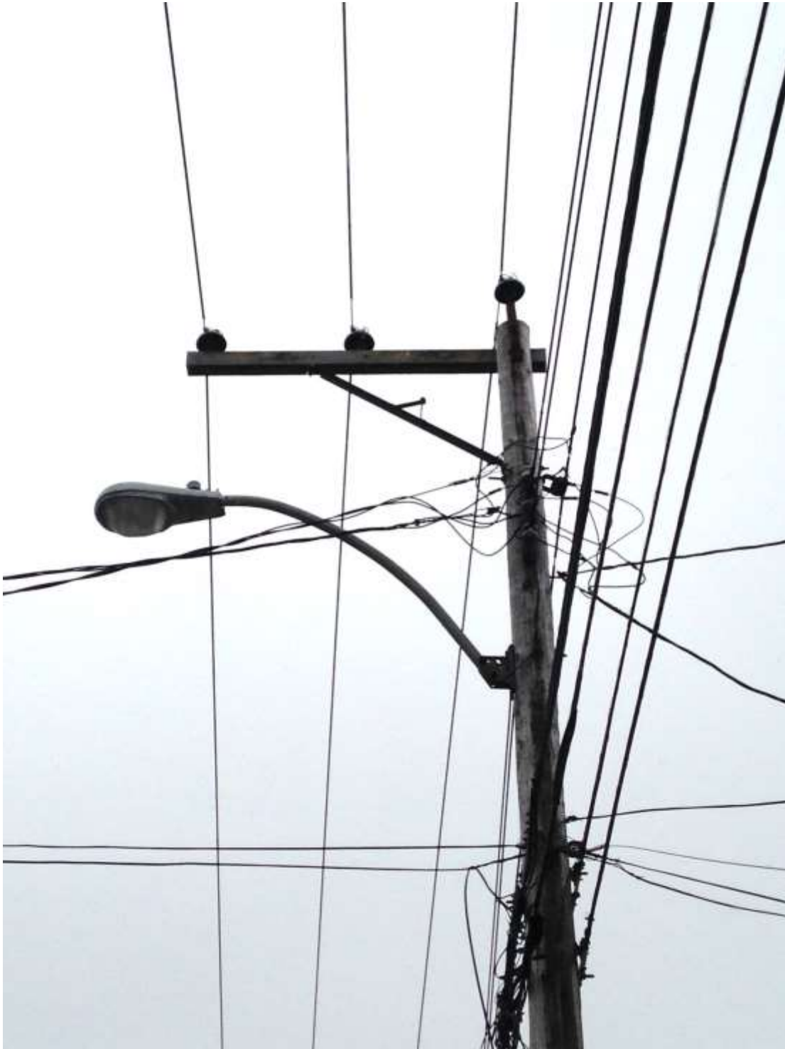
Figure 1 - KBR-10 Pole with Alley Arm Type Crossarm
