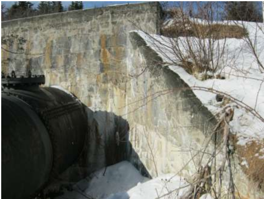
Photo C-14: Anchor block at upstream end of steel penstock
