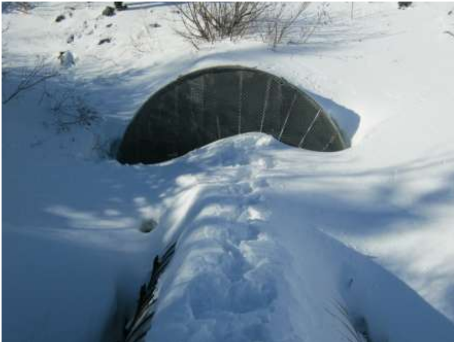
Photo C-65: Penstock entering culvert at downstream toe of dam
