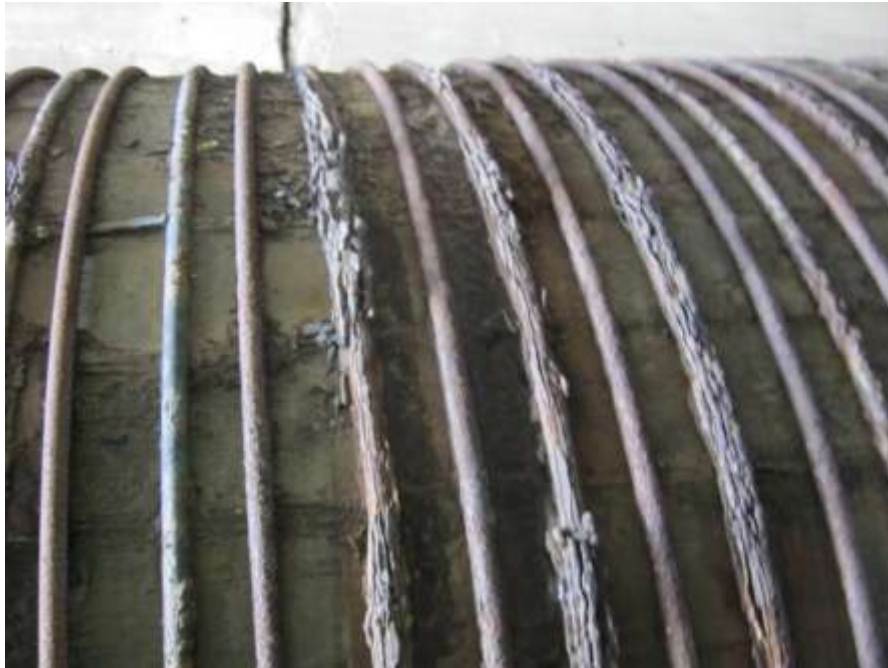
Photo C-44: Corroded bands under highway crossing
