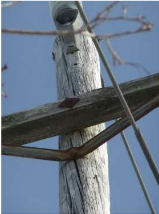
Figure 3 – Pole Checking and Deteriorated Crossarm
