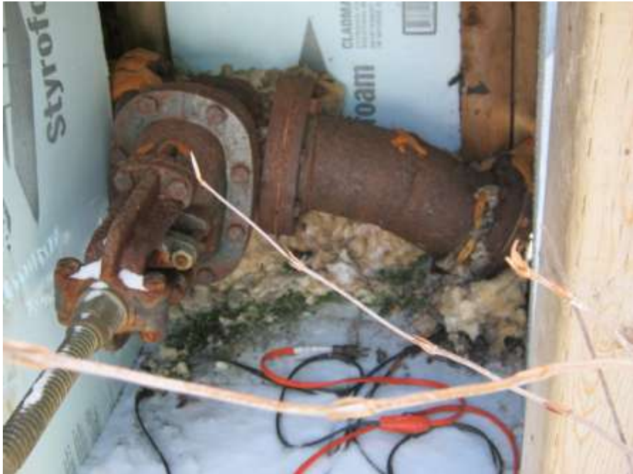
Photo C-26: Water supply line from side of penstock
