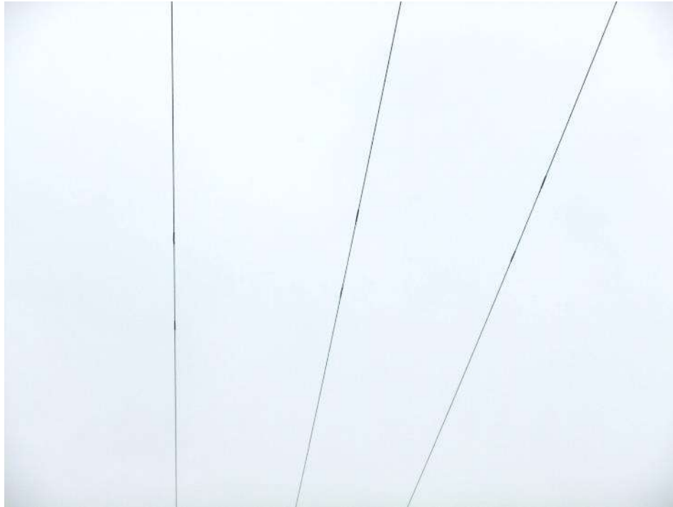
Figure 27 – Repairs to Conductor Due to Phase Contact Damage
