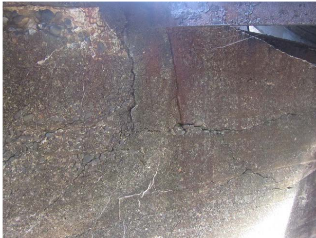
Photo No. 2.4.1.17 – Significant Cracks, Concrete Abutment, Typical
