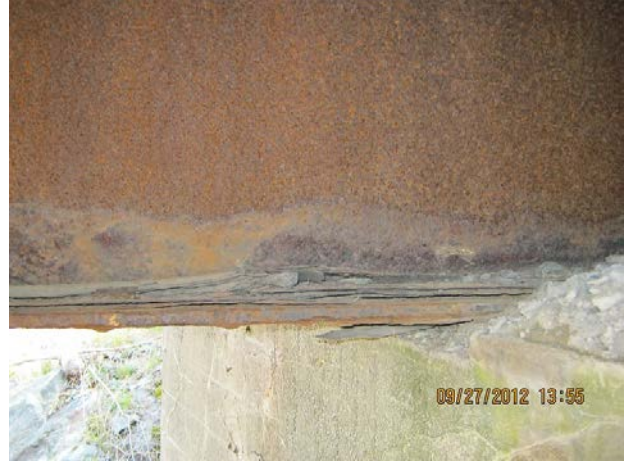
Photo No. 2.2.1.2 - Severe Scaling on Beams, Typical
