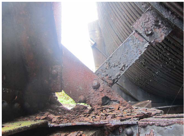
Photo No. 2.4.1.14 – Rust and Scaling on Support Band-Bottom Chord Connection Member, Typical
