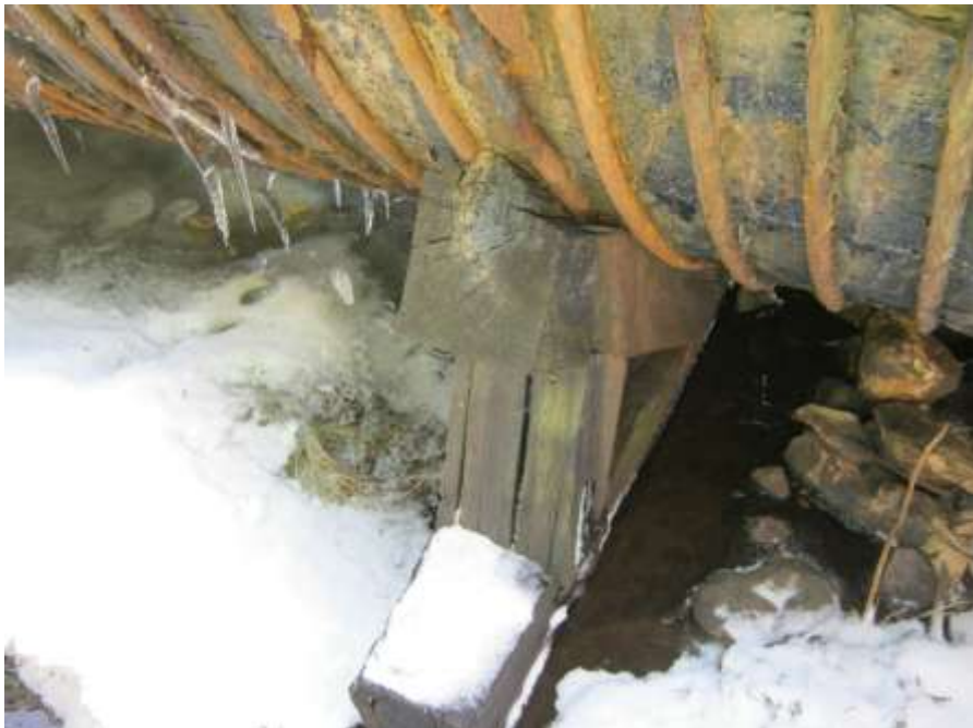
Photo C-19: Deteriorated cradle
