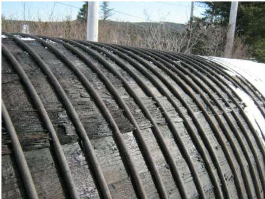
Photo C-23: Example of delaminated stave and crushing under the bands
