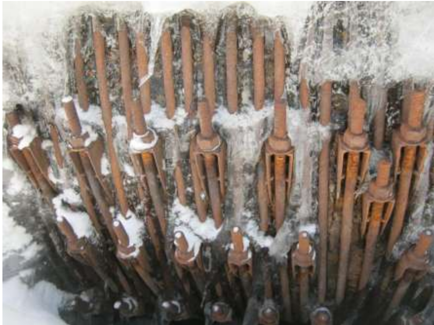
Photo C-16: Bands near downstream end of wood stave penstock
