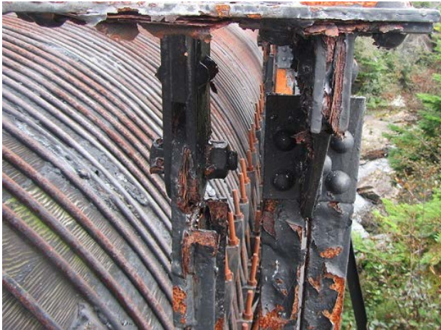
Photo No. 2.4.1.5 – Rust and Scaling on South-Top Chord Connection, Typical
