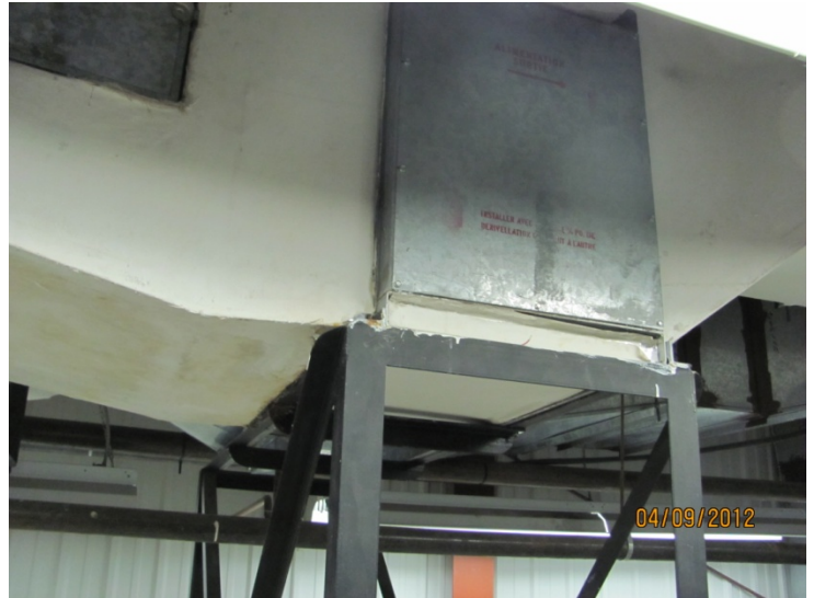
Existing Locker Room Built-Up HRU Unit
