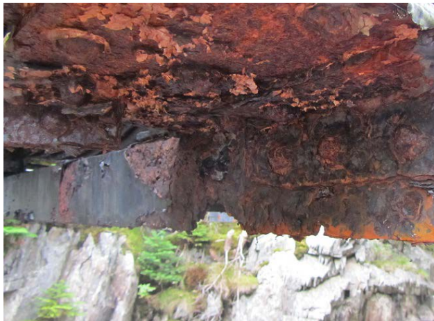
Photo No. 2.4.1.11 – Rust and Scaling on Bottom Chord Connection, Typical
