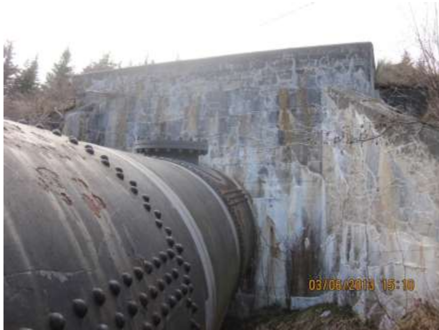
Figure 5: Deteriorated Anchor Block at Transition
