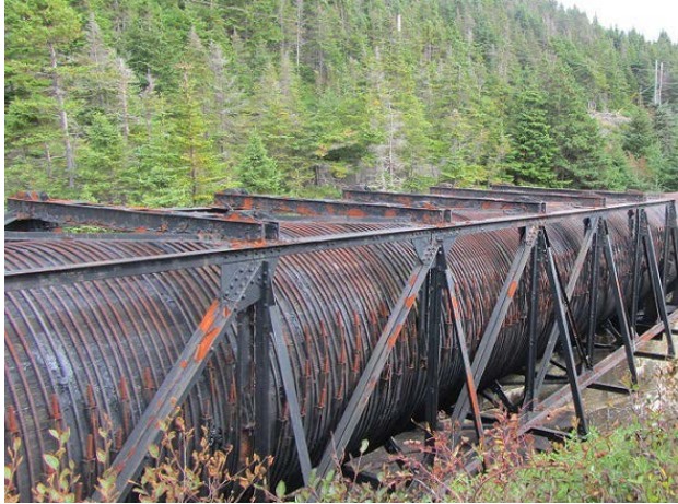
Photo No. 2.4.1.1 – Overall Penstock Truss Structure
