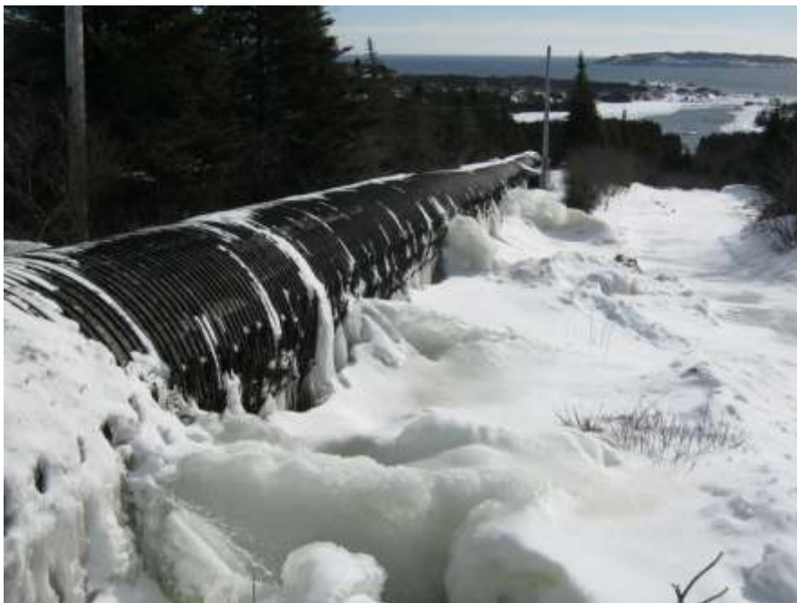
Photo C-24: Penstock immediately downstream of surge tank, showing leakage and sagging
