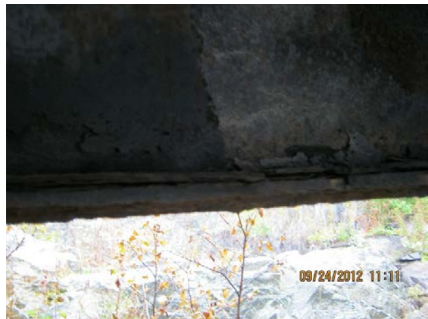
Photo No. 2.3.1.2 - Severe Scaling on Beams, Typical
