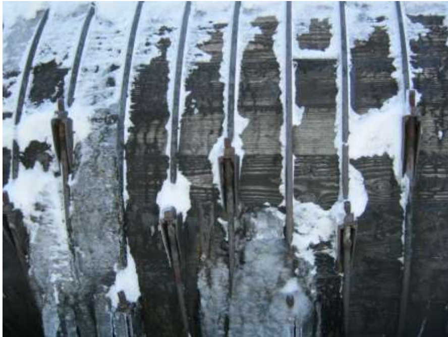
Photo C-48: Typical condition of wood stave preservative treatment upstream of highway crossing
