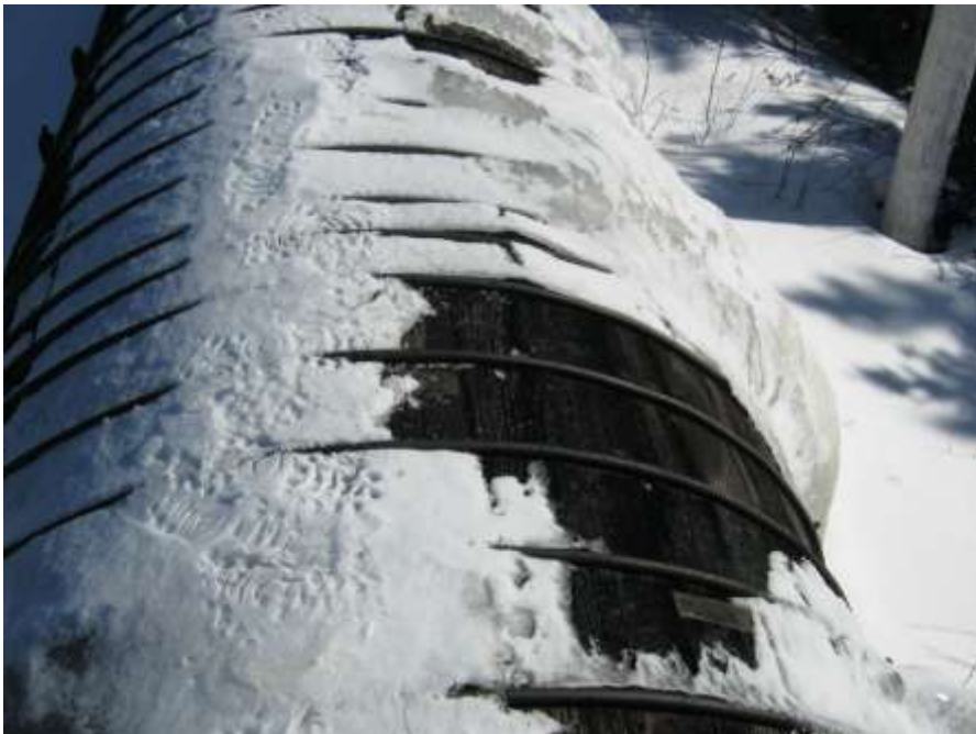
Photo C-61: Damaged ends of wood stave
