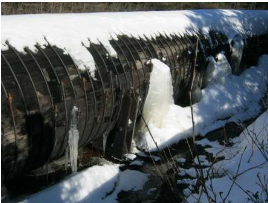
Photo C-57: Poor drainage of penstock bed
