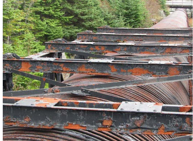
Photo No. 2.4.1.2 – Rust on Top Chord Members, Typical
