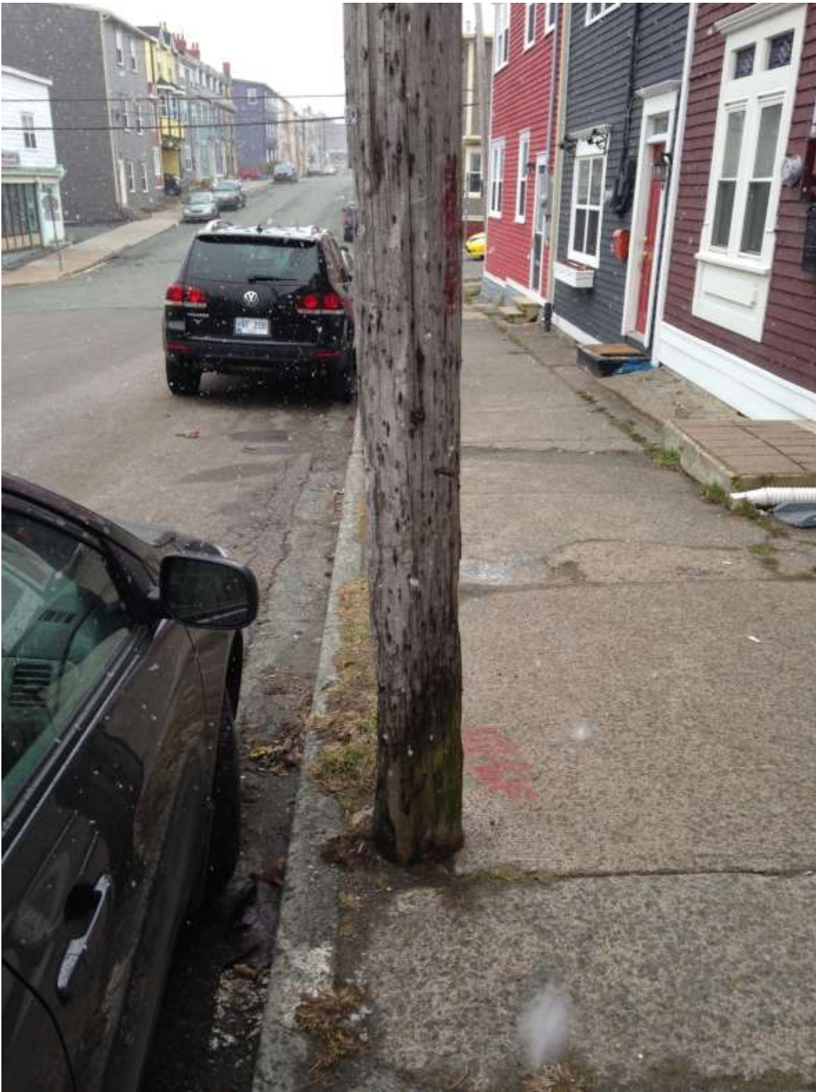
Figure 4 - Loss of Pole Diameter at Base
