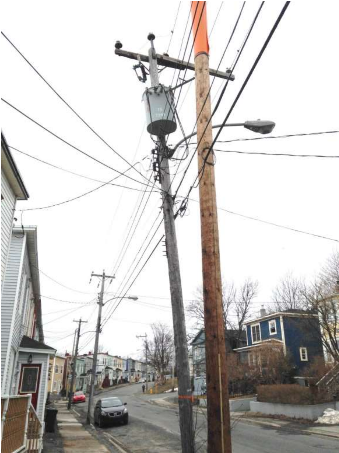
Figure 8 - Broken Crossarm, Leaning Pole, and Pole Replacement in Progress
