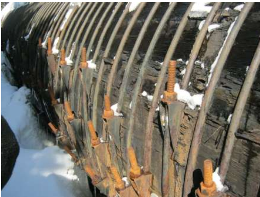
Photo C-31: Deteriorated staves upstream of surge tank (typical)
