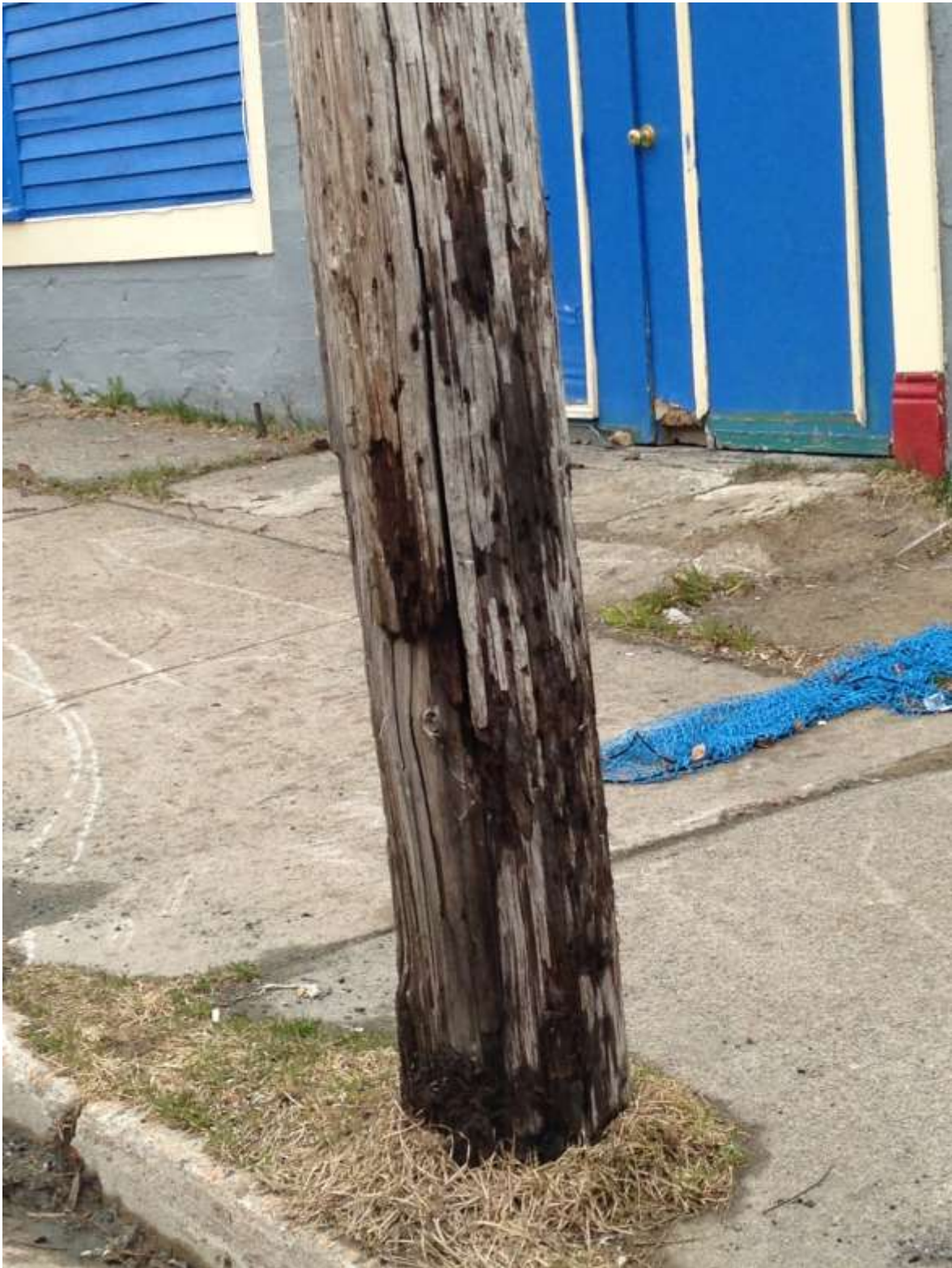
Figure 6 - Deteriorated Pole
