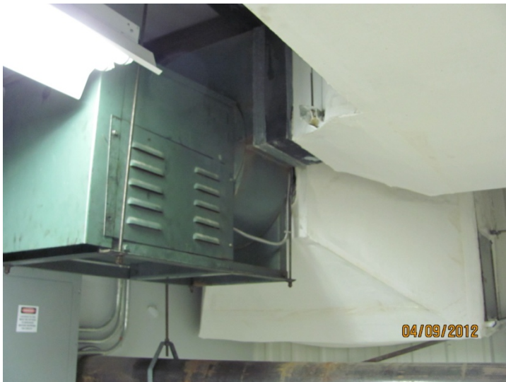
Existing Locker Room Built-Up HRU Unit
