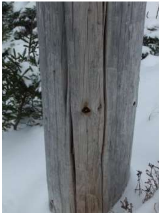
Figure 30 – Pole Shell Separation
