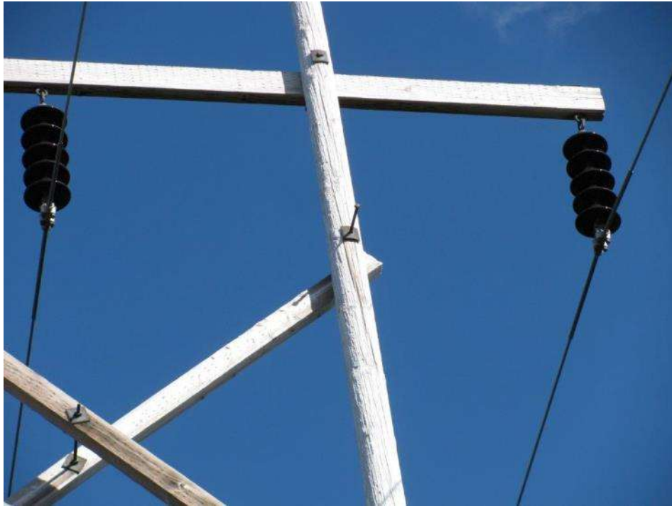
Figure 45 – Bolt No Longer Securing Cross Brace
