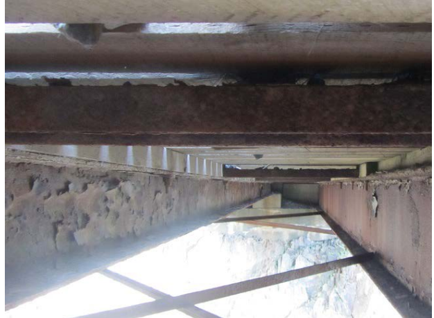
Photo No. 2.3.1.4 – Severe Rust and Scaling on Channels, Typical
