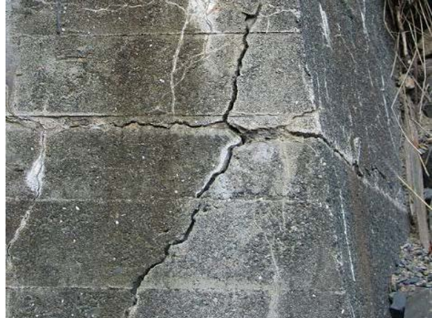
Photo No. 2.2.1.8 – Significant Cracks and Efflorescence, Concrete Abutment
