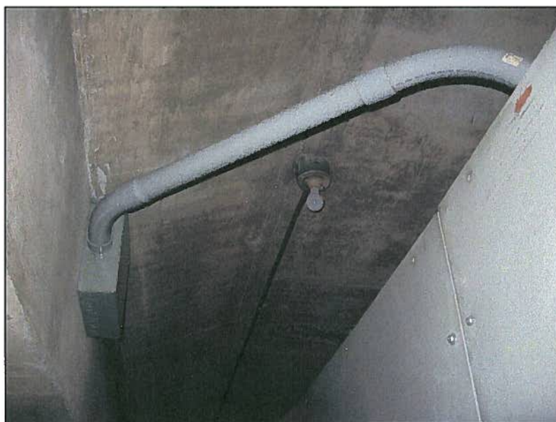
Picture 18: Fibre Optic conduit leaving switchgear.
