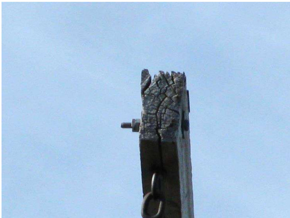
Figure 36 – Deteriorated Crossarm
