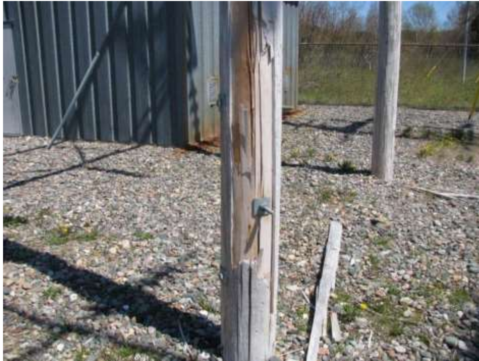
Figure 37 – Bolts Keeping Broken Pole Together
