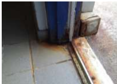
Figure 3 - Corroded Door Frame
