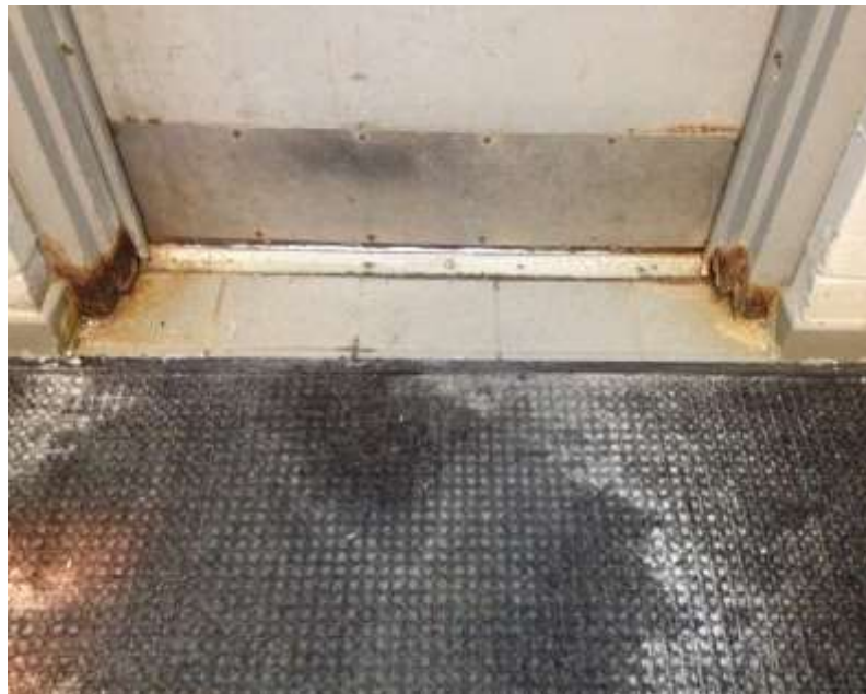
Figure 5 - Corroded Frame (NOTE: Air gap between door and frame)
