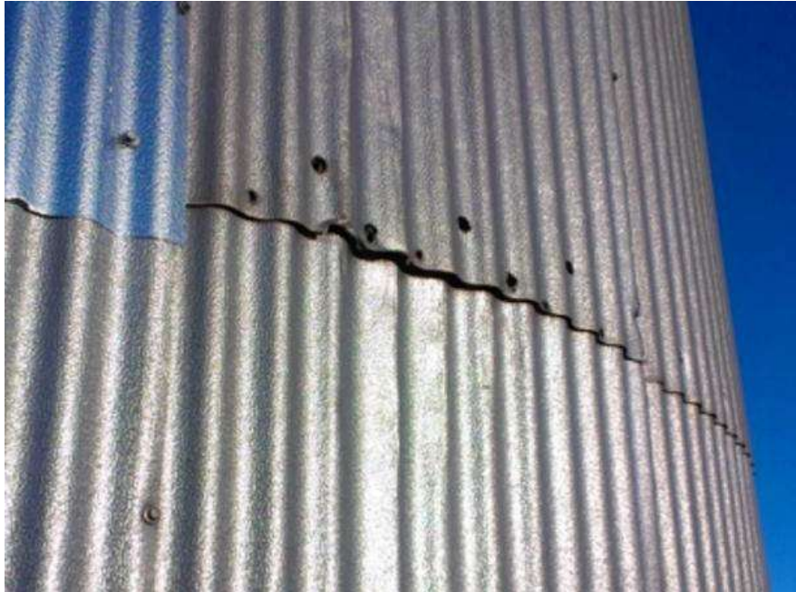
Figure 30: Screws Pulled Through Cladding
