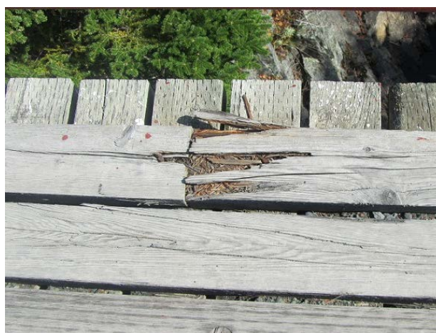
Photo No. 2.3.1.10 – Slight Rotting on Timber Raceway
