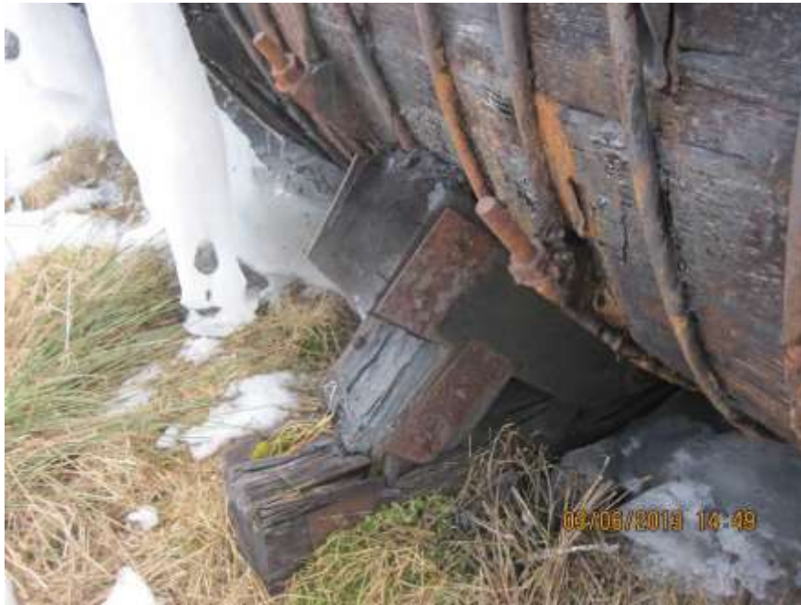
Figure 11: Deteriorated Cradle with Previous Steel Plate Reinforcement
