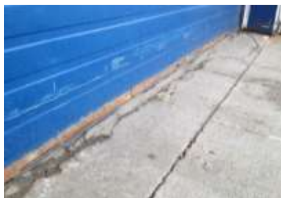
Figure 4 - Corroded Overhead Door
