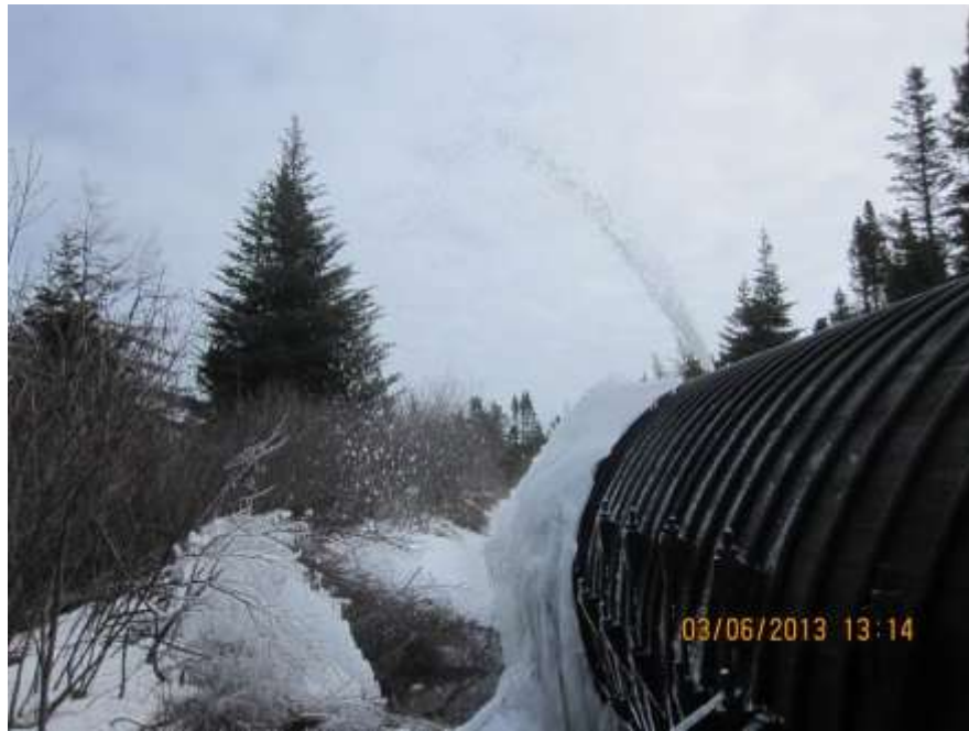
Figure 23: Leakage and Ice Buildup
