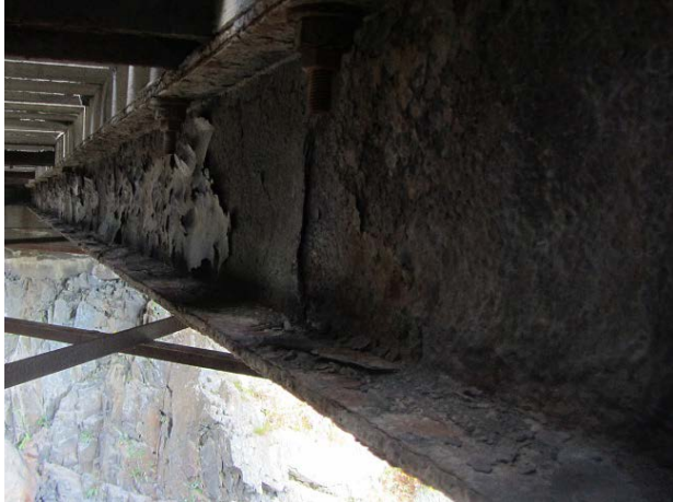
Photo No. 2.3.1.3 – Severe Rust and Scaling on Beams, Typical
