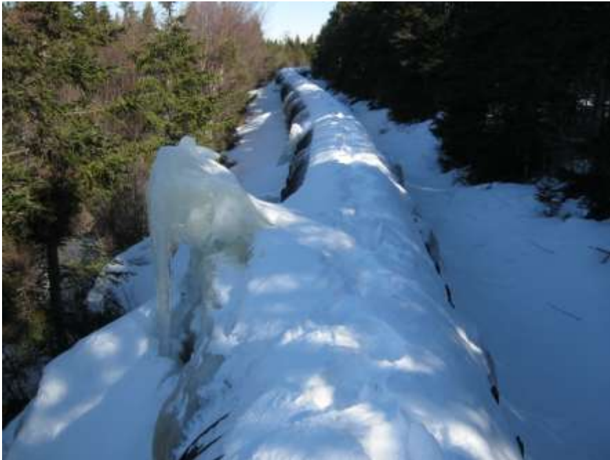
Photo C-58: Areas of significant leakage
