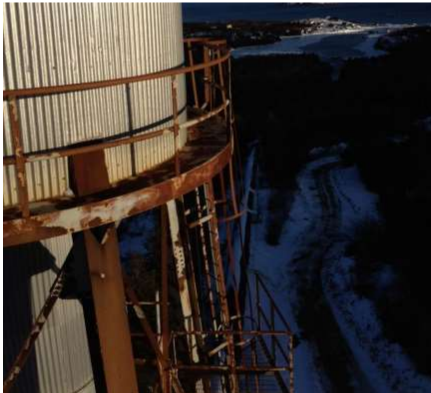
Figure 29: Deteriorated Coating – Deck
