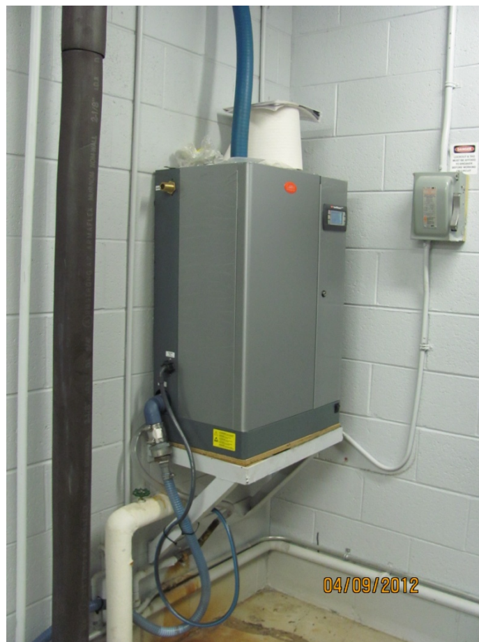
Existing Second Level Humidifier
