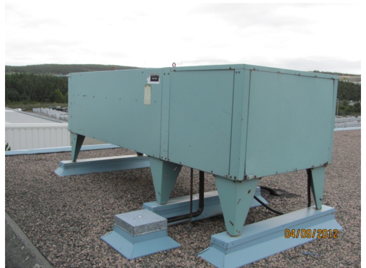
Existing AHU Unit Roof Mounted Condensing Unit
