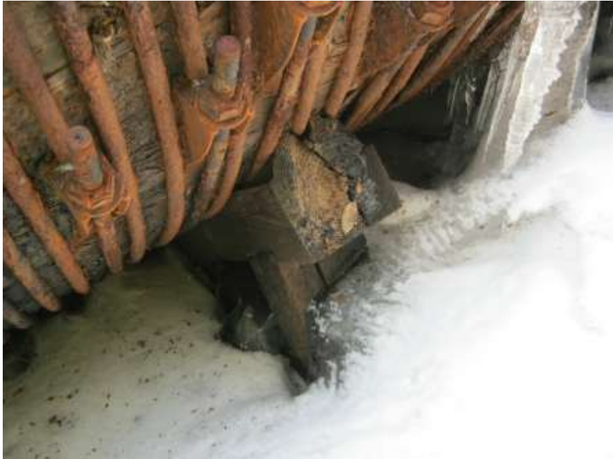
Photo C-18: Deteriorated cradle
