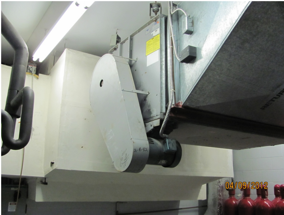
Existing First Floor Return Fan
