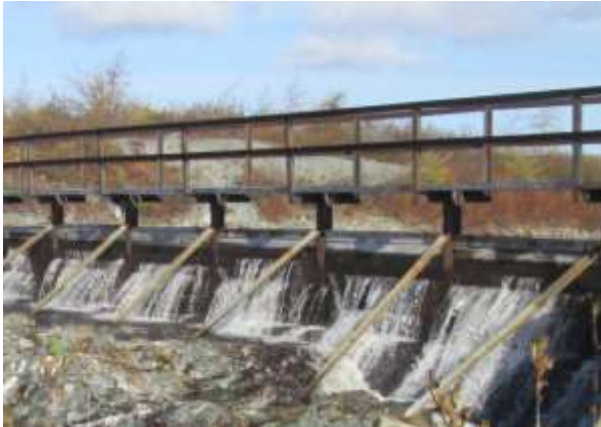
Figure 1 – Slender Structure, Significant Leakage
