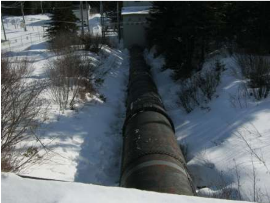
Photo C-1: Overview of steel penstock, as seen from anchor block looking toward powerhouse
