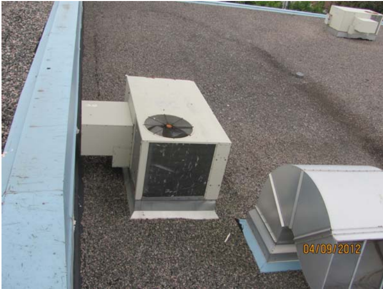
Existing Packaged A/C Units Serving: Stationary, Print Shop and Telecommunications
