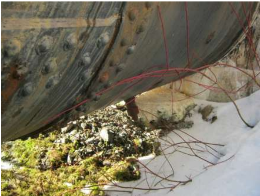
Photo C-10: Tap at underside of penstock near anchor block
