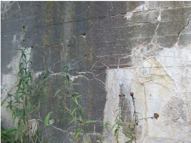
Photo No. 2.2.1.7 – Significant Cracks in Concrete Abutment
