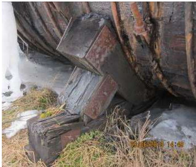
Figure 3 - Deteriorated Cradle
