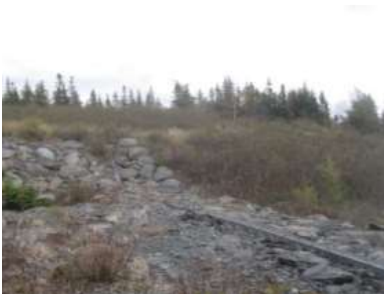
Figure 4 – Undersized Riprap and Damaged Spillway Core
