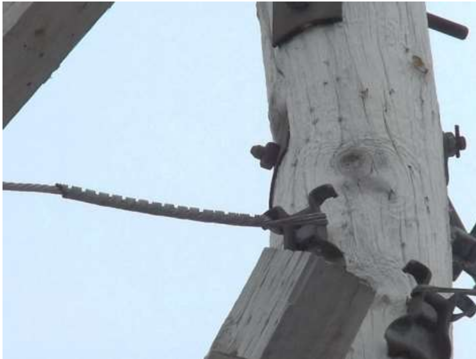
Figure 21 – Pole and Hardware Damage at Guy Wire Attachment
