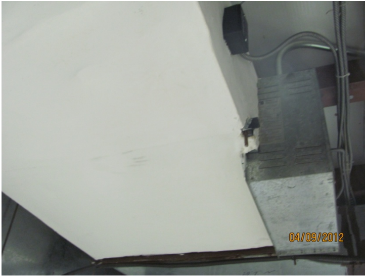
Existing Locker Room Built-Up HRU Unit
