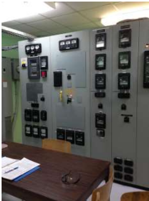
Electromechanical Relay Panels of Transformer, Buses and 110L Protection
