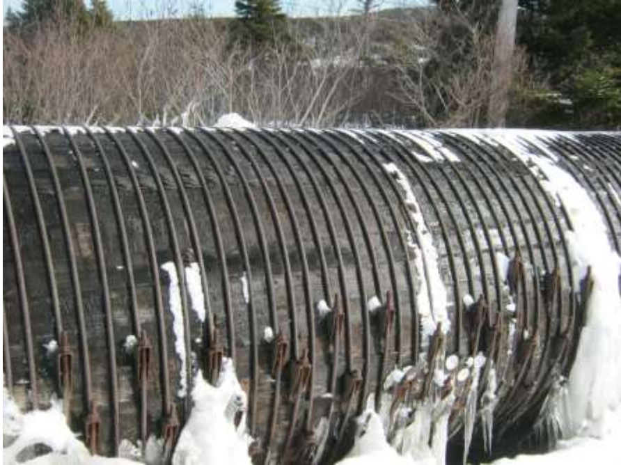
Photo C-22: Example of delaminated stave, and repairs to reduce leakage along the springline
