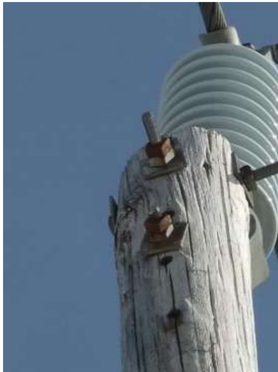
Figure 2 – Deteriorated Pole
