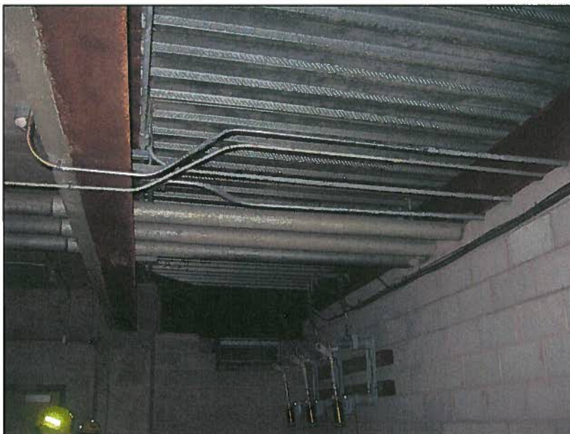
Picture 6: Ceiling without fireproofing
