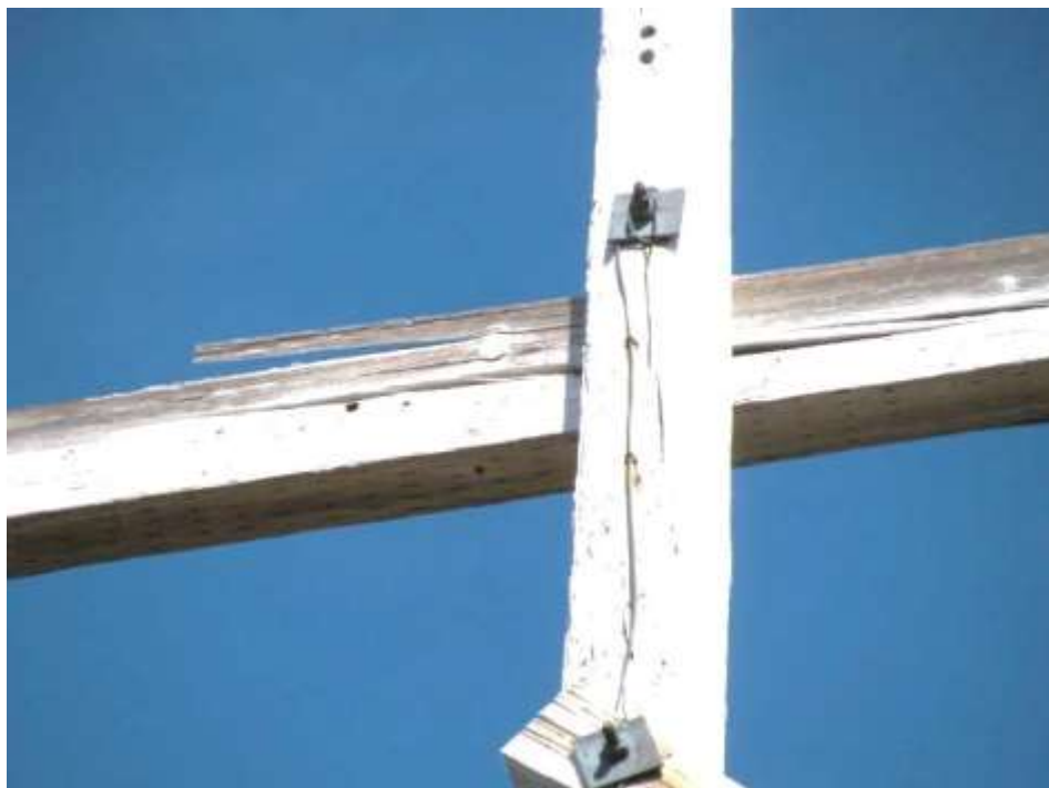
Figure 46 – Broken Crossarm
