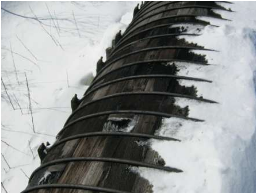
Photo C-54: Delaminated wood stave with broomed end
