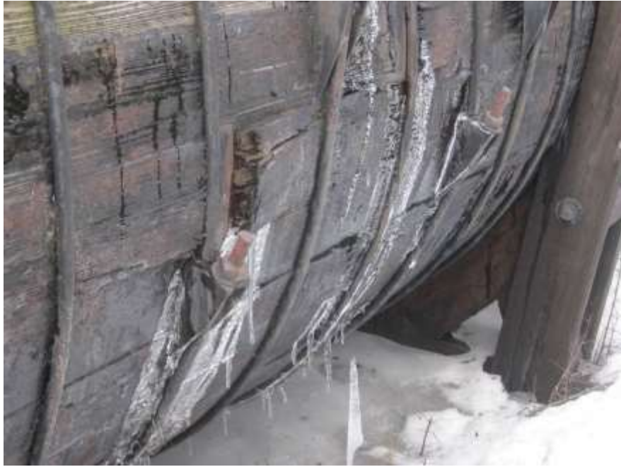
Figure 21: Deteriorated Stave End
