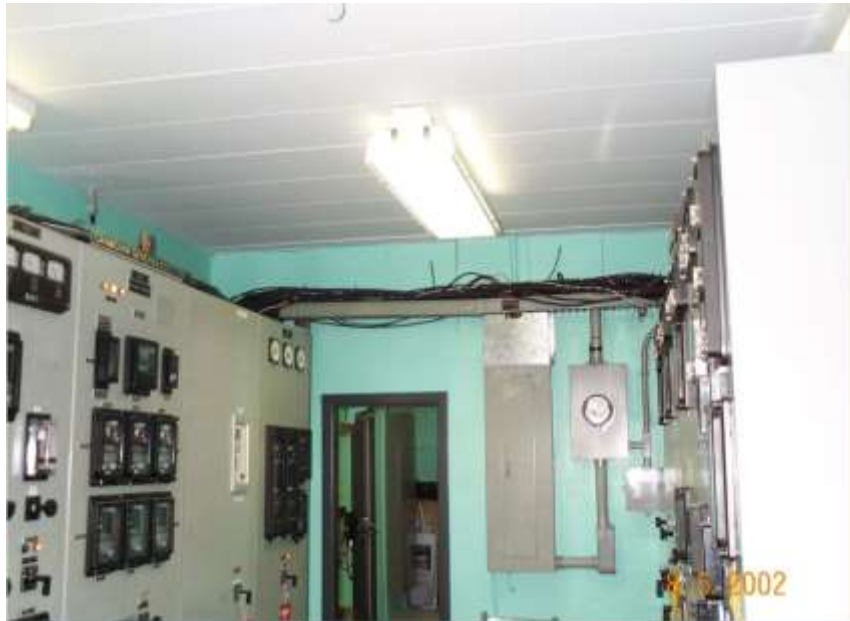
Existing Control Building with Electromechanical Relays
