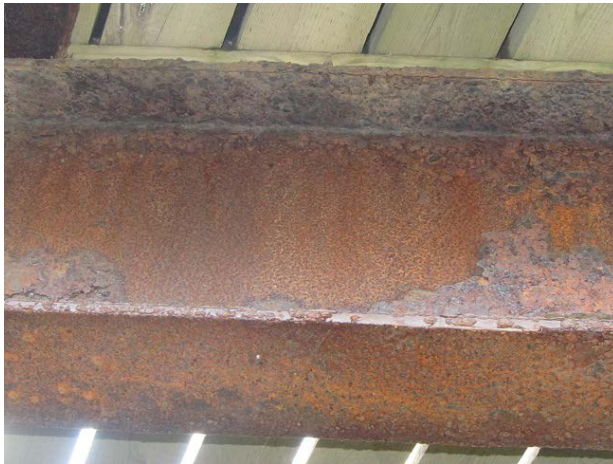
Photo No. 2.2.1.3 – Severe Rust on Beams, Typical
