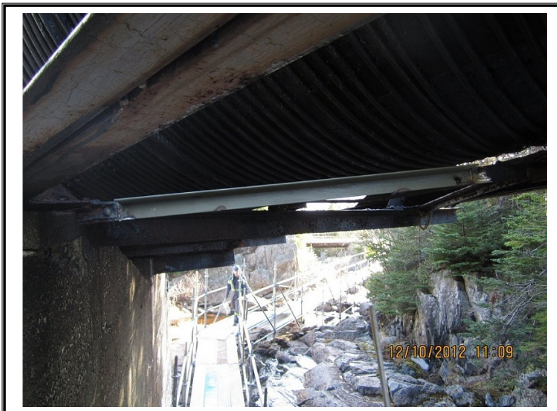
Photo No. 4 – Typical Bottom Truss Horizontal Cross Brace Repair
