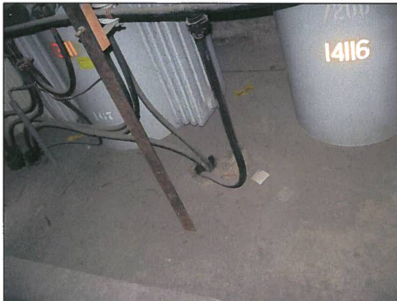
Picture 16: Fibre duct conduit in spill containment
