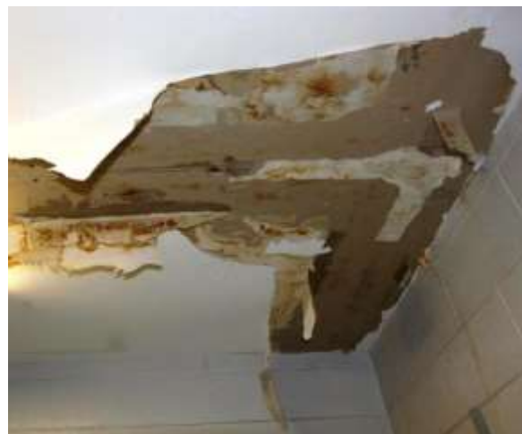
Figure 1 – Damage as a Result of Roof Leakage
