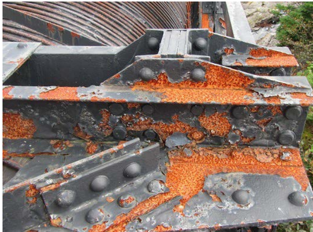
Photo No. 2.4.1.3 – Rust on Top Chord Connection, Typical
