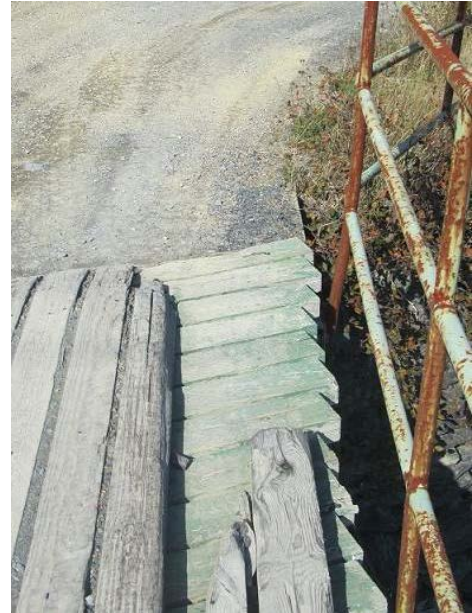
Photo No. 2.2.1.10 – Broken Timber Raceway Members
