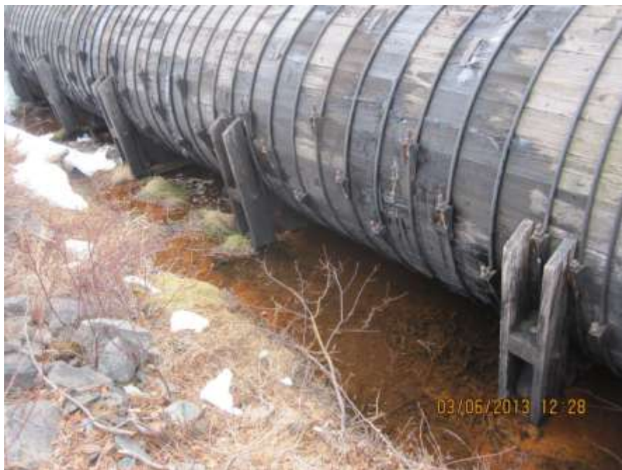
Photo C-63: Poor drainage of penstock bed
