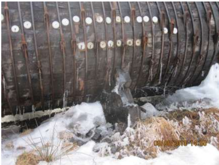
Figure 12: Leak Repair along Springline
