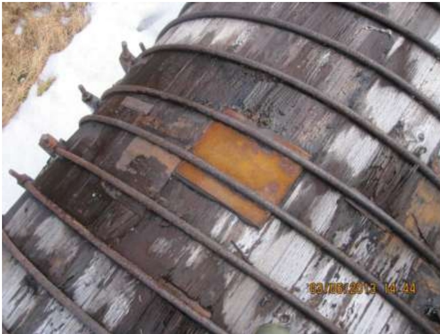
Photo C-50: Repairs and deteriorated staves
