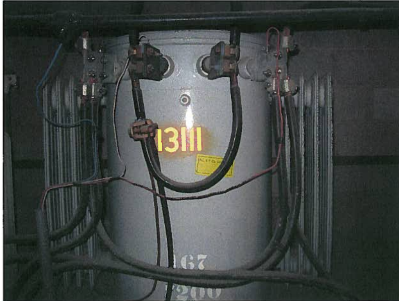
Picture 21: Centre transformer unconnected X2 grounding. Note #10 AWG wiring.
