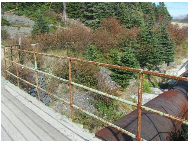
Photo No. 2.2.1.11 – Rust on Handrail
