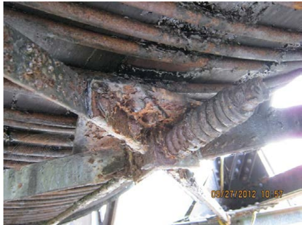
Photo No. 2.4.1.12 – Rust and Scaling on Bottom Chord Cross-bracing Connection, Typical
