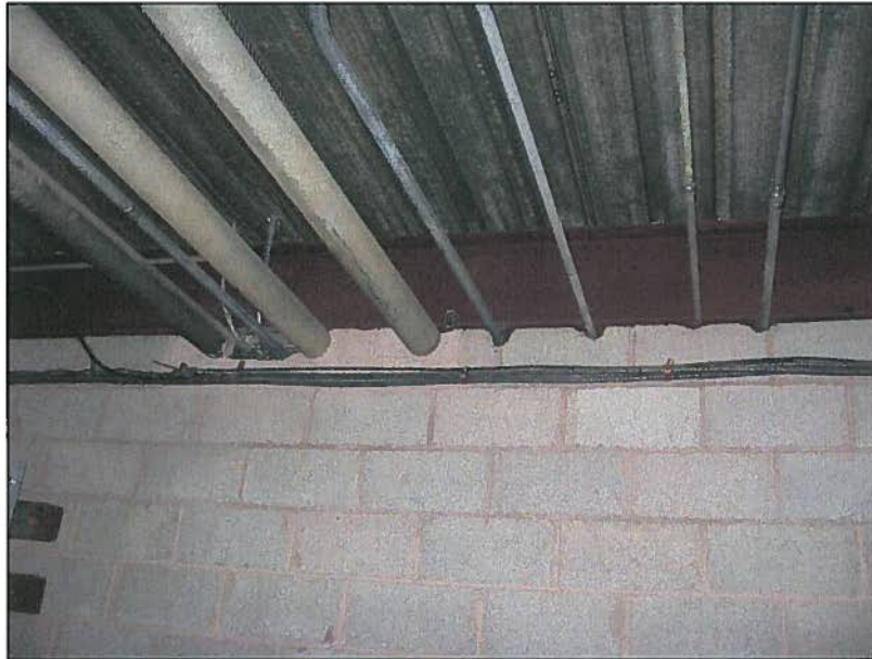
Picture 7: Conduit penetrations without fireproofing sealant.
