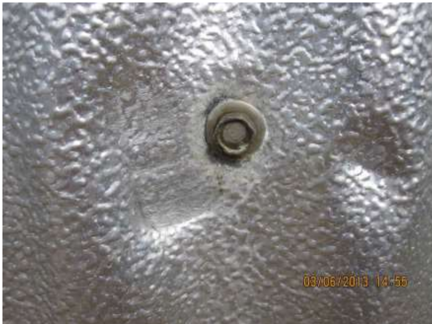
Figure 31: Corrosion at Fastener
