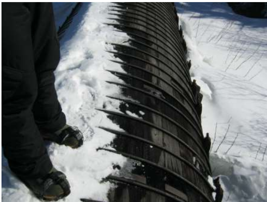
Photo C-55: Typical condition of wood stave preservative treatment
