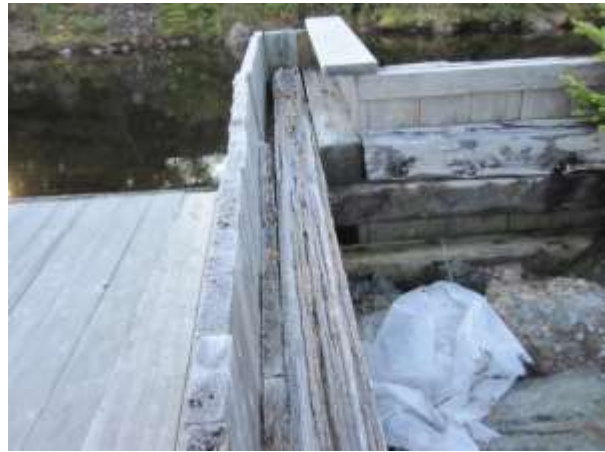
Figure 7 – Deteriorated Timber
