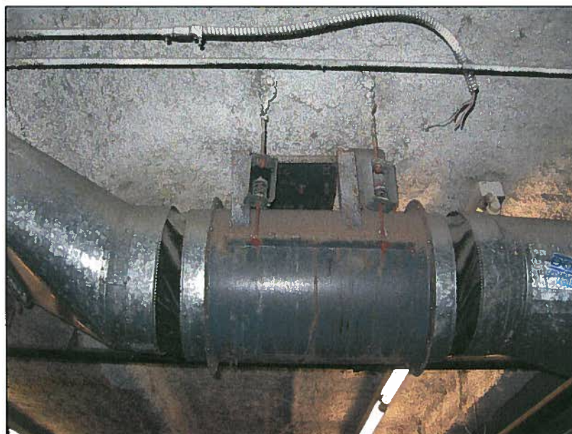
Picture 15: Exhaust ventilation axial fan with empty motor bracket. Note disconnected motor wiring.
