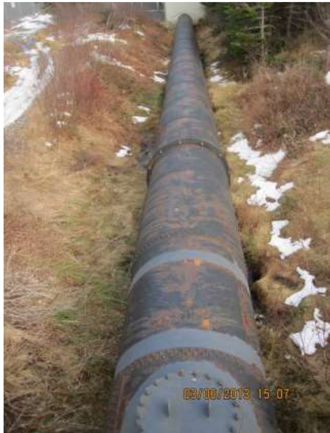
Figure 1: Steel Penstock – Coating Failure
