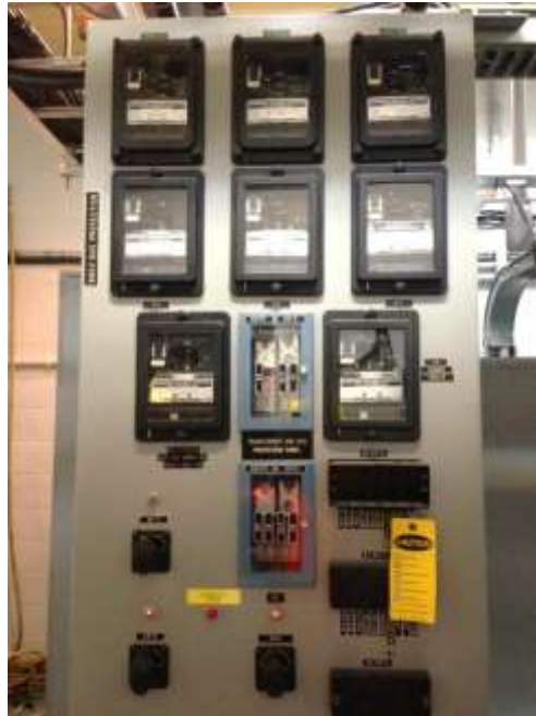
66kV Bus Protection Panel (Electromechanical Relays)
