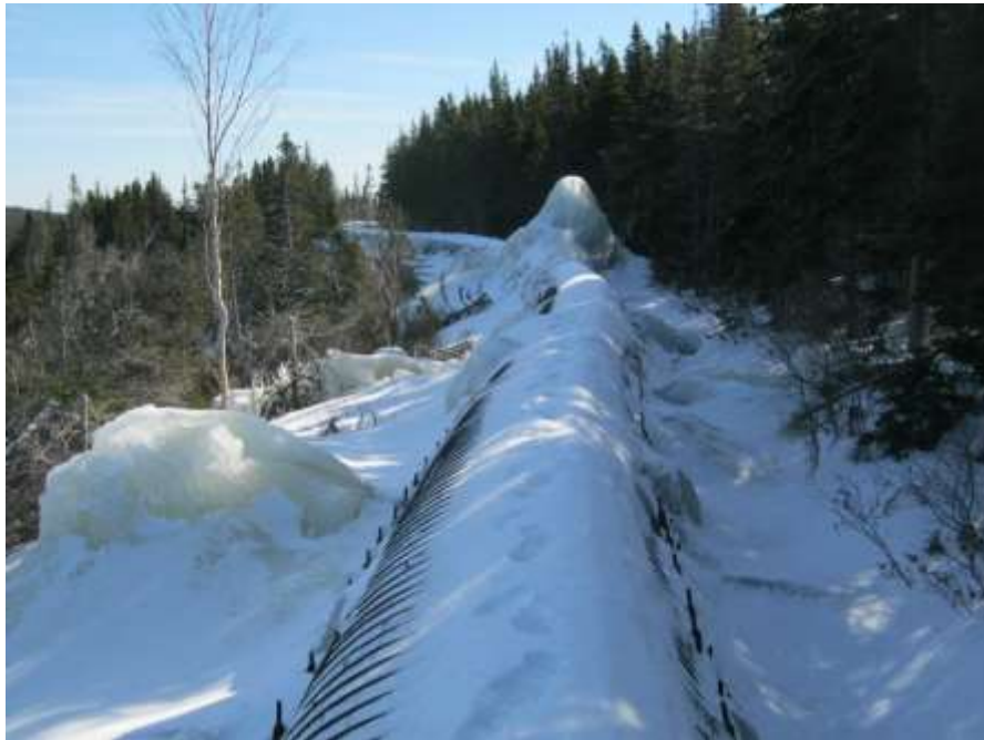
Photo C-38: General view of penstock showing leakage
