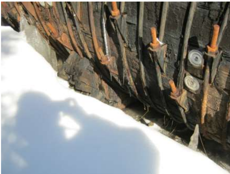
Photo C-30: Deteriorated cradles, staves and patching upstream of surge tank (typical)
