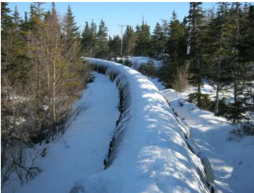
Photo C-59: Leakage along springline of penstock
