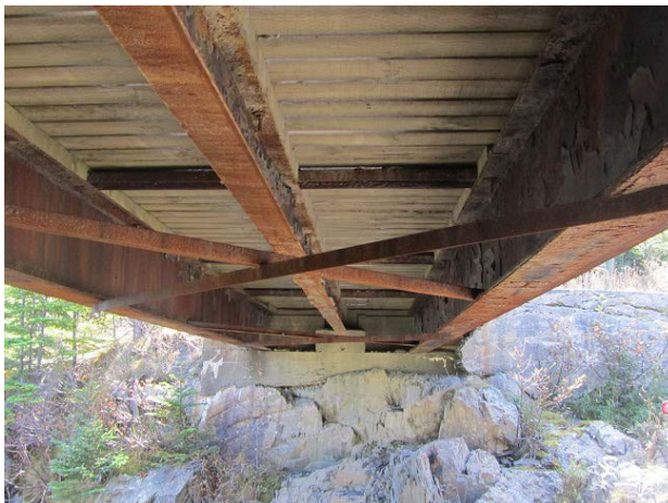
Photo No. 2.3.1.5 – Severe Rust on Angle Cross-bracing, Typical
