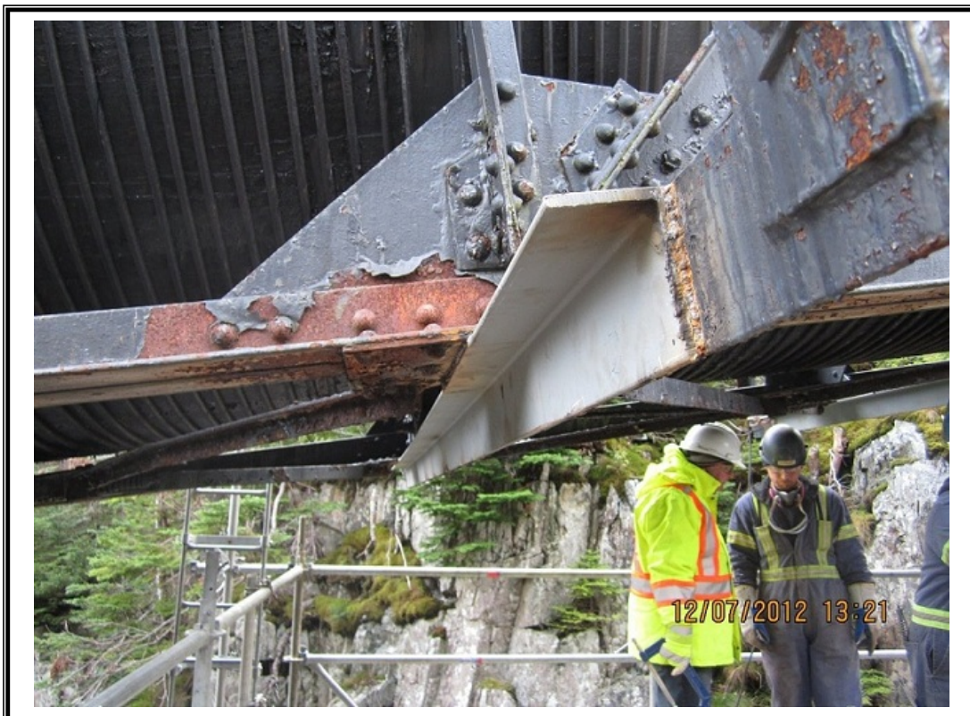
Photo No. 2 – Typical Bottom Truss Transverse Member Repair
