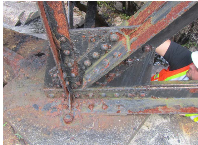
Photo No. 2.4.1.18 – Rust and Scaling on Abutment Baseplate, Typical
