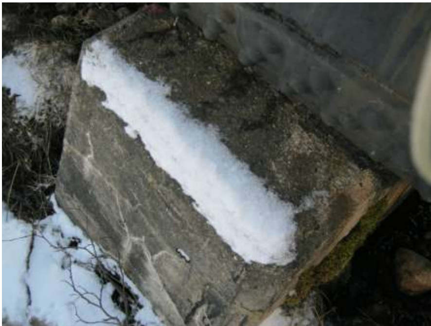
Photo C-12: Concrete cradle support showing signs of deterioration
