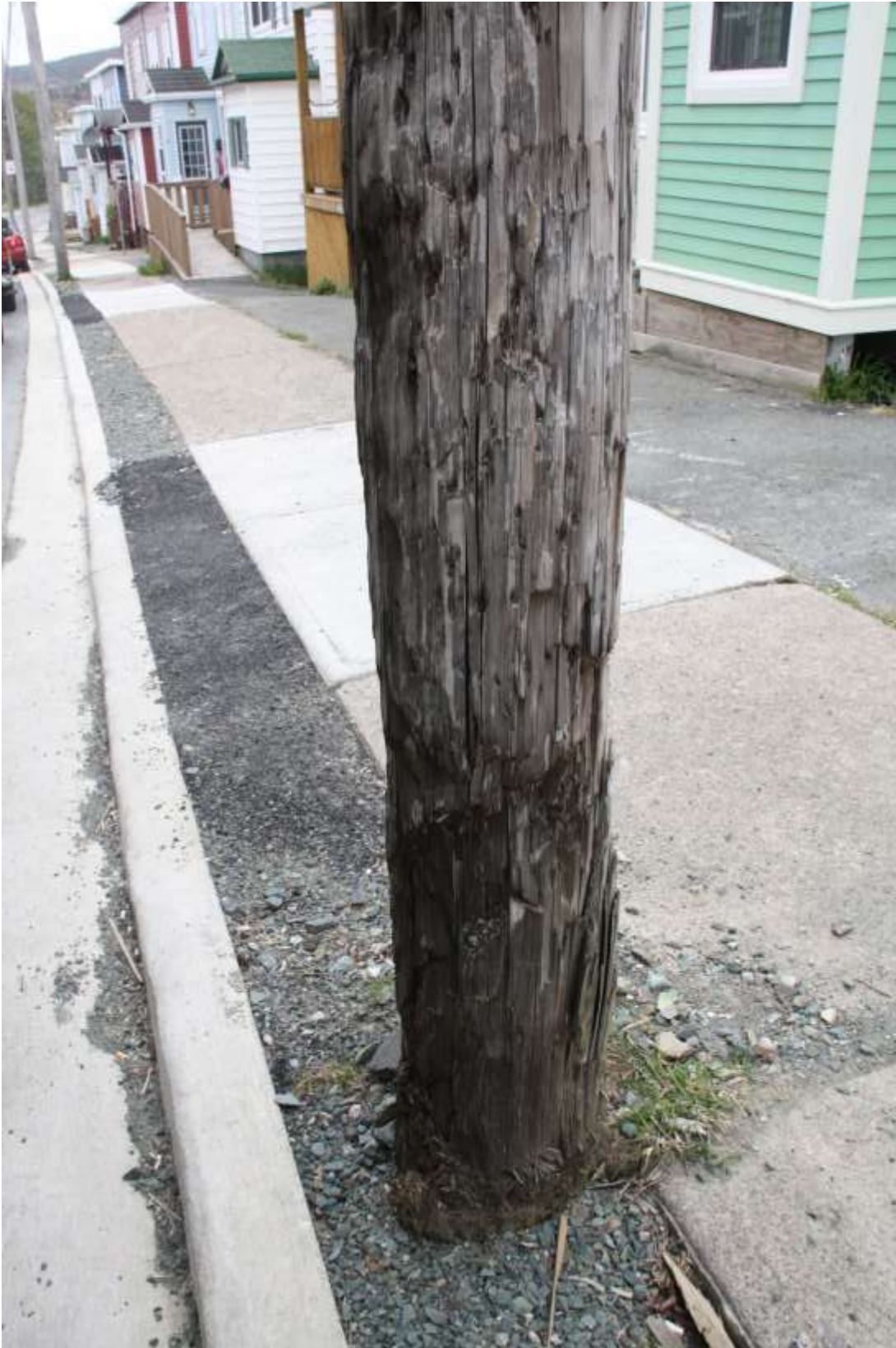
Figure 5 – Pole Damaged by Vehicles
