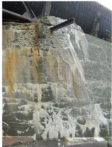
Photo No. 2.4.1.16 – Significant Cracks and Efflorescence, Concrete Abutment, Typical
