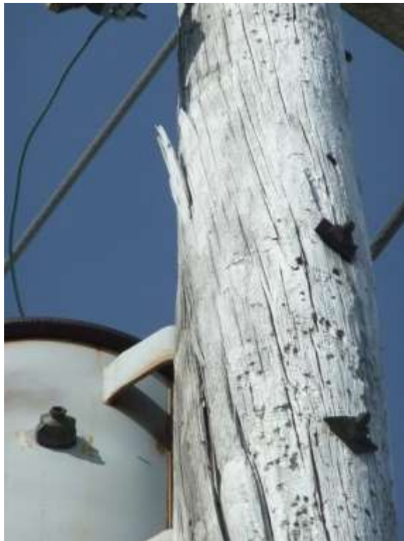
Figure 4 – Pole Shell Damage
