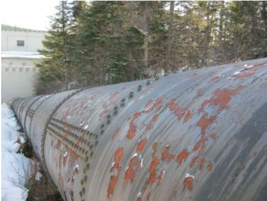
Photo C-5: General condition of steel penstock shell
