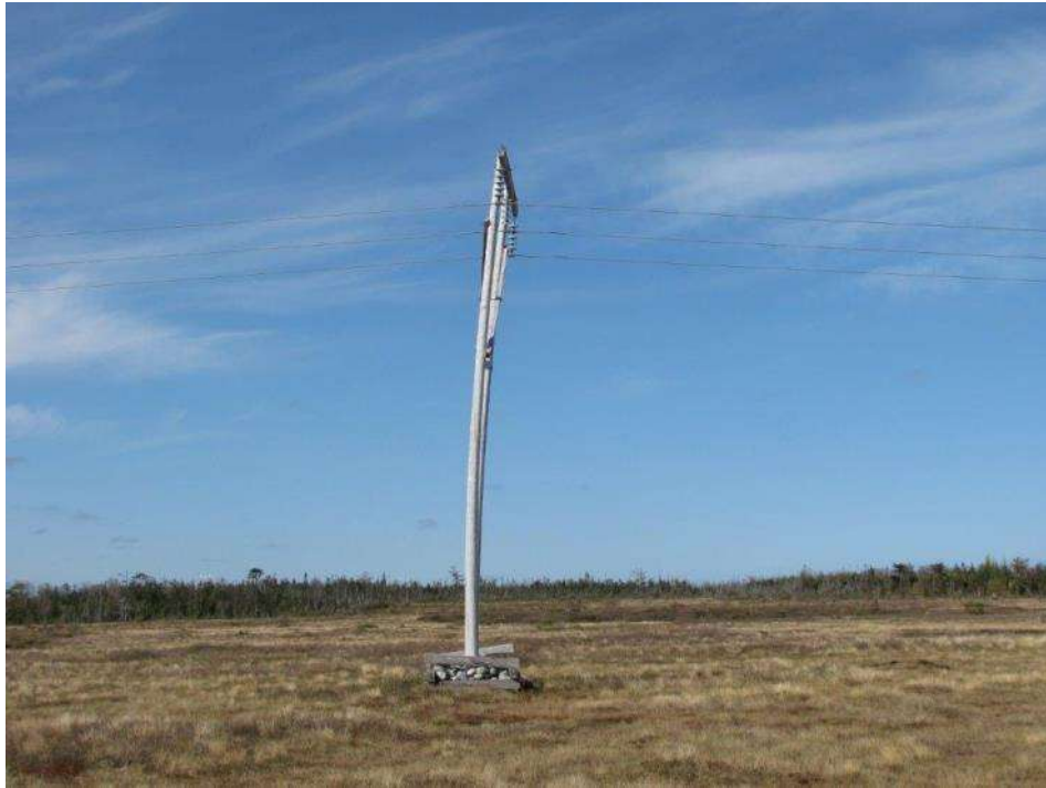
Figure 43 – Bent Structure
