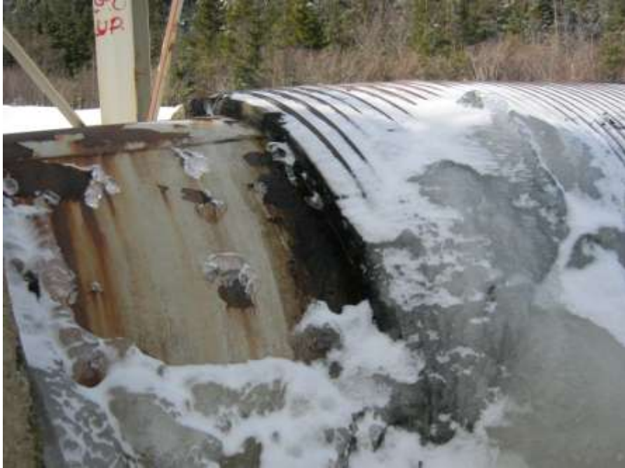
Photo C-28: Wood stave connection to upstream end of surge tank tee
