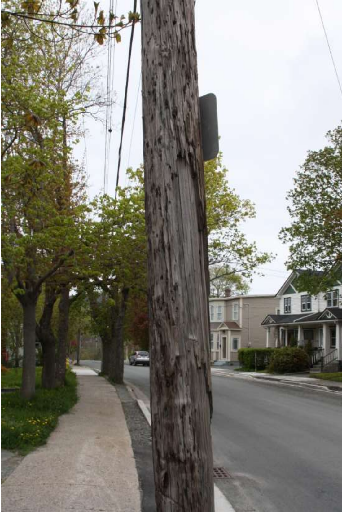
Figure 4 - Outer Shell Damage
