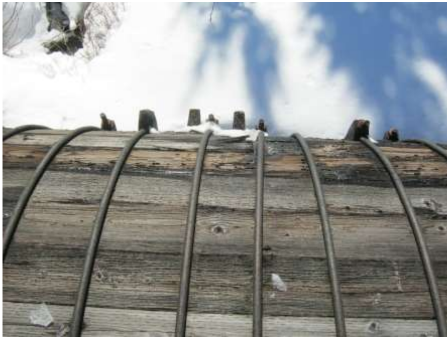
Photo C-62: Typical damaged ends of wood stave and poor preservative treatment
