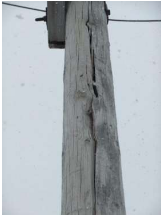
Figure 23 – Significant Pole Checking Due To Shell Separation
