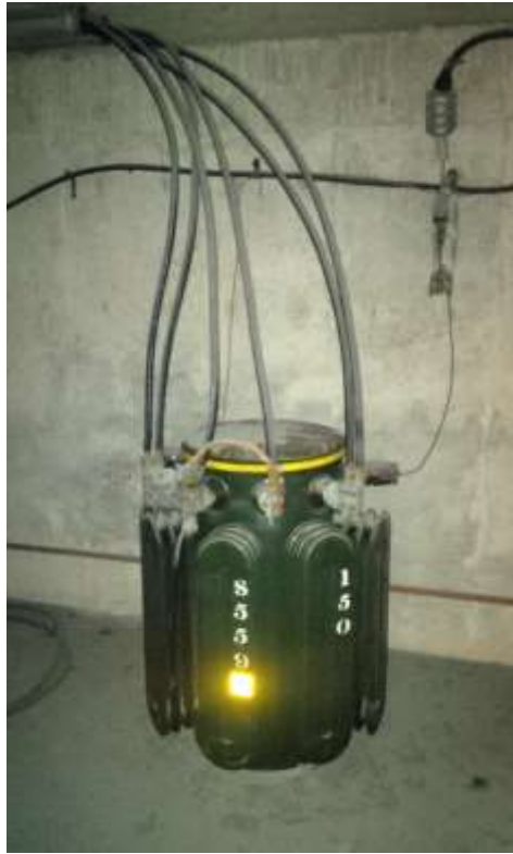
Figure 7: Imperial Optical Vault Transformer
