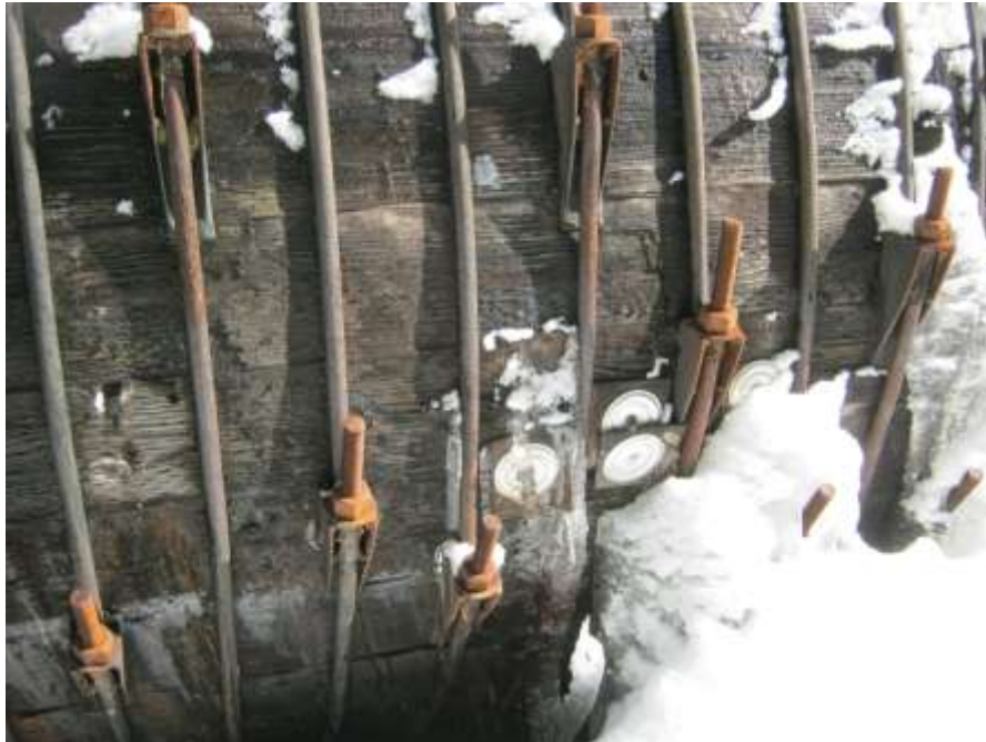
Photo C-32: Deteriorated staves and patching on springline upstream of surge tank (typical)
