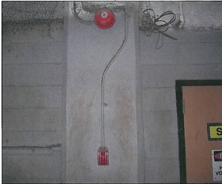
Picture 10: Disconnected receptacle wiring
