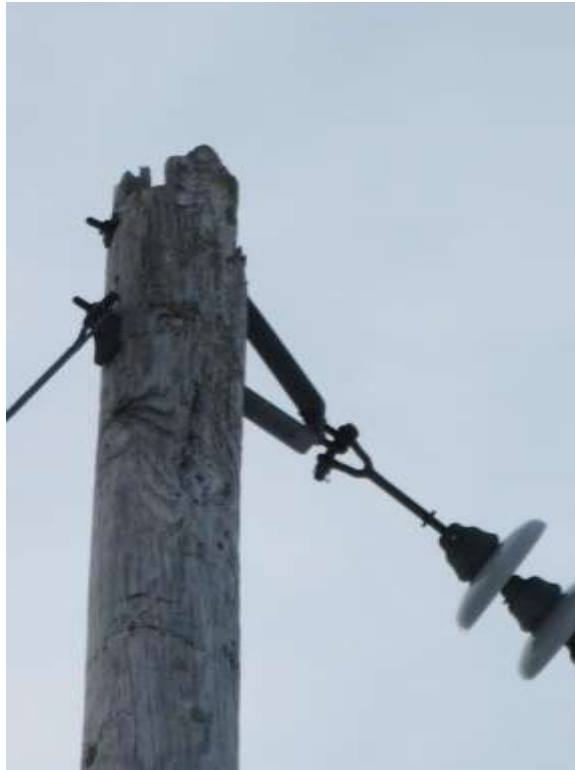
Figure 7 – Deteriorated Pole Top
