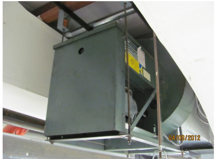
Existing Locker Room Built-Up HRU Unit
