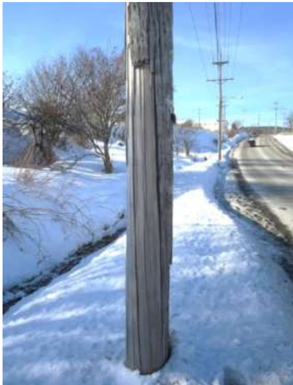
Figure 6 – Damaged Pole
