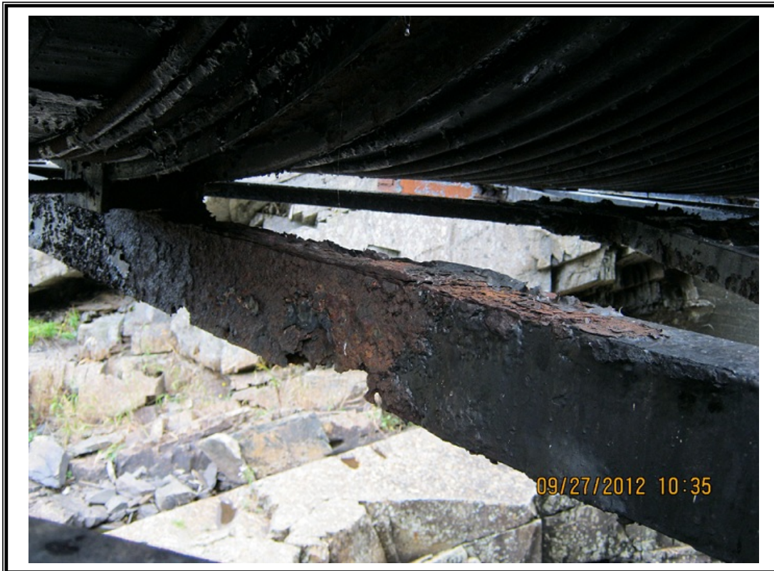
Photo No. 1 – Severely Deteriorated Bottom Truss Transverse Member
