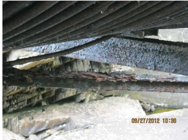
Photo No. 2.4.1.10 – Rust and Scaling on Bottom Chord Cross-bracing Member, Typical
