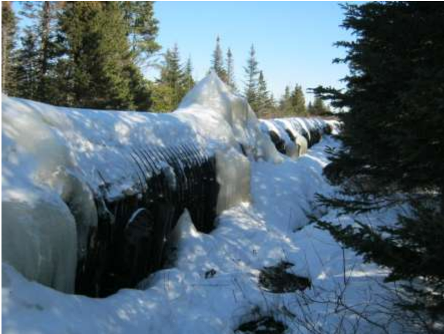
Photo C-56: Widespread leakage along springline of pipe
