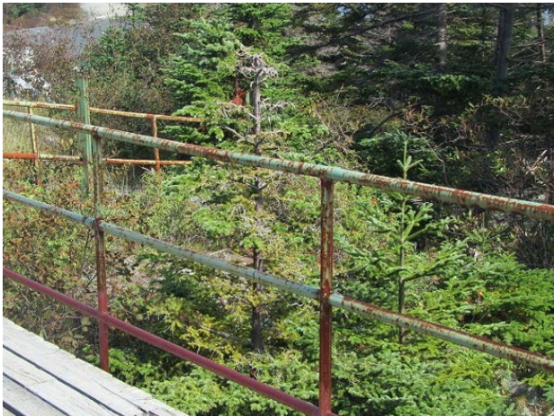
Photo No. 2.3.1.12 – Rust on Handrail
