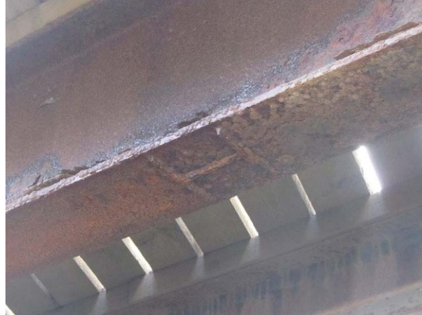
Photo No. 2.2.1.6 – Remaining Section of Steel Column, Typical
