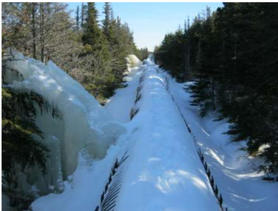
Photo C-41: General view of penstock showing leakage
