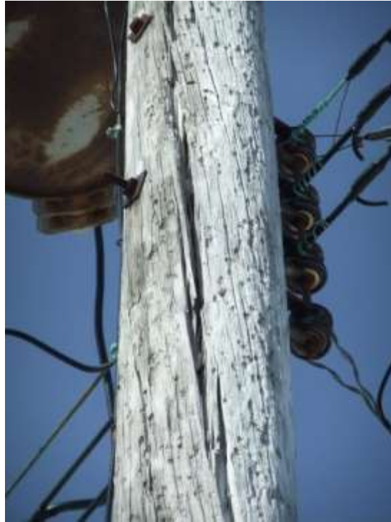
Figure 1 – Severe Checking in Pole
