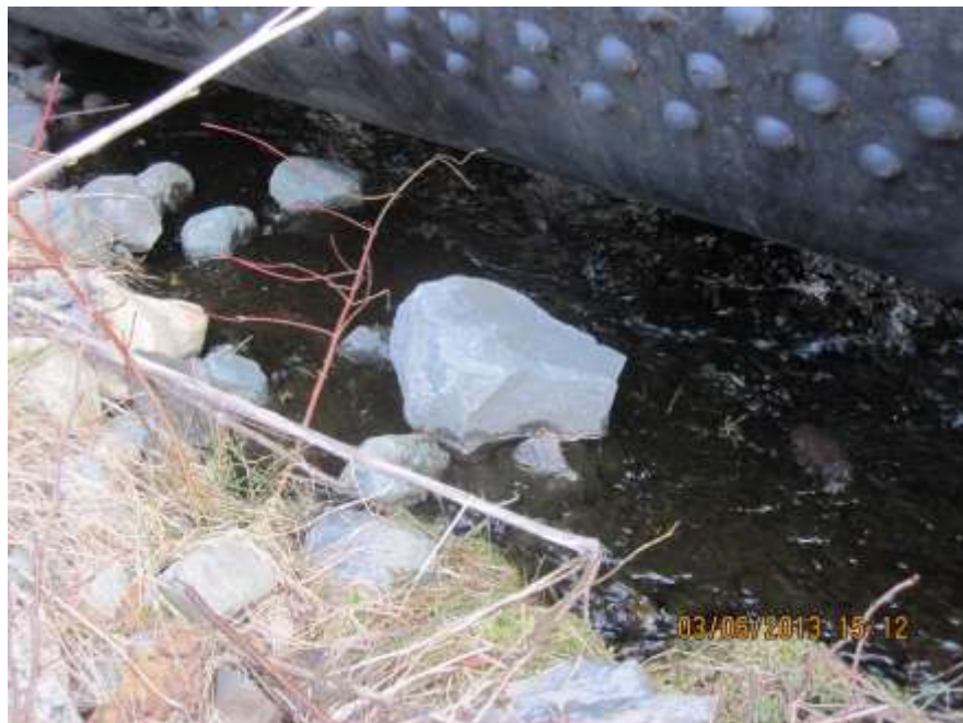
Figure 4: Water Flowing Along Penstock Bed
