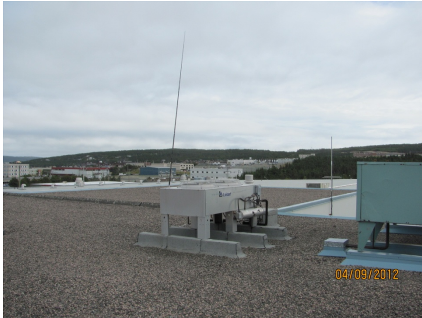
Existing Server Room Roof Mounted Condensing Unit
