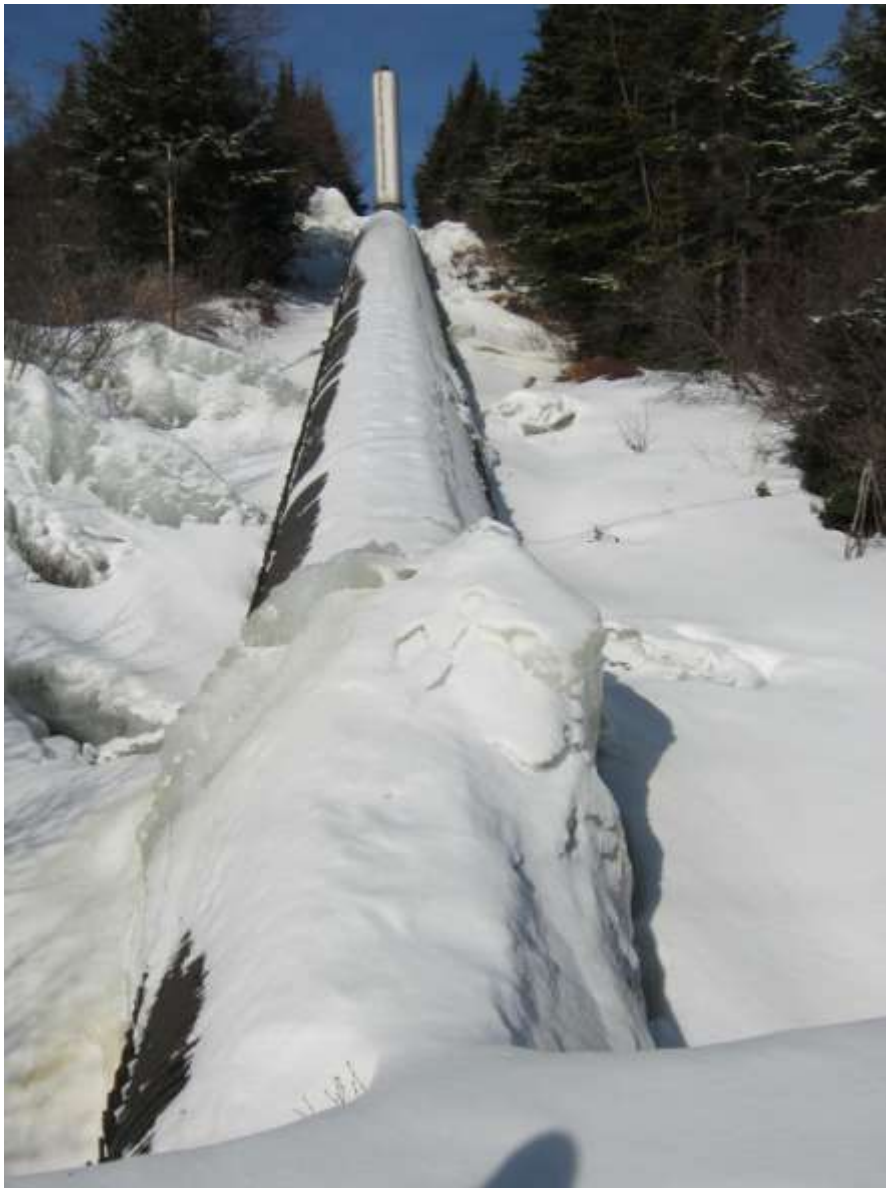
Photo C-15: Looking upstream at wood stave penstock from anchor block to surge tank
