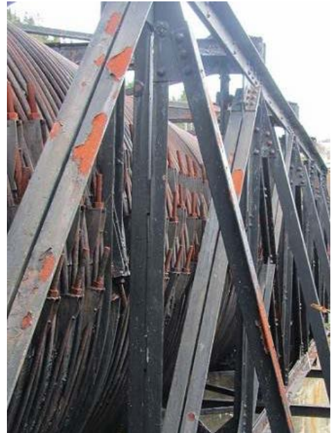
Photo No. 2.4.1.4 – Rust on South Chord Member, Typical
