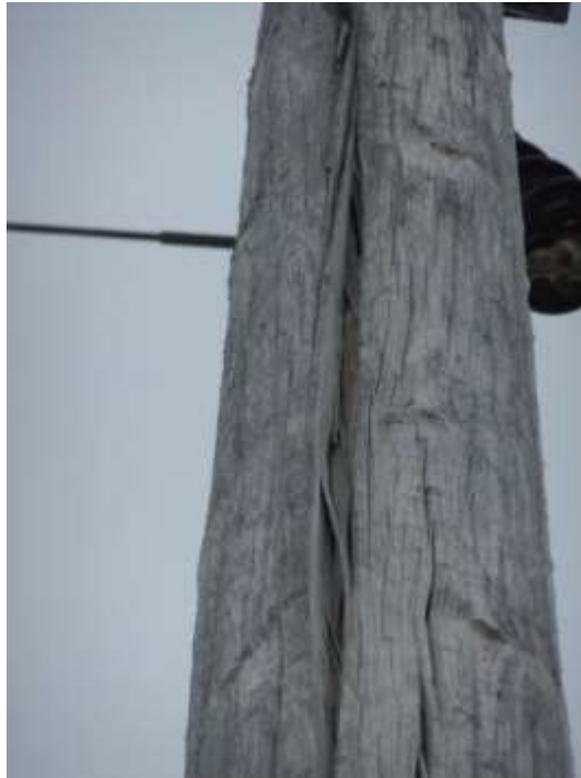
Figure 29 – Deep Checking Due to Shell Separation
