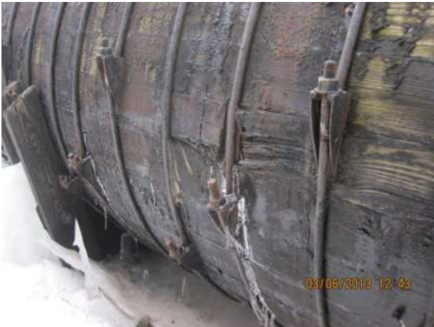
Photo C-51: Damaged ends of wood staves
