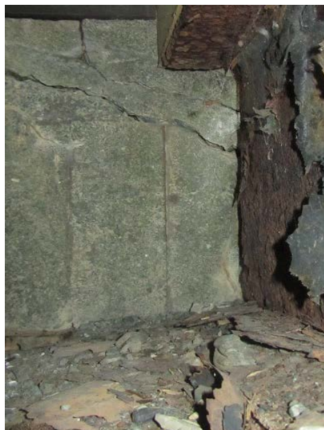
Photo No. 2.3.1.7 – Significant Cracks in Concrete Abutment
