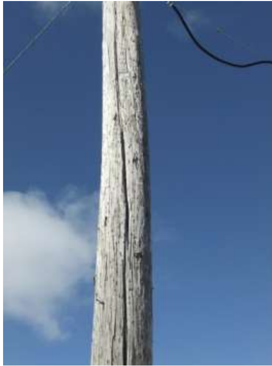
Figure 9 – Pole Checking
