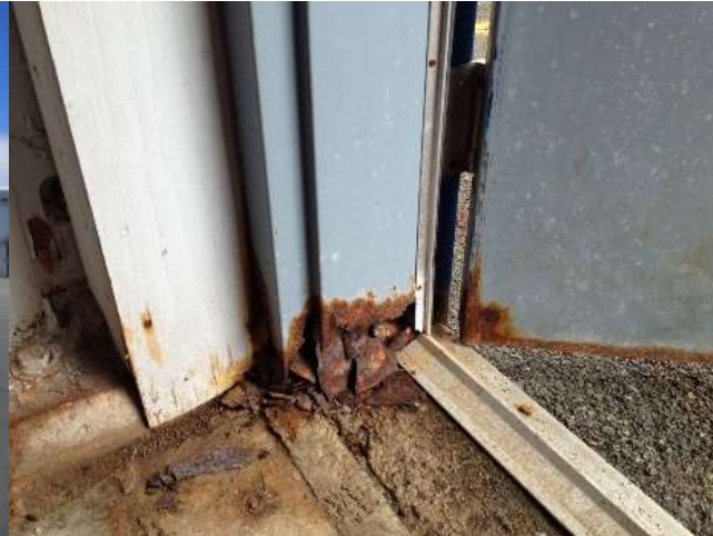
Figure 14 - Corroded Door and Frame
