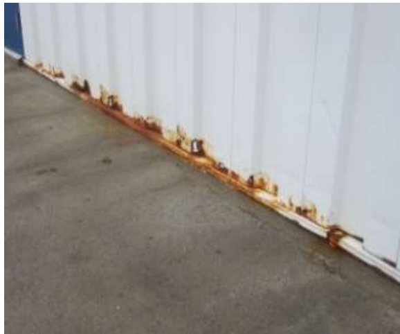
Figure 2 - Corroded Siding
