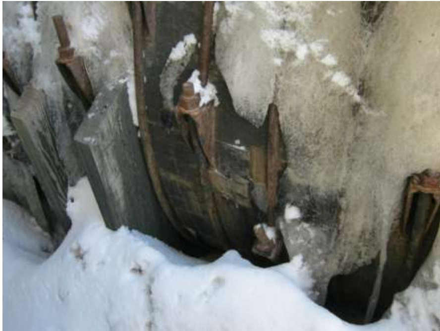
Photo C-46: Typical damaged end of stave
