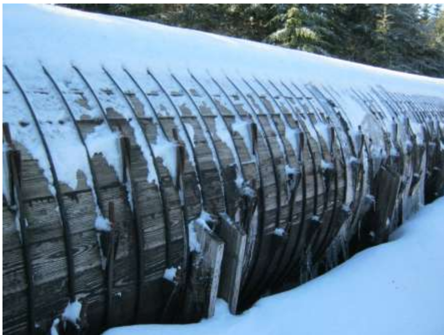
Photo C-47: Typical condition of wood stave preservative treatment upstream of highway crossing
