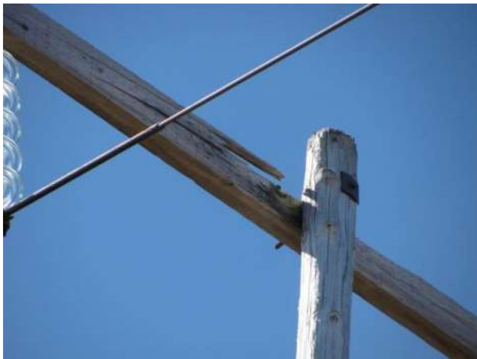
Figure 44 – Broken Crossarm
