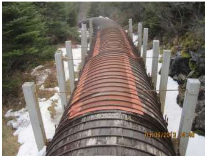
Figure 5 - Additional Support at Blowout
