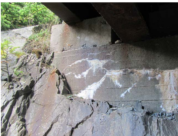
Photo No. 2.3.1.8 – Significant Cracks and Efflorescence, Concrete Abutment
