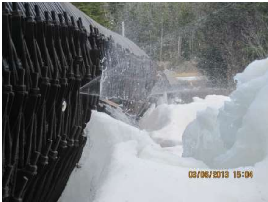
Figure 13: Leaks along Springline
