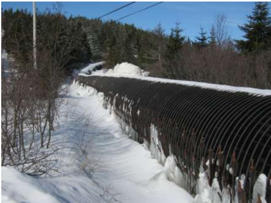
Photo C-29: Wood stave penstock immediately upstream of surge tank
