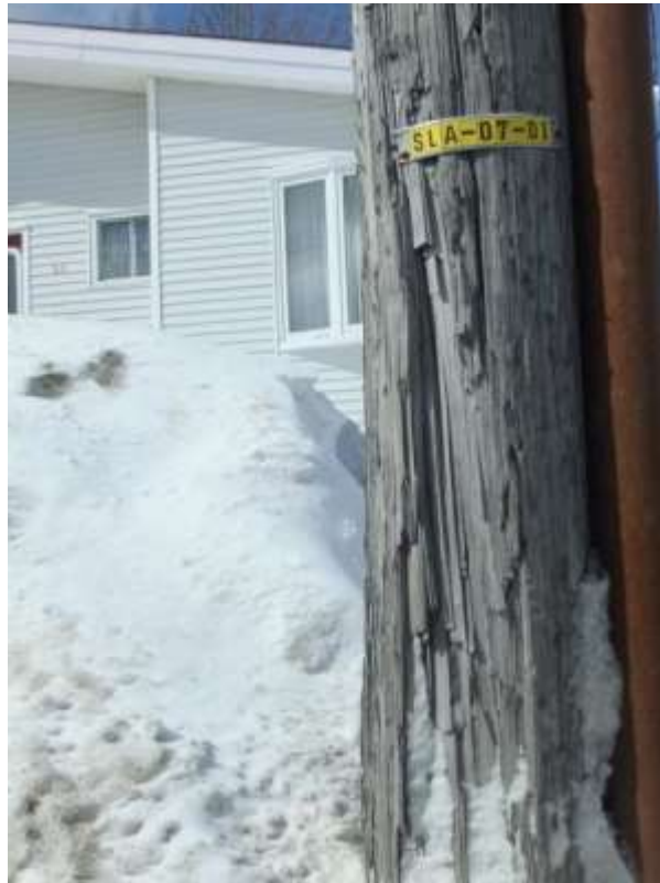
Figure 17 – Pole Damage
