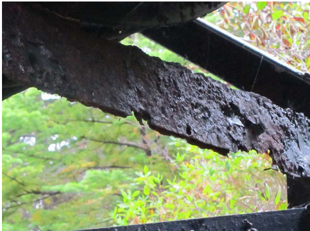
Photo No. 2.4.1.9 – Heavy Corrosion Forming Holes in Bottom Chord Member, Typical
