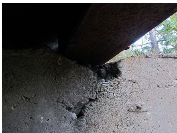
Photo No. 2.3.1.9 – Concrete Severely Deteriorated Under Beam
