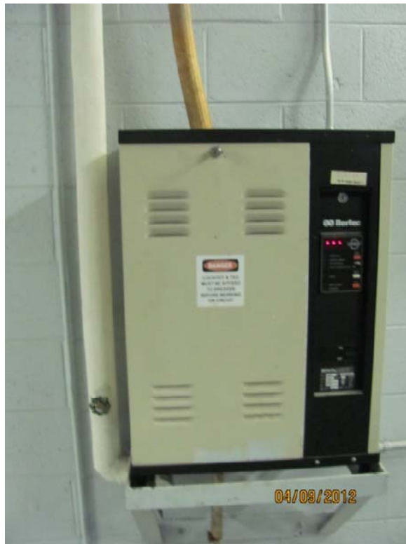
Existing First Floor Humidifier
