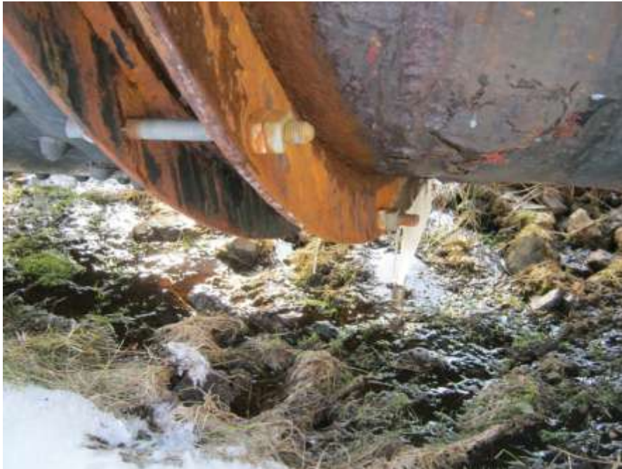
Photo C-9: Underside of penstock at mechanical expansion joint, showing minor leakage
