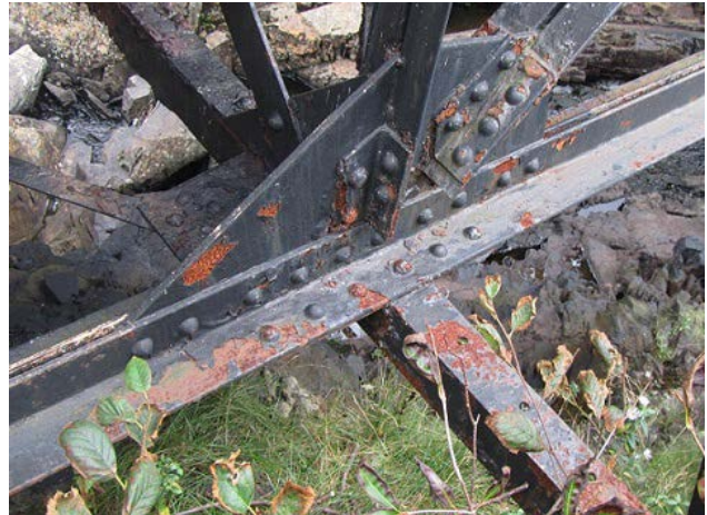
Photo No. 2.4.1.6 – Rust on South-Bottom Chord Connection, Typical
