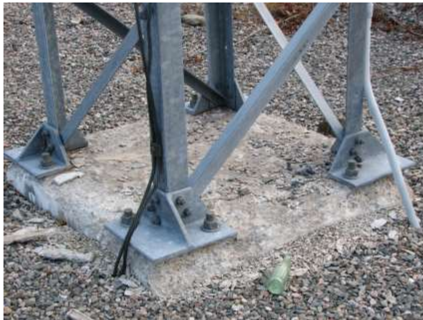
A 138 kV Pier Foundation that Requires Refurbishment
