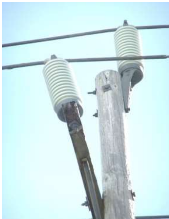
Figure 18 – Damaged Crossarm
