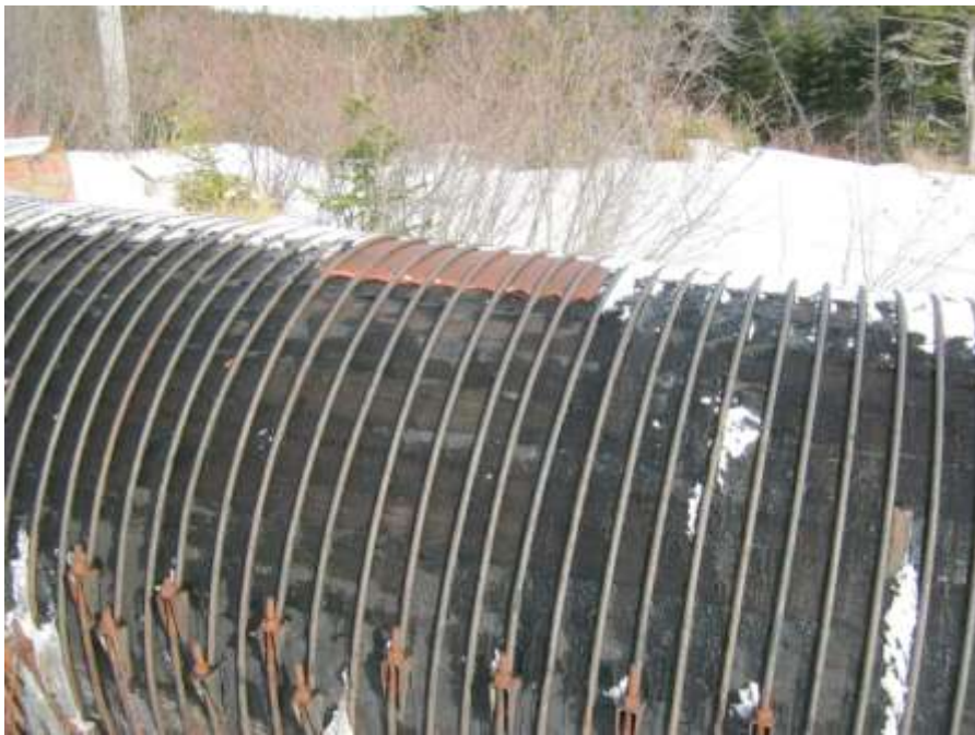
Photo C-21: Metal patch in top of penstock
