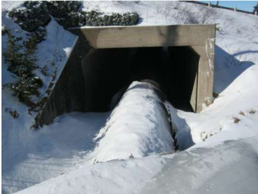
Photo C-42: Penstock at highway crossing
