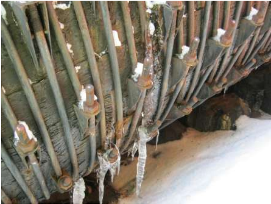
Photo C-20: Crushed staves, and broomed ends of staves
