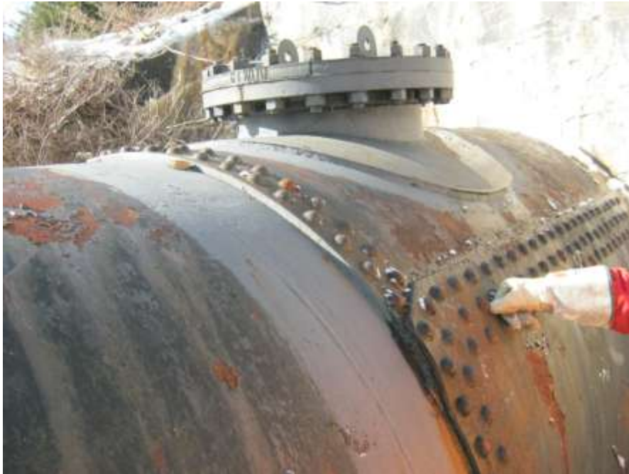
Photo C-7: Access hole near anchor block
