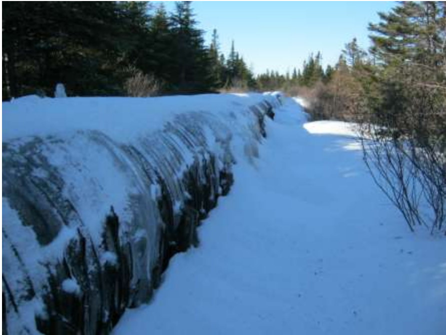
Photo C-52: Widespread leakage at springline
