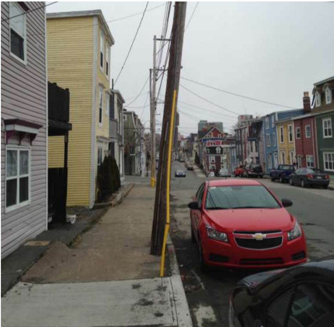
Figure 3 - Pole Leaning Towards Traffic
