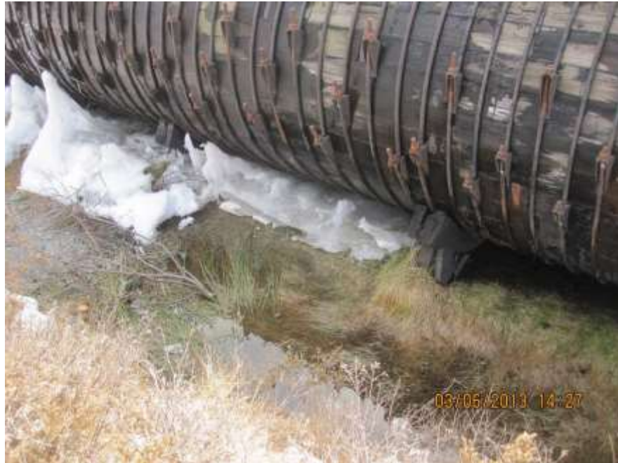
Figure 7: Deteriorated Cradle (Typical) and Saturated Penstock Bed
