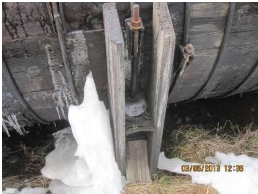
Figure 18: Deteriorated 190 Degree Cradle
