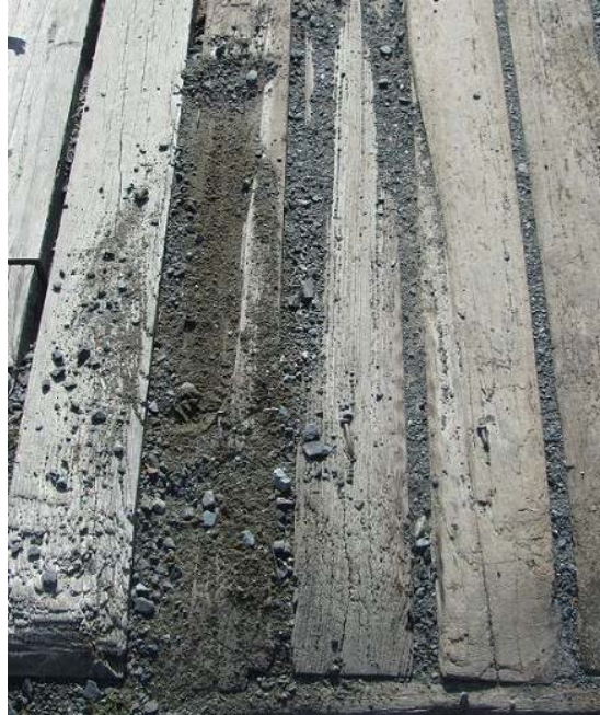
Photo No. 2.3.1.11 – Broken Timber Raceway Members
