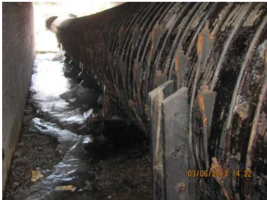
Figure 14: Transition from 190° to 120° Cradles
