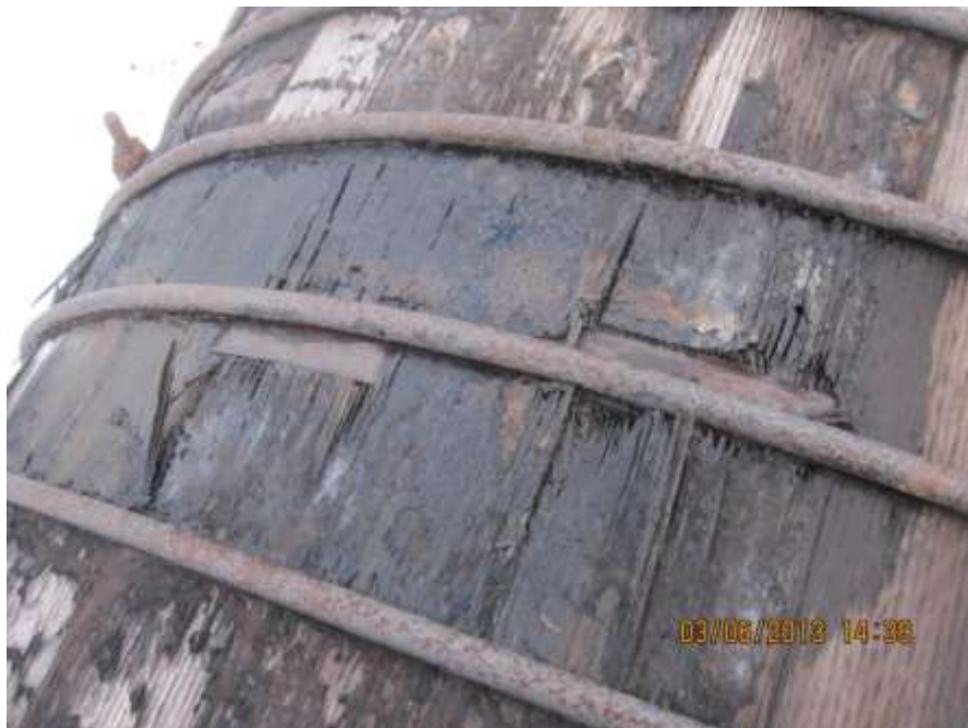
Photo C-49: Damaged ends of wood staves
