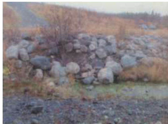
Figure 5 – Eroded Armour Stone
