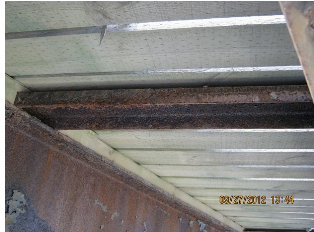
Photo No. 2.2.1.4 – Severe Rust and Scaling on Channels, Typical
