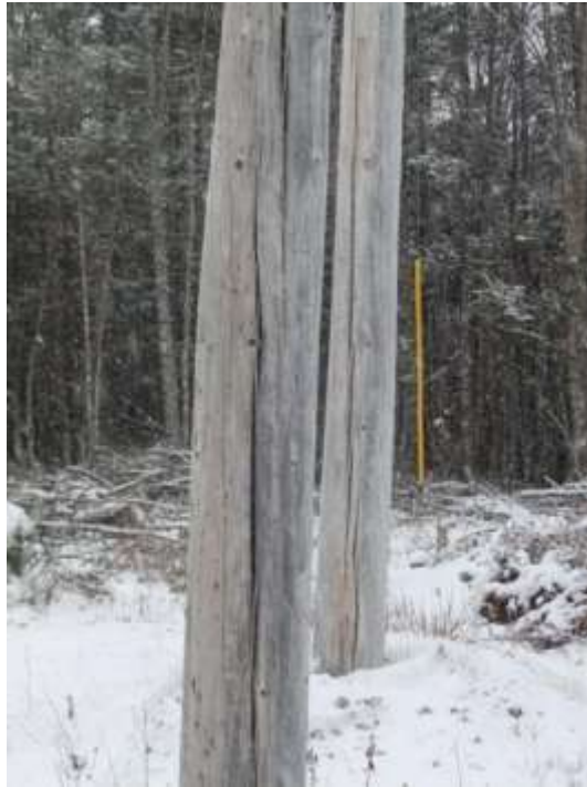
Figure 31 – Deep Pole Checking
