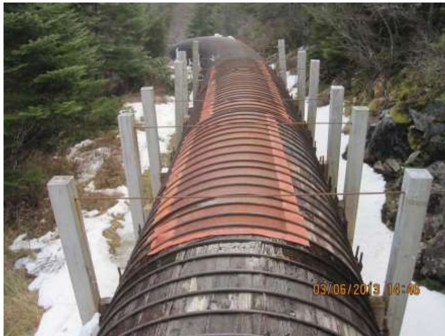
Figure 9: Repair and Stabilization of Past Blowout
