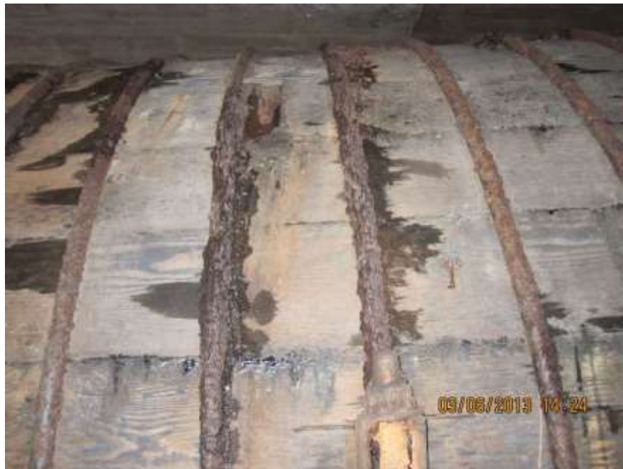
Figure 15: Severely Corroded Bands (near Route 10 crossing)
