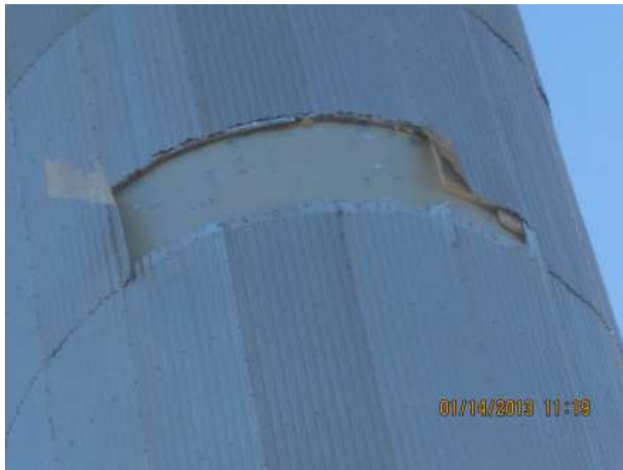
Figure 27: Frost Casing Failure – January 2013
