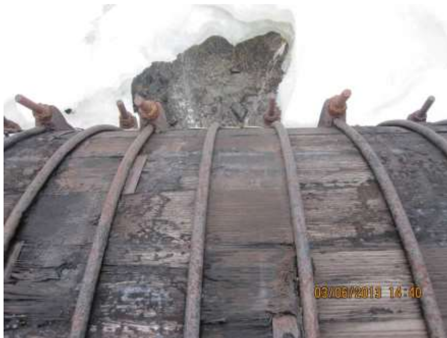
Figure 8: Corroded Bands and Nuts
