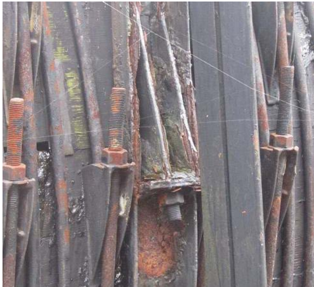
Photo No. 2.4.1.13 – Rust and Scaling on Penstock Support Band, Typical
