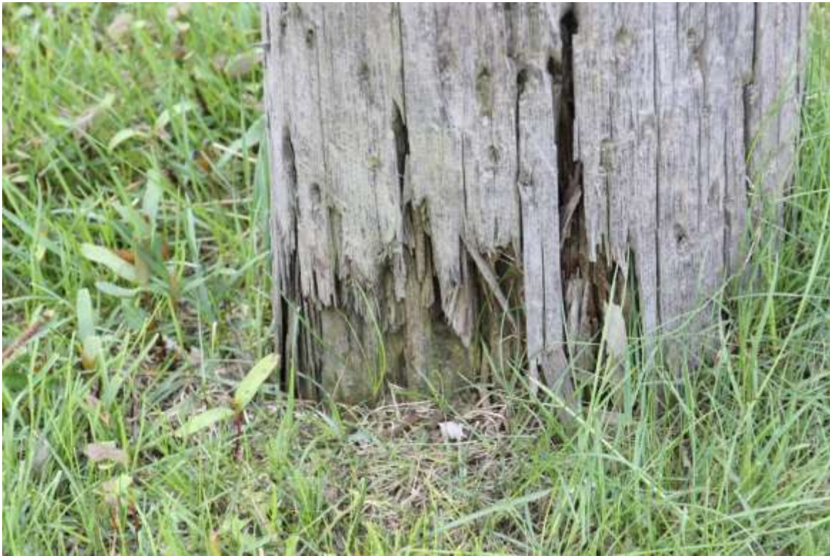
Figure 7 – Pole Deteriorated at ground line
