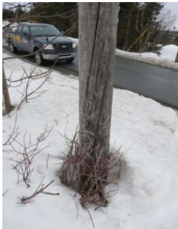
Figure 20 – Deteriorated Pole
