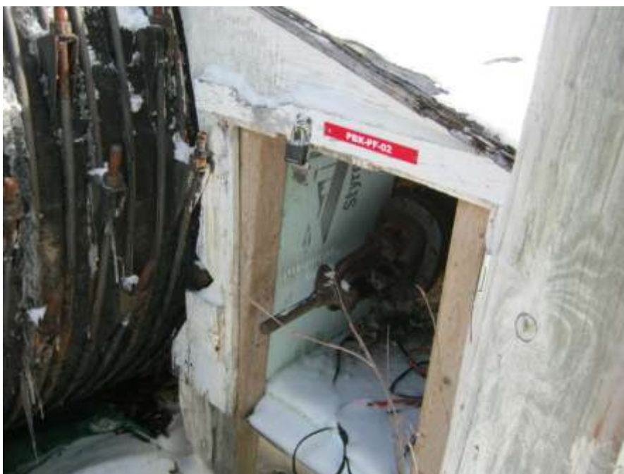
Photo C-25: Water supply line from side of penstock
