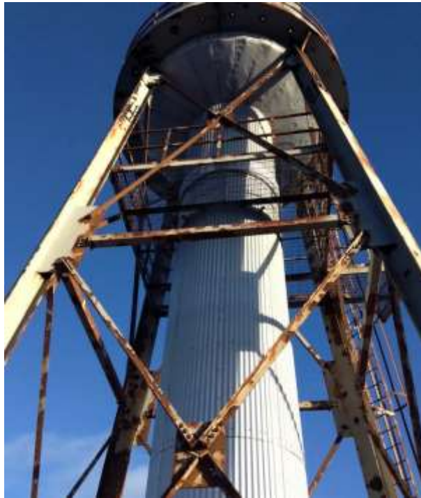
Figure 28: Deteriorated Coating – Surge Tank Support
