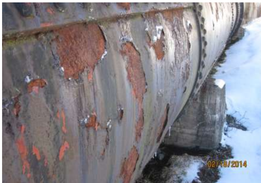
Figure 2: Coating Failure and Surface Cracks on Cradle
