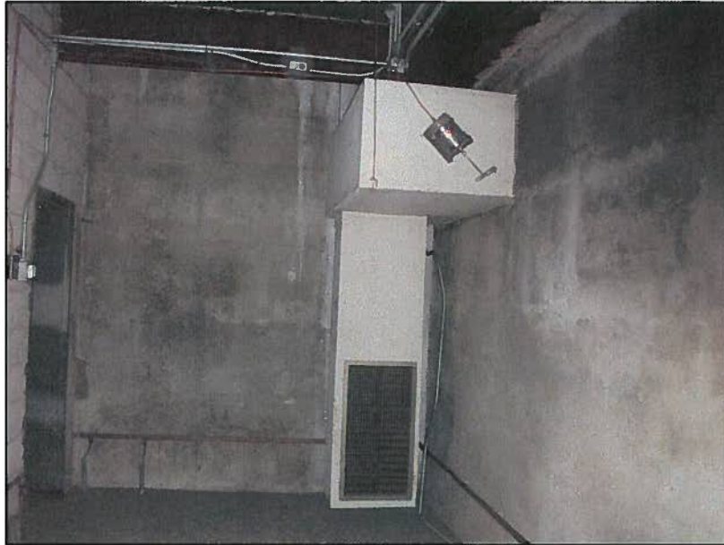
Picture 12: Fresh air intake. Note ceiling without fireproofing.
