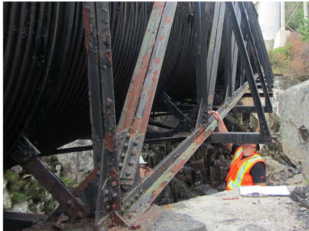
Photo No. 2.4.1.7 – Rust on North Chord Member, Typical
