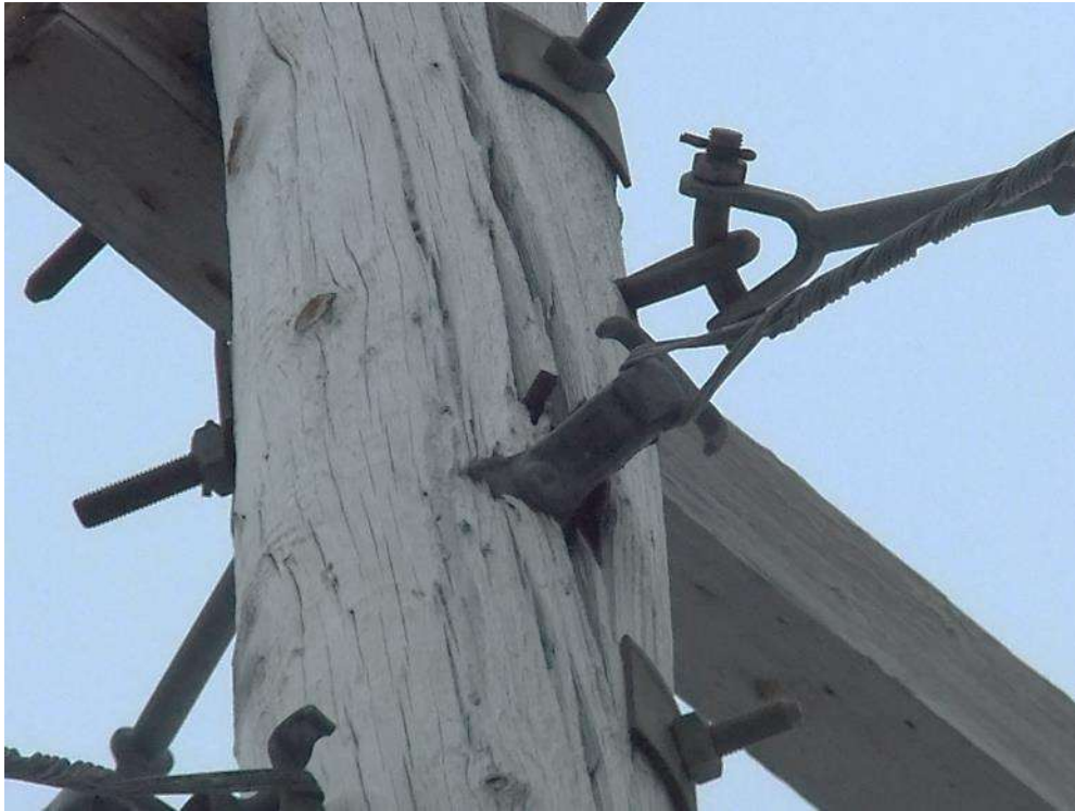
Figure 25 – Severe Pole Checking Due to Shell Separation
