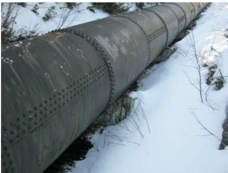
Photo C-4: General condition of steel penstock
