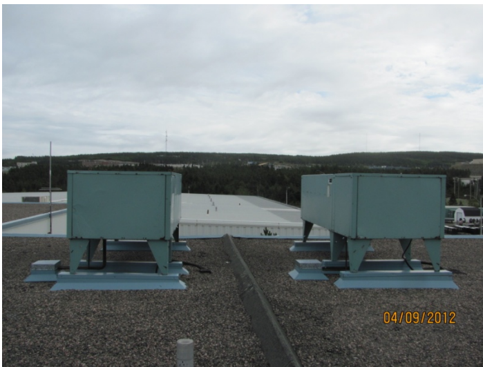
Existing AHU Unit Roof Mounted Condensing Unit
