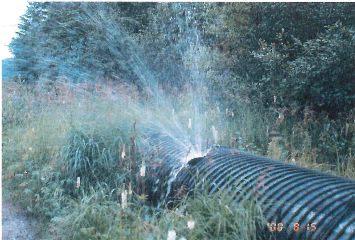
Photo 11: View of water leaking from penstock, August 2000.
