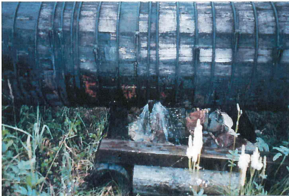
Photo #9: Water leaking from penstock, August 2000.
