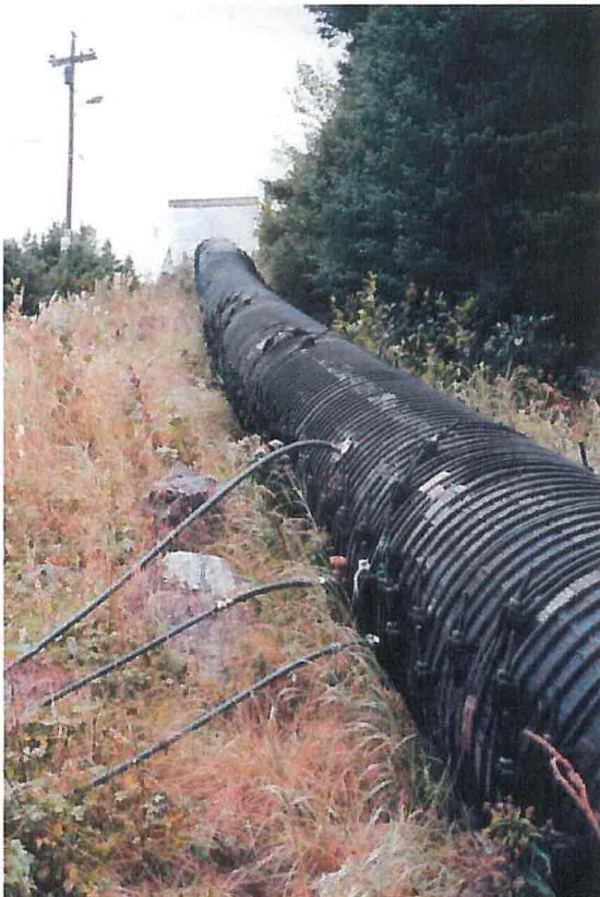
Photos #26 & #27: Water take-offs to adjacent homes (left) and Nugget Pond gold mine security building (right), August 2000.
