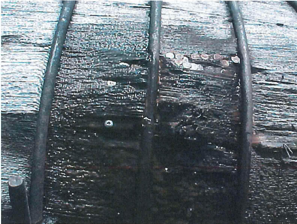
Photo #12: Nails driven into penstock to stop leaks, June 2001.
