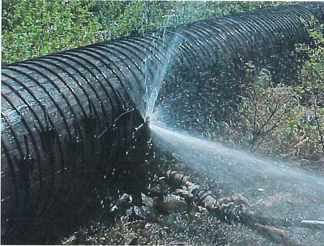
Photo #28: Location of abandoned water tap in penstock, June 2001.
