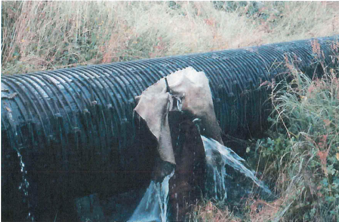
Photo #10: Water leaking from penstock, August 2000.
