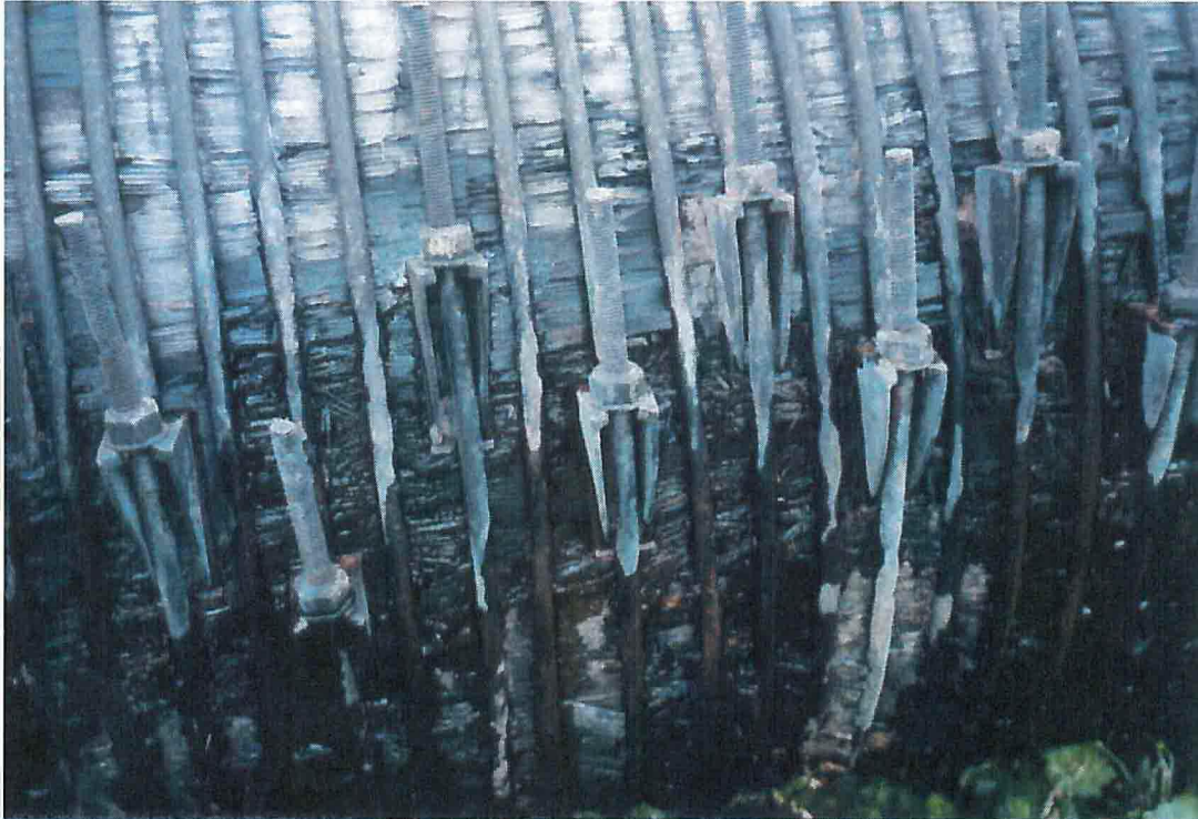
Photo #4: View of crushing and brooming of wooden staves, August 2000.
