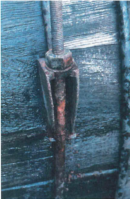
Photo #7: View of corrosion below threads, August 2000.
