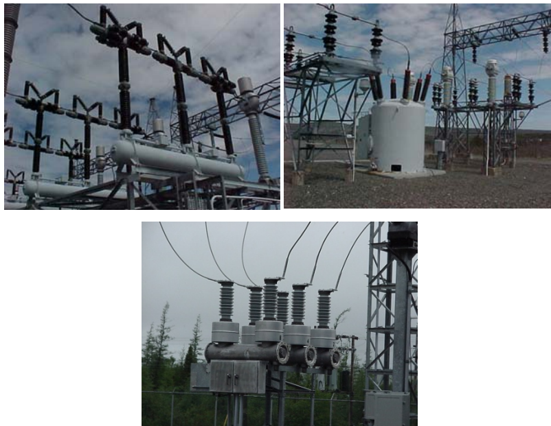
Figure 2: Circuit Breakers - Air Blast (top left), Oil (top right) and SF 6 (bottom)
