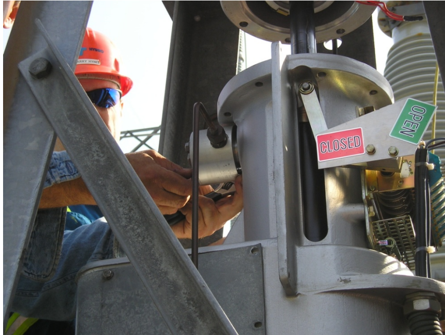
Figure 5: SF 6 Circuit Breaker during a Refurbishment
